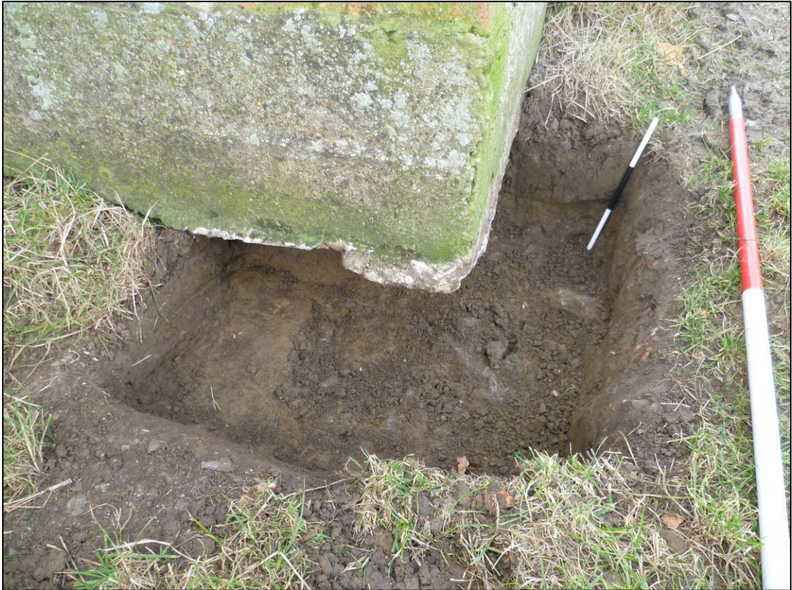
Plate 6: Completed excavation for new foundations under porch of Building R3, looking SW (photo 1/906).
