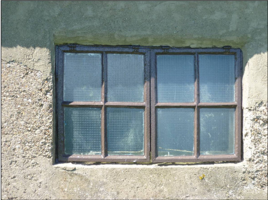
Plate 11: Repairs complete to window W1 in Building R4, looking NW (photo 2/683).
