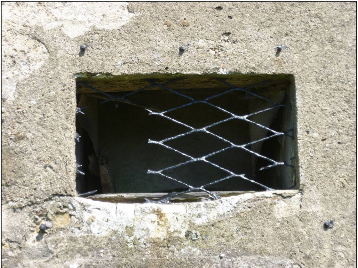
Plate 4: Repairs to vent grill on W side of Building R2, looking NE (photo 2/666).
