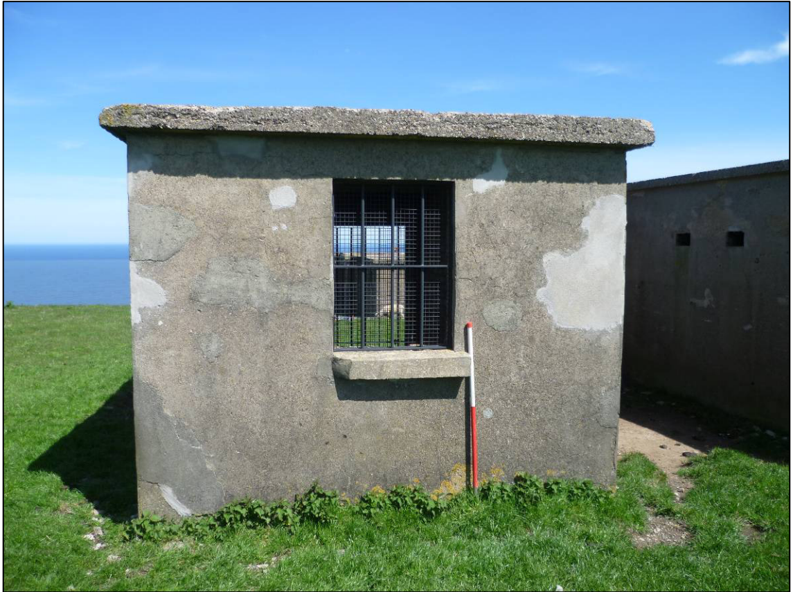
Plate 1: Repairs to render and inserted window screen, W side of Building R1, looking NE (photo 2/658).
