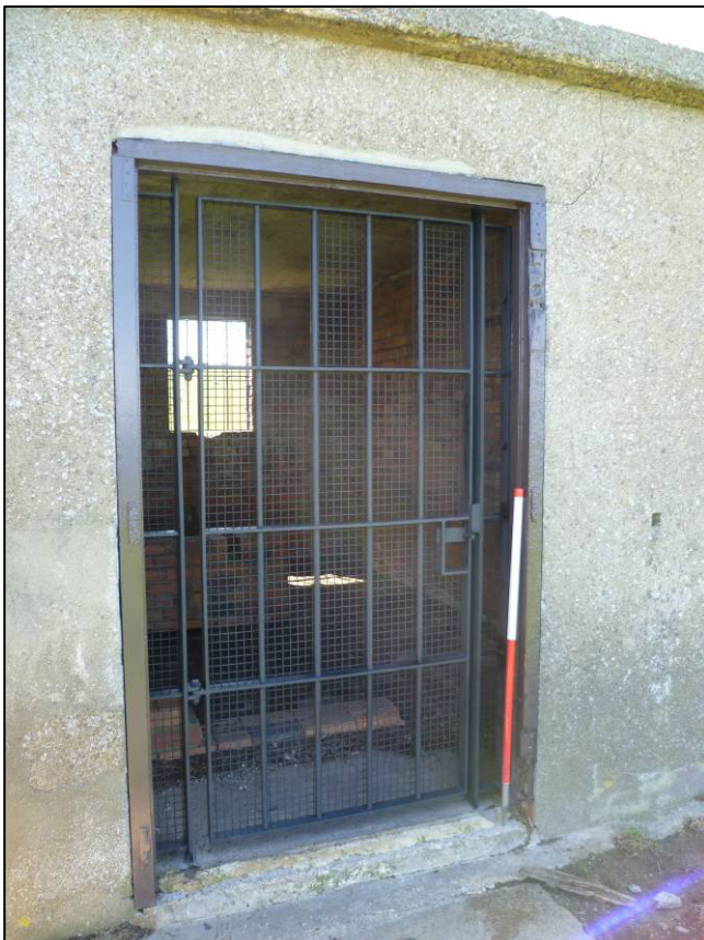
Plate 2: Inserted door screen to Building R1, looking SW (photo 2/655).
