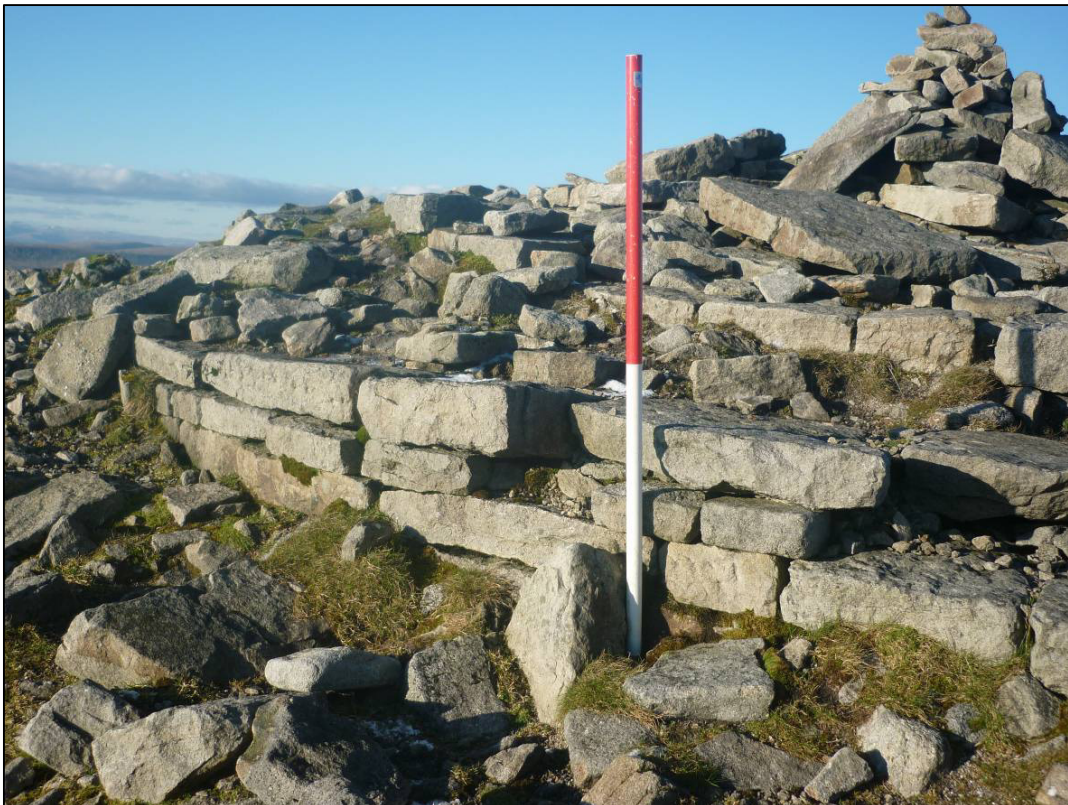
Plate 42: Hospice Tower (5), typical coursing to base of tower, looking N (photo 3/659).
