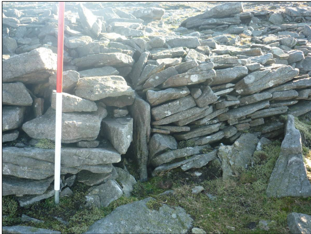
Plate 36: Perimeter Section 4 (4/5), 'Farrer through' in external revetment wall, looking SW (photo 1/395).
