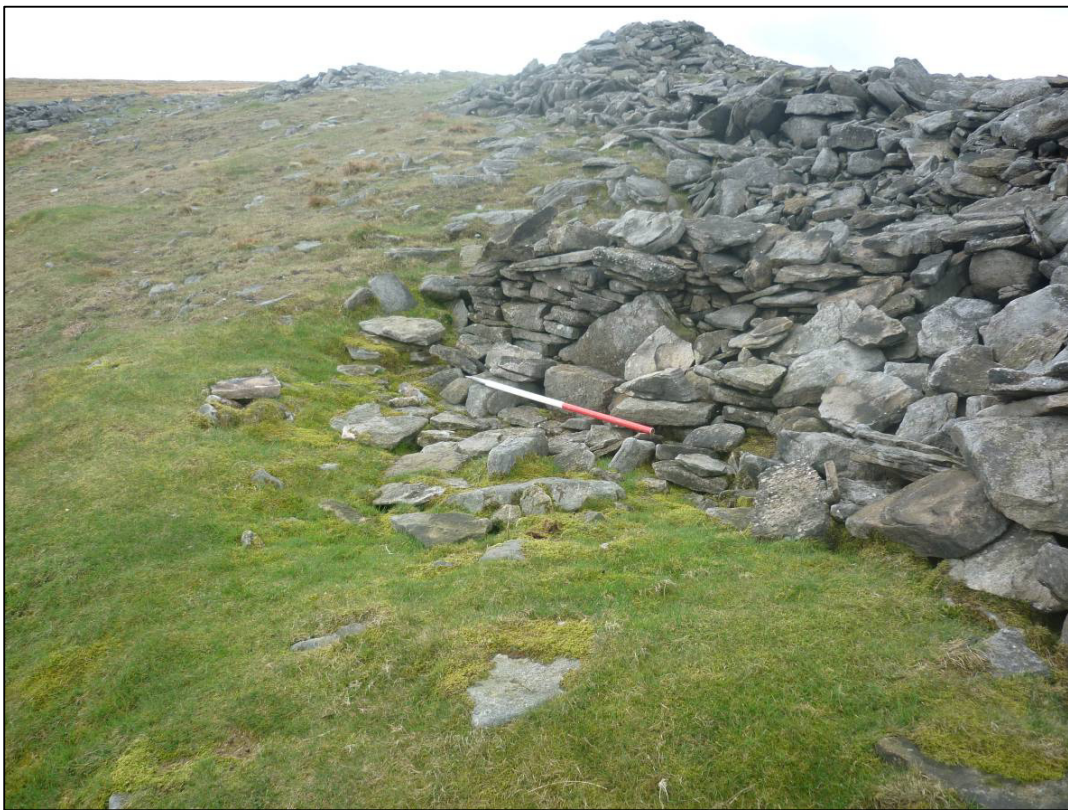
Plate 12: Perimeter Section 1 (1/15), modern shelter, looking SW (photo 6/769).
