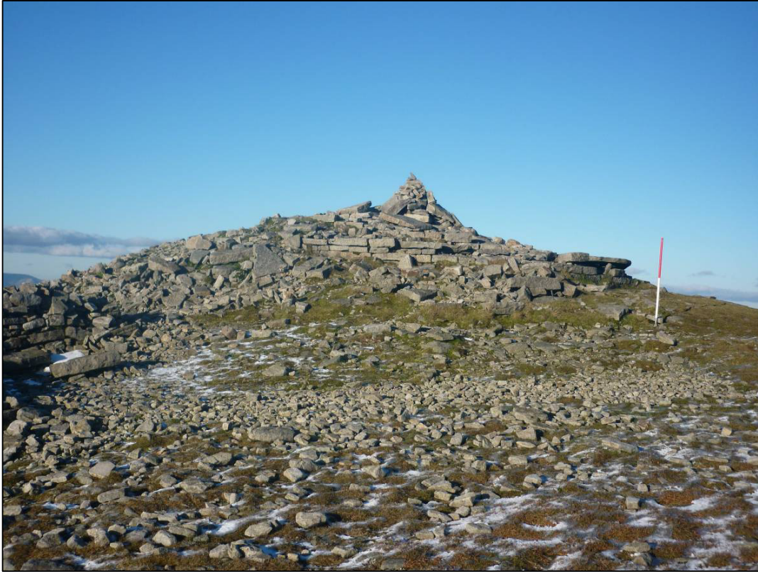
Plate 41: Hospice Tower (5), looking W (photo 3/657).
