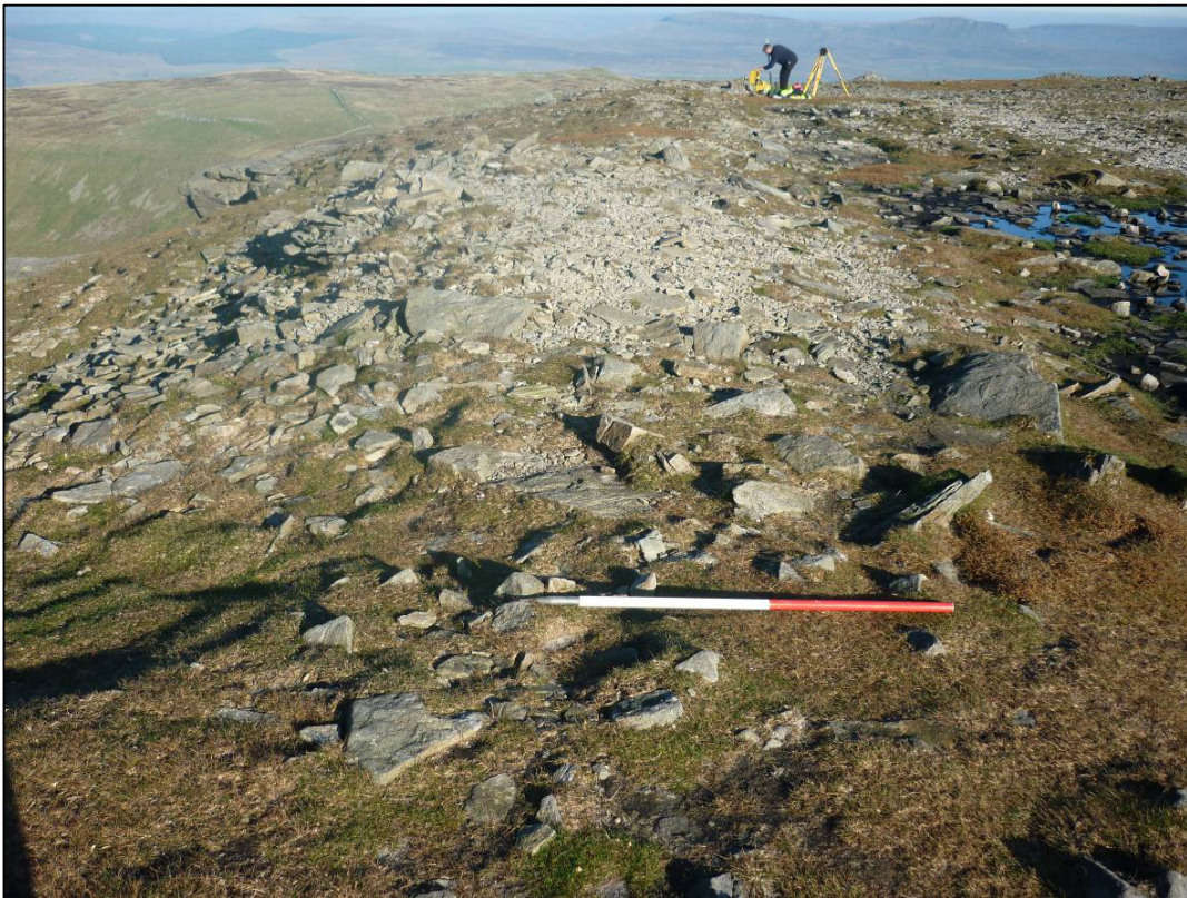
Plate 38: Perimeter Section 4 (4/10 - west end), showing small and large rubble construction, looking E (photo 1/388).
