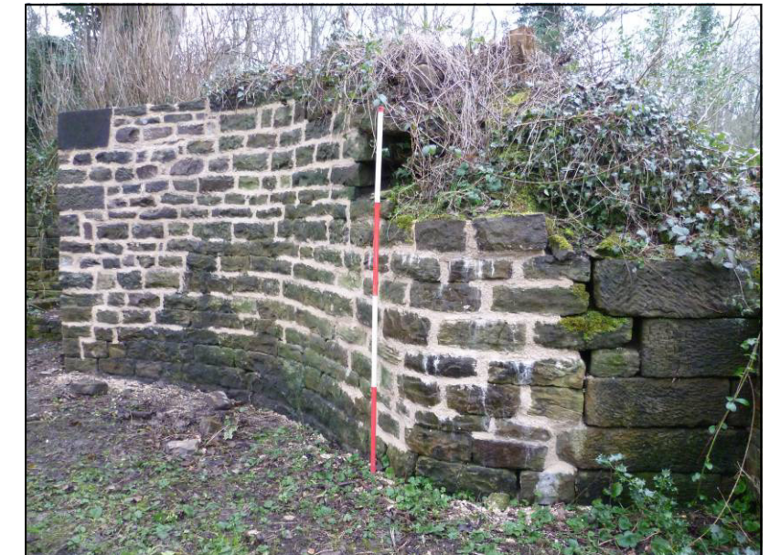
Plate 15: Area 2 dam wall, two months after completion, looking S (photo 4/680).
