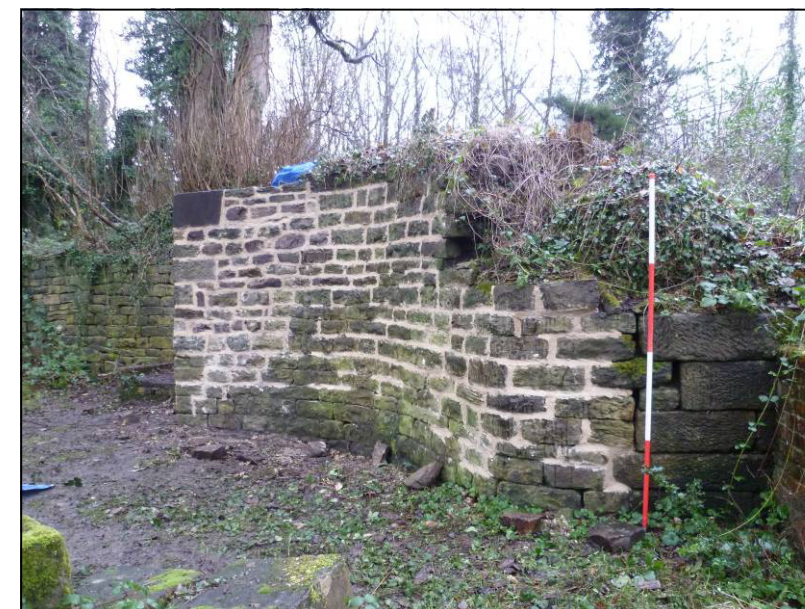
Plate 14: Area 2 dam wall immediately after repointing, looking S (photo 3/505).
