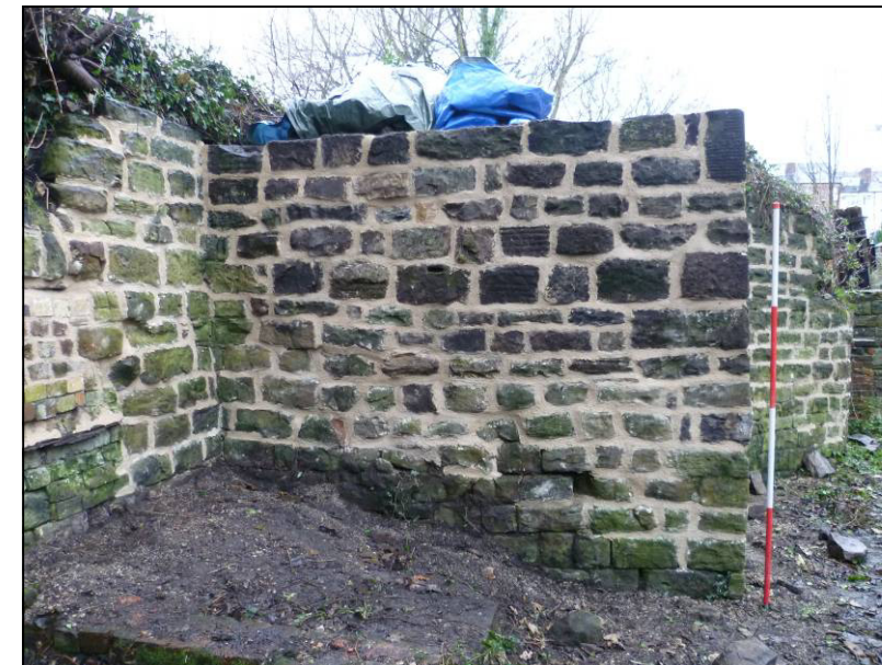
Plate 13: Area 2 dam wall immediately after repointing, looking W (photo 3/504).
