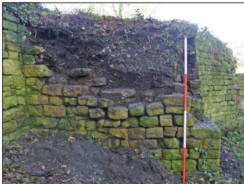
Plate 11: Area 2 dam wall with clearance complete, looking W (photo 2/422).
