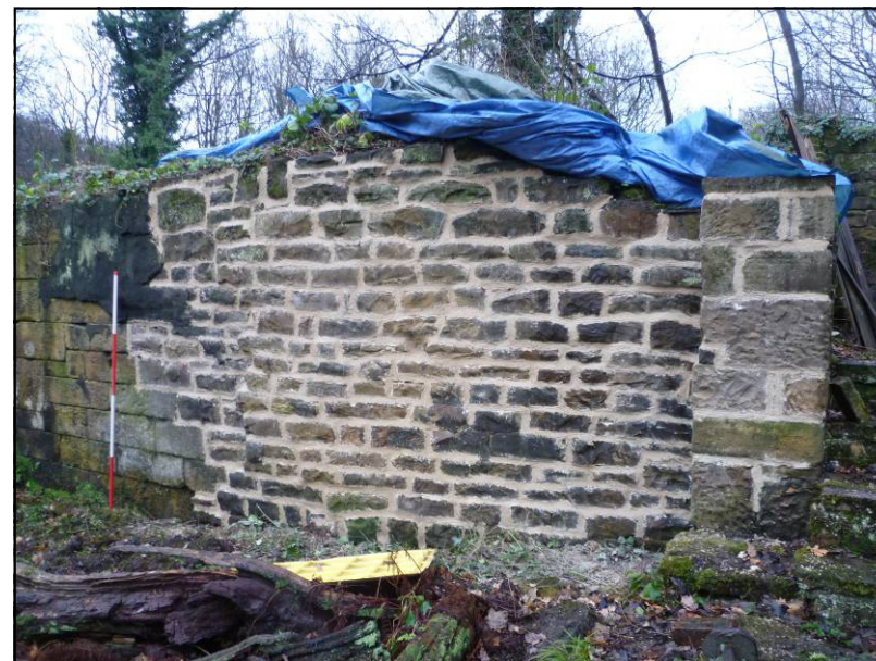
Plate 7: Area 1 dam wall immediately after repointing, looking SE (photo 3/508).
