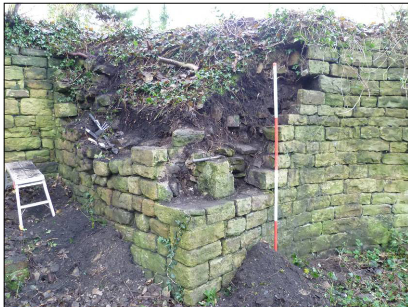
Plate 10: Area 2 dam wall during clearance, looking SW (photo 2/416).
