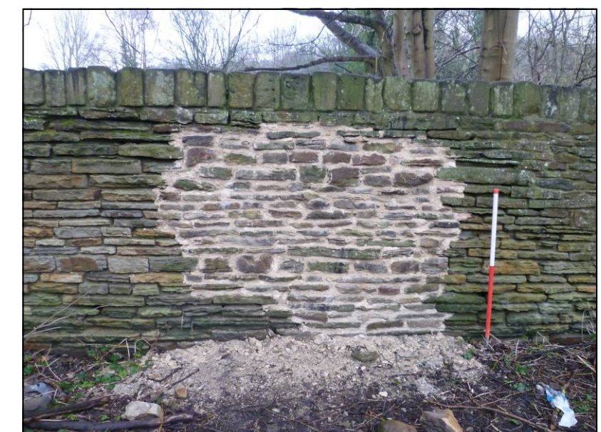
Plate 28: Area 4 boundary wall (external), two months after completion, looking E (photo 4/692).
