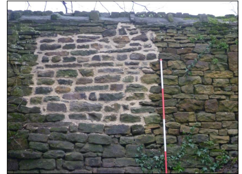
Plate 27: Area 4 boundary wall (internal), two months after completion, looking W (photo 4/686).
