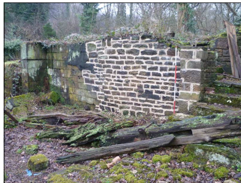
Plate 8: Area 1 dam wall two months after completion, looking SE (photo 4/685).
