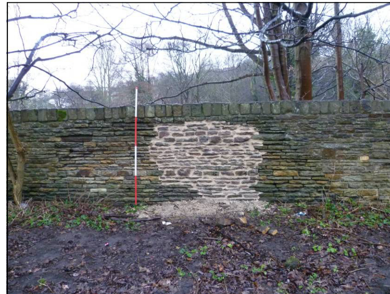
Plate 26: Area 4 boundary wall (external) immediately after repointing, looking E (photo 3/511).
