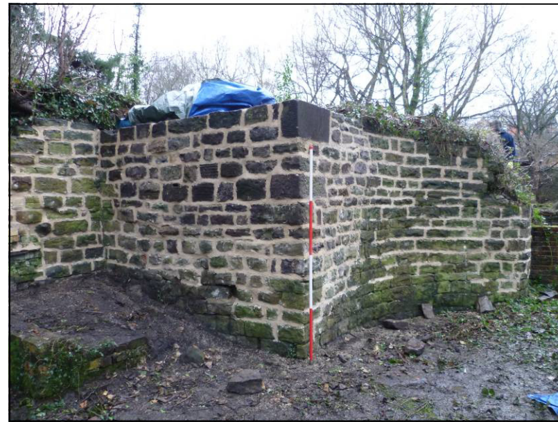
Plate 12: Area 2 dam wall immediately after repointing, looking SW (photo 3/499).
