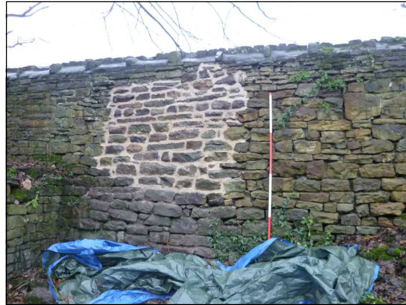
Plate 25: Area 4 boundary wall (internal) immediately after repointing, looking W (photo 3/496).
