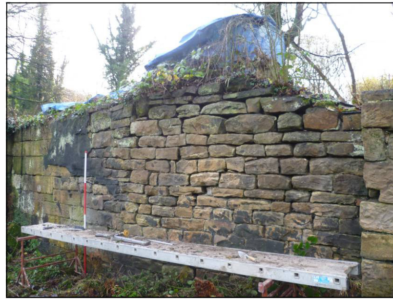
Plate 4: Area 1 dam wall, work in progress, looking SE (photo 2/412).
