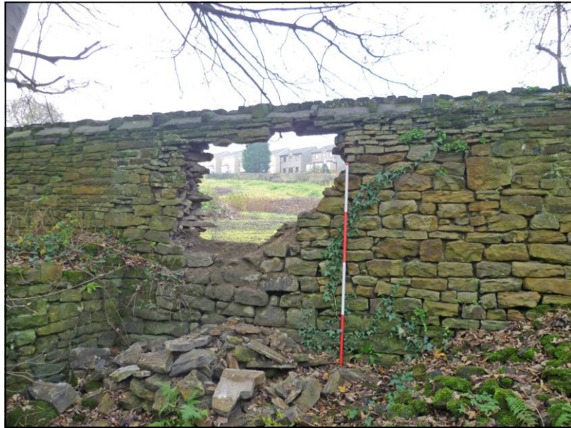
Plate 23: Area 4 boundary wall (internal) prior to repair, looking W (photo 1/363).
