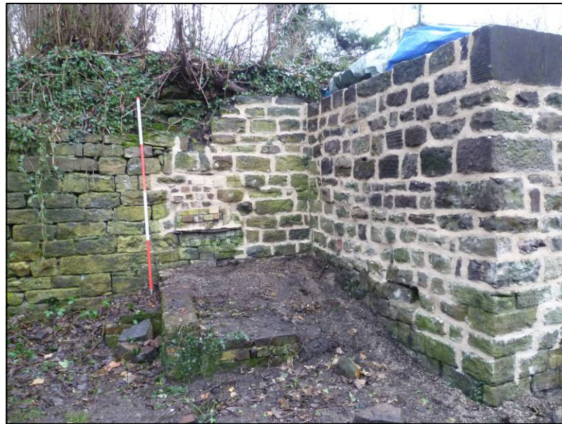
Plate 19: Area 3 dam wall immediately after repointing, looking SW (photo 3/502).
