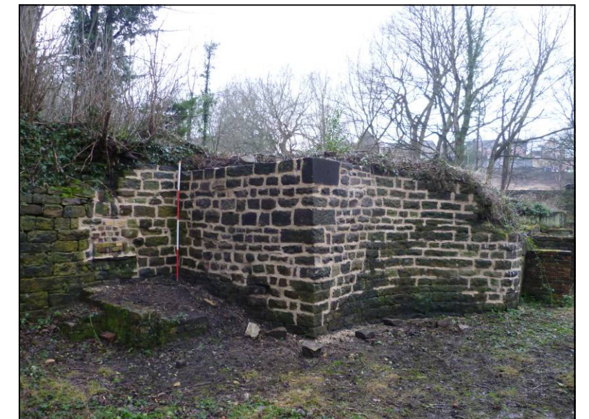
Plate 16: Area 2 dam wall, two months after completion, looking SW (photo 4/673).
