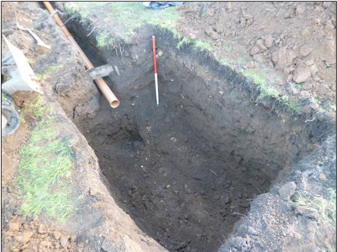
Plate 2: Soakaway pit after excavation, looking S.
