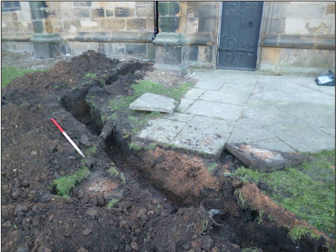
Plate 1: Excavation of Trench 1 in progress, looking S.
