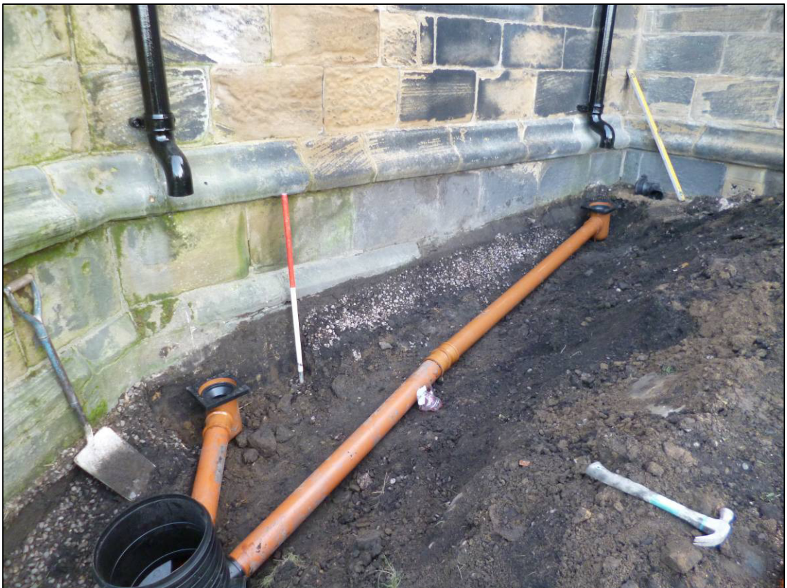
Plate 4: Trench 2 after excavation, looking SE.
