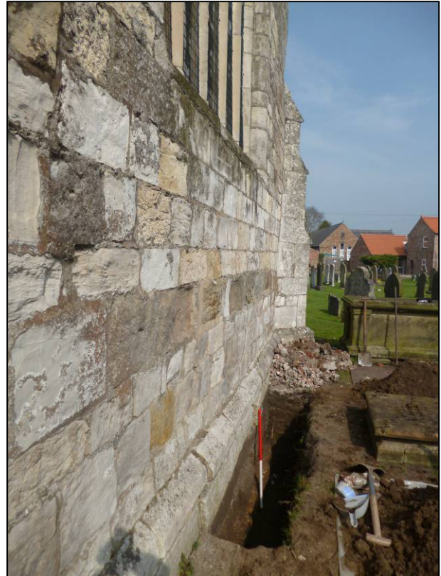
Plate 2: Trench after excavation, looking N.
