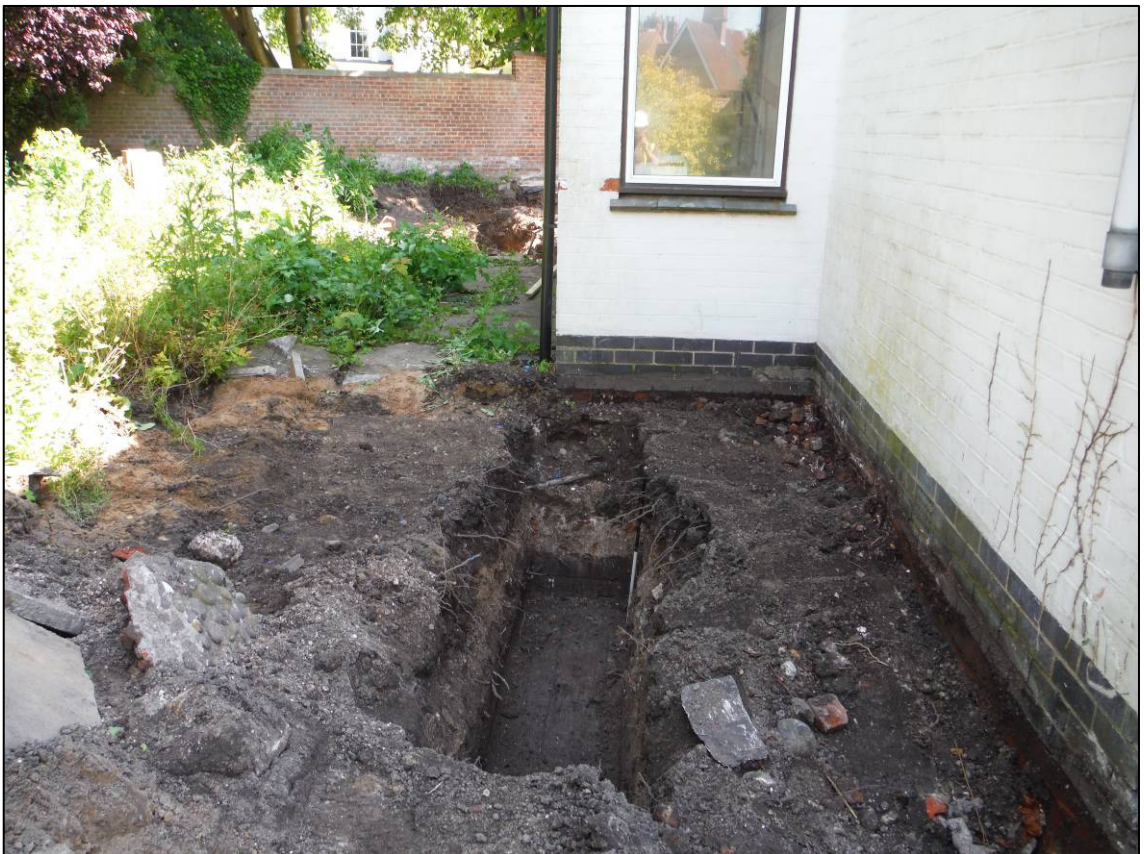
Plate 4: General view of Trench 2 for northern extension, looking E.
