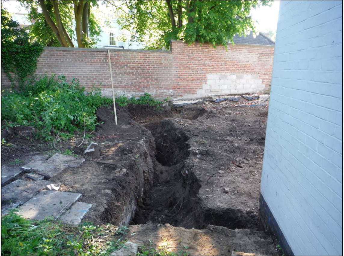
Plate 1: General view of Trench 1 for eastern extension, looking E.
