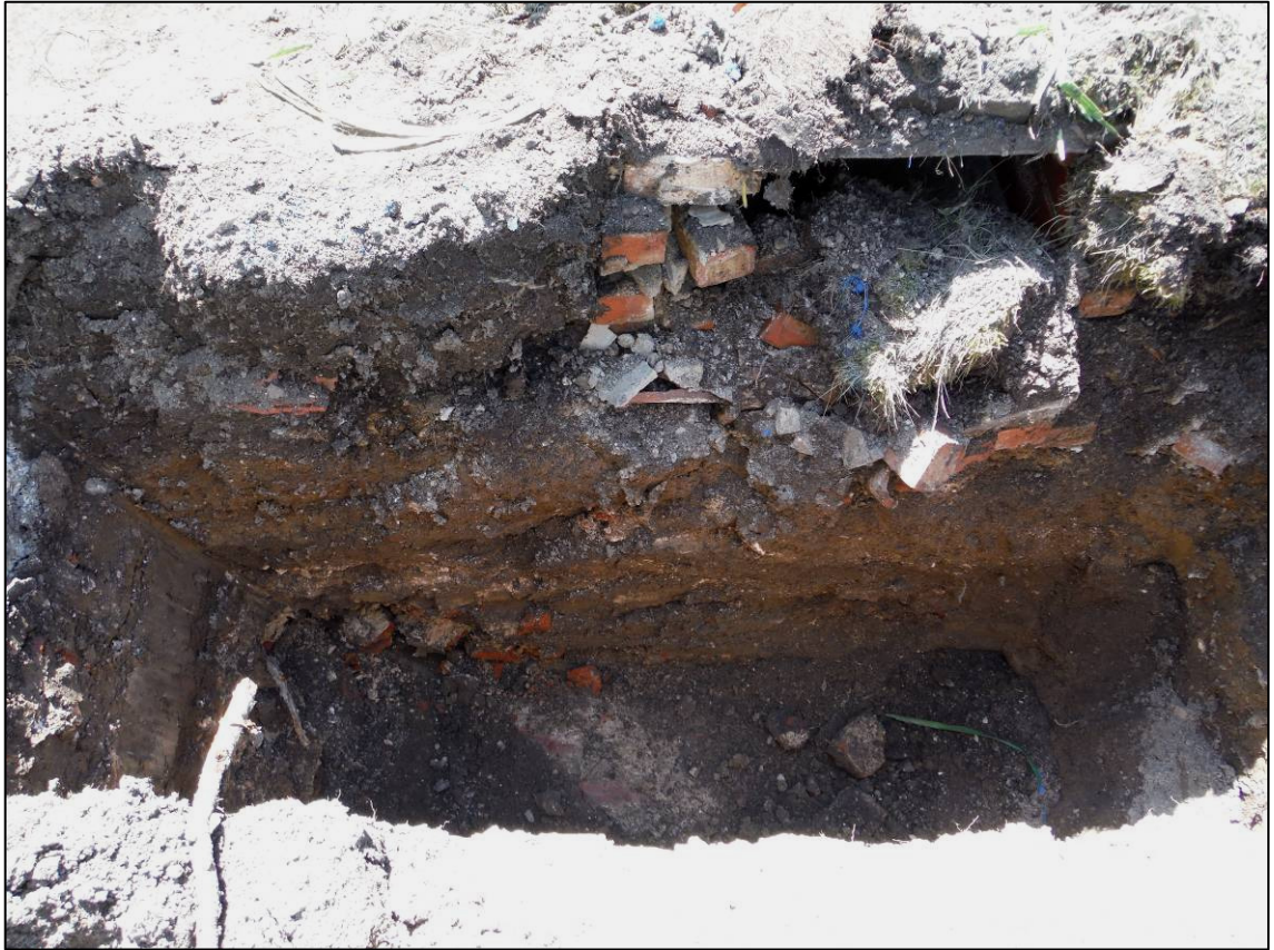
Plate 5: West side of culvert (304) in base of Trench 3 (western extension), with modern manhole above, looking N.
