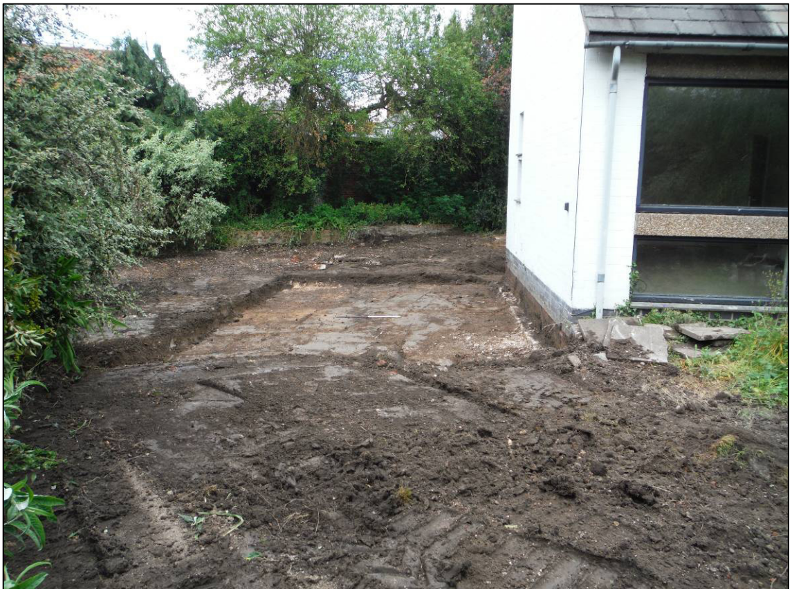
Plate 6: General view of stripped area for western extension, looking N.
