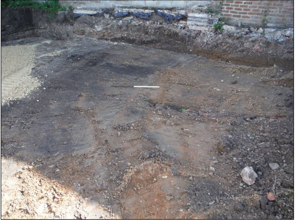
Plate 3: General view of stripped area for eastern extension, looking NE.
