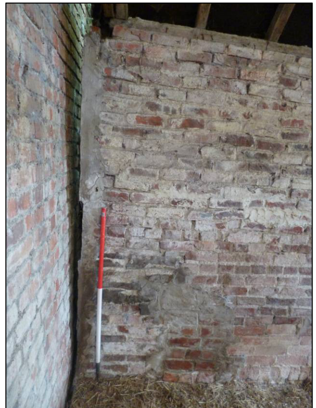
Plate 9: 'To-be-demolished' building, south end of west wall, looking W (photo 1/611).
