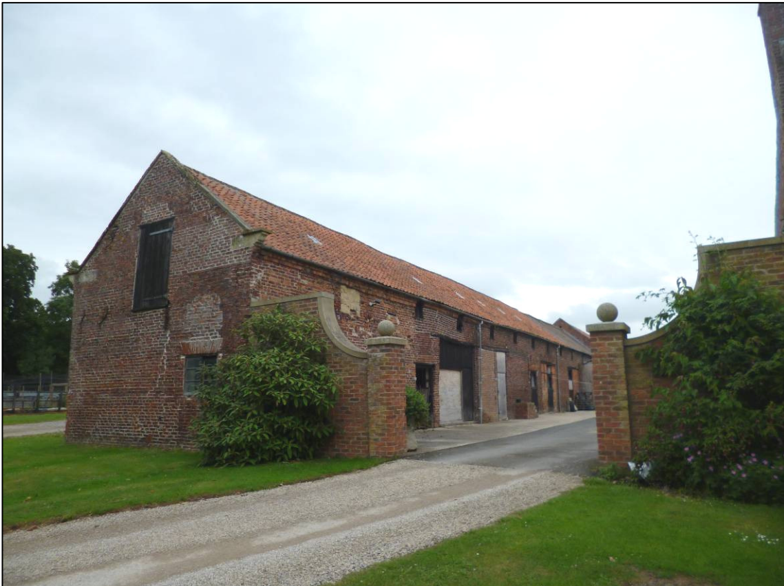
Plate 2: West end of north range and inserted recent gateway, looking NE.
