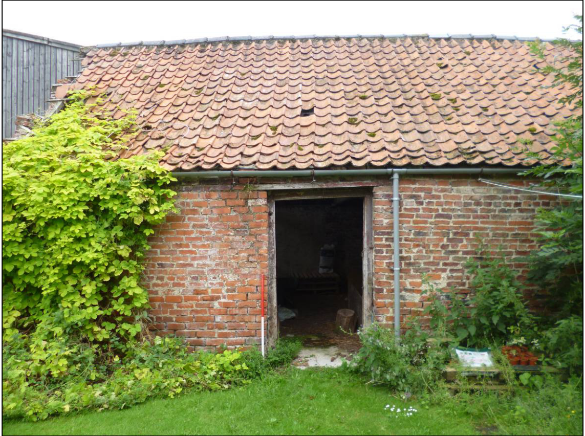
Plate 10: 'To-be-demolished' building, west elevation, looking E (photo 1/578).
