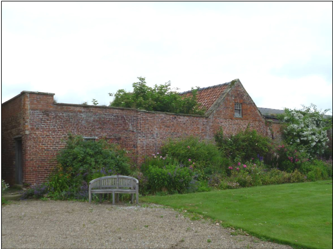
Plate 5: Garden wall running east from house, with south gable of 'to-be-demolished' building built over, looking NE (photo 1/520).
