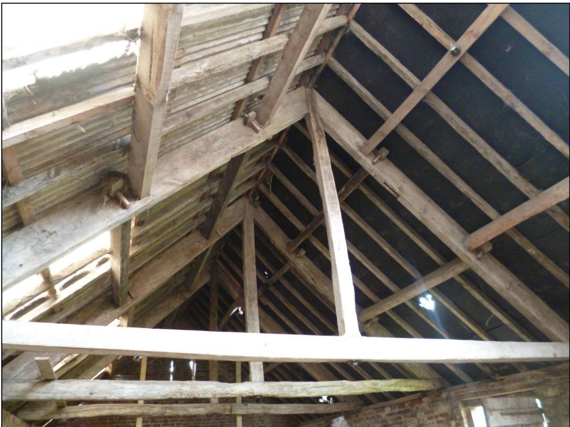
Plate 15: 'To-be-demolished' building, roof trusses, looking S (photo 1/624).
