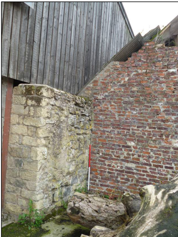
Plate 8: 'To-be-demolished' building, east side of north gable, looking SE (photo 1/573).
