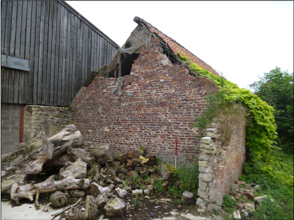
Plate 7: 'To-be-demolished' building, north gable, looking S (photo 1/570).
