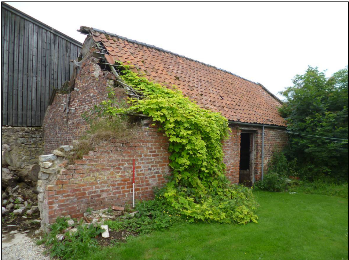
Plate 6: 'To-be-demolished' building, looking SE (photo 1/575).
