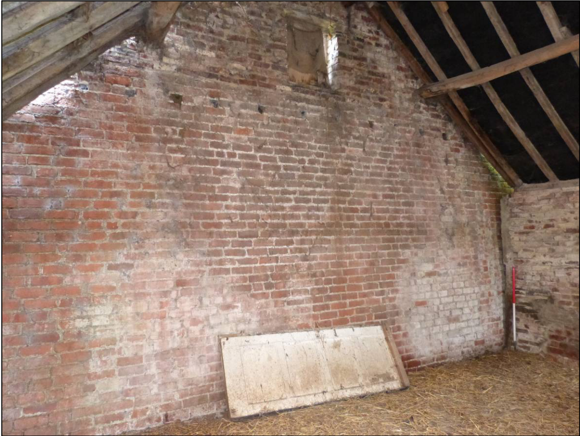
Plate 14: 'To-be-demolished' building, south wall, looking S (photo 2/090).
