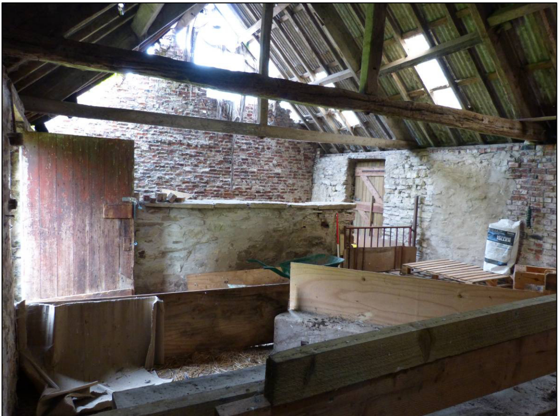
Plate 13: 'To-be-demolished' building, general view of interior, looking NE (photo 1/524).
