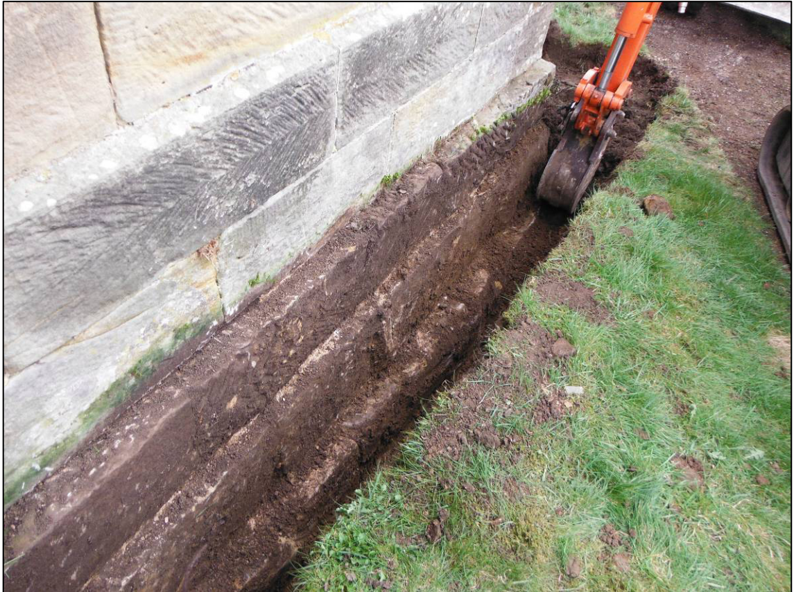
Plate 3: Trench 2 under excavation, showed stepped footings (205) of west wall, looking SE.
