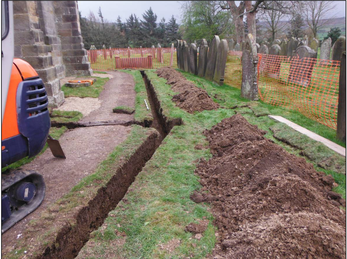
Plate 5: Trench 3 under excavation, looking S.
