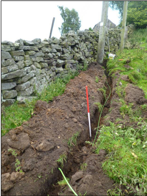
Plate 1: South end of trench after excavation, looking S.
