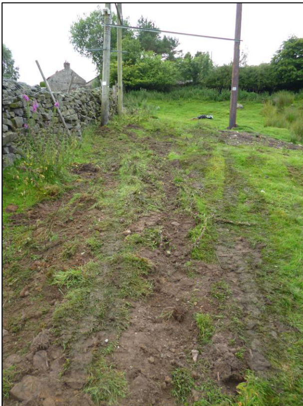
Plate 3: South end of trench after reinstatement, looking S.
