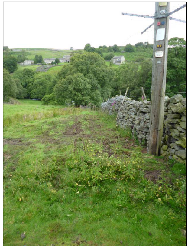
Plate 4: North end of trench after reinstatement, looking N.
