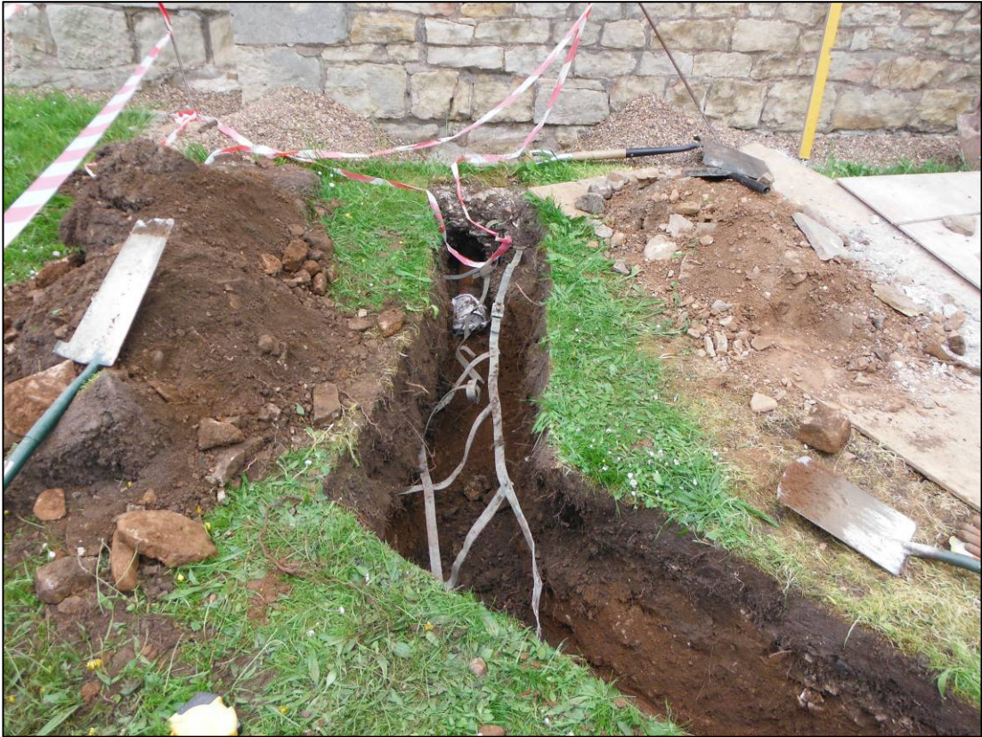
Plate 5: Trench 2 under excavation, showing metal-earthing straps, looking E.
