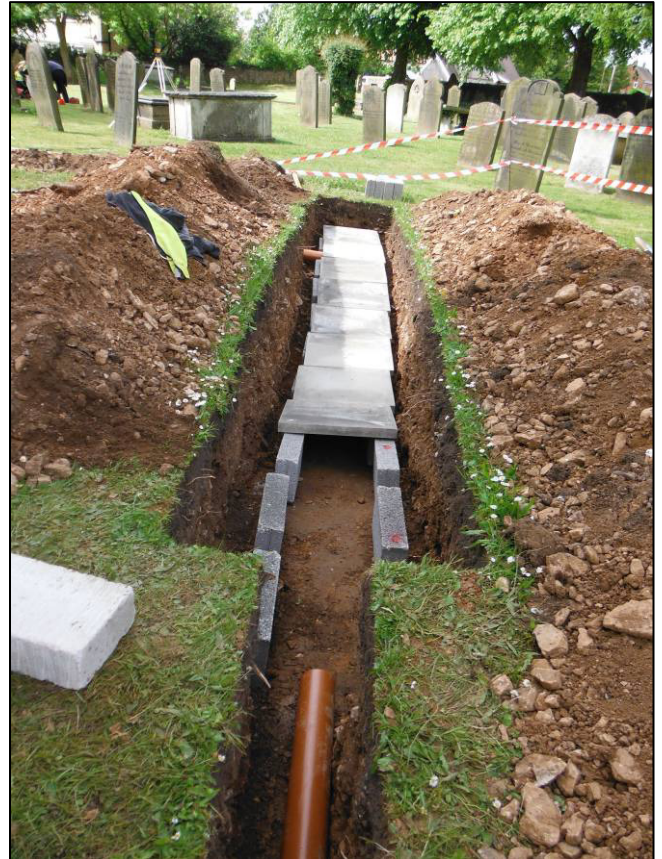
Plate 8: Construction of Trench Arch drain in Trench 1, looking SW.
