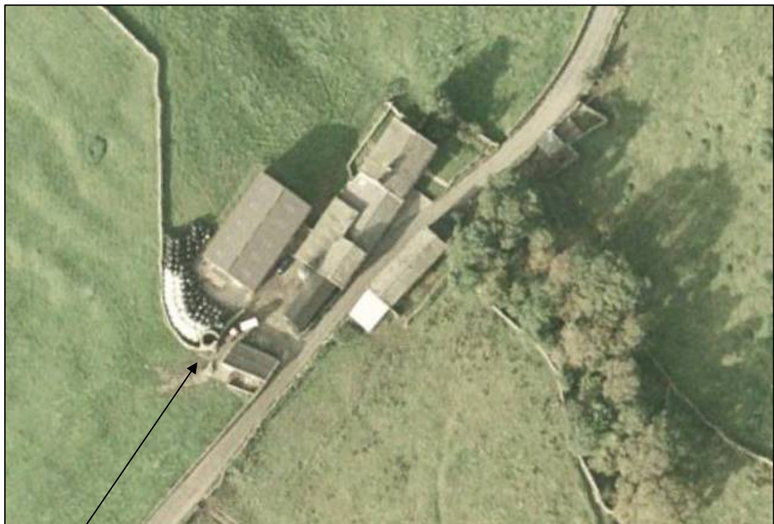
West Shaw circular silage silo (Source: Google Earth).
