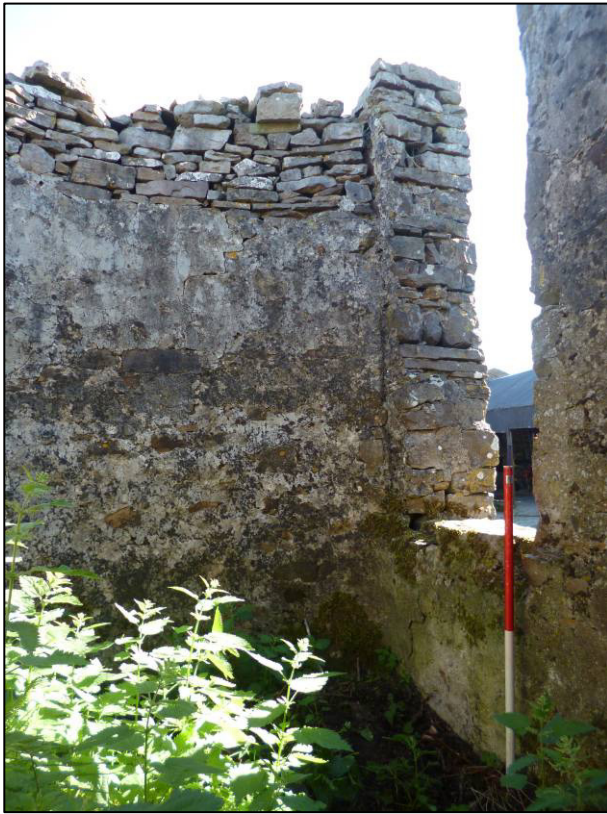
Plate 4: Interior of silo, looking N (photo 1/388).
