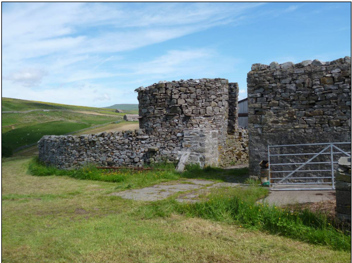
Plate 5: General view of silage silo, looking NW (photo 1/414).
