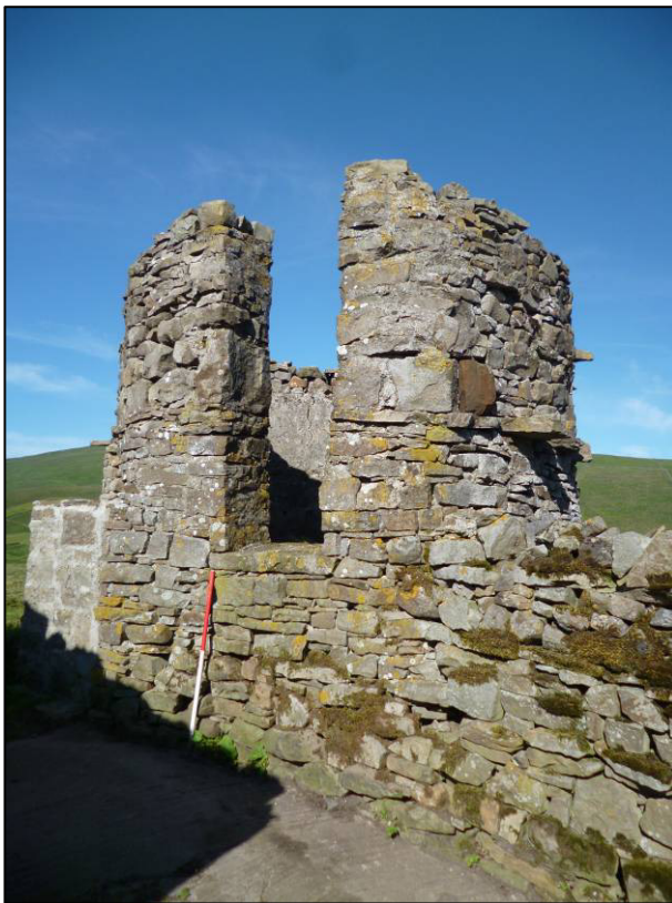
Plate 2: East side of silo, looking SW (photo 1/359).
