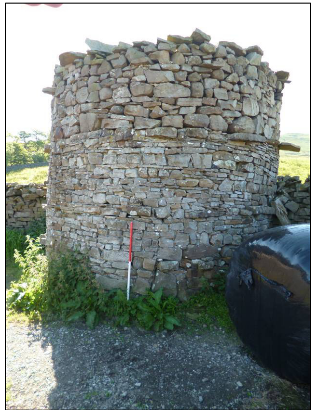
Plate 3: West side of silo, looking E (photo 1/380).
