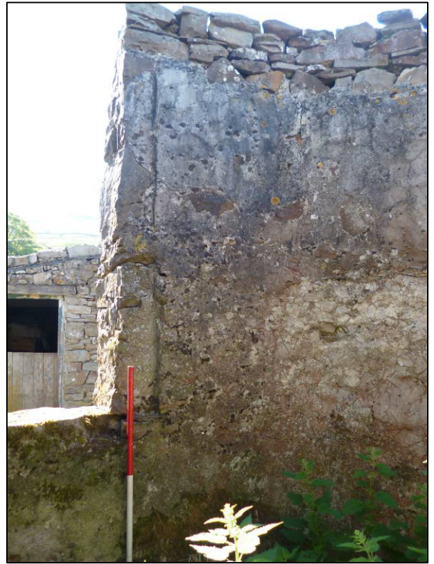
Plate 5: Interior of silo, looking E (photo 1/386).
