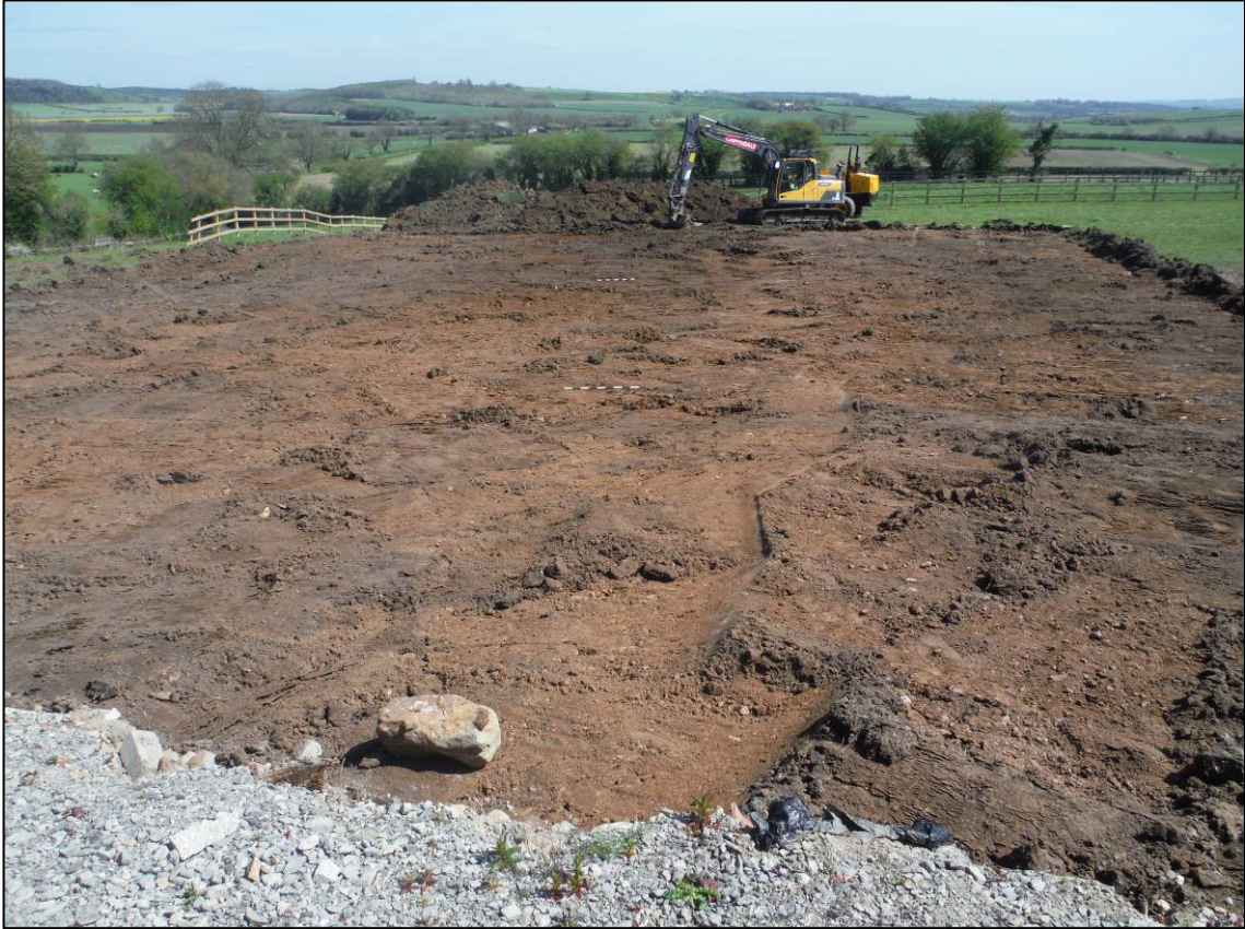
Plate 1: General view of topsoil strip in progress, looking E.
