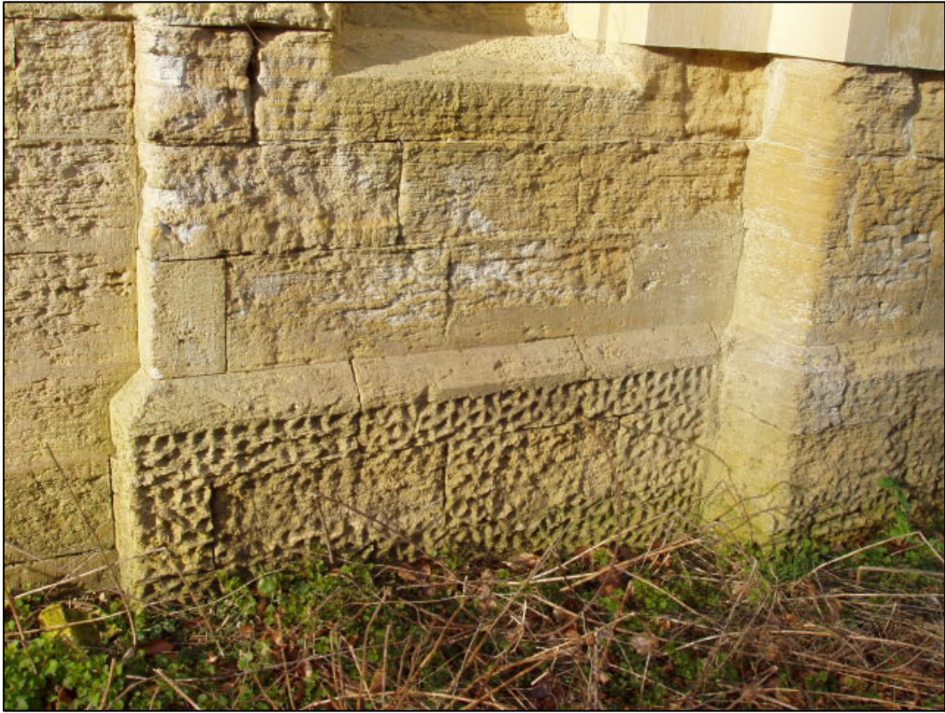
Plate 9: Vermiculated plinth on south elevation of central cell, looking N (Peter Pace photograph).
