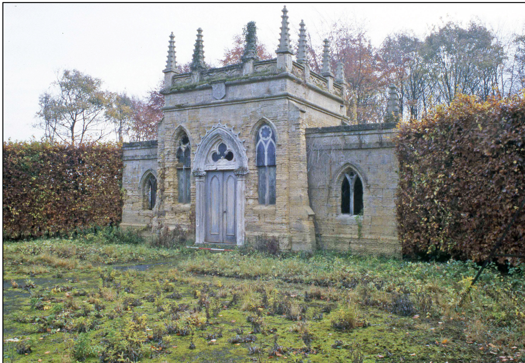
Plate 2: North elevation, looking E (photo 4/09).
