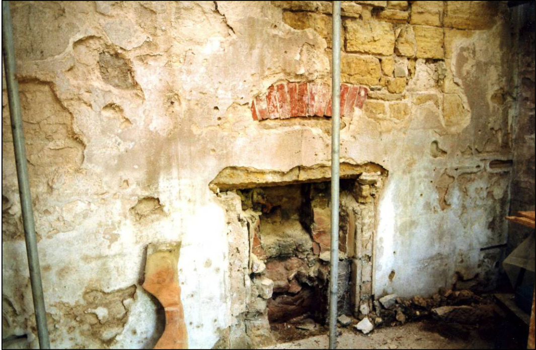
Plate 13: Internal south wall of central cell during renovation, showing fireplace and shelf scarring, looking SE (photo 6/10).
