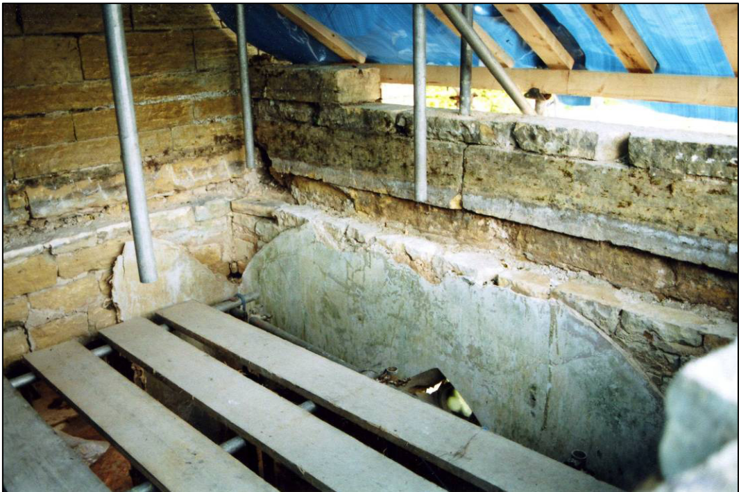
Plate 14: West wing after removal of concrete roof, looking NW (photo 5/31).
