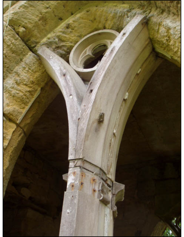
Plate 6: Wooden tracery to north elevation of west wing, looking SE (Peter Pace photograph).
