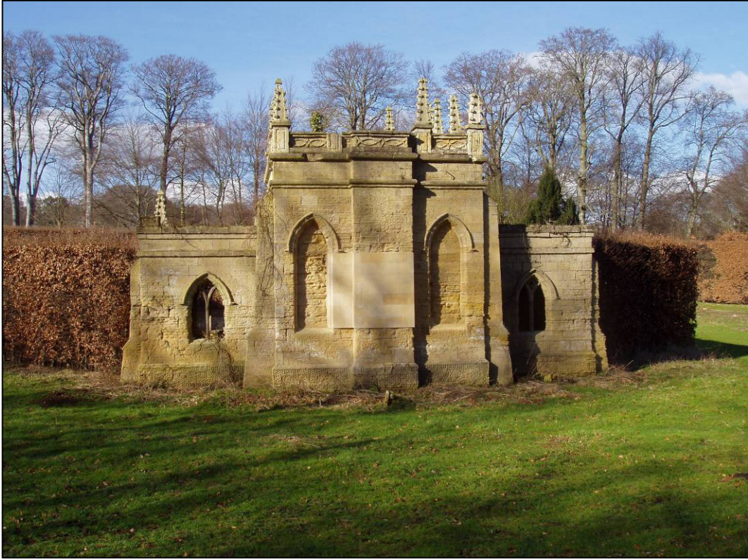
Plate 3: South elevation, looking NW (Peter Pace photograph).
