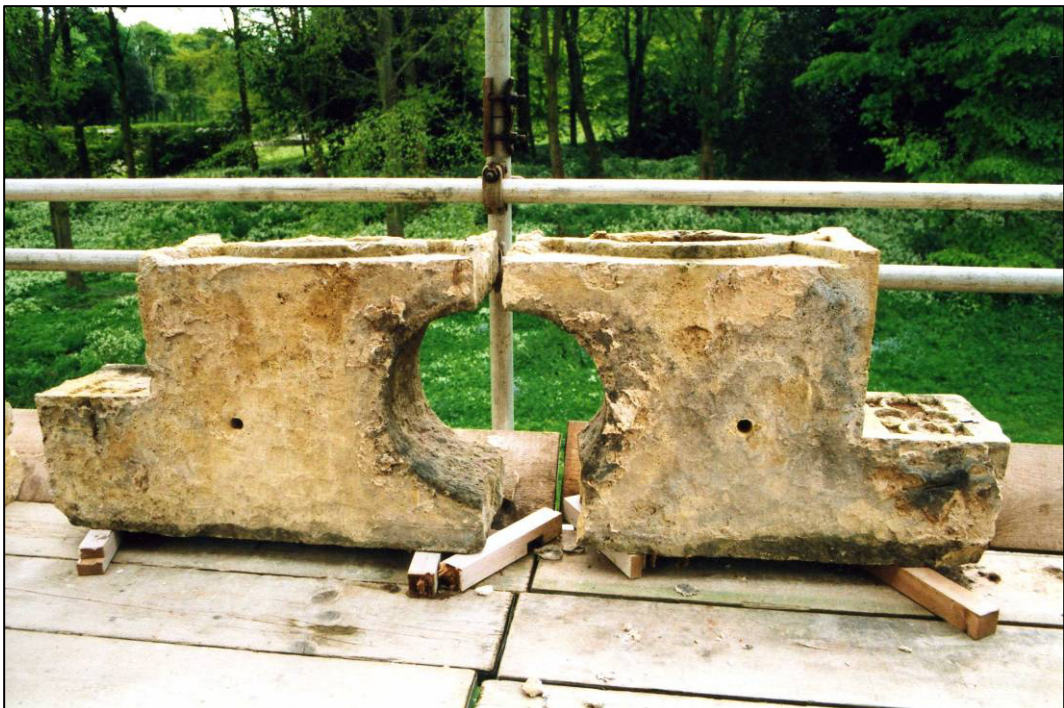
Plate 10: Capping stone of chimney flue (photo 5/36).
