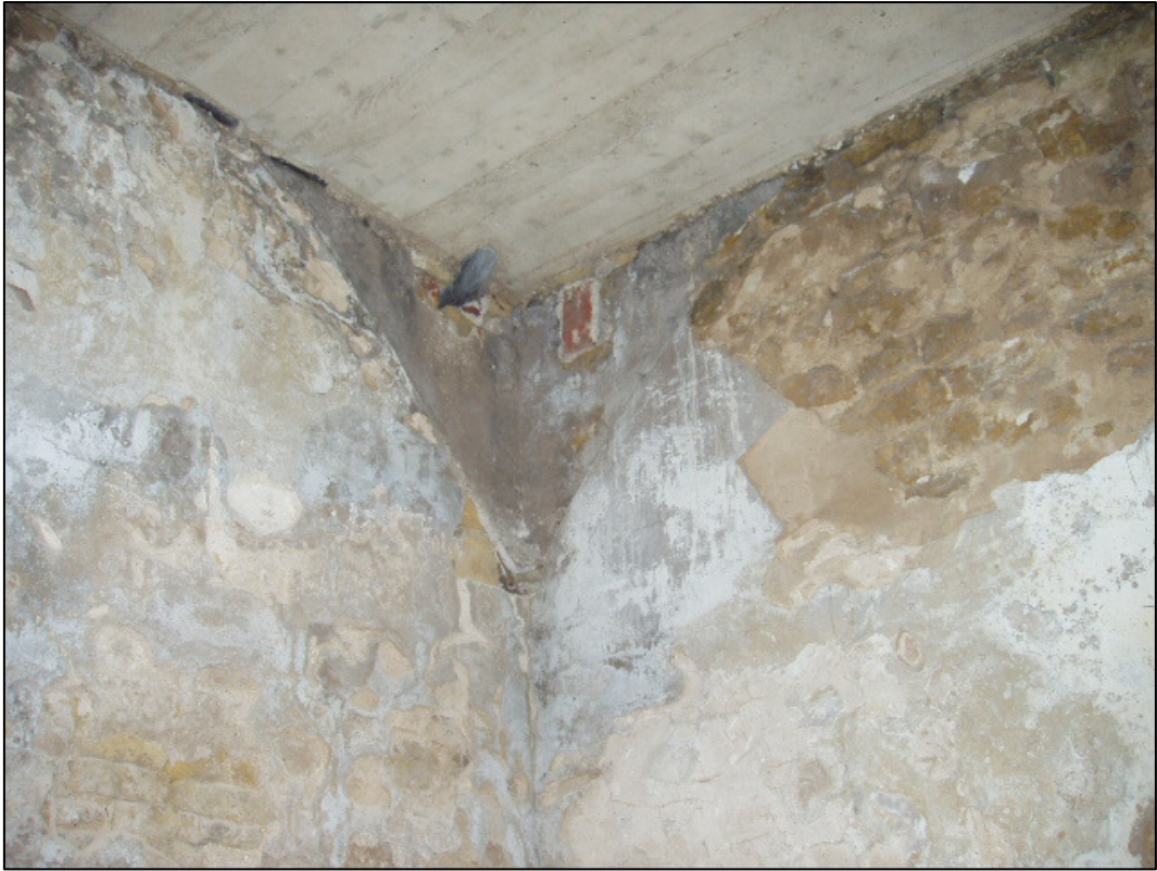
Plate 11: Profile of former cross-vault over central cell, looking SE (Peter Pace photograph).
