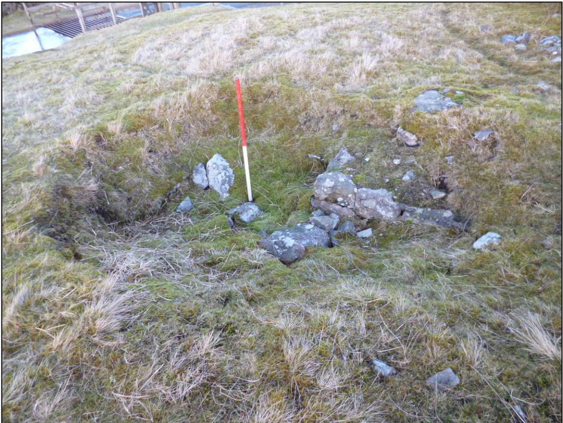
Plate 34: Pulley pit and associated structure (Site 23) at end of incline, looking N (photo 3/051).
