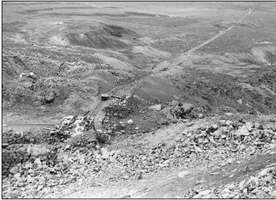
a) 1946 view looking N down the east incline (Site 17) (J O Myers) (source: Swaledale Museum IMG5).
