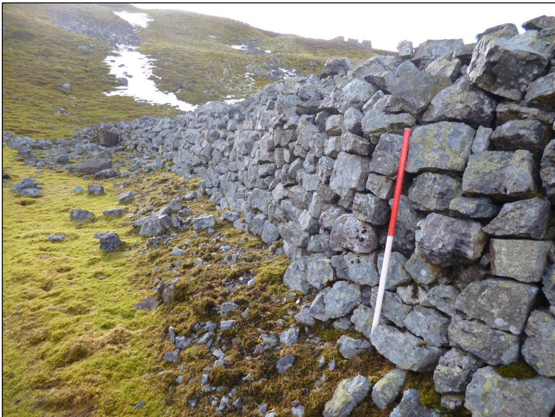
Plate 20: Revetted east face of western chert dressing heap (Site 14a), looking S (photo 3/953).
