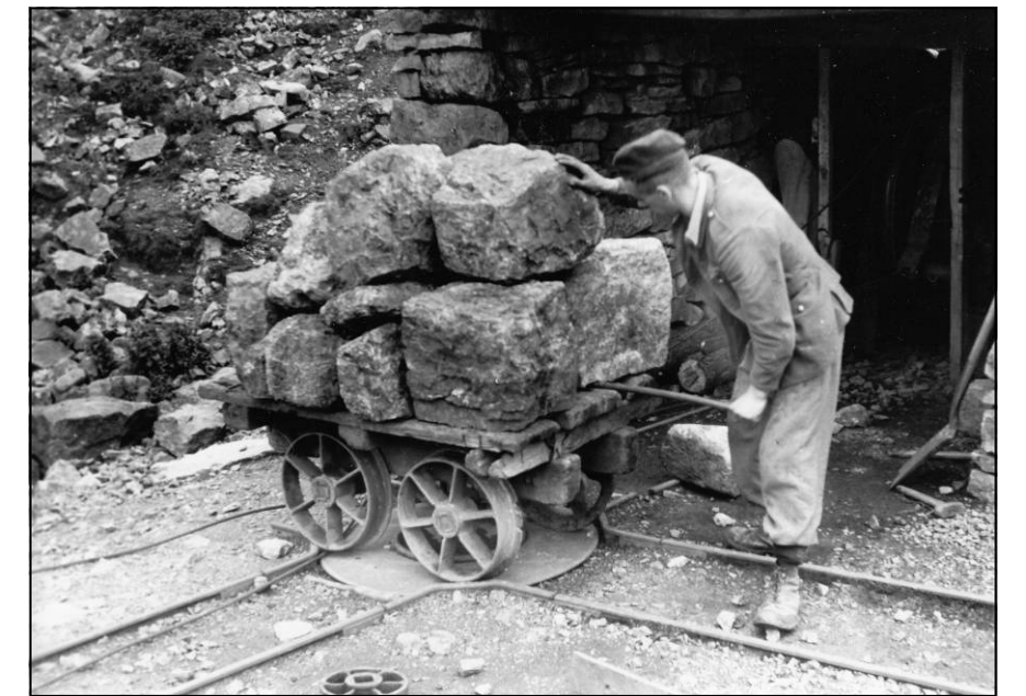
f) Turntable at head of east incline (Site 17) leading to siding and loading bay (Site 13), with lower brake house (Site 12) to rear, looking S (J O Myers) (source: Swaledale Museum IMG3).
