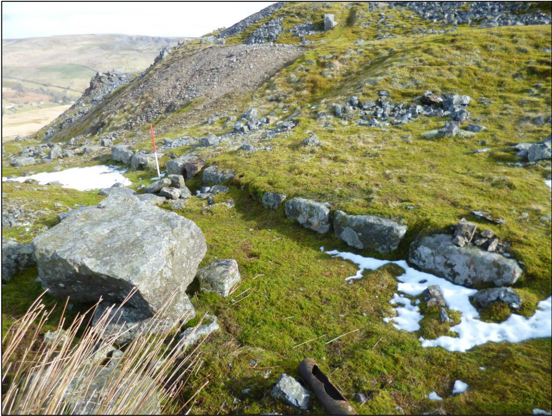
Plate 21: Siding/loading bay (Site 15) at head of west incline, looking NE (photo 3/895).
