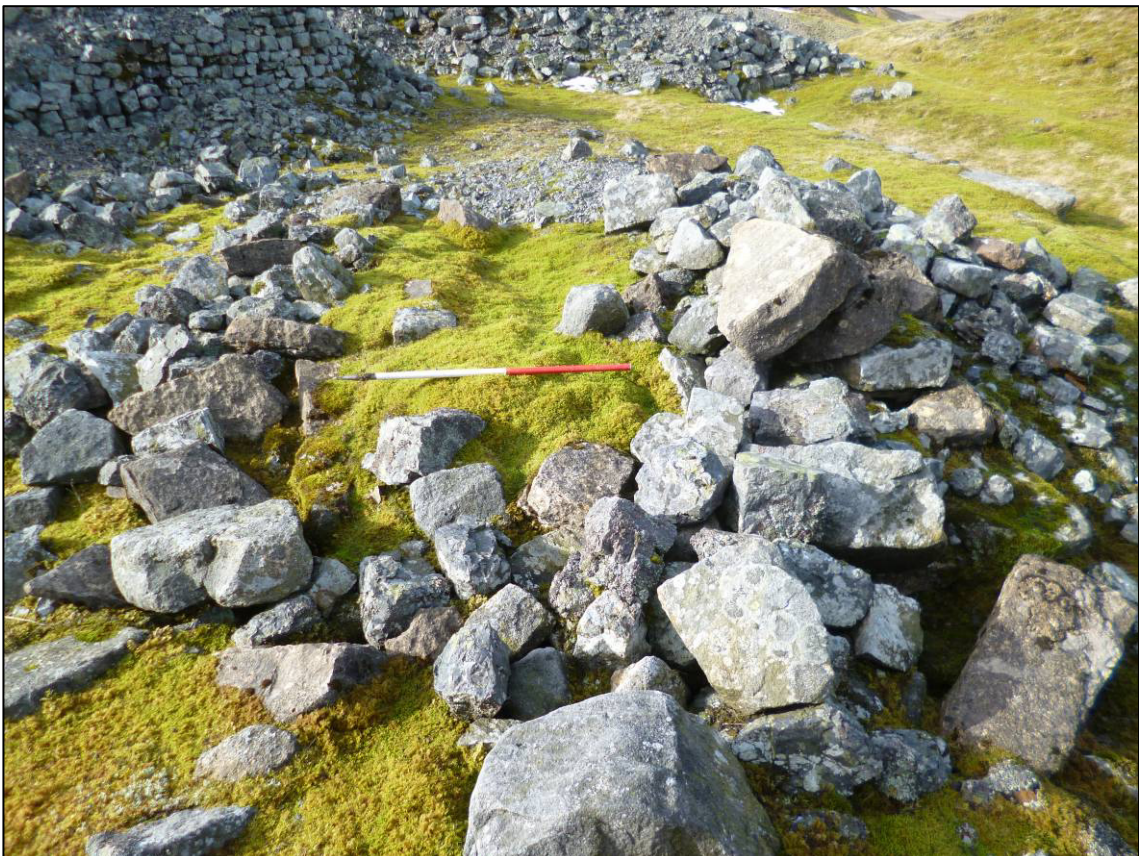
Plate 18: Remains of crane stay (Site 13b) above siding/loading bay at head of east incline, looking W (photo 3/939).
