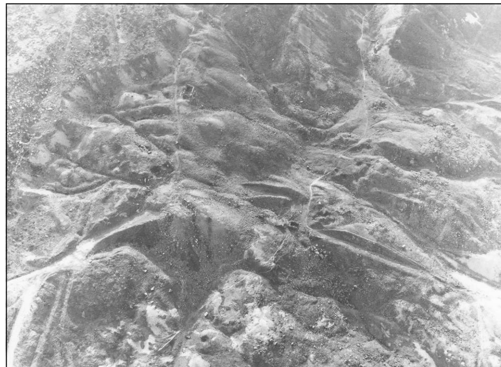
e) Aerial photograph of the chert quarry complex, looking W, taken 5th May 1990, showing ruined smithy (top) and east incline with lower brake house and chert dressing heaps (source YDNPA 040/030).
