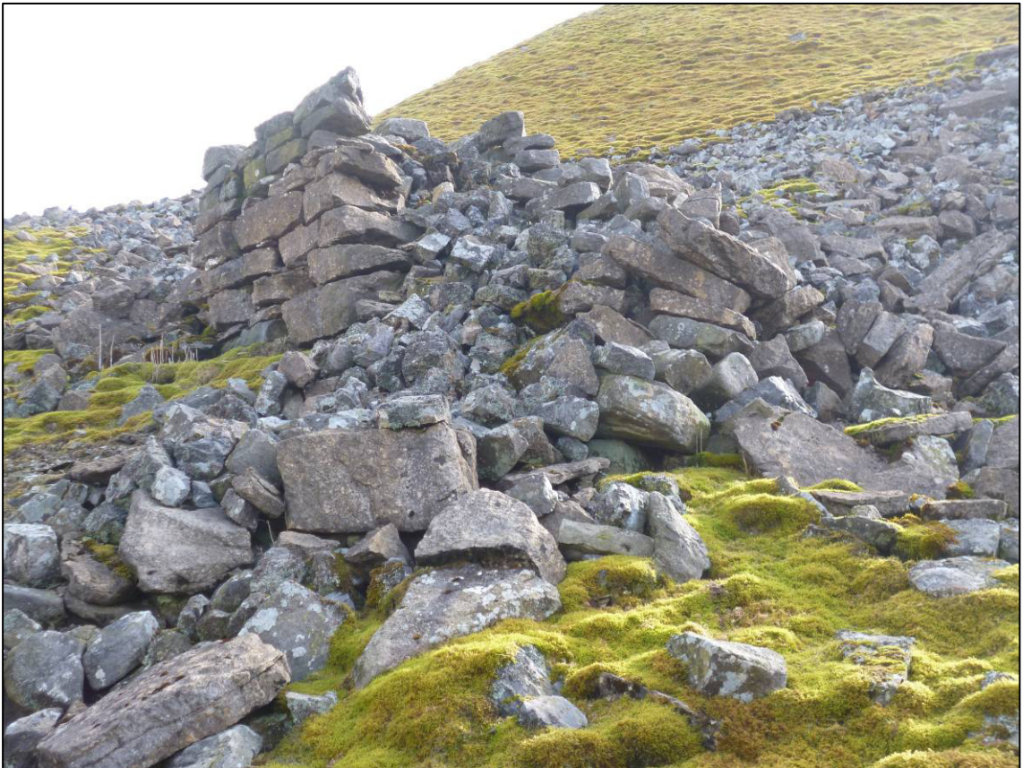
Plate 14: Remains of pier to upper incline (Site 11b), looking SW (photo 3/941).
