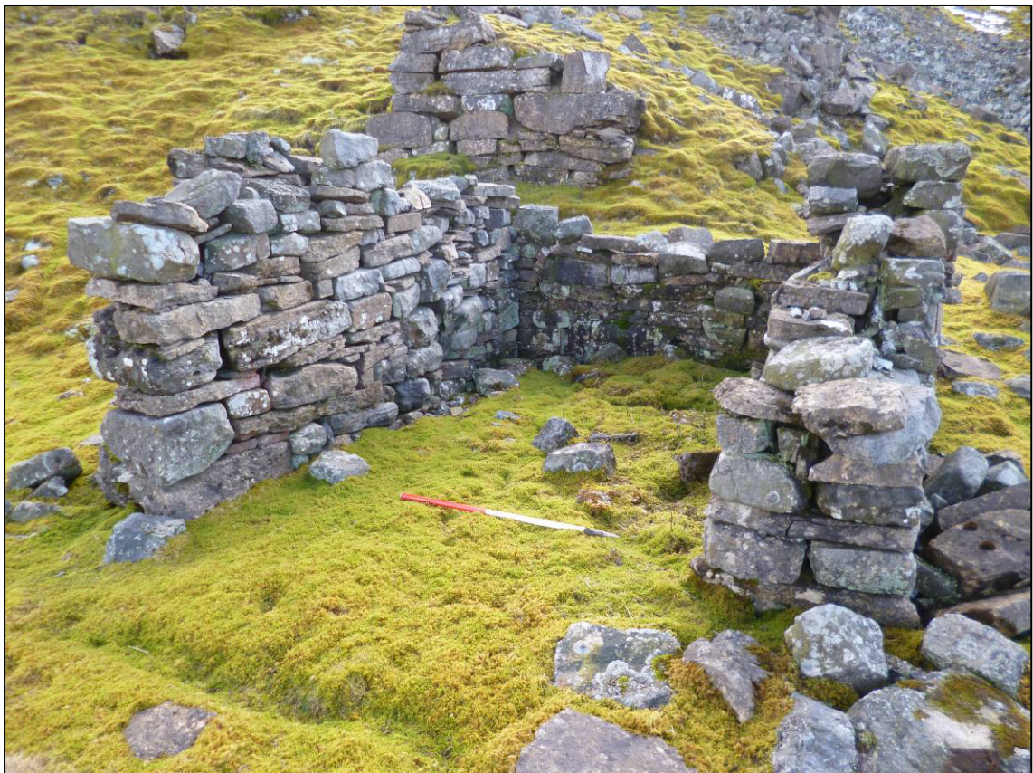
Plate 16: Remains of lower brake house (Site 12), looking SE (photo 3/962).
