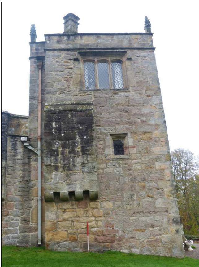
Plate 7: Tower, west elevation, looking NE (photo 1/135).
