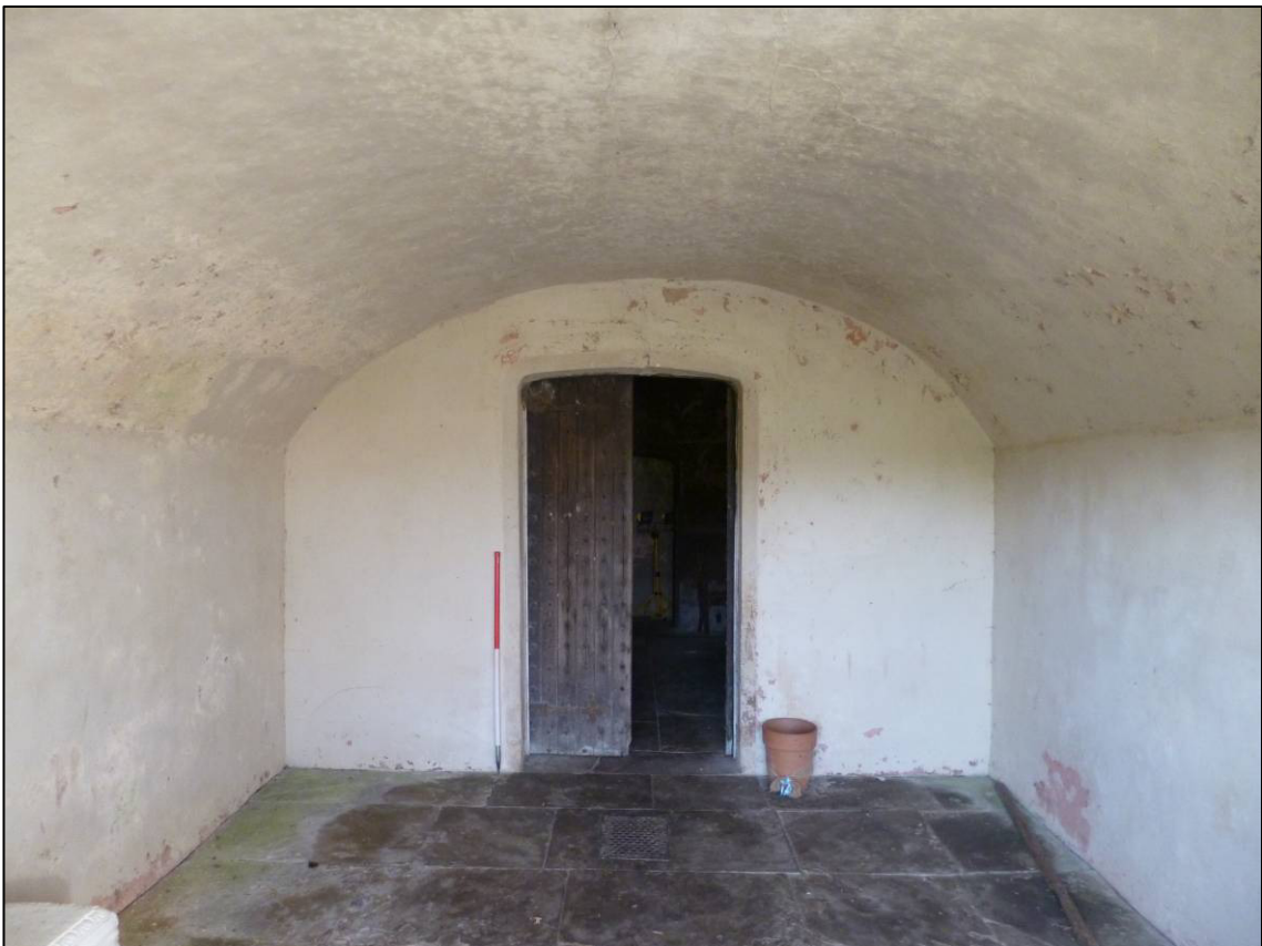
Plate 18: Tower, lower ground floor entrance chamber interior, looking NW (photo 2/648).
