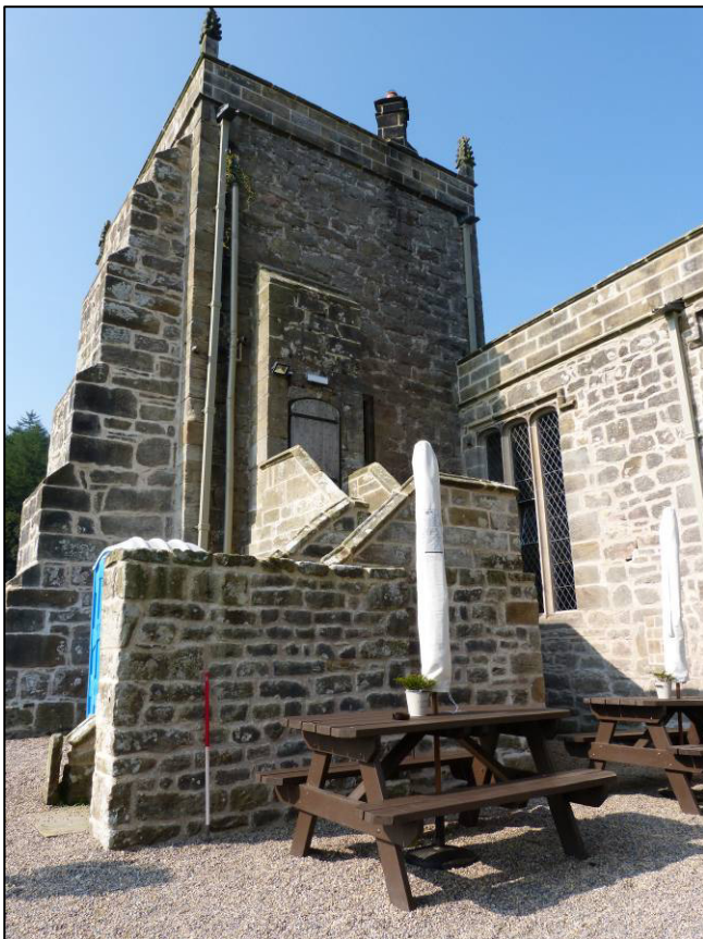
Plate 38: Tower, east elevation and steps, works complete, looking W (photo 7/581).
