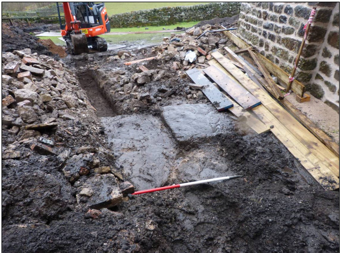
Plate 36: Drainage trench T4, wall footings (008), looking S (photo 6/923).
