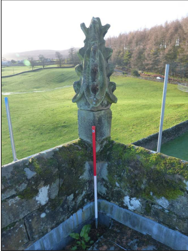
Plate 26: Tower, south-west corner pinnacle, looking S (photo 2/316).
