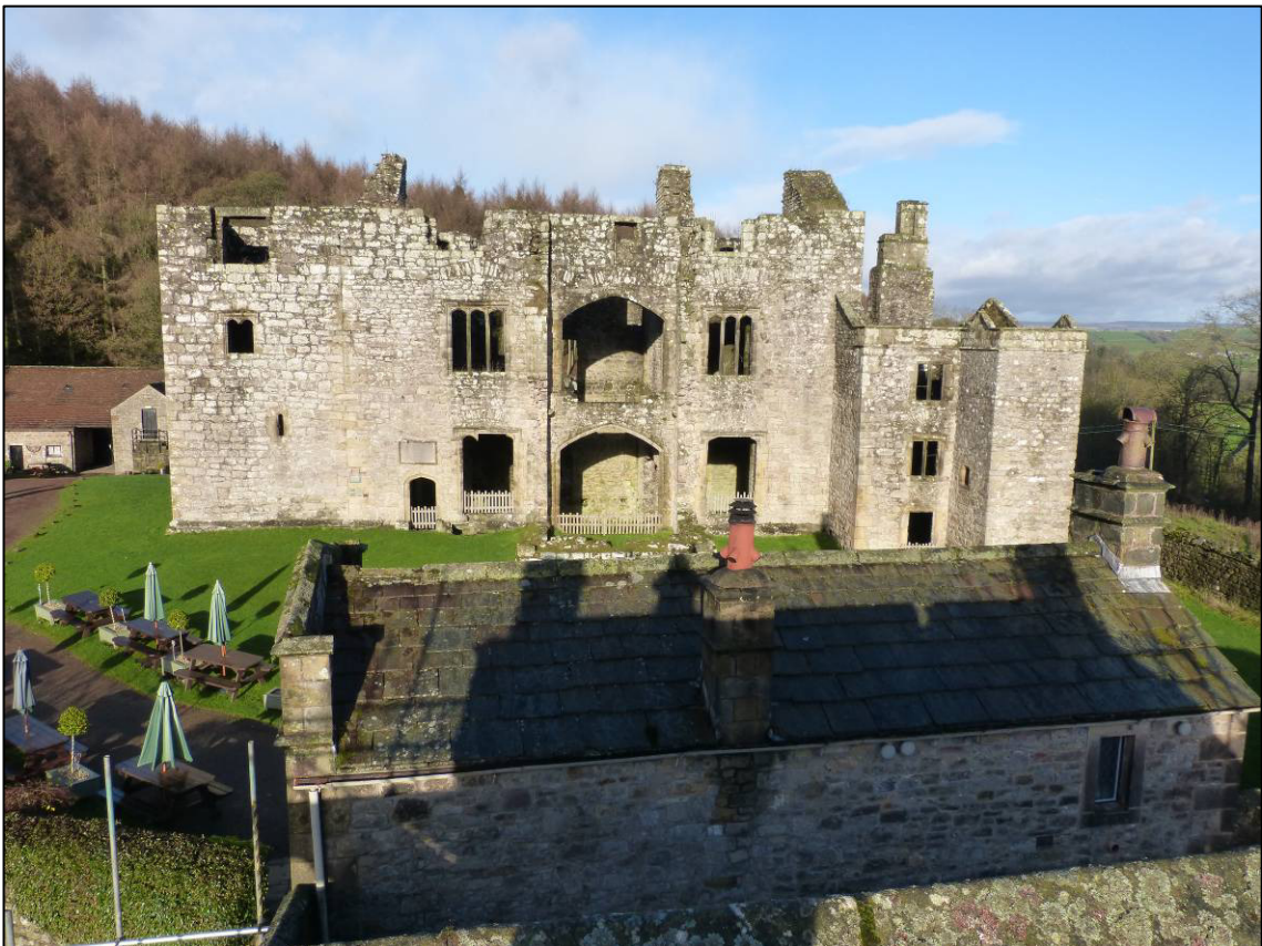
Plate 2: Barden tower, from roof of Priest's House tower, looking NW (photo 2/319).
