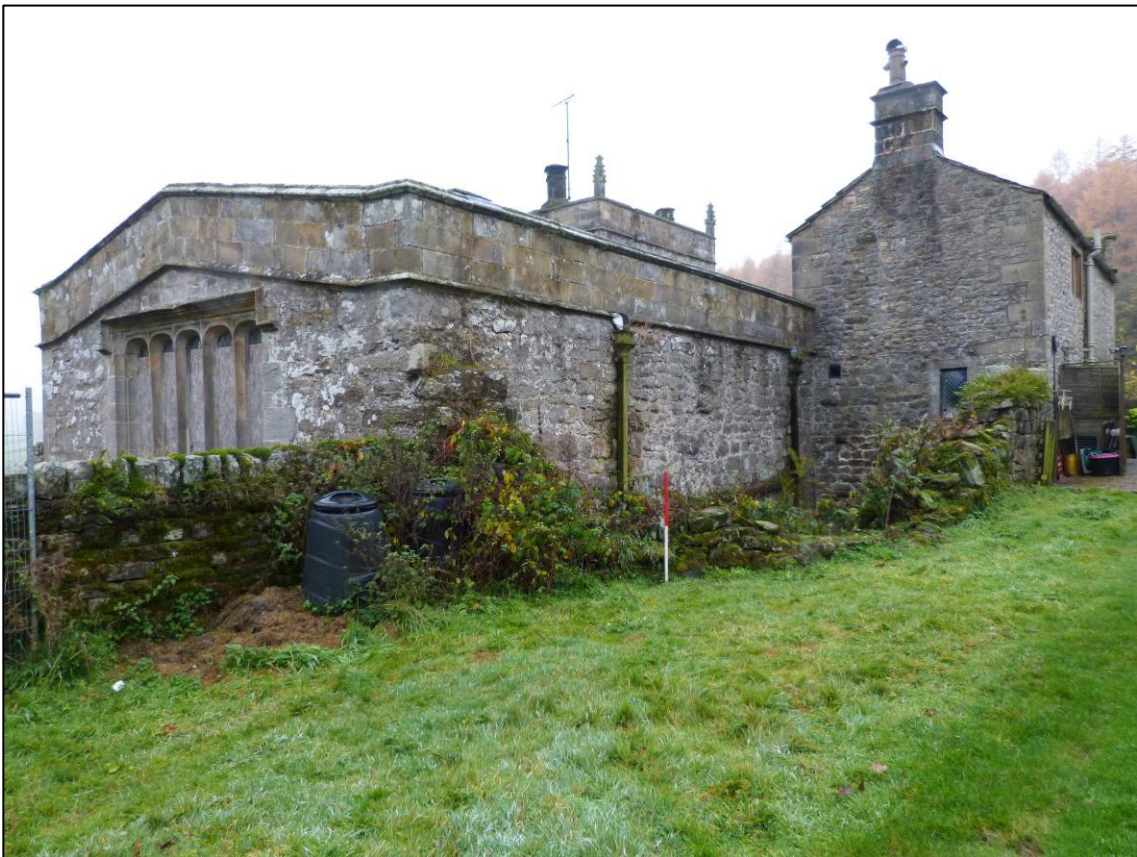
Plate 13: Chapel and domestic block, looking SW (photo 1/101).
