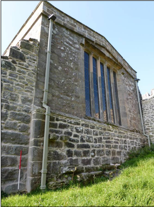
Plate 40: Chapel, east gable, works complete, looking NW (photo 7/590).
