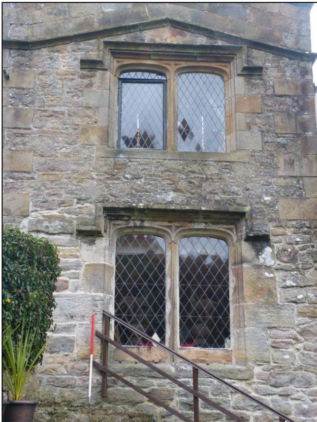
Plate 4: Domestic block, windows in west elevation, looking NE (photo 1/130).
