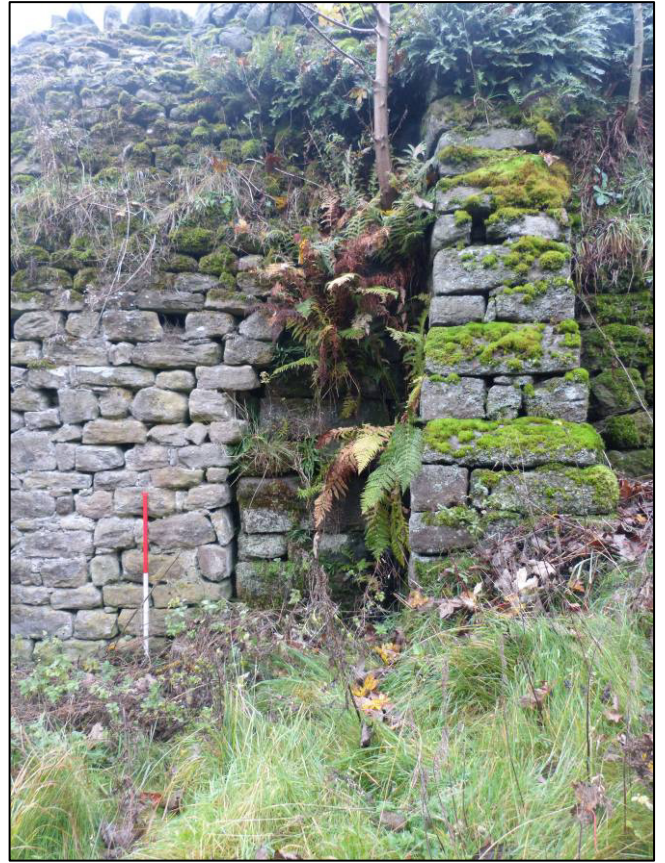
Plate 20: Retaining wall, north-east of chapel, east elevation, looking SW (photo 1/201).
