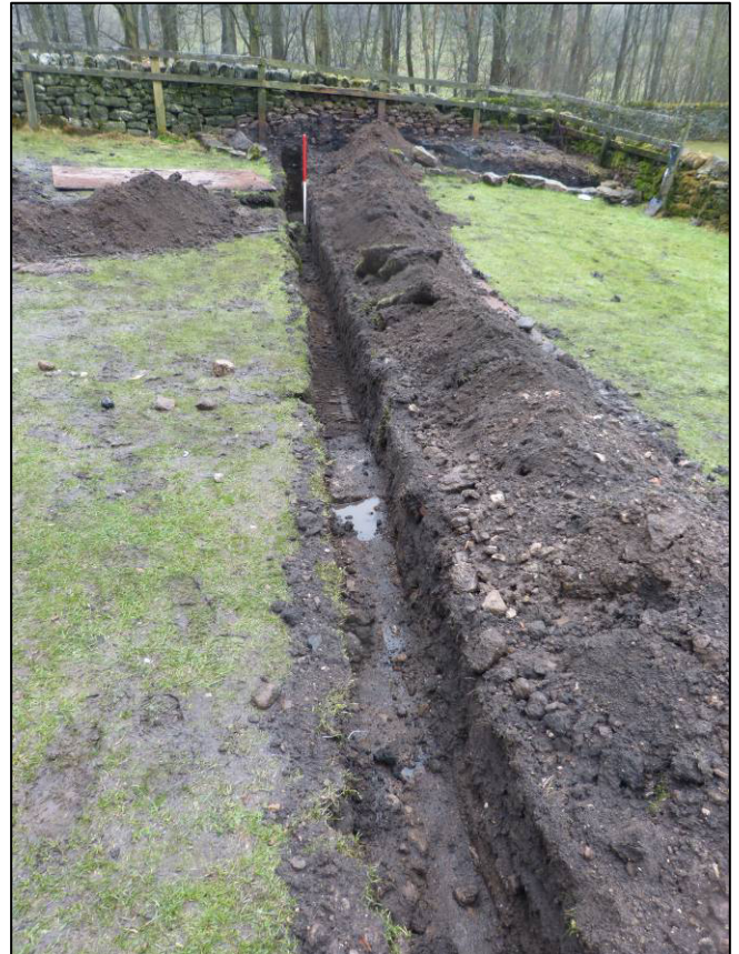
Plate 32: Drainage trench T2, east end, looking E (photo 6/929).
