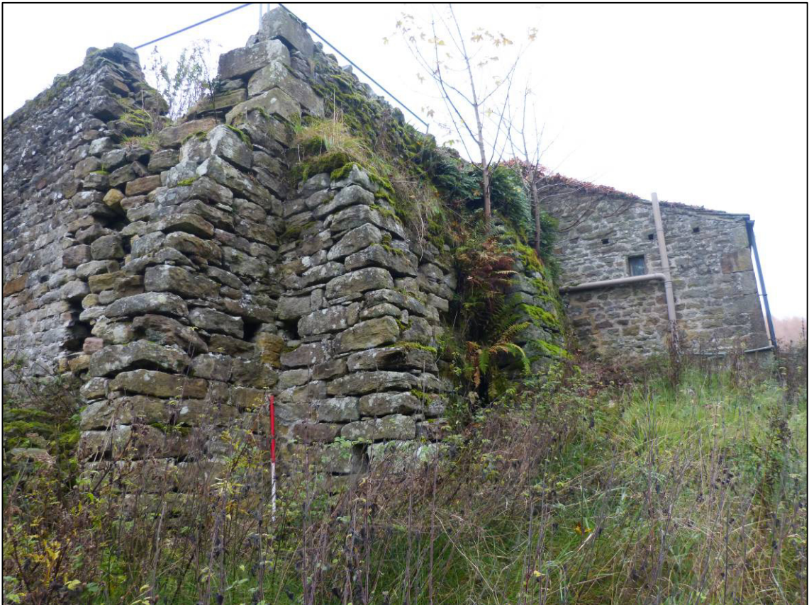
Plate 24: Retaining wall, north-east of chapel, corner buttress, looking NW (photo 1/198).
