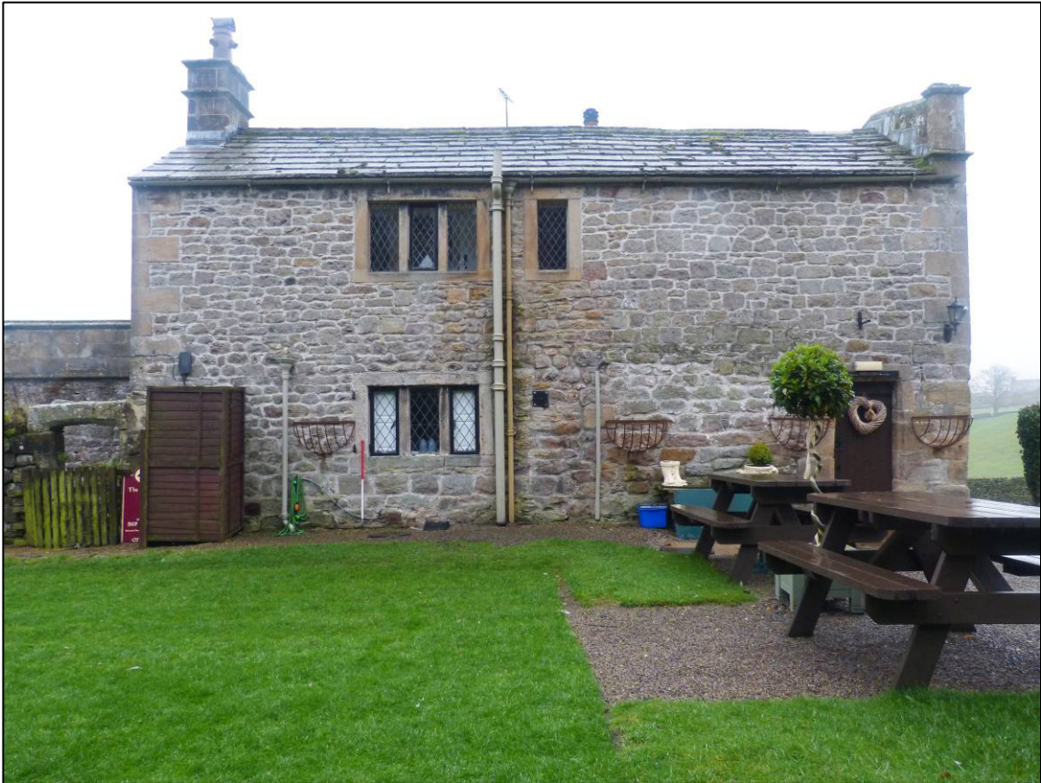
Plate 17: Domestic block, north elevation, looking SE (photo 1/118).
