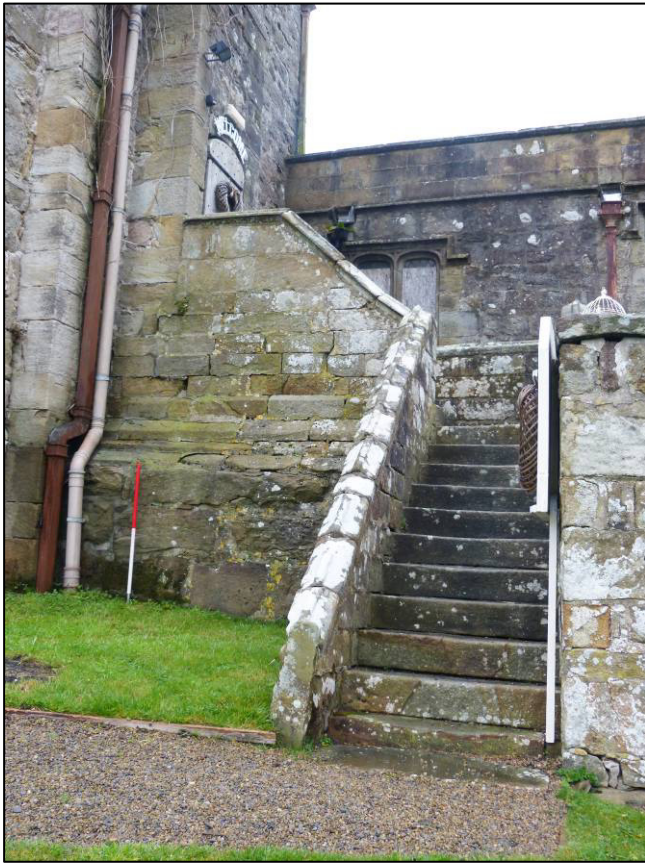
Plate 9: Tower, staircase on east elevation, looking NW (photo 1/157).
