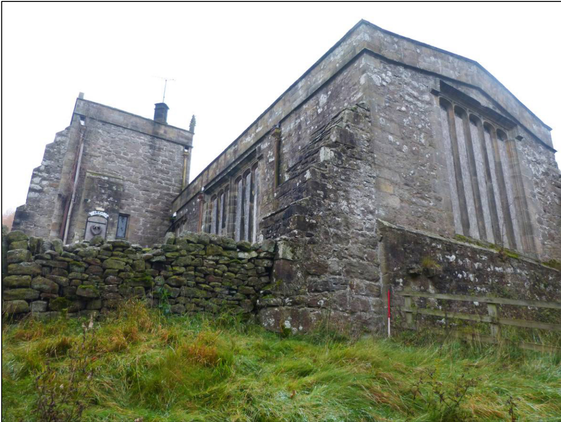
Plate 12: Chapel, east gable and buttress, looking W (photo 1/187).
