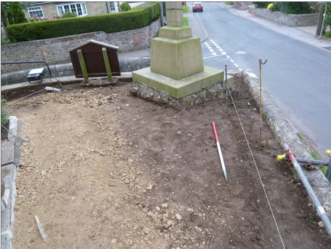
Plate 2: War memorial after excavations for landscaping works, looking W.
