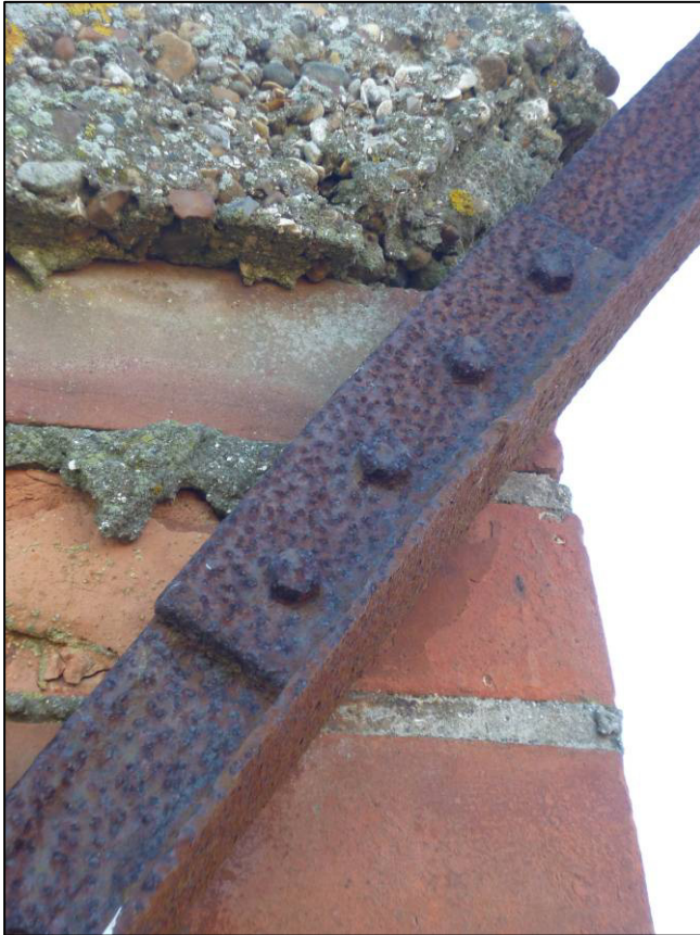
Plate 8: Structure A2 (canteen), rib detail, looking SW (photo 1/598).
