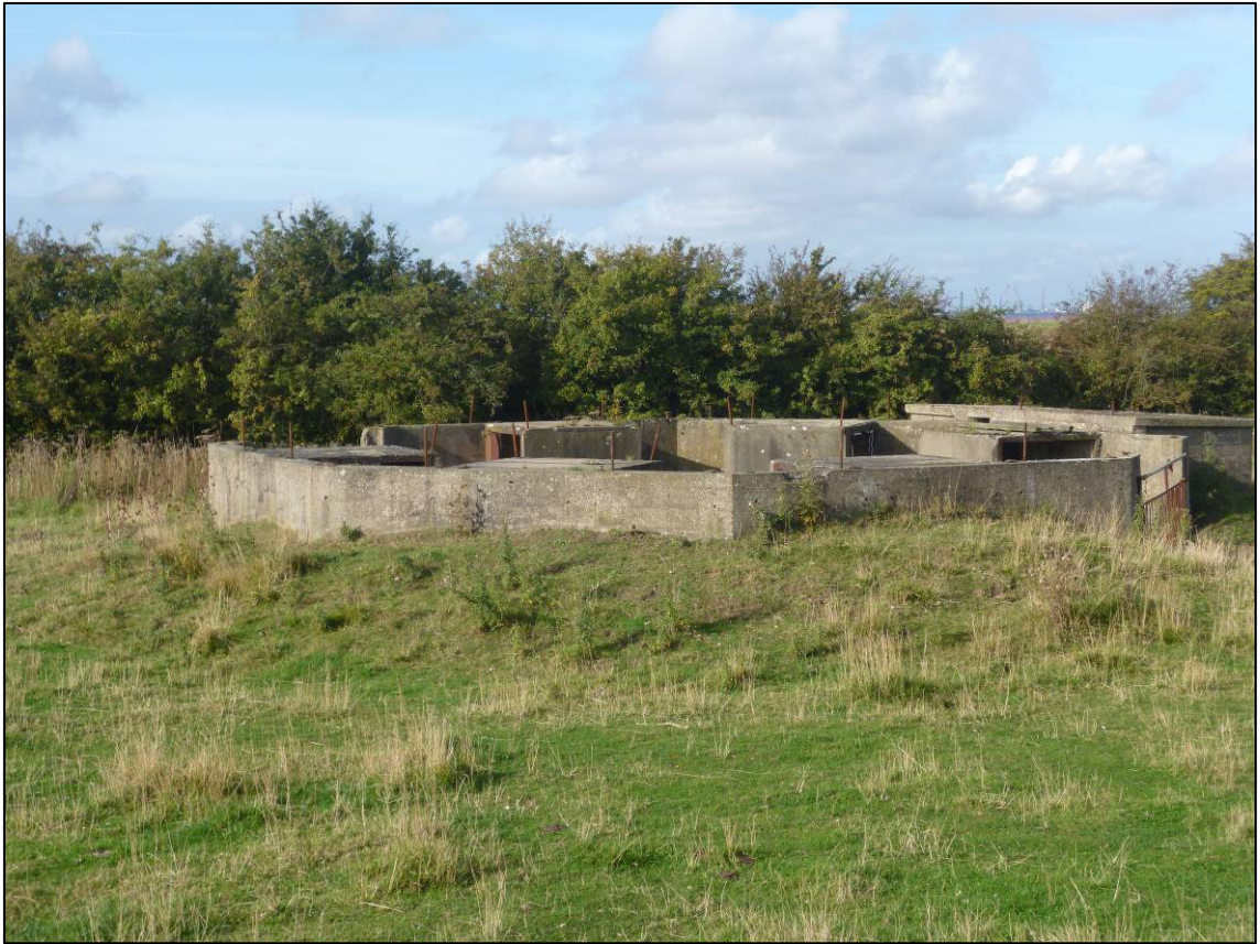
Plate 54: Structure G (gun emplacement), looking SW (photo 2/119).
