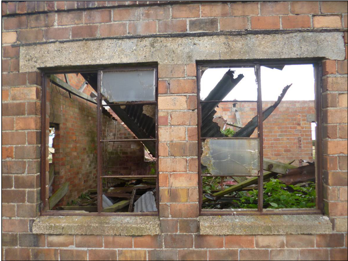
Plate 14: Structure A3 (cookhouse), window detail in central part of west elevation, looking E (photo 1/704).
