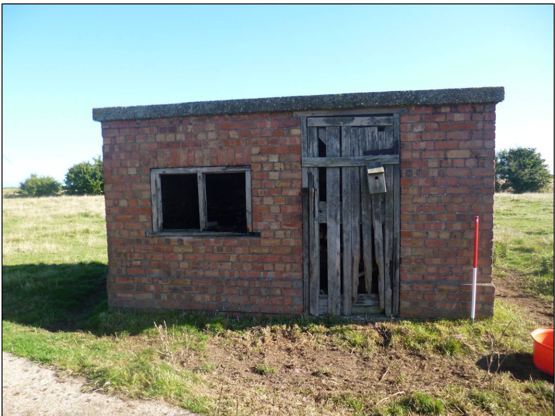
Plate 5: Structure A1 (sub-station), W elevation, looking NE (photo 1/537).
