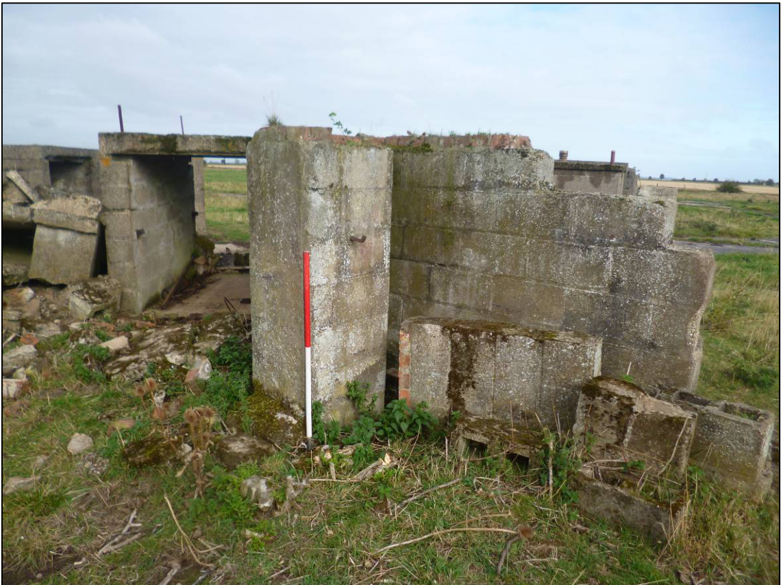
Plate 48: Structure D (gun emplacement), remains of shelter on south side, looking N (photo 3/298).
