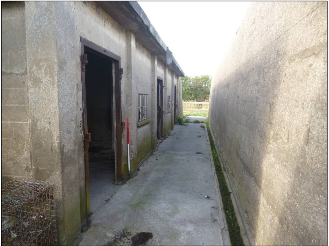
Plate 68: Structure H (magazine), passage inside north blast wall, looking SW (photo 2/210).
