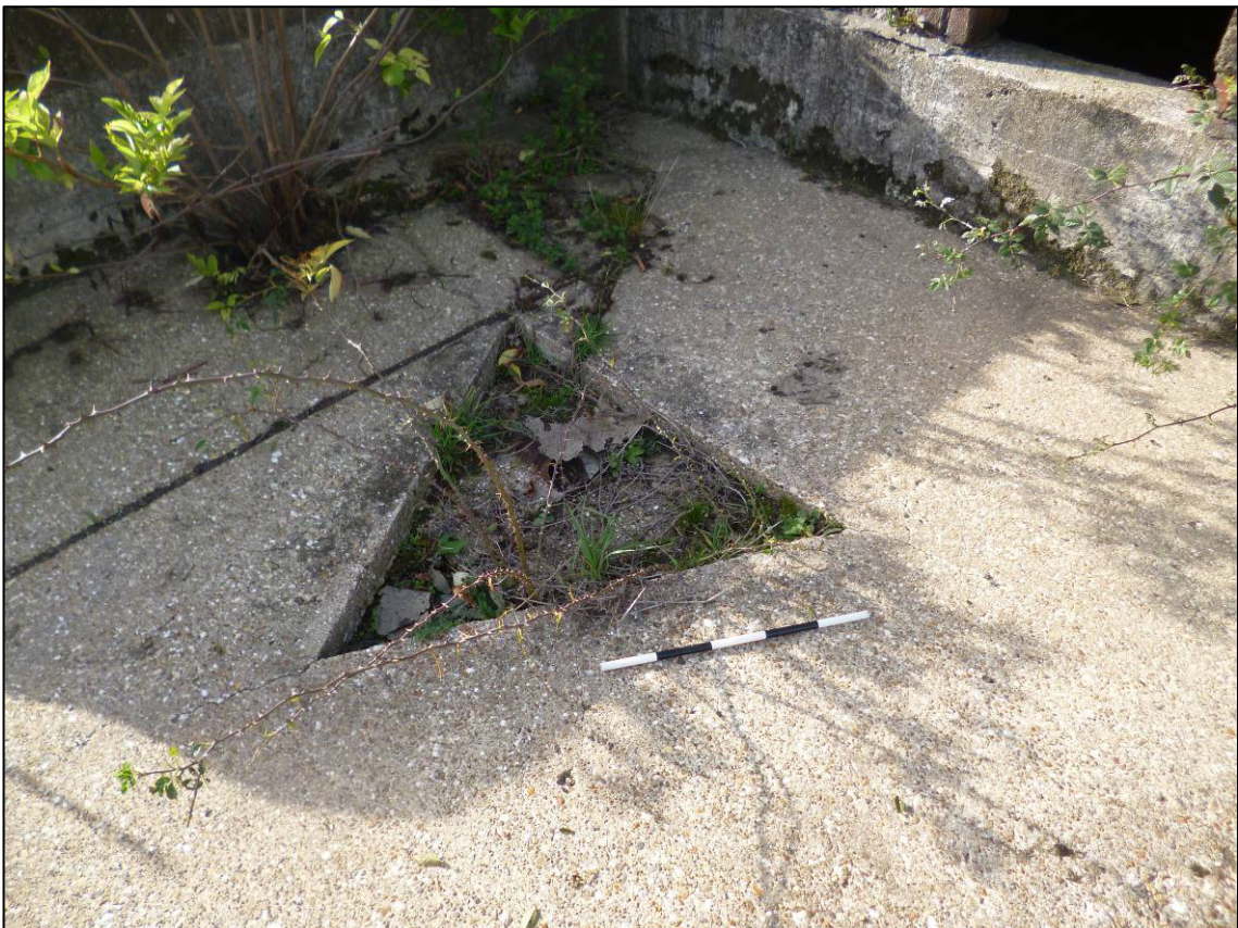
Plate 33: Structure B (command post), recess in predictor platform, looking NW (photo 2/160).
