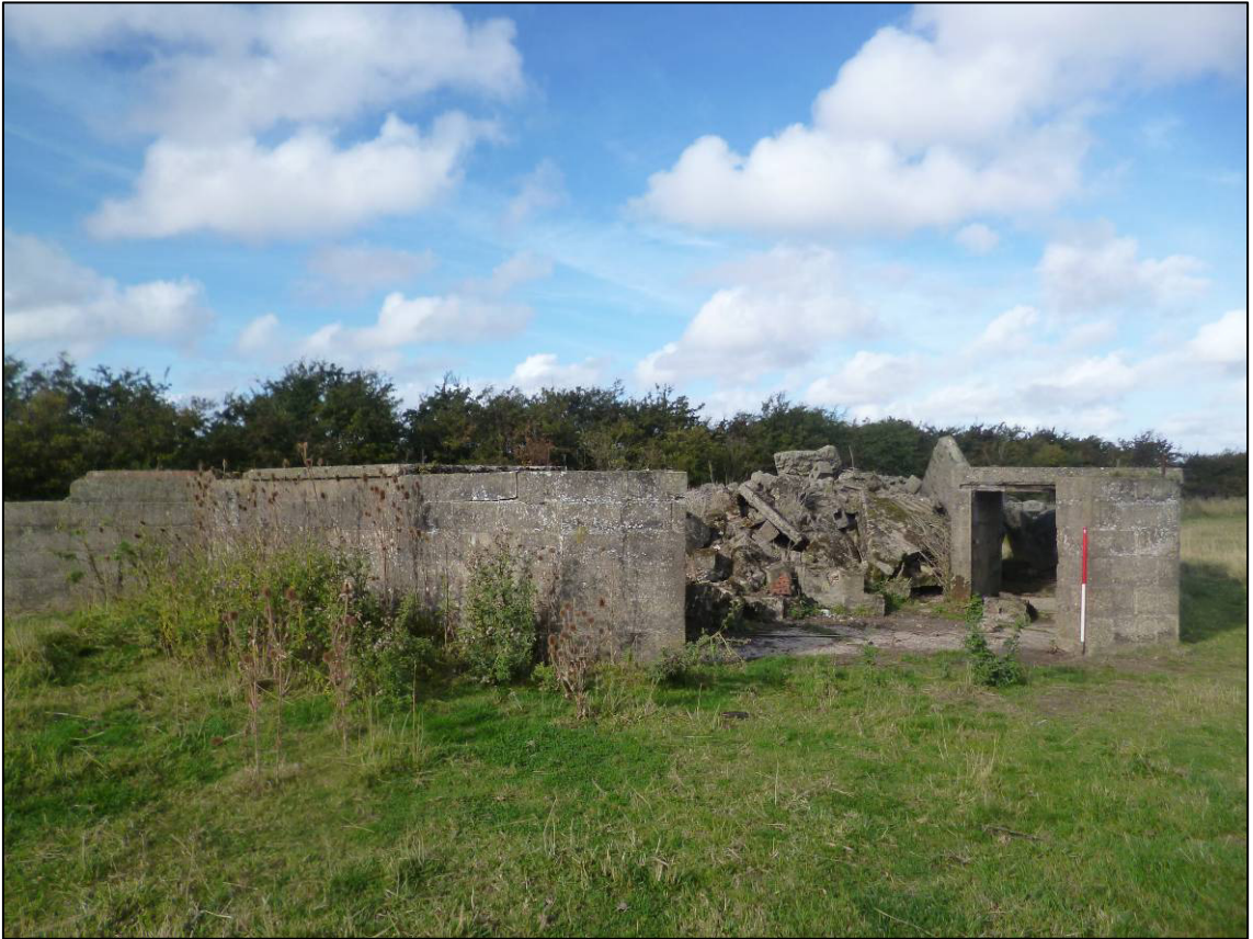
Plate 47: Structure D (gun emplacement), south side, looking NW (photo 2/178).
