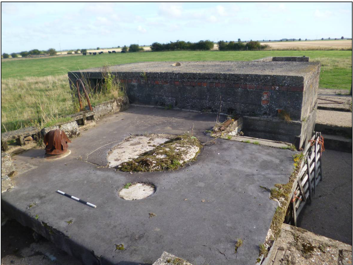
Plate 37: Structure B (command post), Room 2 roof, looking NE (photo 2/159).
