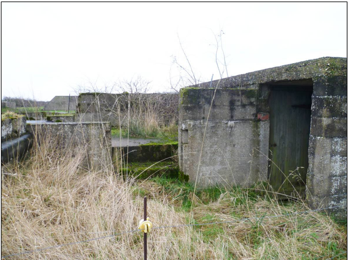
Plate 24: Structure B (command post), entrance in north elevation, looking SE (photo 6/693).
