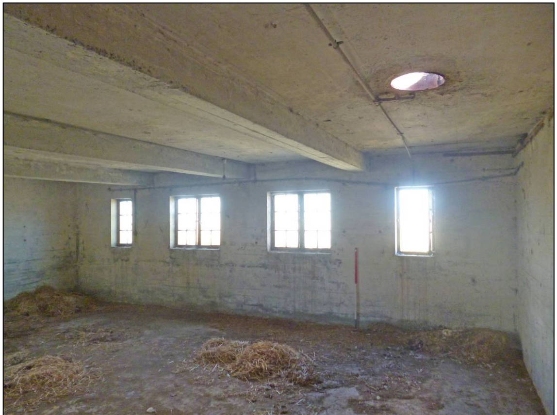
Plate 65: Structure E (gun store), internal view, looking E (photo 2/231).
