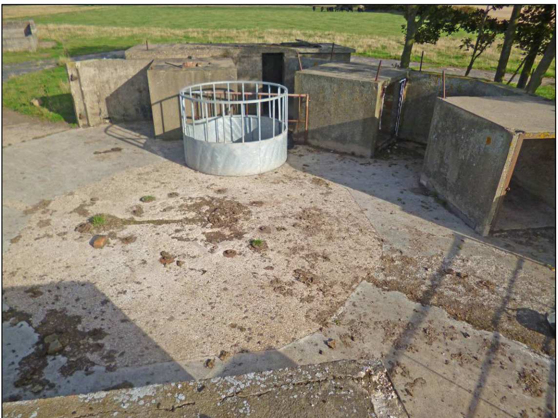
Plate 50: Structure F (gun emplacement), holdfast and ammunition recesses, with shelter to the rear, looking NE (photo 2/118).
