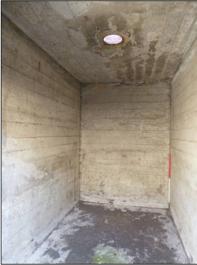
Plate 70: Structure H (magazine), east internal bay, looking SE (photo 2/219).
