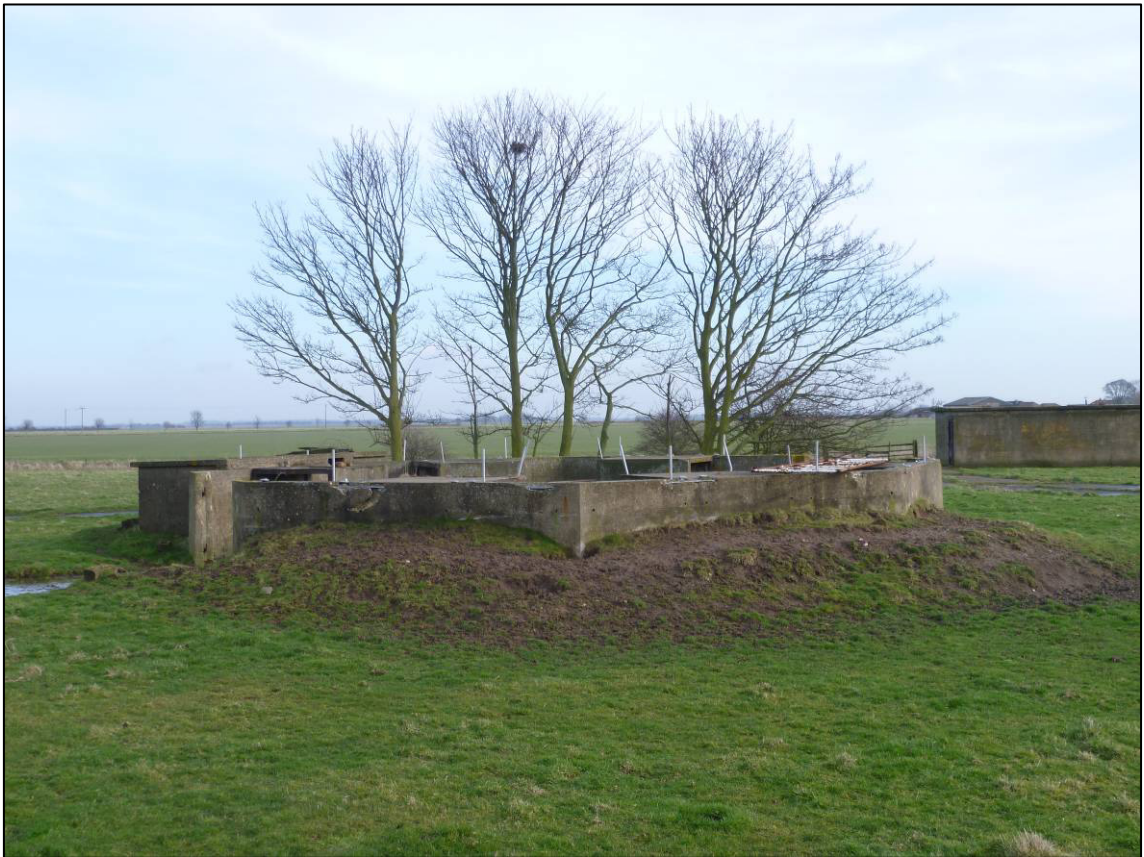
Plate 49: Structure F (gun emplacement), looking E (photo 4/701).
