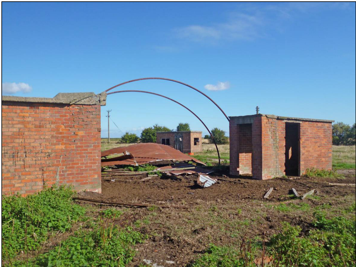
Plate 7: Structure A2 (canteen) showing ribs of collapsed Nissen hut and east entrance structure, looking N (photo 1/584).
