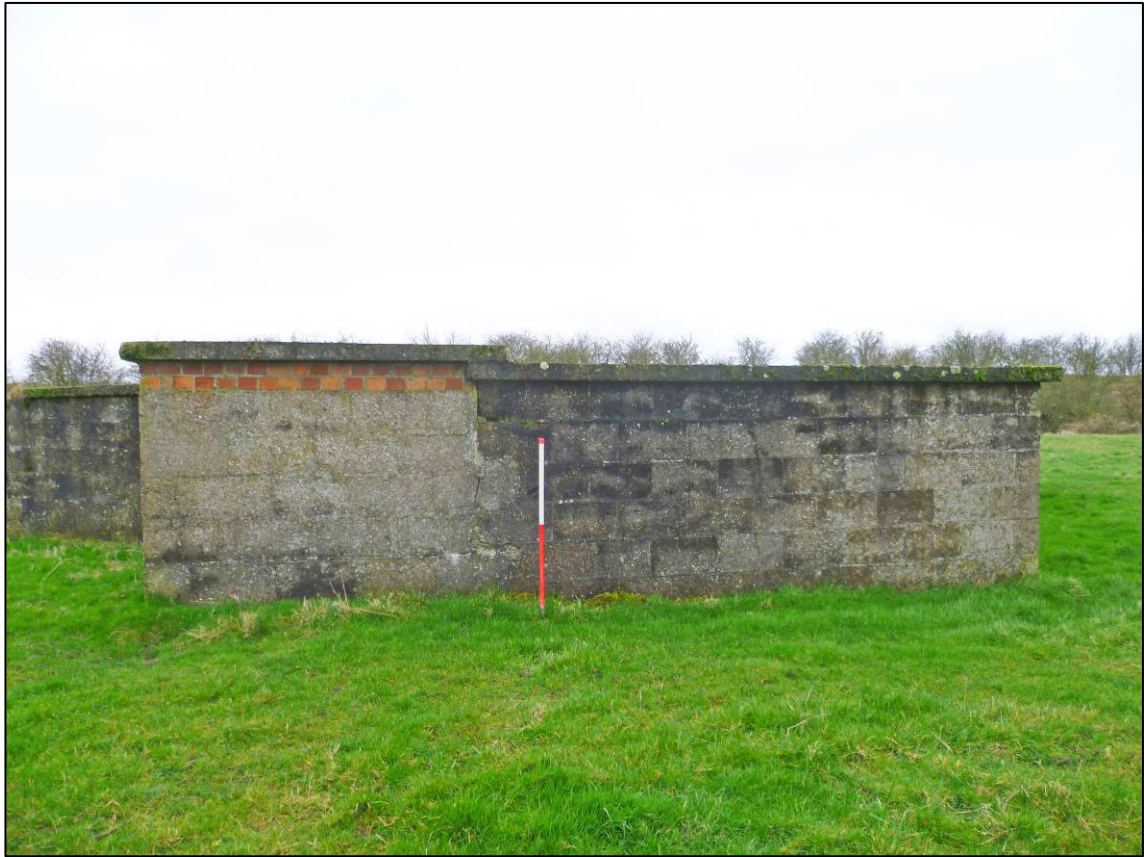
Plate 44: Structure C (gun emplacement), extension to shelter, looking SW (photo 6/697).
