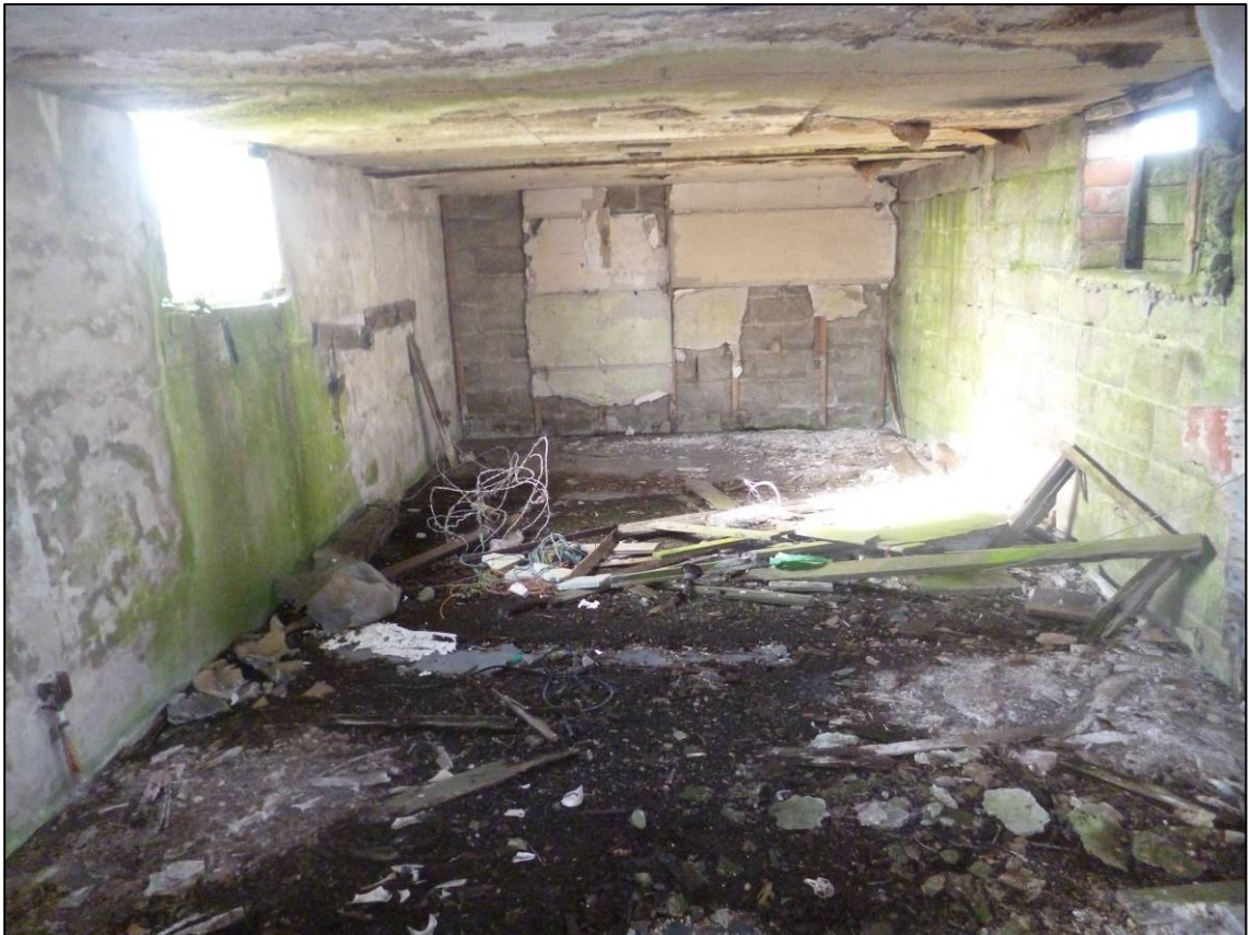
Plate 39: Structure B (command post), interior of Room 3, looking SW (photo 2/168).
