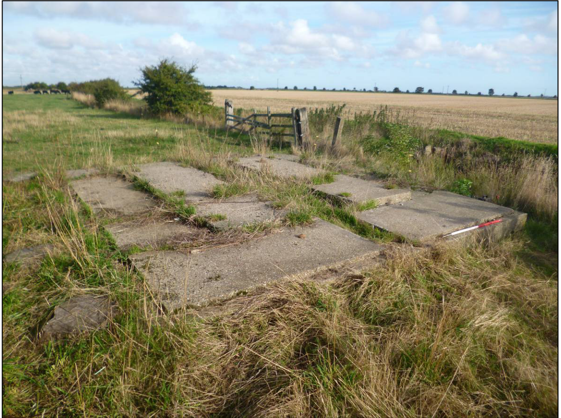
Plate 66: Structure E (gun store), concrete bases to east, looking N (photo 2/104).
