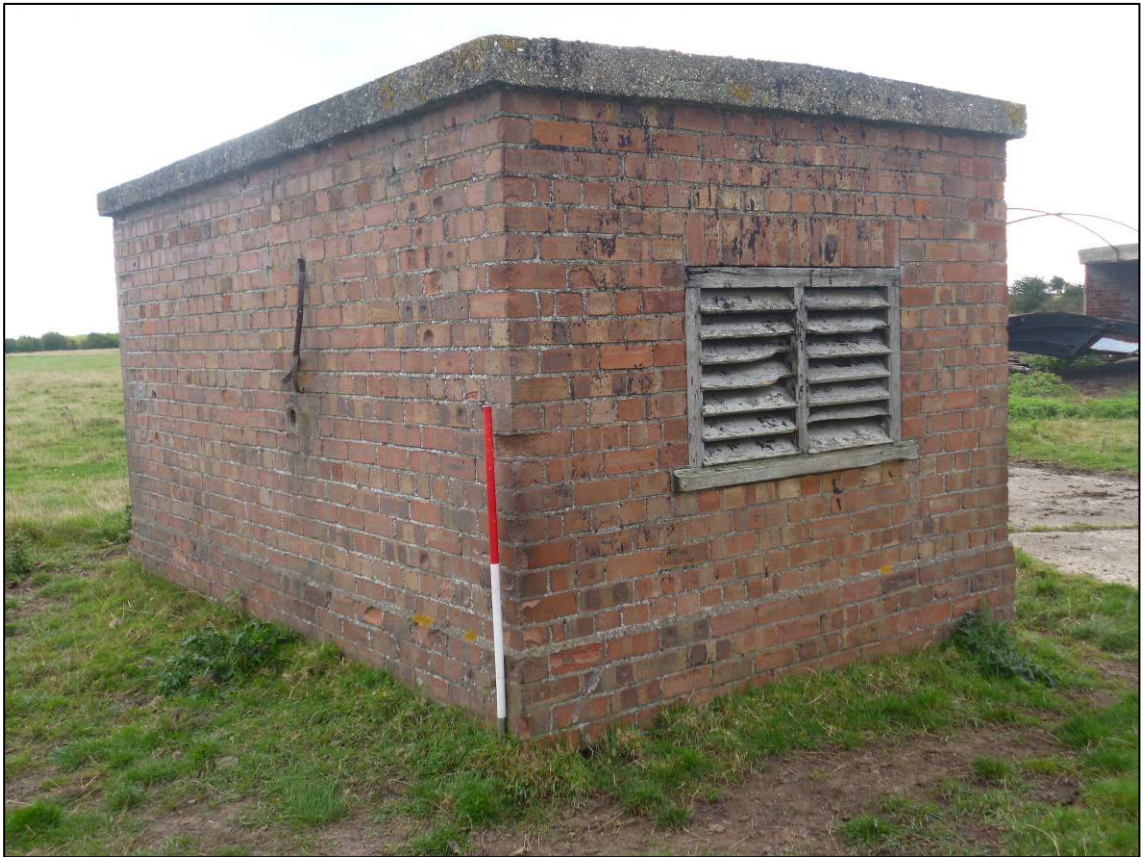
Plate 4: Structure A1 (sub-station), looking S (photo 1/691).
