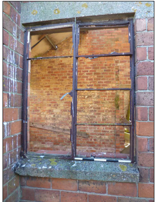
Plate 13: Structure A3 (cookhouse), north gable, central window detail, looking S (photo 1/617).
