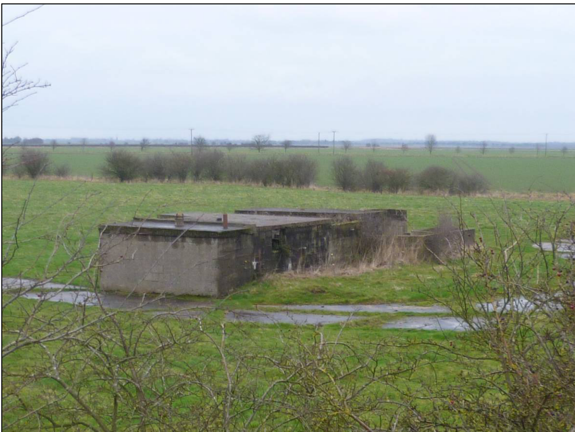
Plate 22: Structure B (command post), general view, looking NE (photo 6/738).
