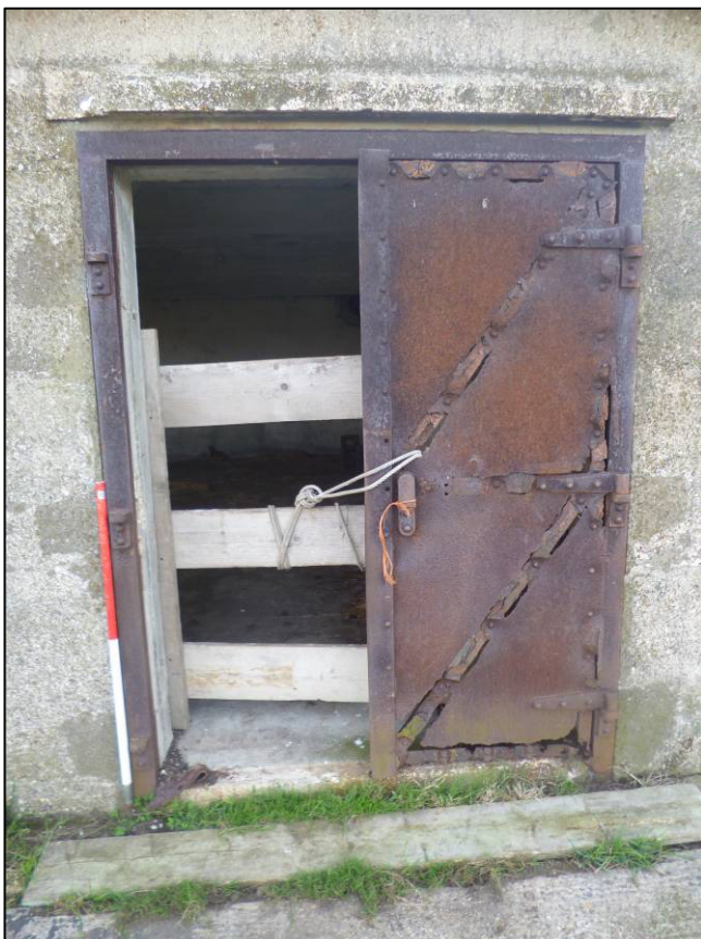
Plate 62: Structure E (gun store), north elevation, blast door, looking SE (photo 2/087).
