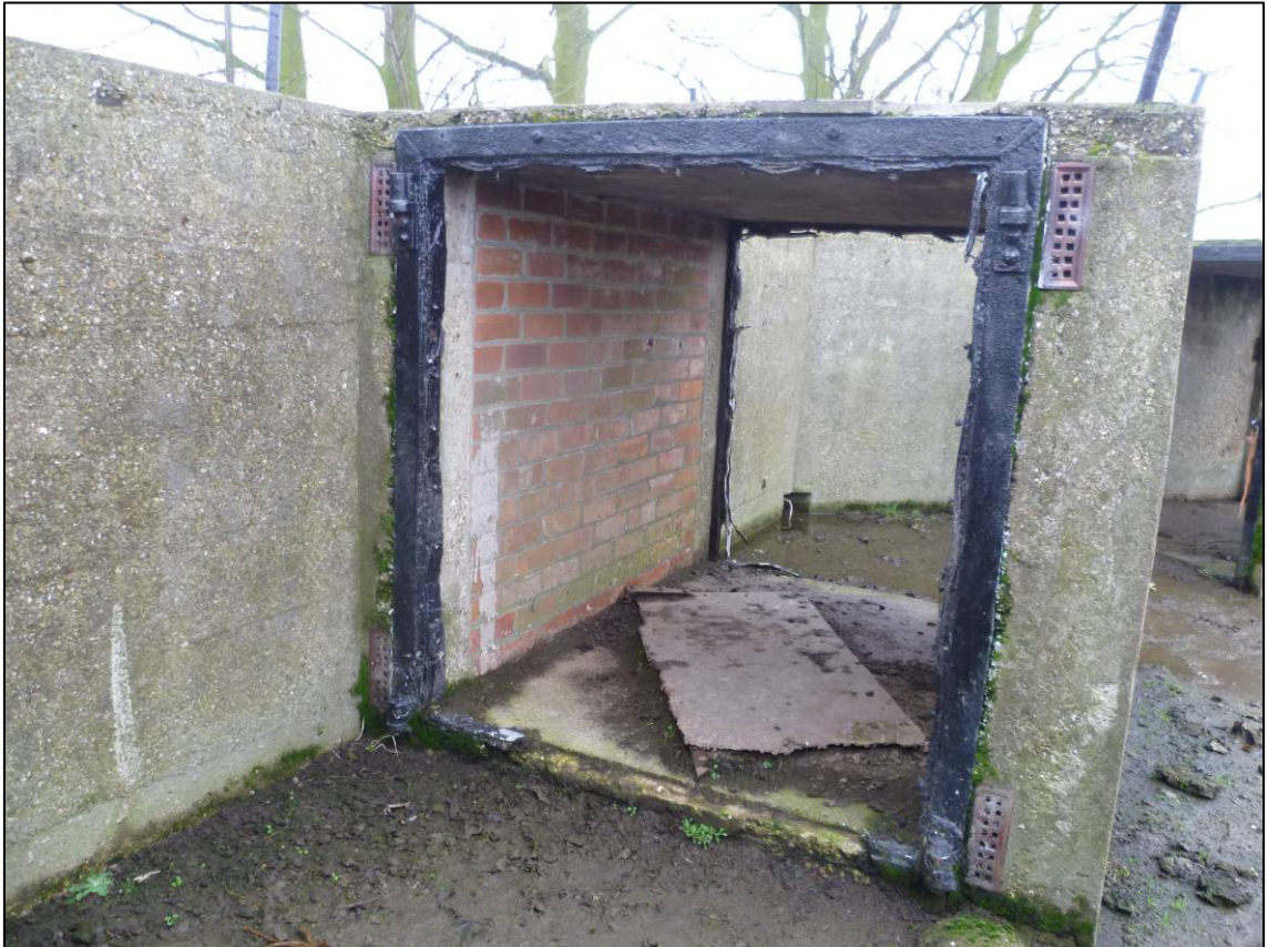
Plate 51: Structure F (gun emplacement), Type 2 ammunition recess, looking NW (photo 6/723).
