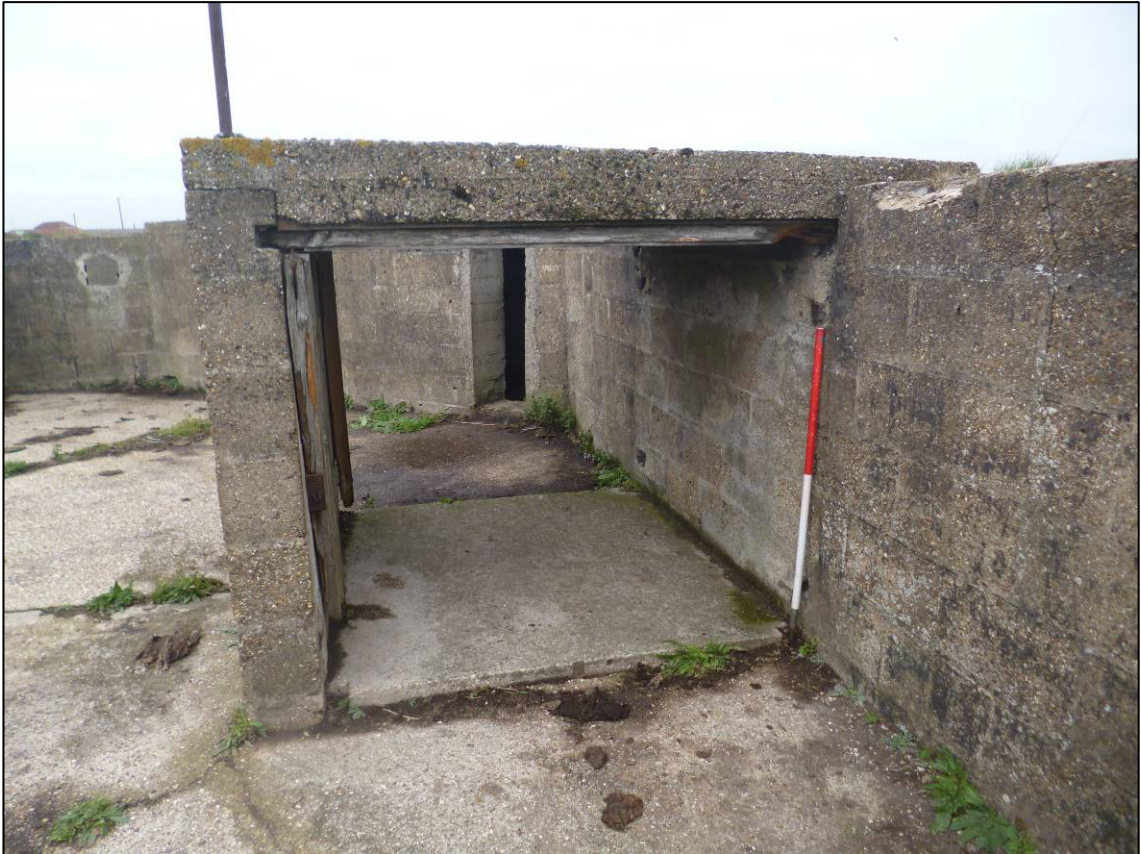
Plate 42: Structure C (gun emplacement), Type 1 ammunition recess, looking N (photo 3/303).
