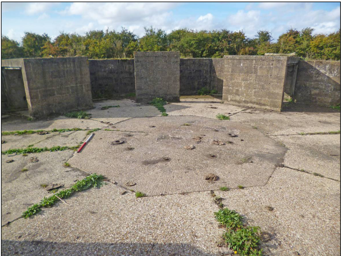
Plate 41: Structure C (gun emplacement), holdfast and ammunition recesses, looking W (photo 2/194).
