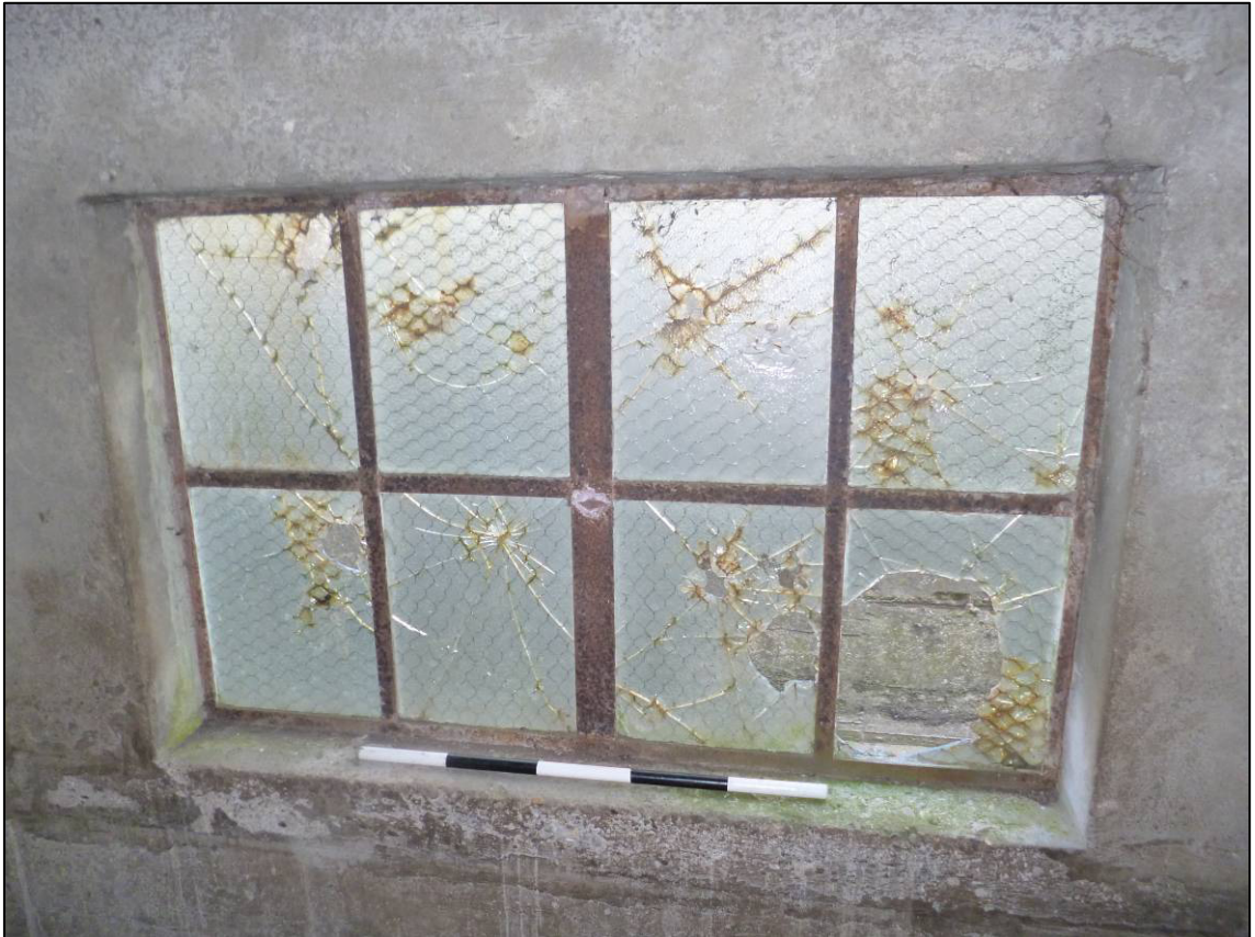
Plate 69: Structure H (magazine), internal window, looking NW (photo 2/222).
