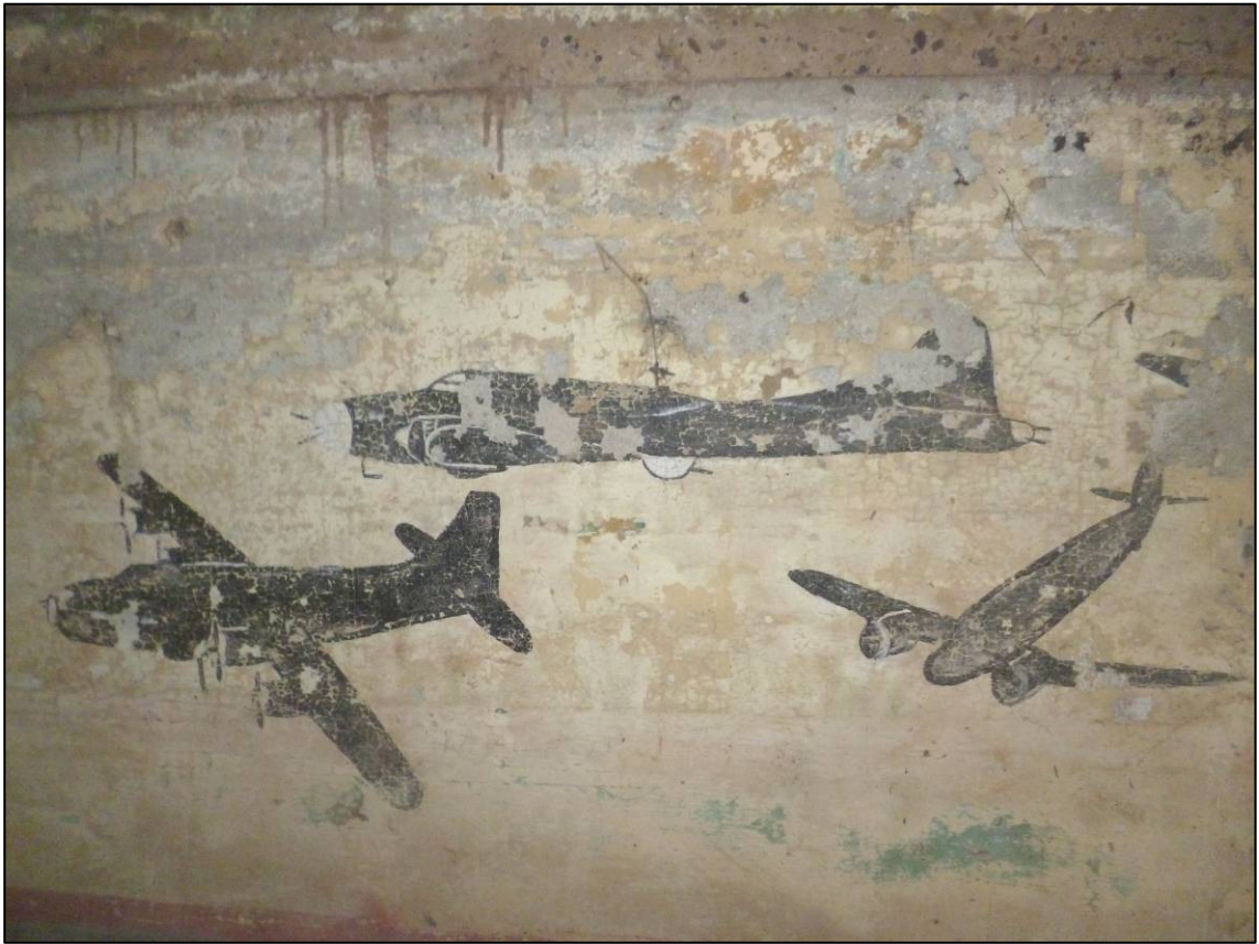
Plate 59: Structure G (gun emplacement), wall paintings to internal south wall of shelter: US Consolidated Privateer (left), B17 Flying Fortress (centre) and Bristol Beaufighter or Douglas C47 Dakota (right) (photo 2/258).
