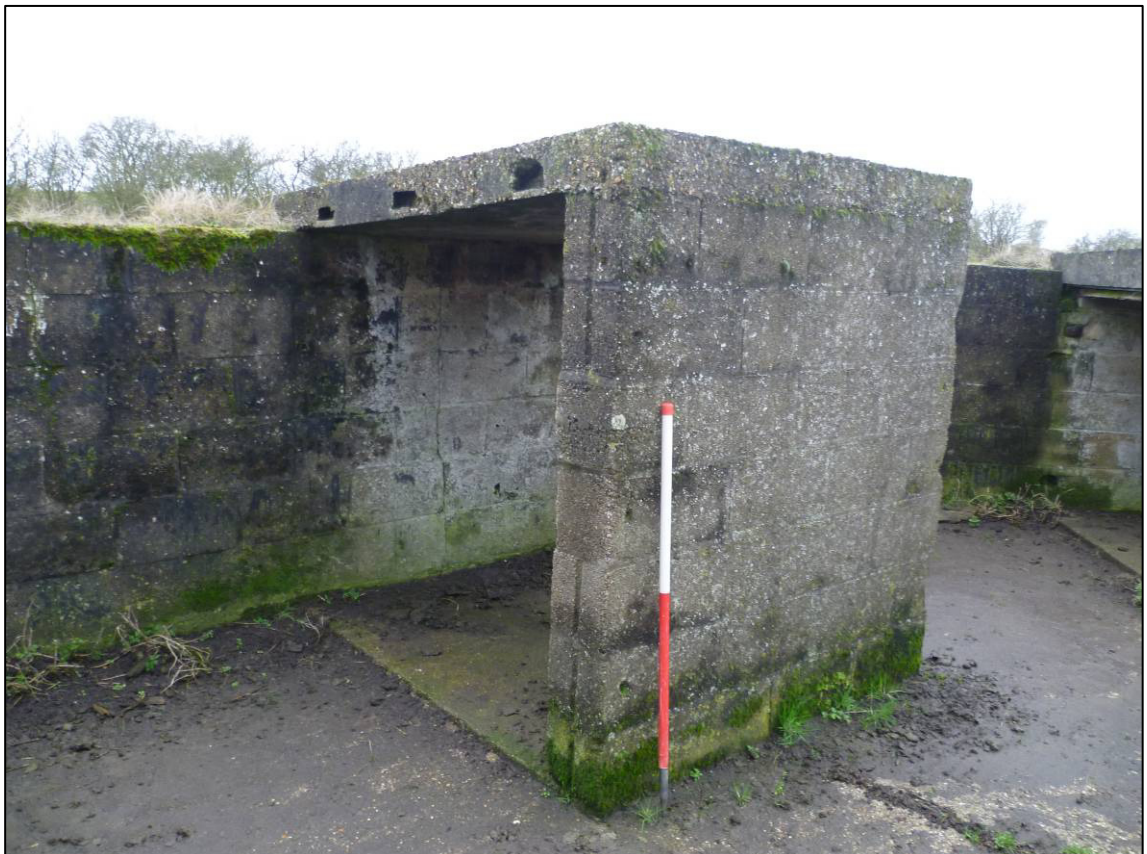
Plate 43: Structure C (gun emplacement), limber gunner recess, looking W (photo 6/725).
