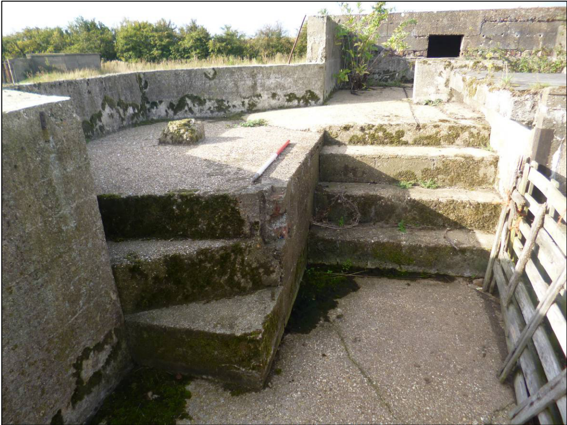
Plate 32: Structure B (command post), spotting telescope platform to left, predictor platform to rear, looking SW (photo 2/147).
