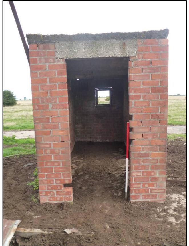
Plate 9: Structure A2 (canteen), west elevation of east entrance, looking E (photo 1/696).
