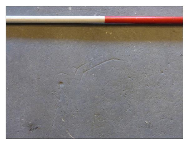
Plate 3: Indentation in lime-ash floor to Room 1 (photo 1/975) (1m scale).
