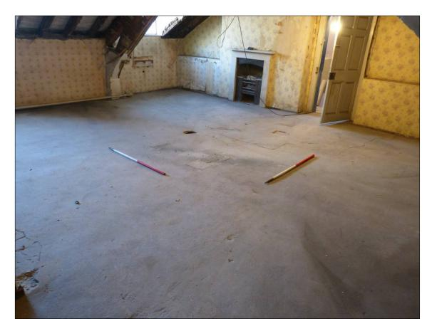
Plate 2: Lime-ash floor to Room 1, looking SE (photo 1/966) (2 x 1m scales).
