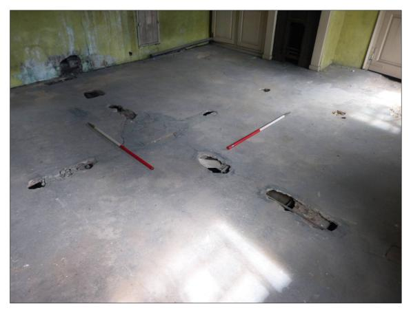
Plate 7: Lime-ash floor to Plant Room, looking SE (photo 1/007) (2 x 1m scales).
