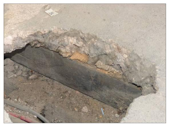
Plate 11: Plant Room, section through lime-ash floor (photo 1/025).
