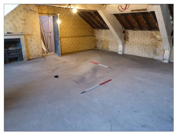
Plate 1: Lime-ash floor to Room 1, looking SW (photo 1/963) (2 x 1m scales).
