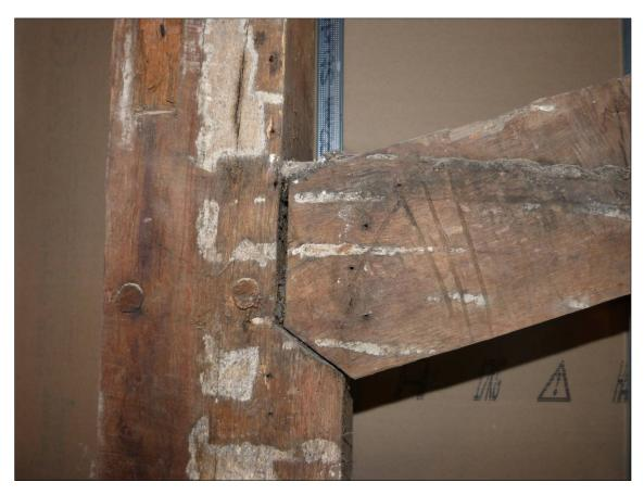
Plate 6: Room 1, carpenter's marks to truss in north wall, looking N (photo 1/994).
