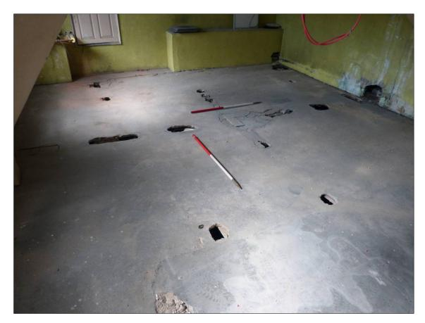
Plate 8: Lime-ash floor to Plant Room, looking N (photo 1/008) (2 x 1m scales).
