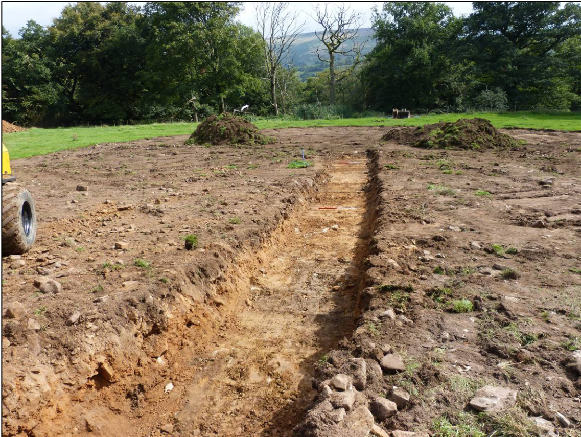
Plate 4: Excavation of exploratory trench, showing subsoil (003), looking SE (photo 2/223).
