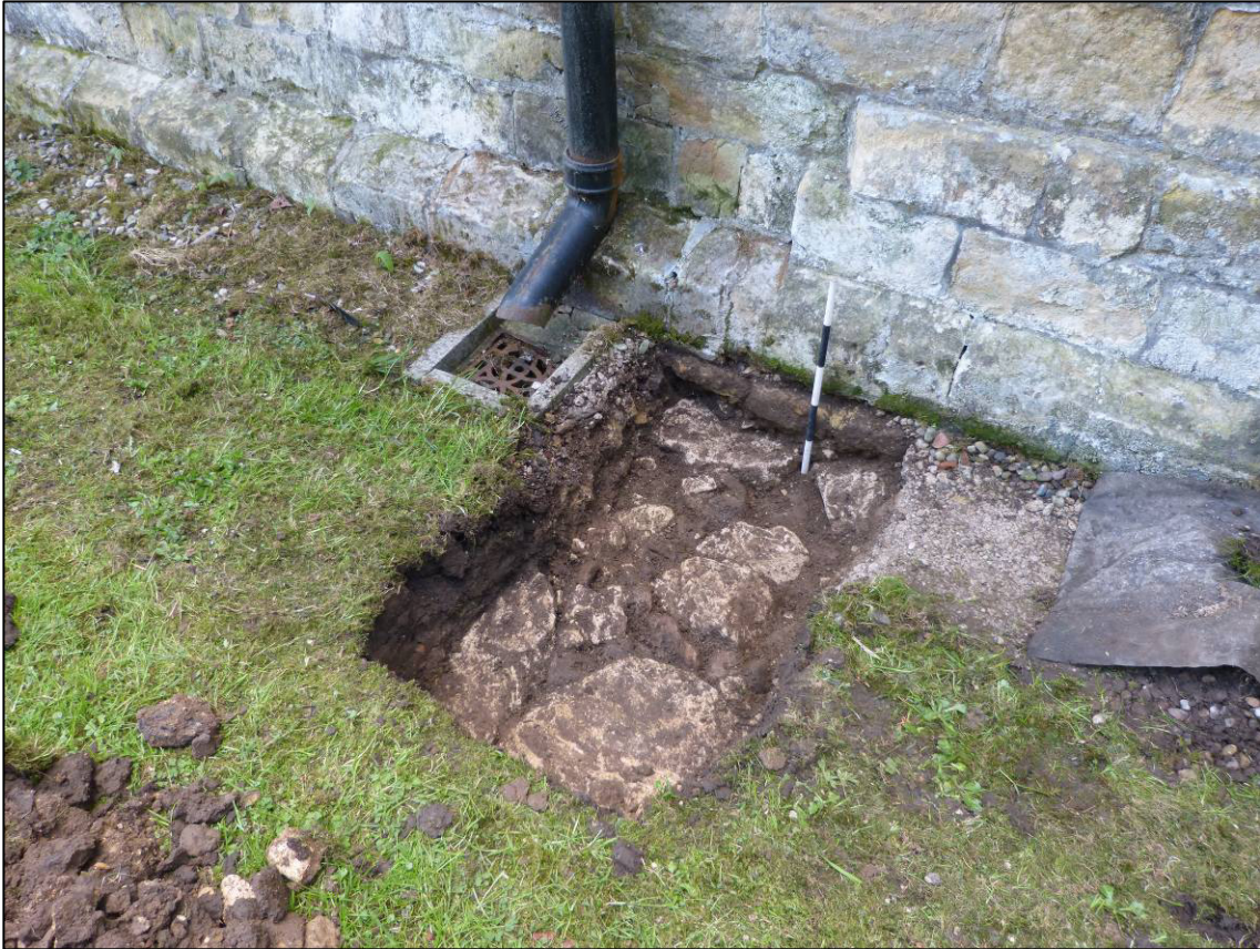
Plate 1: Phase 1 excavation complete in Test Pit 1, showing nave foundations (004), looking SE.
