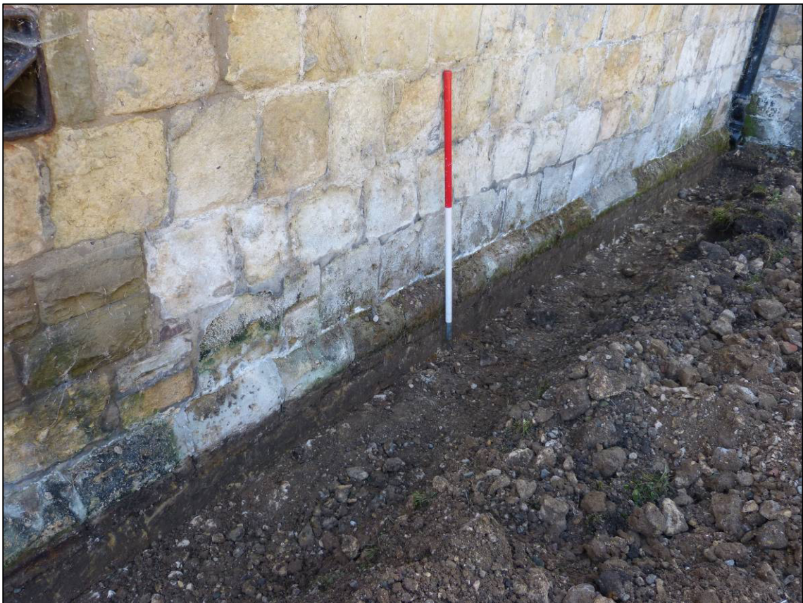
Plate 4: Phase 2 drainage trench excavated along chancel north wall, looking SW.
