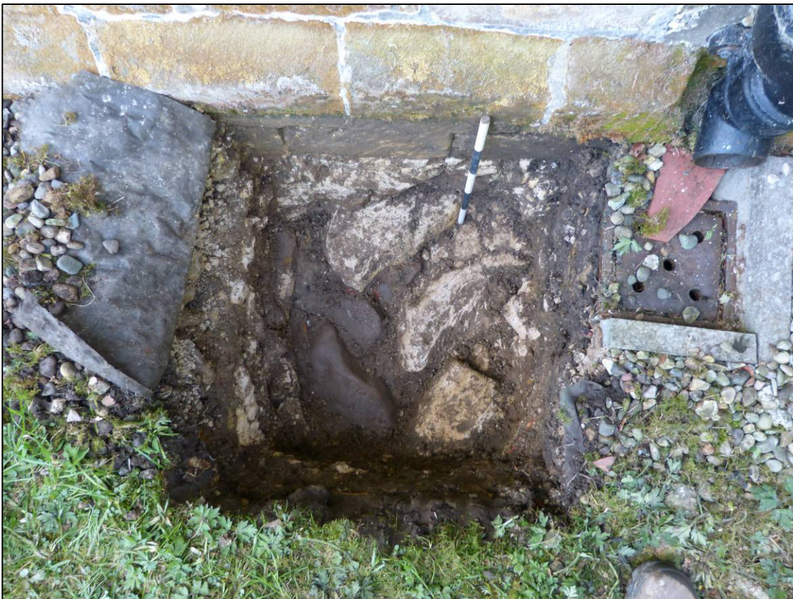
Plate 2: Phase 1 excavation complete in Test Pit 2, showing chancel foundations (006), looking S.
