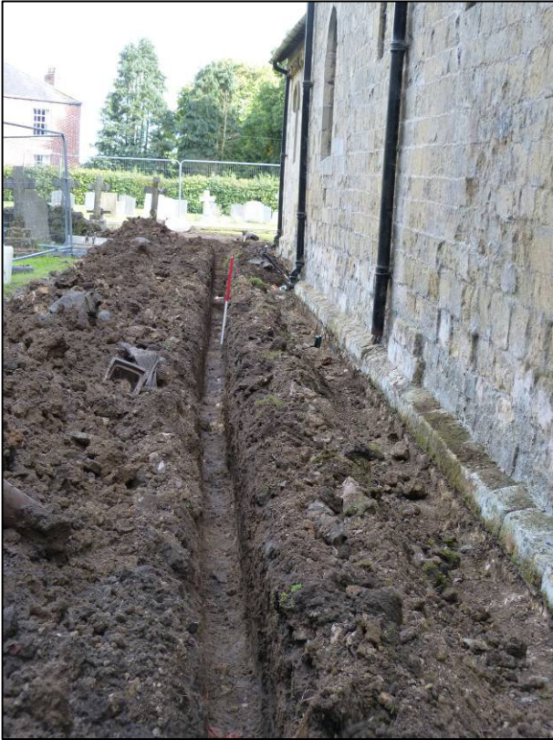
Plate 5: Phase 2 drainage trench excavated north of north church wall, looking E.
