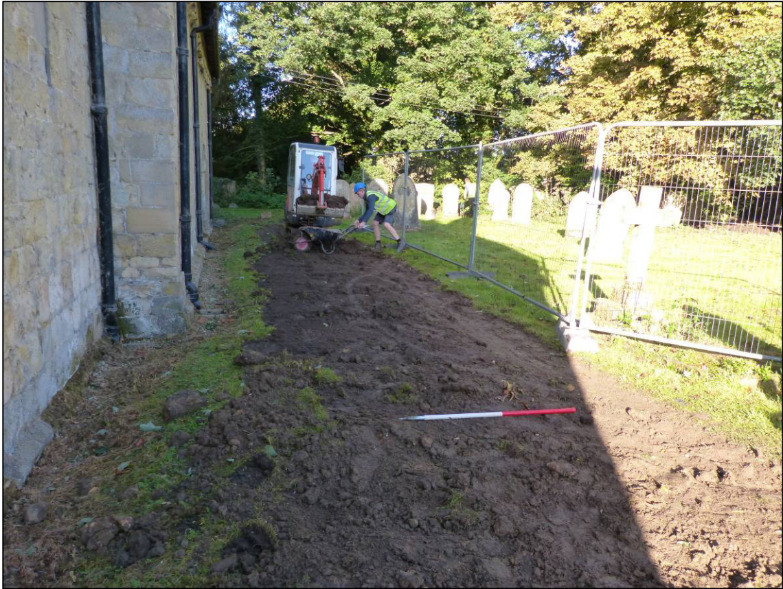
Plate 3: Phase 2 topsoil stripping in progress, looking W.
