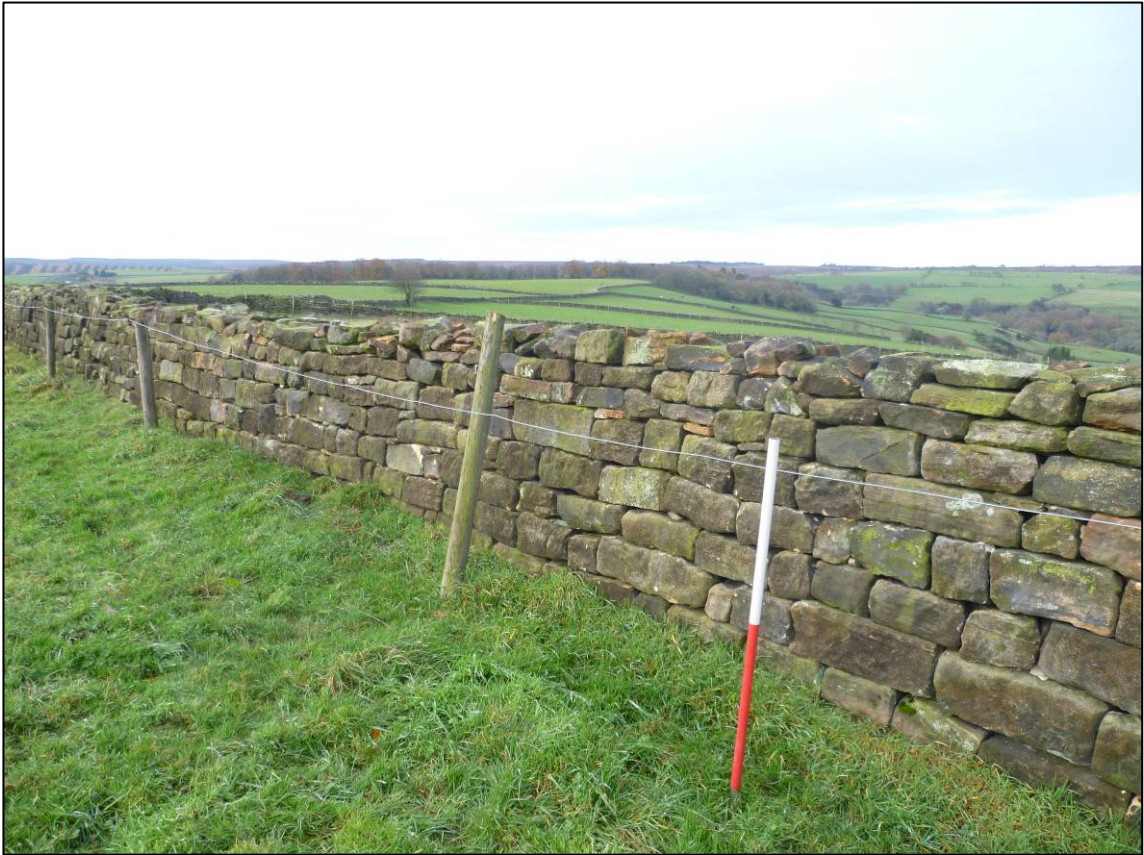
Plate 13: Repaired wall alignment, W of Cross 29, S side, looking W (photo 5/200).
