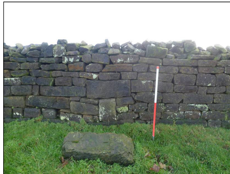
Cross 28 north Top: 1991 photograph 23/S40. Bottom: 8th November 2016 (photo 2/470).
