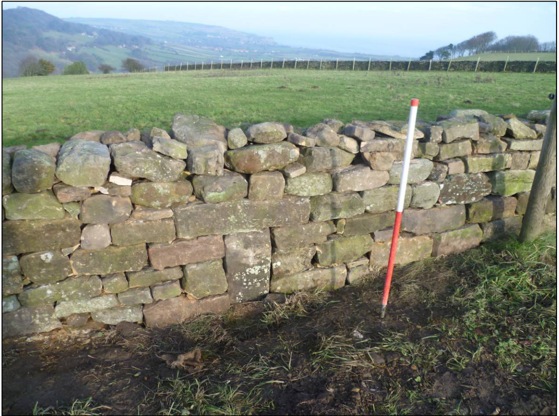
Plate 19: Cross 9, south side, after repairs (photo 3/611).
