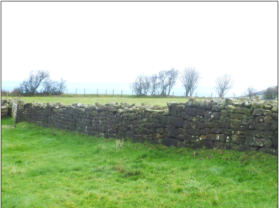
Plate 4: Possible section of original walling between crosses 47 and 48, north side, looking E (photo 2/447).
