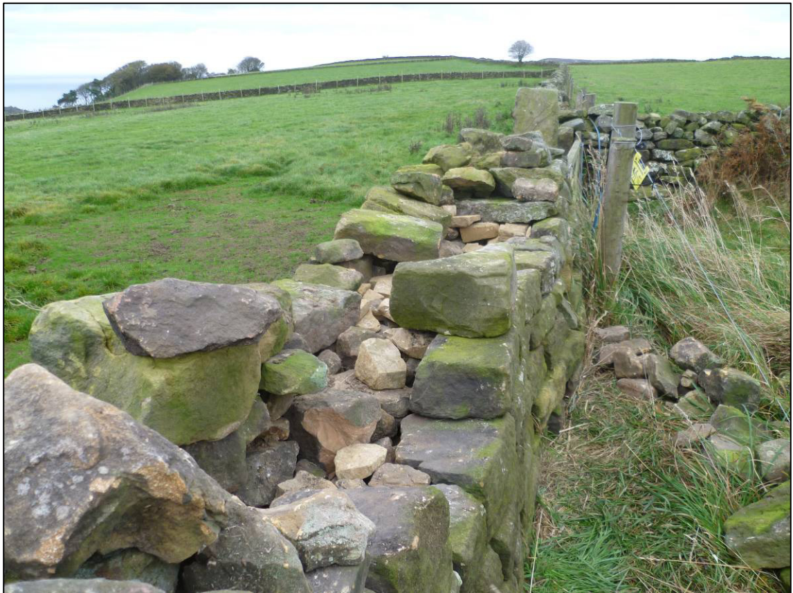
Plate 5: Repairs in progress, east of cross 5, looking E (photo 1/270).
