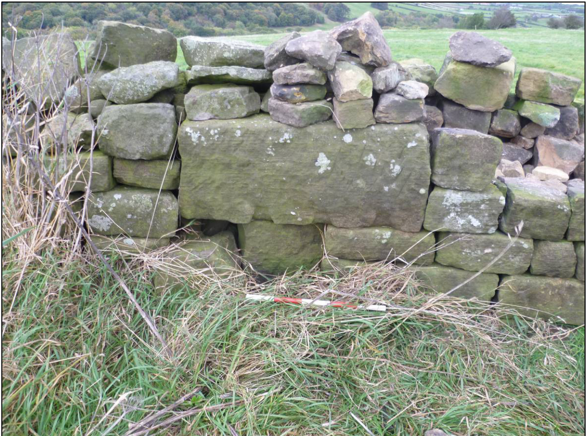
Plate 14: Cross 5, south side, showing plug and feather marks to upper lintel (photo 1/267).
