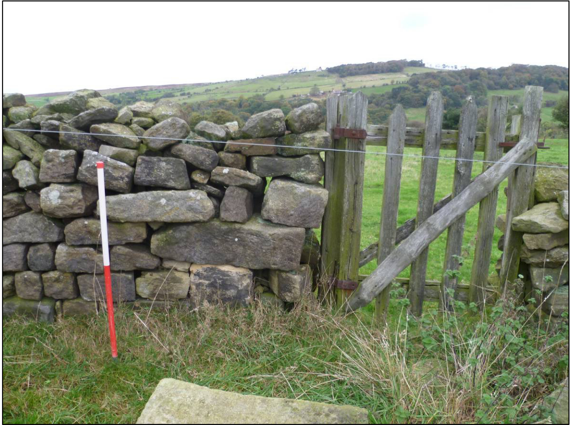
Plate 9: Cross 46 and wooden gate, south side (photo 1/306).
