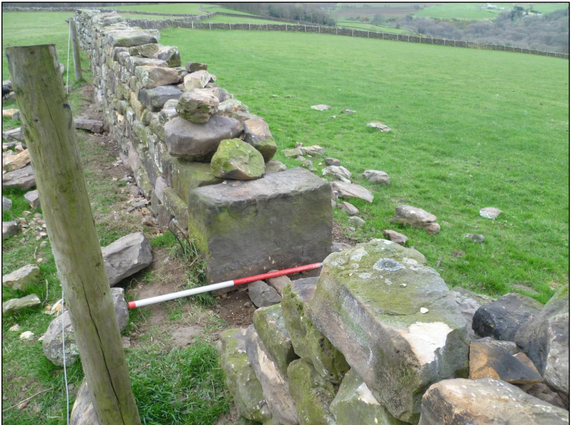
Plate 18: Cross 18, repairs in progress (photo 4/023).
