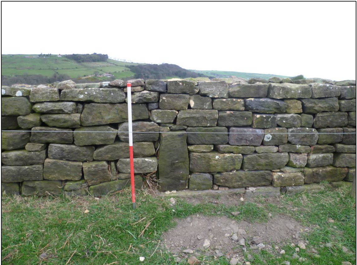
Plate 12: Cross 20, S side, after repairs to adjoining courses (photo 4/031).
