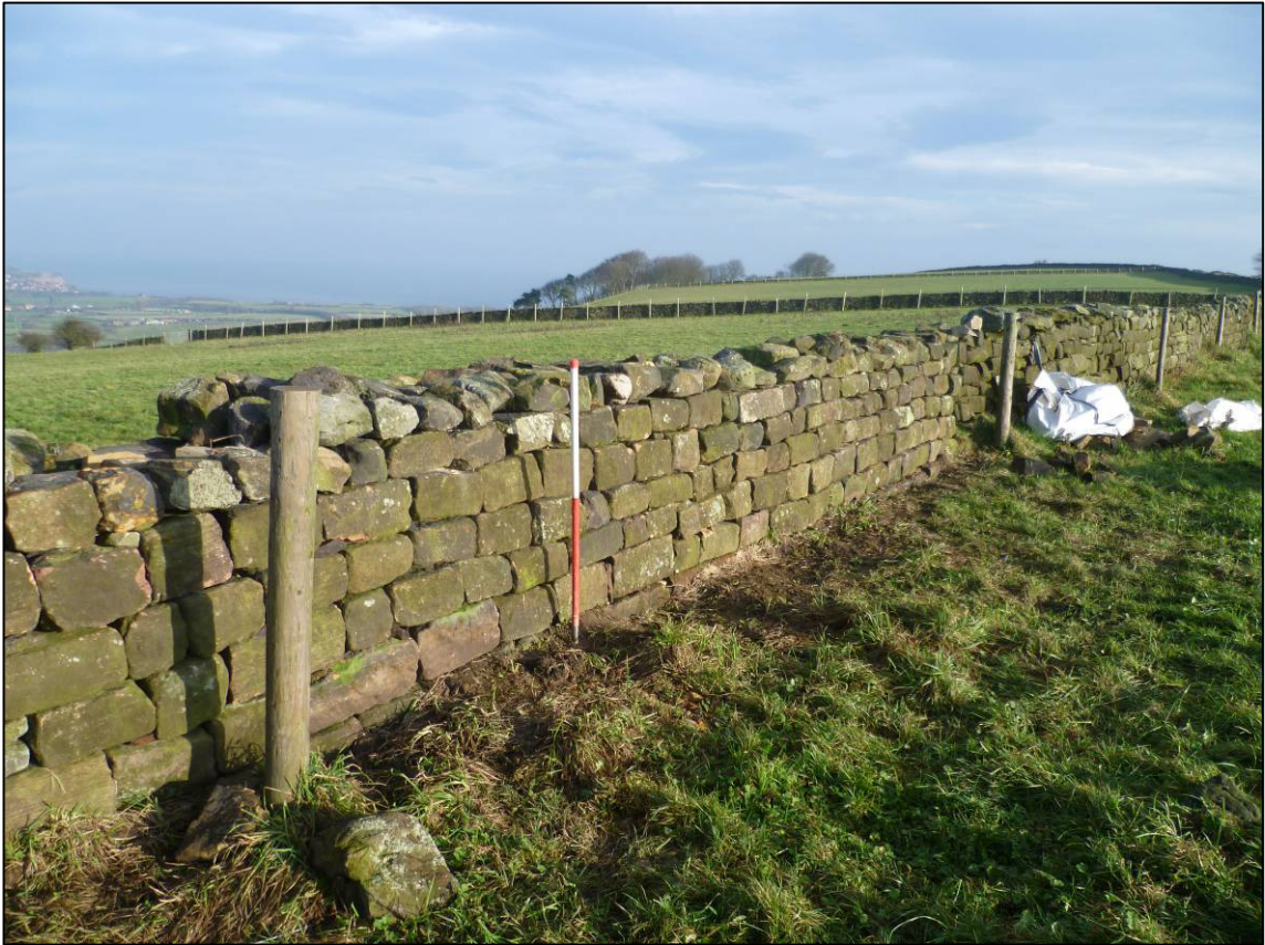
Plate 11: Section of completed repairs, between crosses 8 and 9, south side (photo 3/606).
