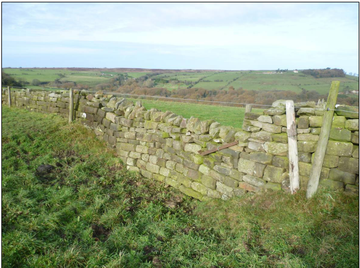
Plate 10: Recently blocked gate between crosses 12 and 13, S side, looking NW (photo 5/222).
