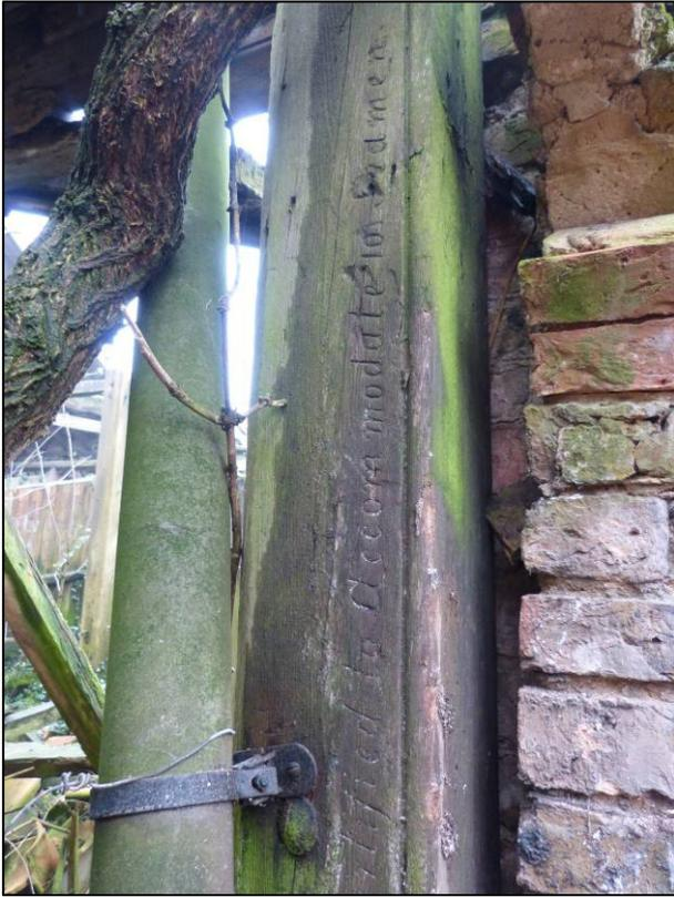
Plate 7: West range (Building D), re-used timber to collapsed doorway in east elevation, looking NW (photo 1/722).
