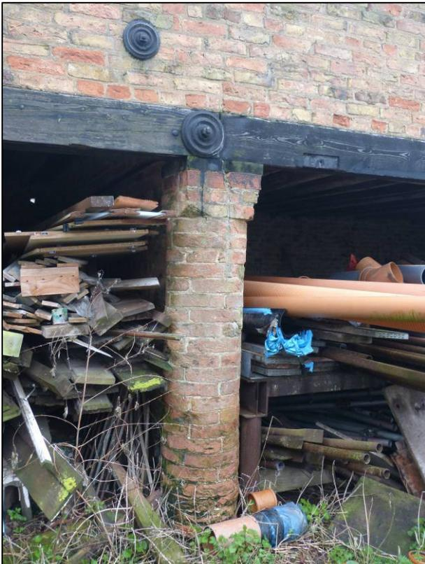
Plate 13: East range (Barn A), east elevation, original circular pillar, looking NW (photo 1/746).
