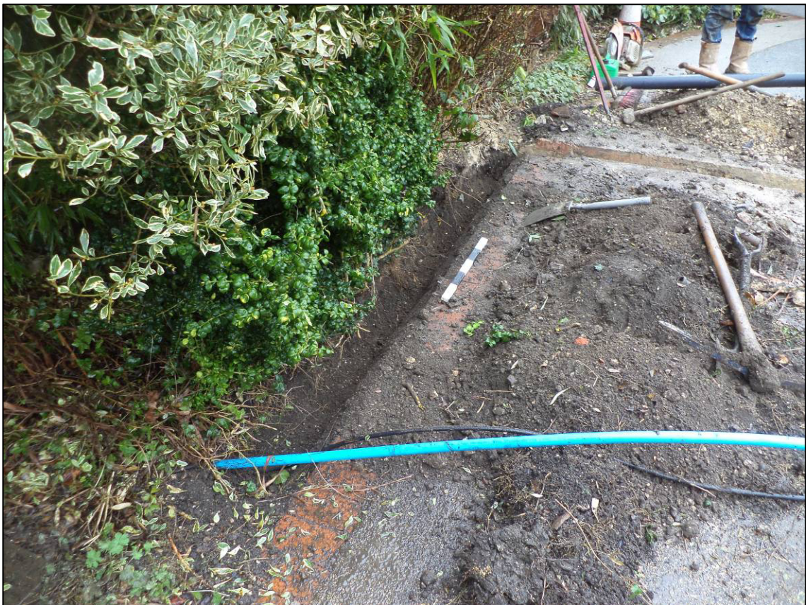
Plate 2: General view of excavated shorter trench arm, looking SW.
