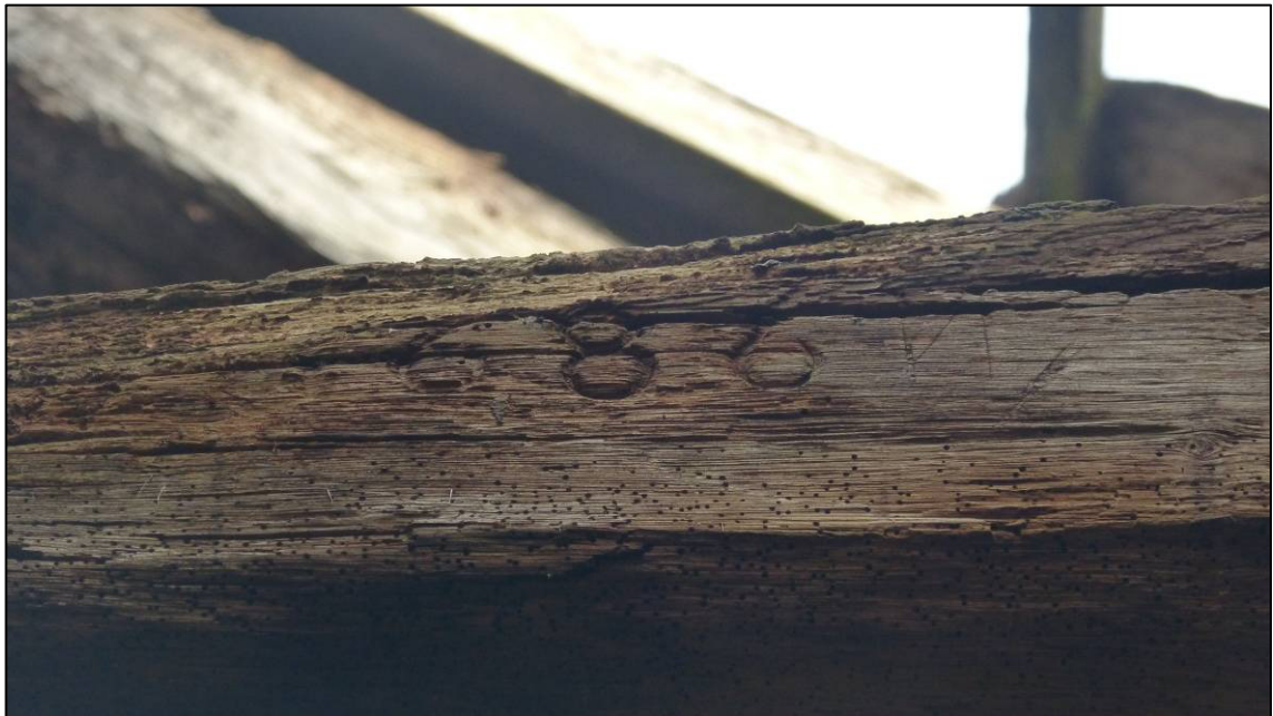
Plate 14: East range, north part, numbers to south face of roof truss tie-beam, looking N (photo 1/389).
