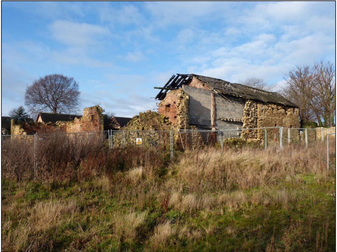
Plate 3: East range, east elevation, looking NW (photo 1/328).
