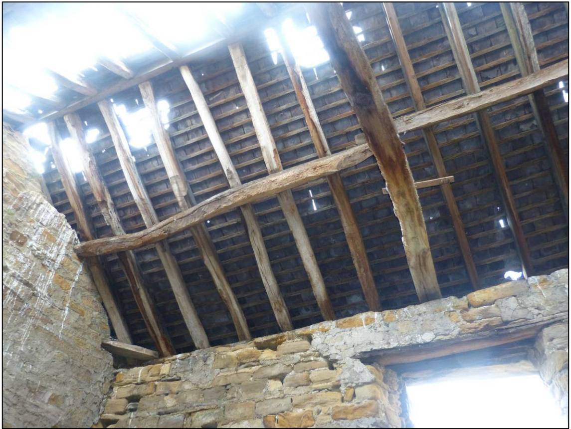
Plate 15: East range, north part, roof structure, looking W (photo 1/382).
