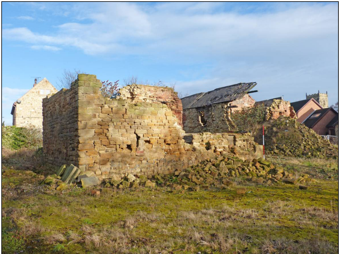
Plate 16: Barn, surviving west end of south elevation, looking NE (photo 1/336).
