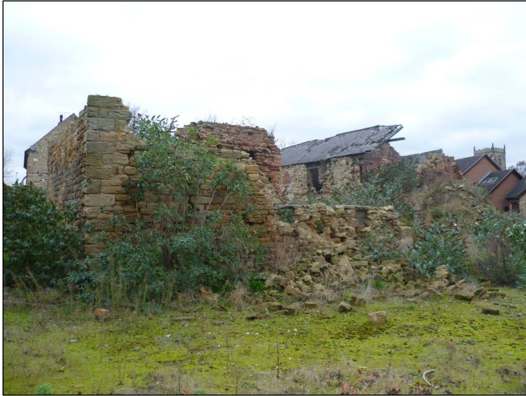
Plate 1: Remains of east-west agricultural range, showing upstanding western half and demolished eastern half, looking NE.
