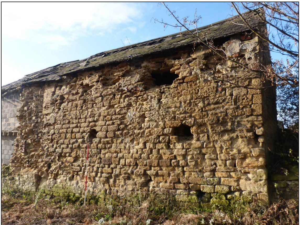
Plate 4: East range, north end of east elevation, looking SW (photo 1/329).
