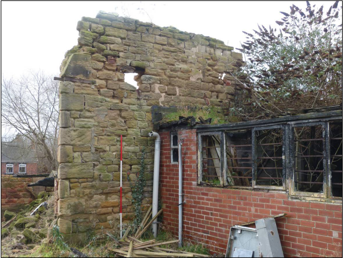
Plate 17: Barn, north elevation showing cart entrance jamb, looking SW (photo 1/396).
