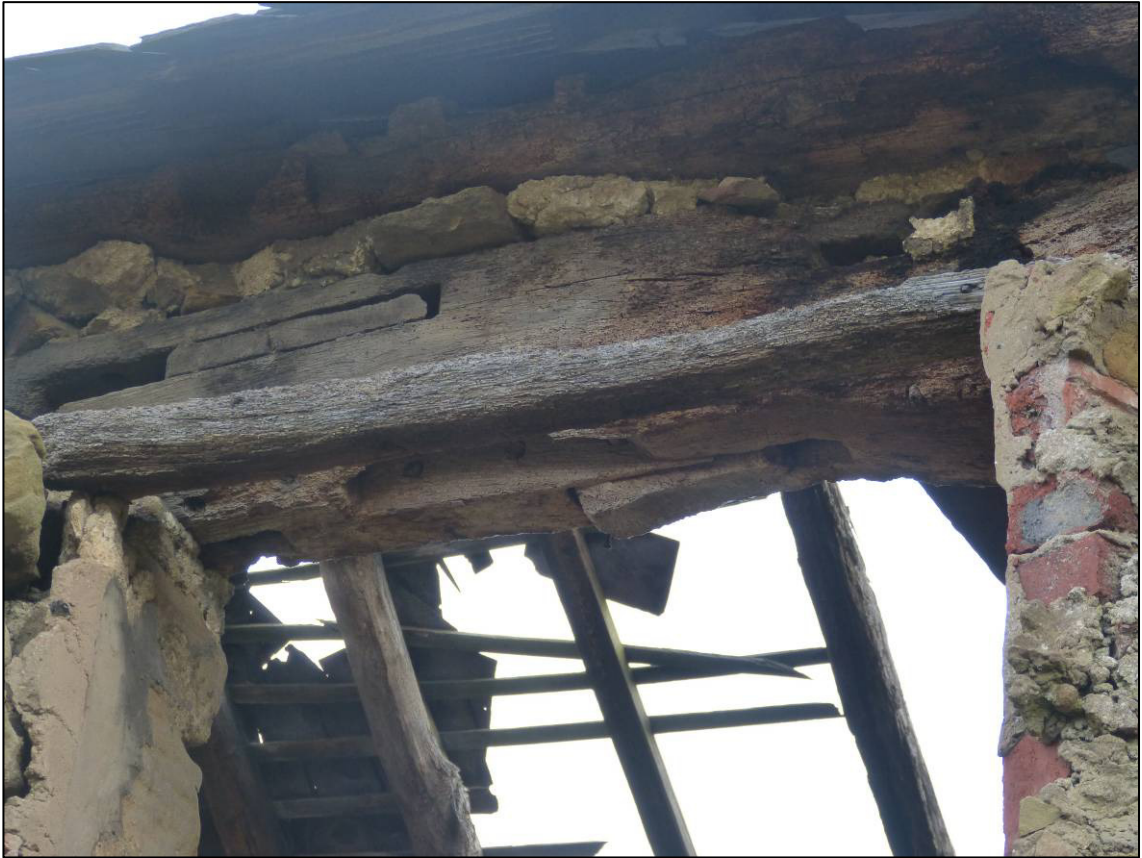
Plate 8: East range, south part, west elevation, re-used wall plate in first floor window, looking NW (photo 1/365).
