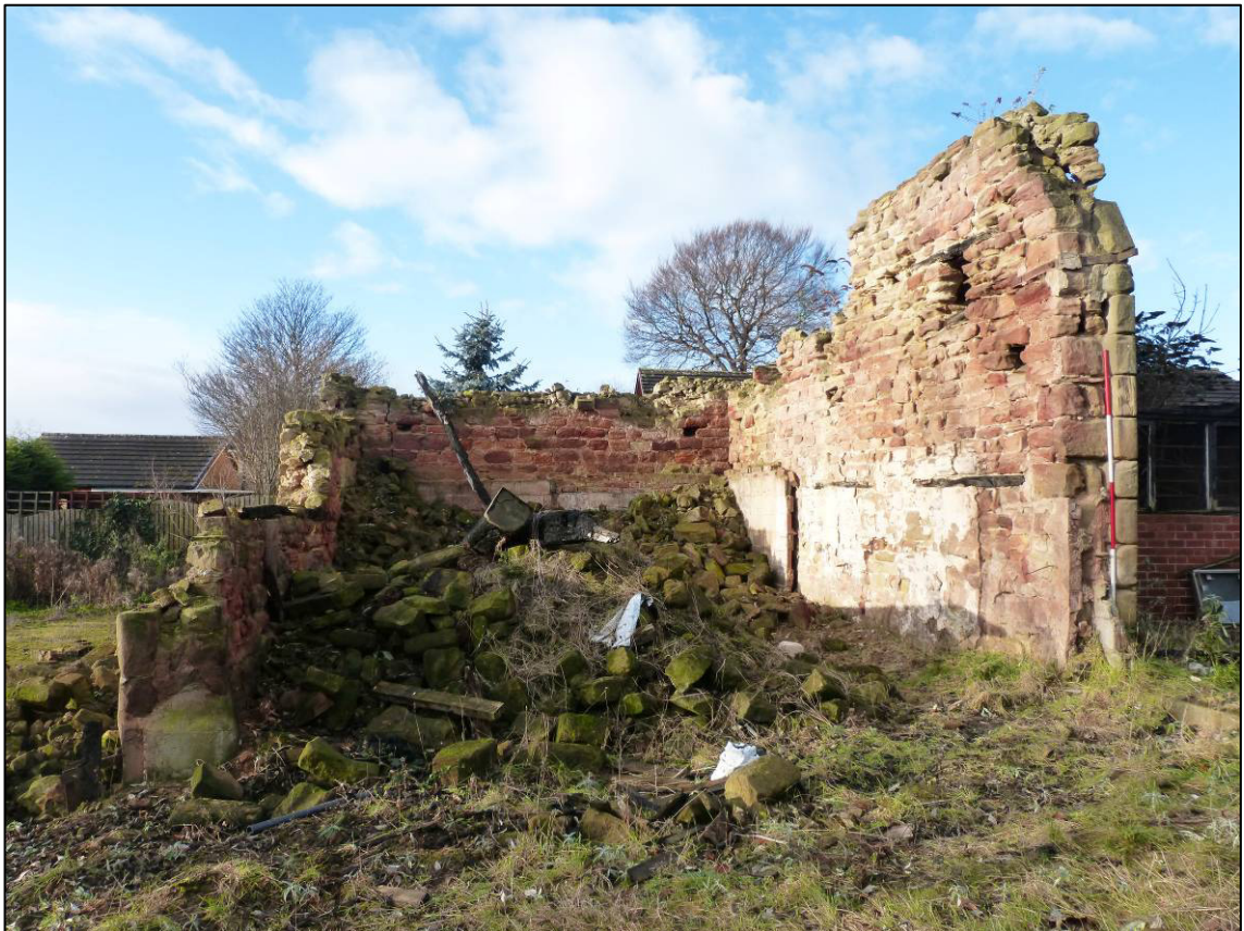
Plate 18: Barn, interior, looking W (photo 1/341).
