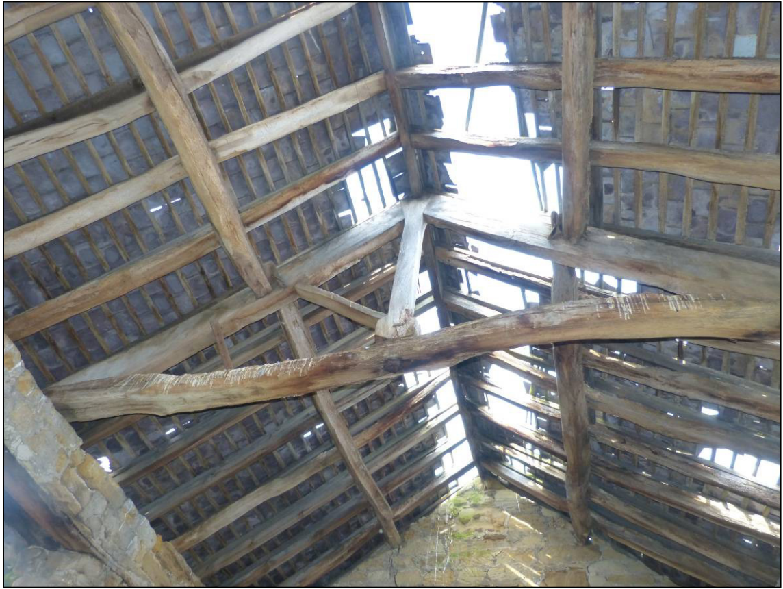
Plate 13: East range, north part, roof structure, looking N (photo 1/386).
