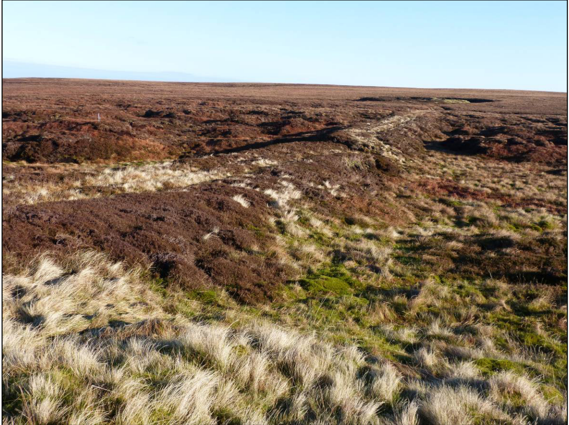
Plate 13: King's Pit Colliery, causeway west of King's Pit High Gin (Site 7), looking SW.
