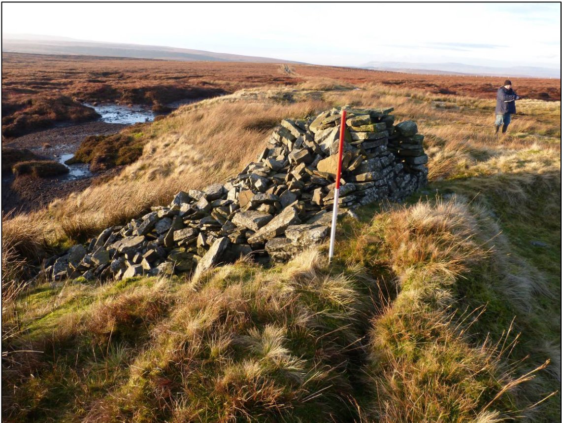
Plate 2: Tan Hill Colliery, south-west pier to whim circle at Tan Hill High Gin (Site 1), looking NE.
