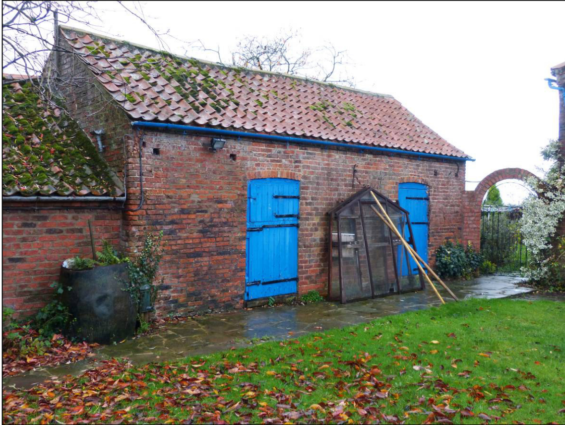
Plate 9: Stables, part of building B, looking SW (photo 1/625).
