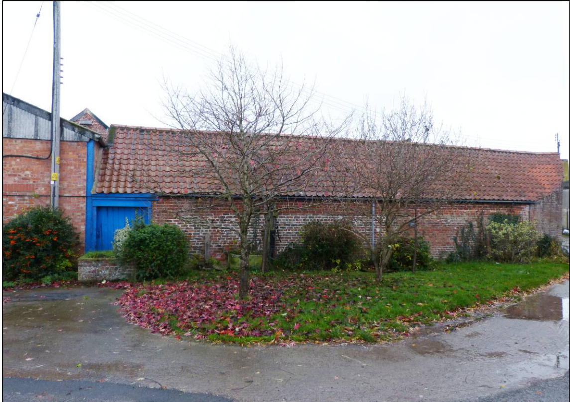
Plate 13: West range (Building E), west elevation, looking E (photo 1/628).
