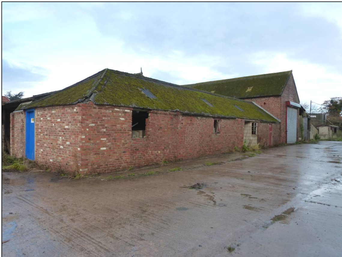
Plate 10: East range (Building D), east elevation, looking NW (photo 1/602).
