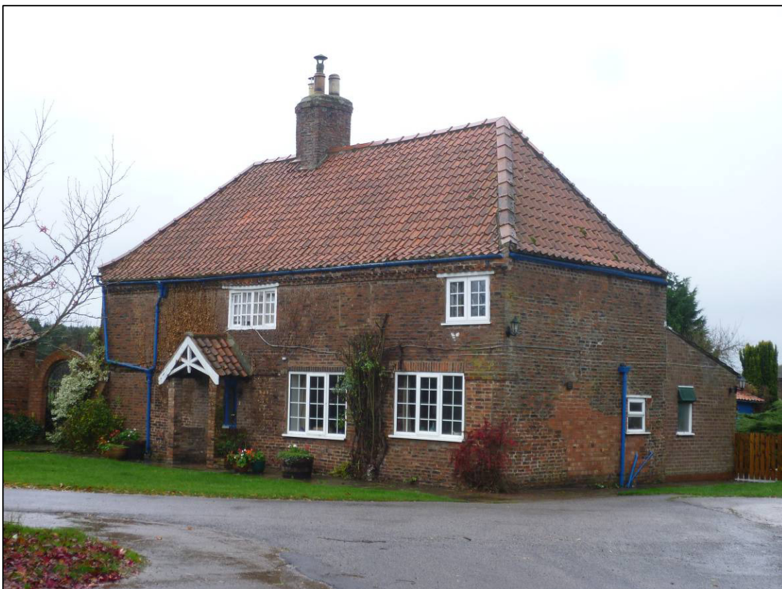
Plate 6: Farmhouse (Building A), north-south range, looking SW (photo 2/018).
