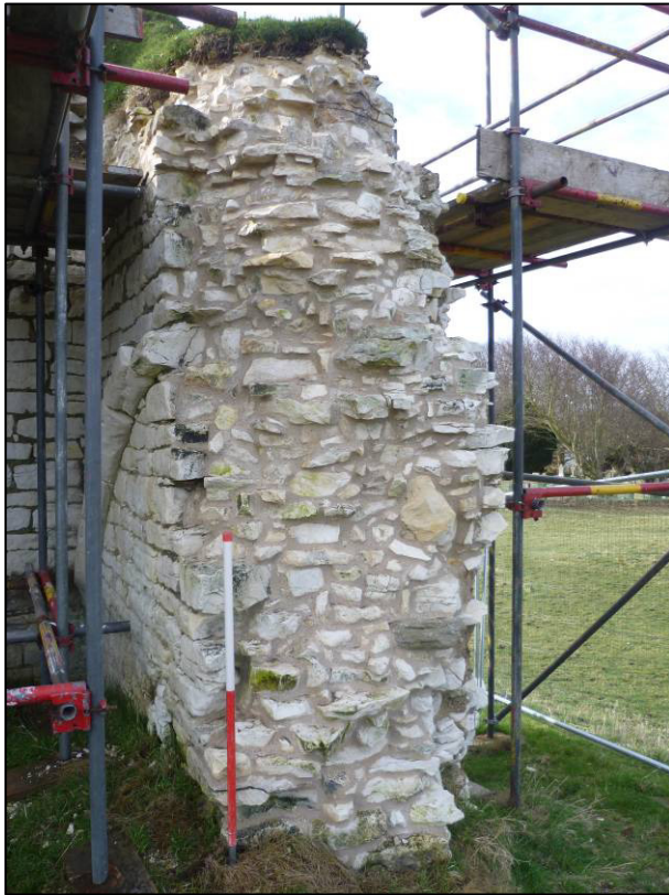
Plate 43: Castle (Site 6G), north end of west wall after repairs and soft capping, looking S (photo 5/835).
