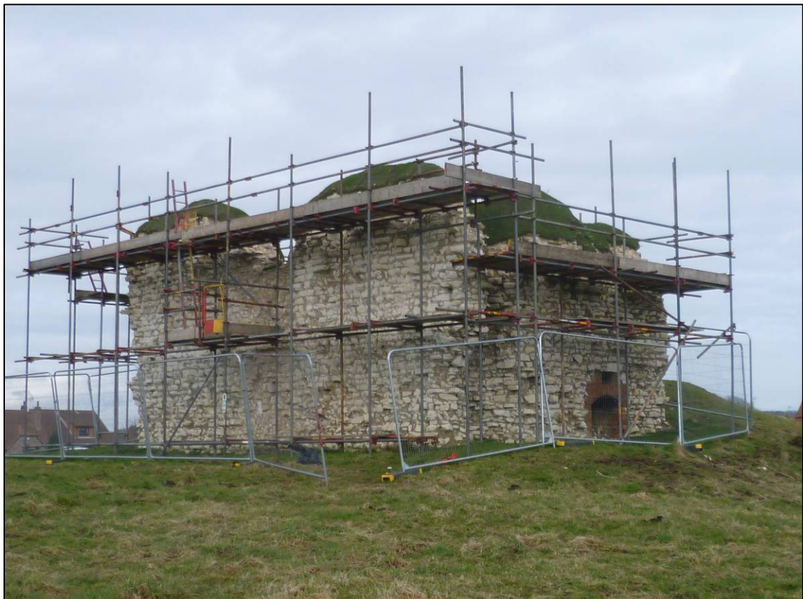
Plate 45: Castle (Site 6G), south and east elevations with soft capping, looking NW (photo 5/874).
