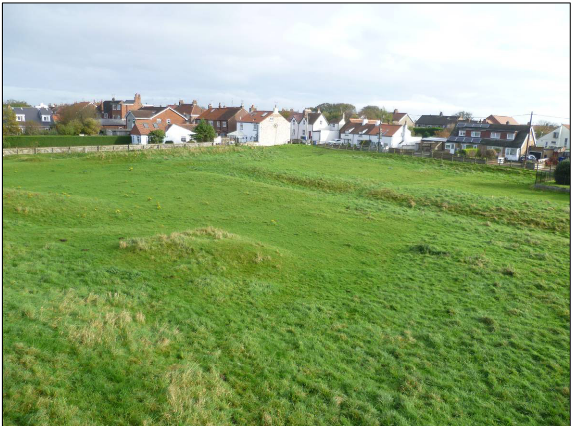
Plate 8: View of gardens area (Site 5) from top of castle, looking NE (photo 2/969).
