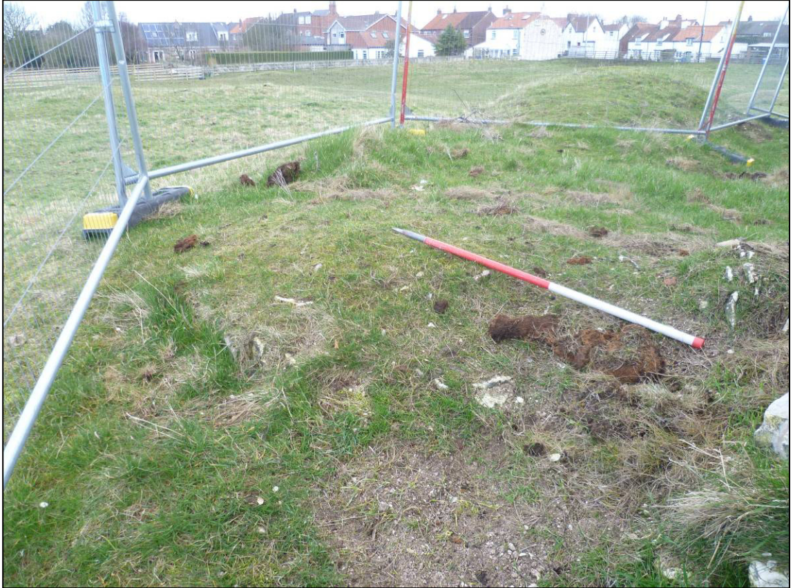
Plate 28: Castle (Site 6G), remains of former buttress at north-west corner, looking NE (photo 5/809).
