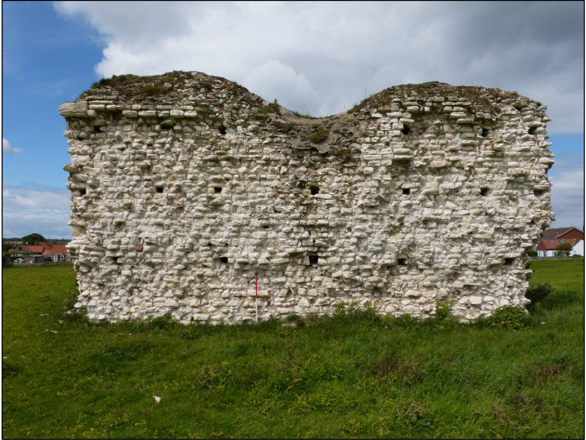
Plate 31: Castle (Site 6G), south external elevation, looking N (photo 1/804).
