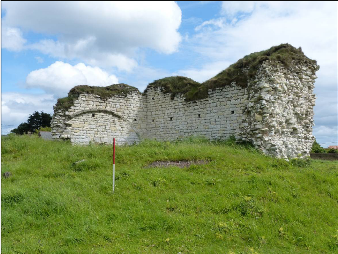
Plate 25: Castle (Site 6G), internal elevations, looking SE (photo 1/815).
