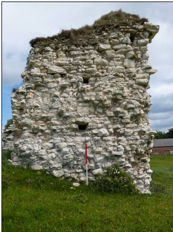
Plate 26: Castle (Site 6G), west external elevation, looking E (photo 1/803).
