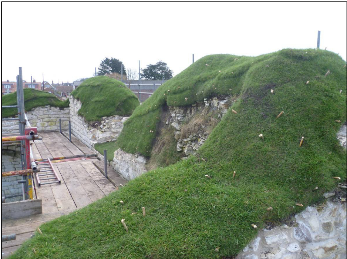
Plate 42: Castle (Site 6G), general view of soft capping, looking SE (photo 5/822).
