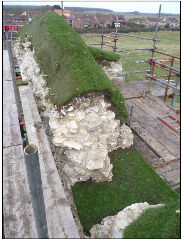
Plate 44: Castle (Site 6G), south elevation wall top, window opening after soft capping, looking E (photo 5/817).
