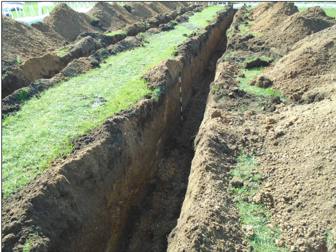
Plate 13: General view of excavated soakaway trenches, looking SW.
