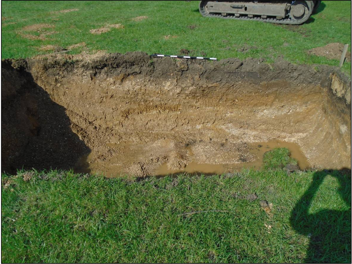
Plate 11: Excavated septic tank, looking S.
