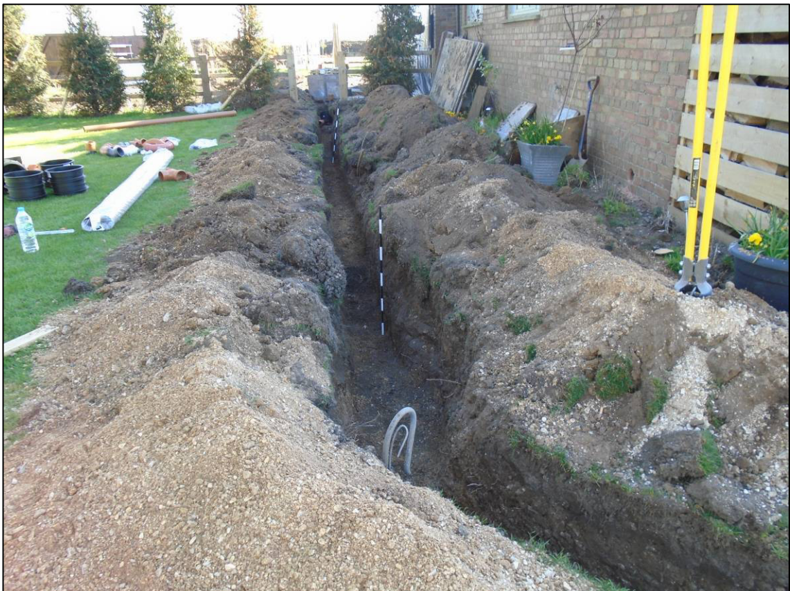
Plate 12: Excavated drainage trench along east side of barn, looking S.
