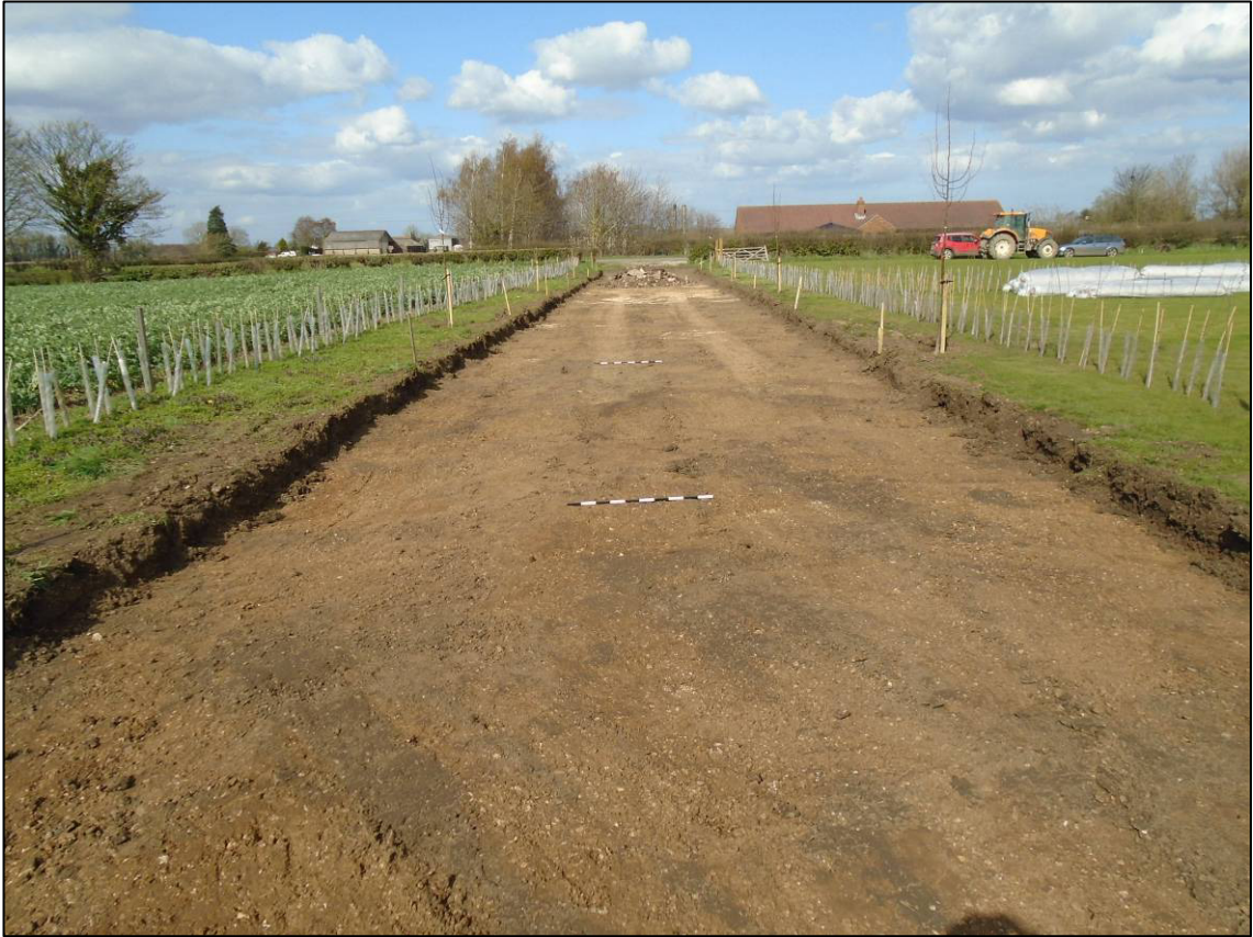
Plate 1: General view of north-south section of stripped access road, looking N.
