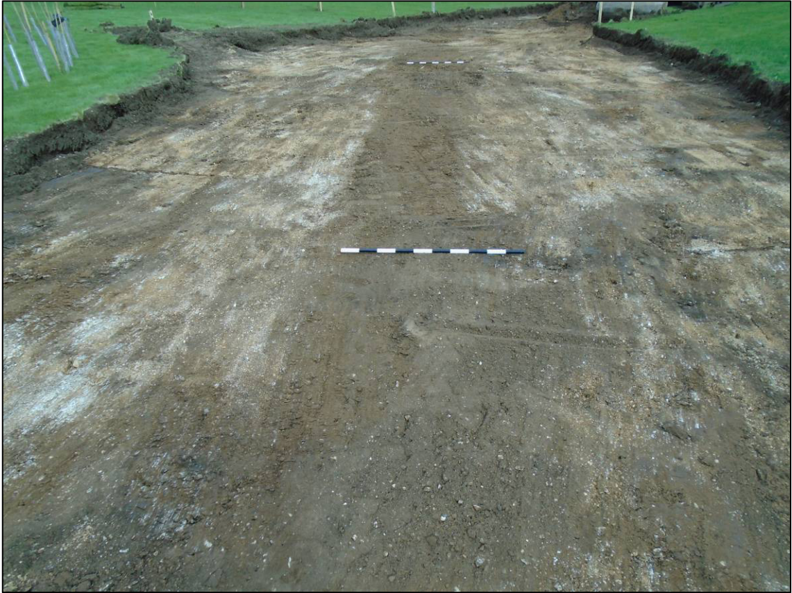
Plate 5: Exposure of hedge line [110] in southern car park area, prior to excavation, looking NE.
