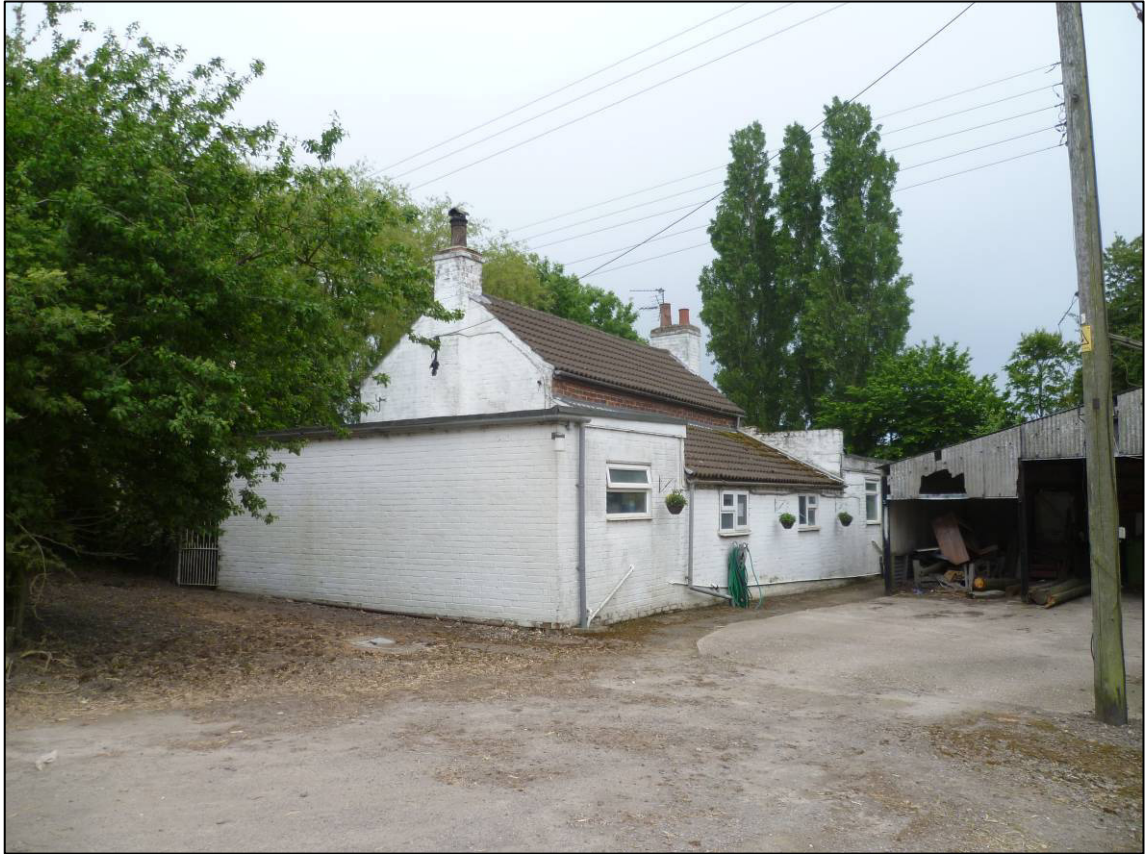
Plate 1: View of rear of former farmhouse, looking SE.
