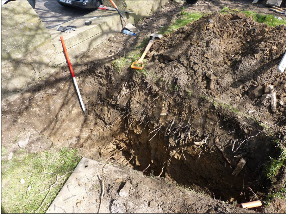
Plate 3: Inspection chamber, adjacent to churchyard wall, looking E.
