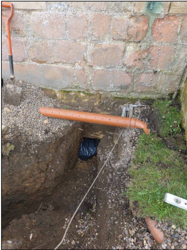
Plate 4: Tower footings in drainage trench, looking E.
