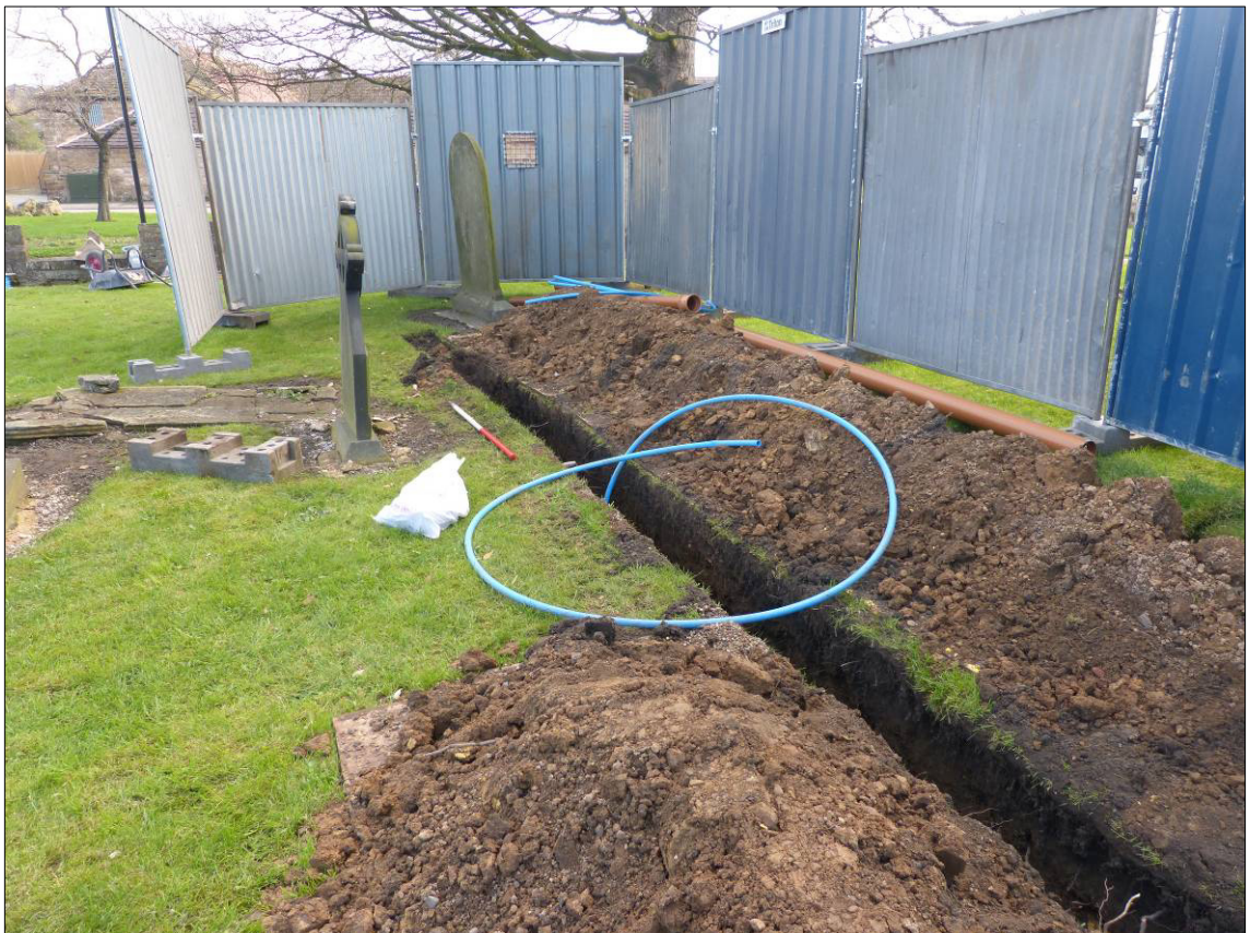
Plate 2: General view of drainage trench, central section, looking NE.
