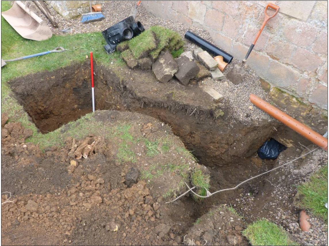
Plate 1: Drainage trench and inspection chamber adjacent to tower, looking NE.
