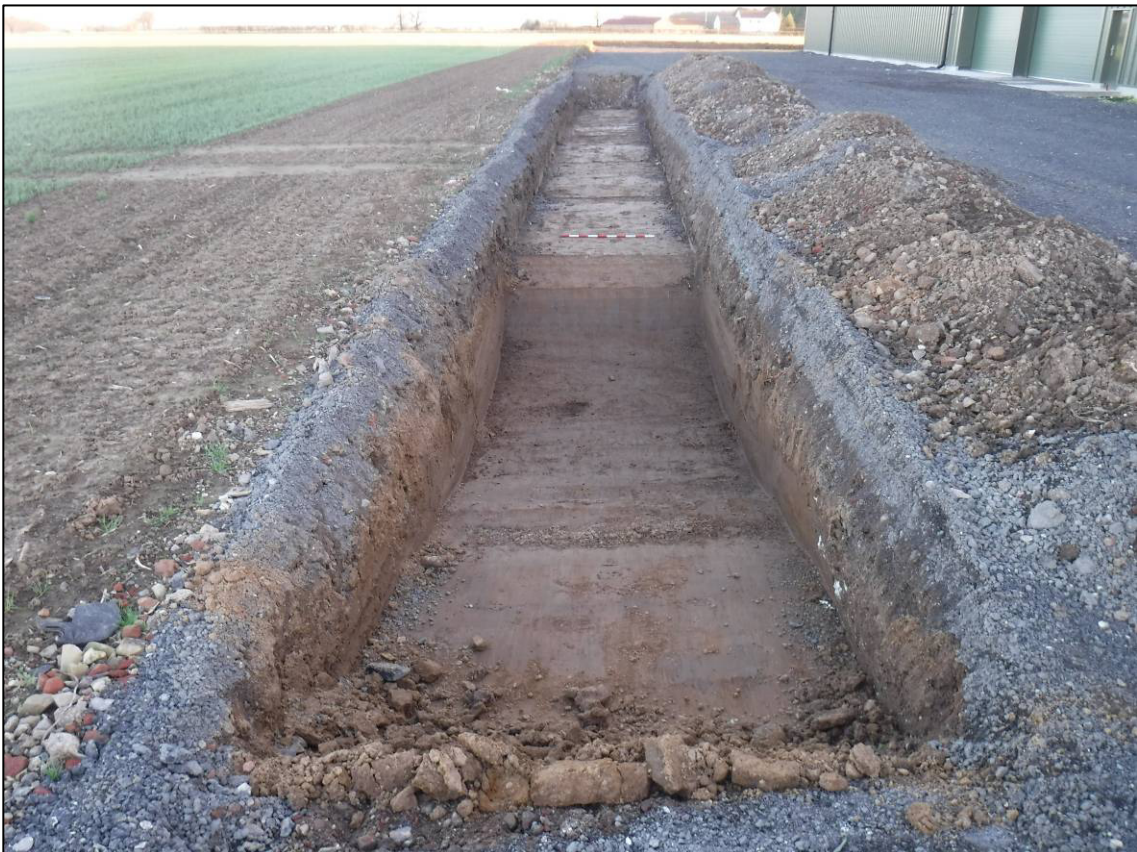
Plate 6: Trench 2, after excavation, showing deeper sondage at NW end, looking SE.
