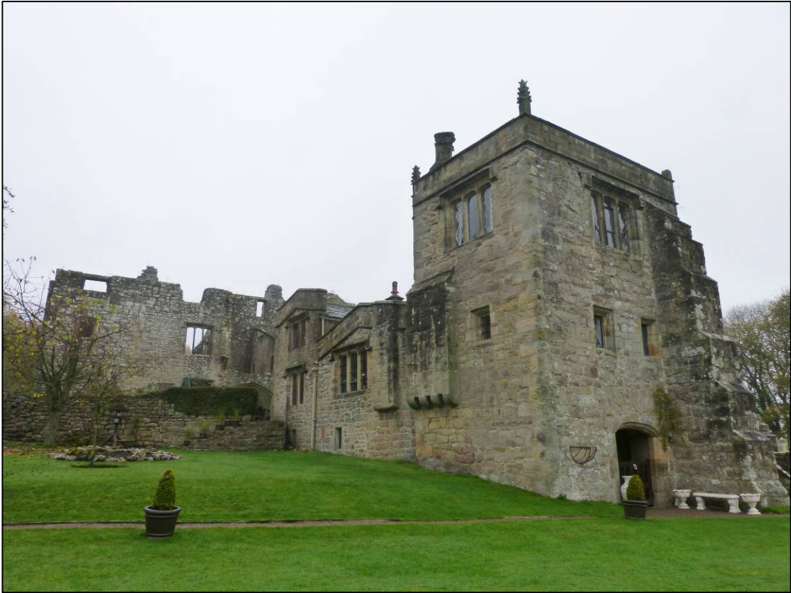
Plate 1: Priest's House and Chapel complex, with Barden Tower to rear, looking NE (November 2015).
