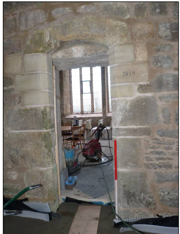
Plate 13: North face of unblocked and raised doorway in north wall of chapel, looking S (photo 5/268).
