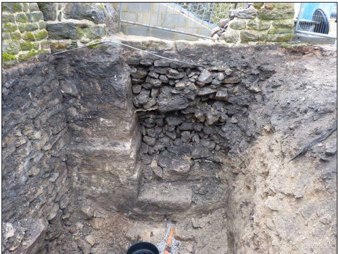
Plate 11: Re-excavation of 2015-16 area, showing buttress to north-east corner of chapel, looking W (photo 5/270).
