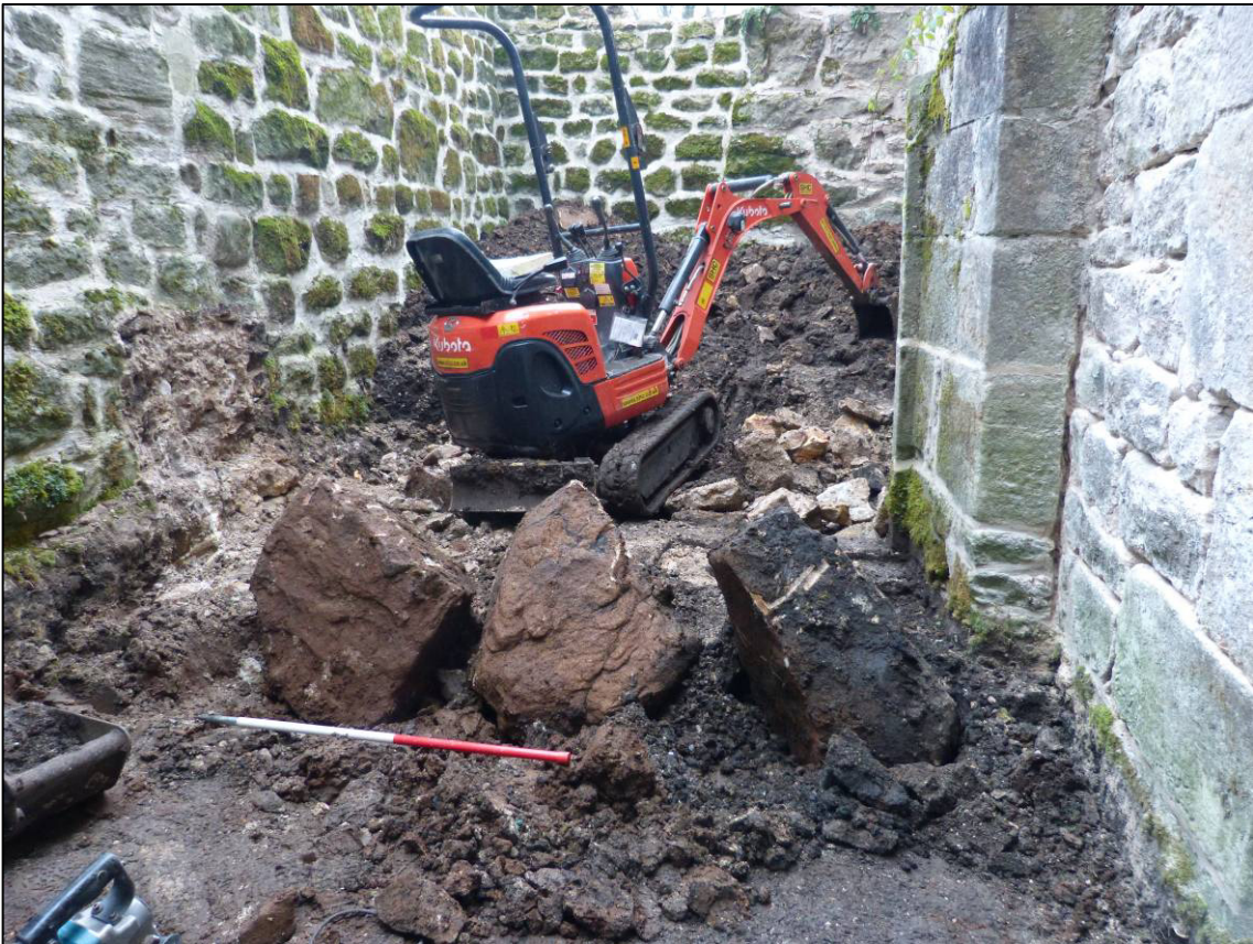
Plate 7: Grubbed up footings of cross-wall in sunken area, looking NE (photo 2/821).
