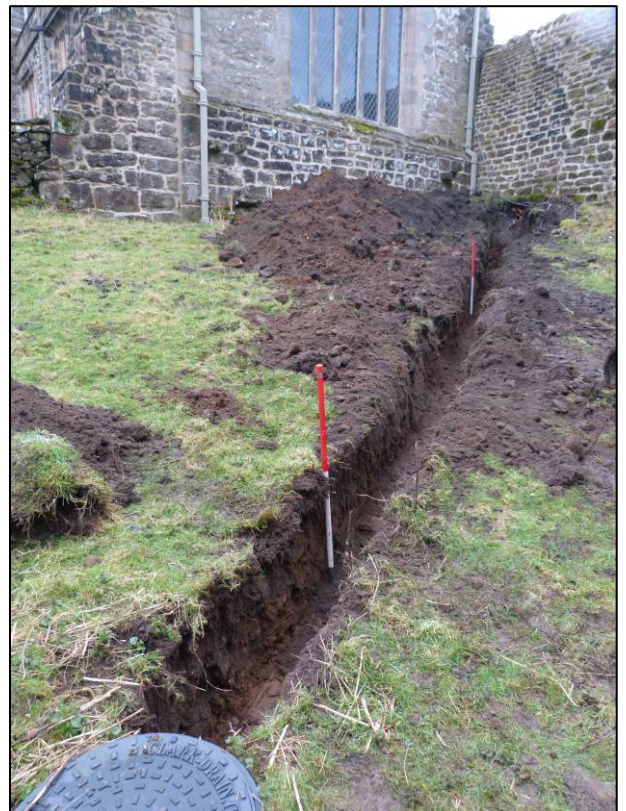
Plate 16: Main drainage trench (Trench 1), looking NW (photo 5/266).
