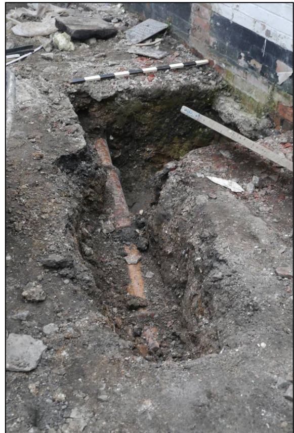
Plate 8: Trench 1, salt-glazed drain (118) and cut [117], looking E.
