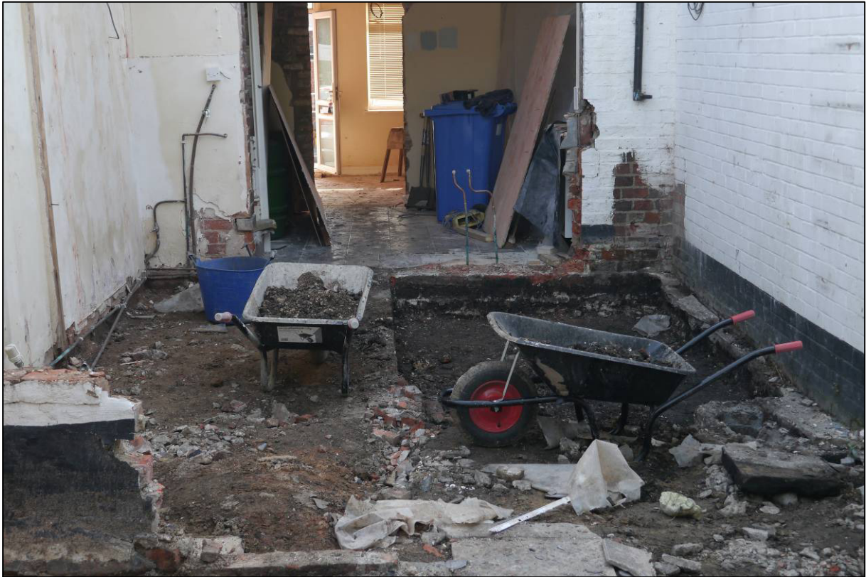
Plate 1: Initial stages of site construction, showing Trench 2, looking E.
