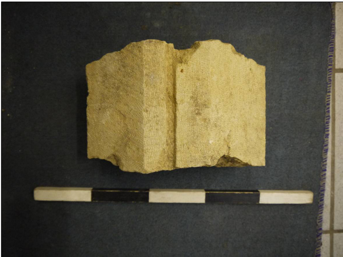
Plate 12: Ashlar M4 (mullion from Trench 1, 119), showing internal and external chamfers and vertical grooves for glazing bars.
