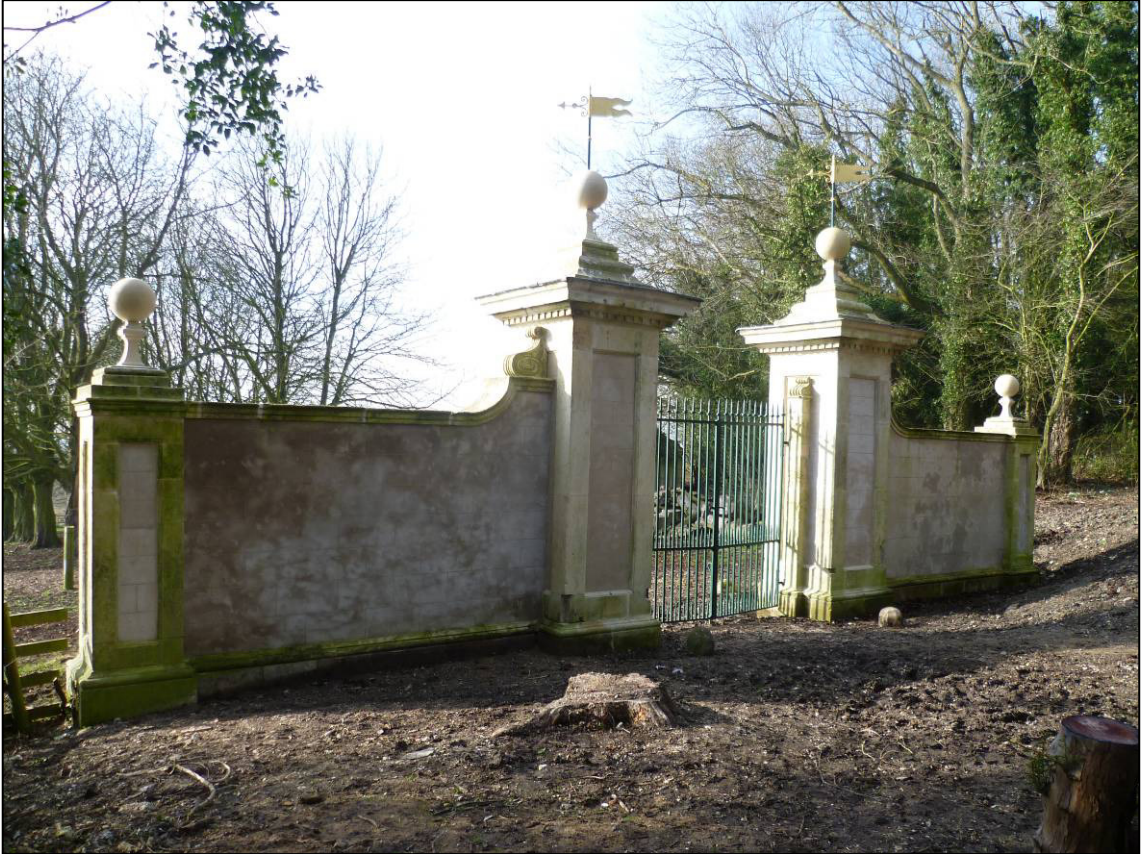
Plate 21: Completed rebuilding and restoration work, looking S (photo 5/148).
