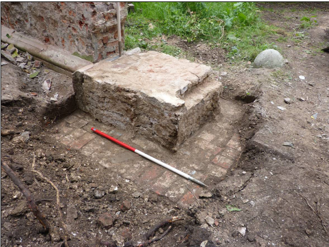
Plate 12: Exposure of pier base and brick platform to Pier 3, looking S (photo 2/042).
