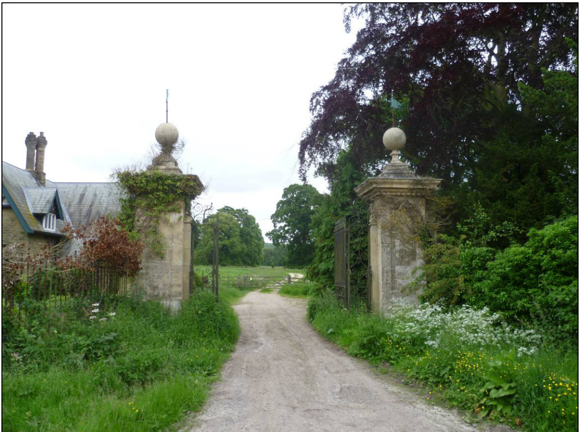
Plate 8: The Lodge gateway, looking E (June 2018).
