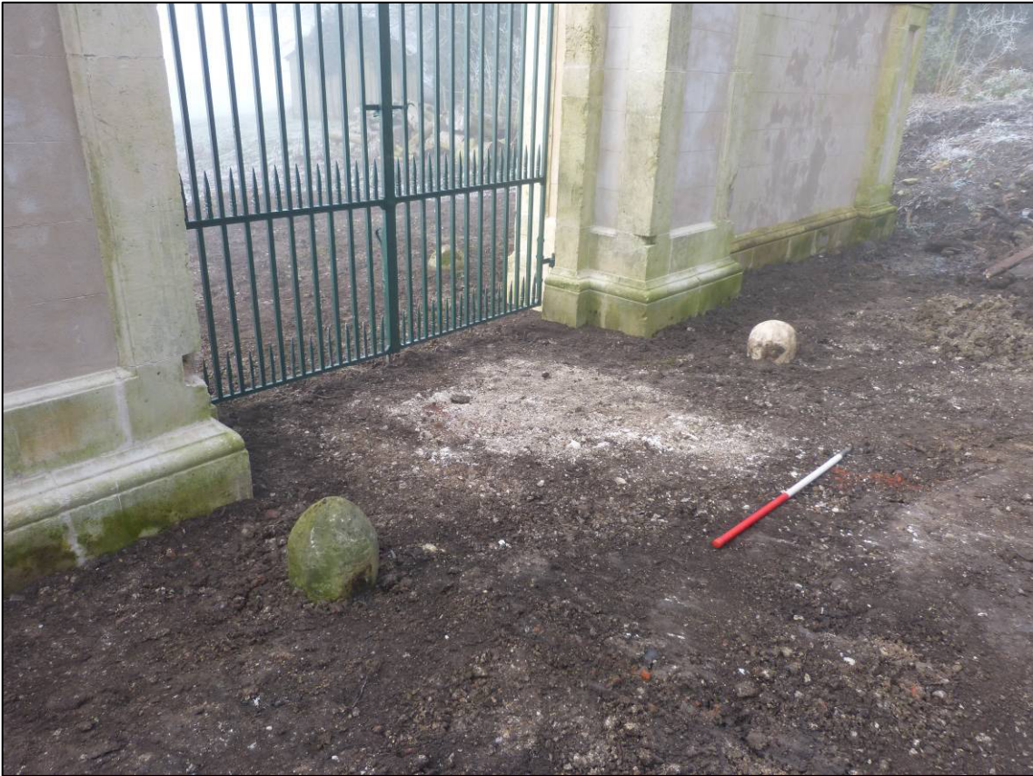
Plate 19: Chalk surface (003) in gateway, with re-instated wheel stones, looking W (photo 4/973).
