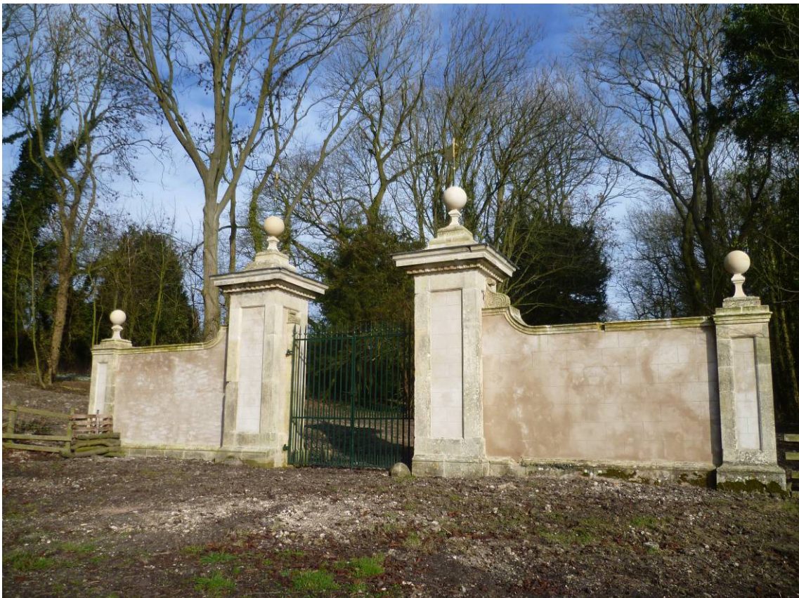
Plate 20: Completed rebuilding and restoration work, looking N (photo 5/146).
