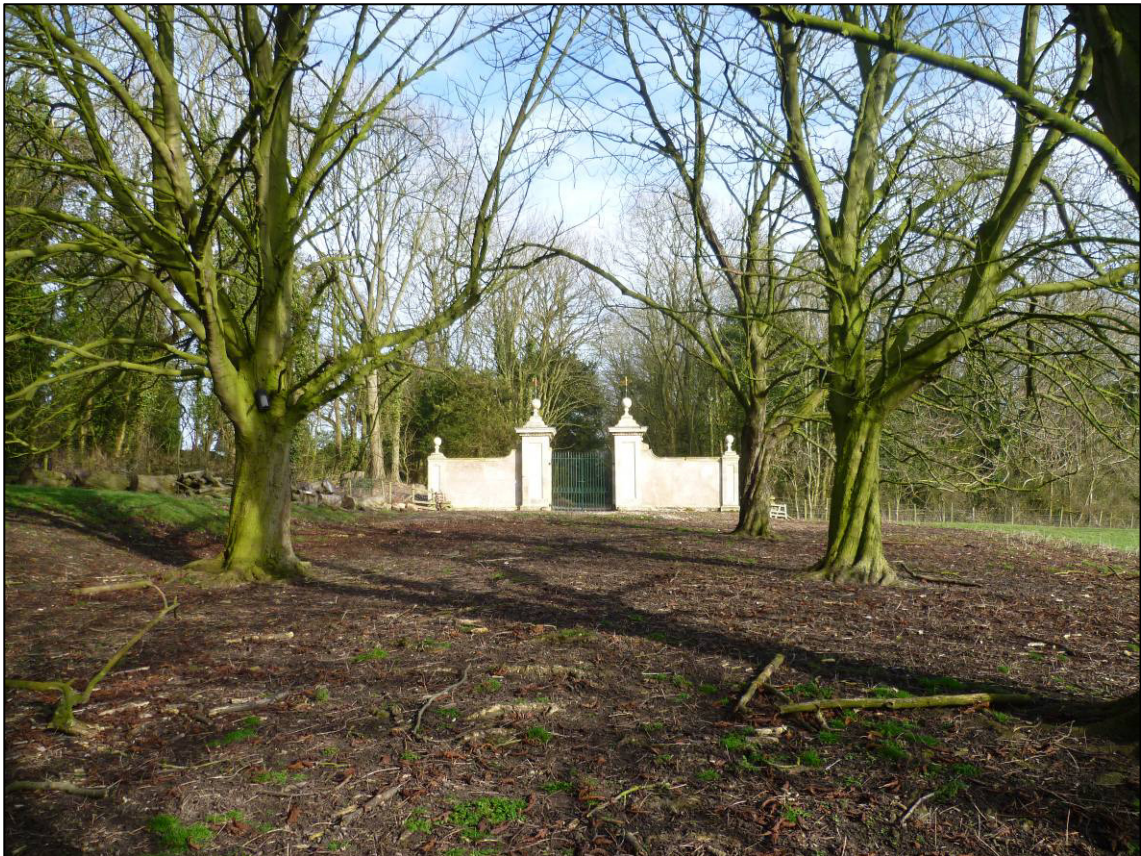
Plate 22: Completed rebuilding and restoration work, looking NE (photo 5/156).
