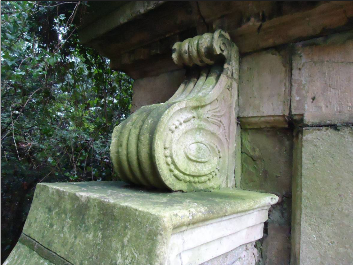
Plate 9: Detail of volute surmounting closing projection on Pier 3, prior to restoration, looking E (December 2016) (photo courtesy Peter Pace).
