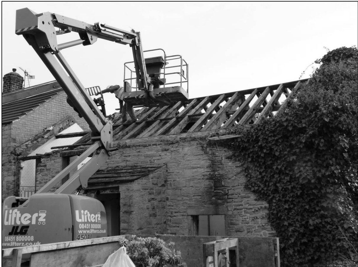
Plate 108: Barn Cottage range, S part, roof being dismantled, looking NE (photo 10/943).
