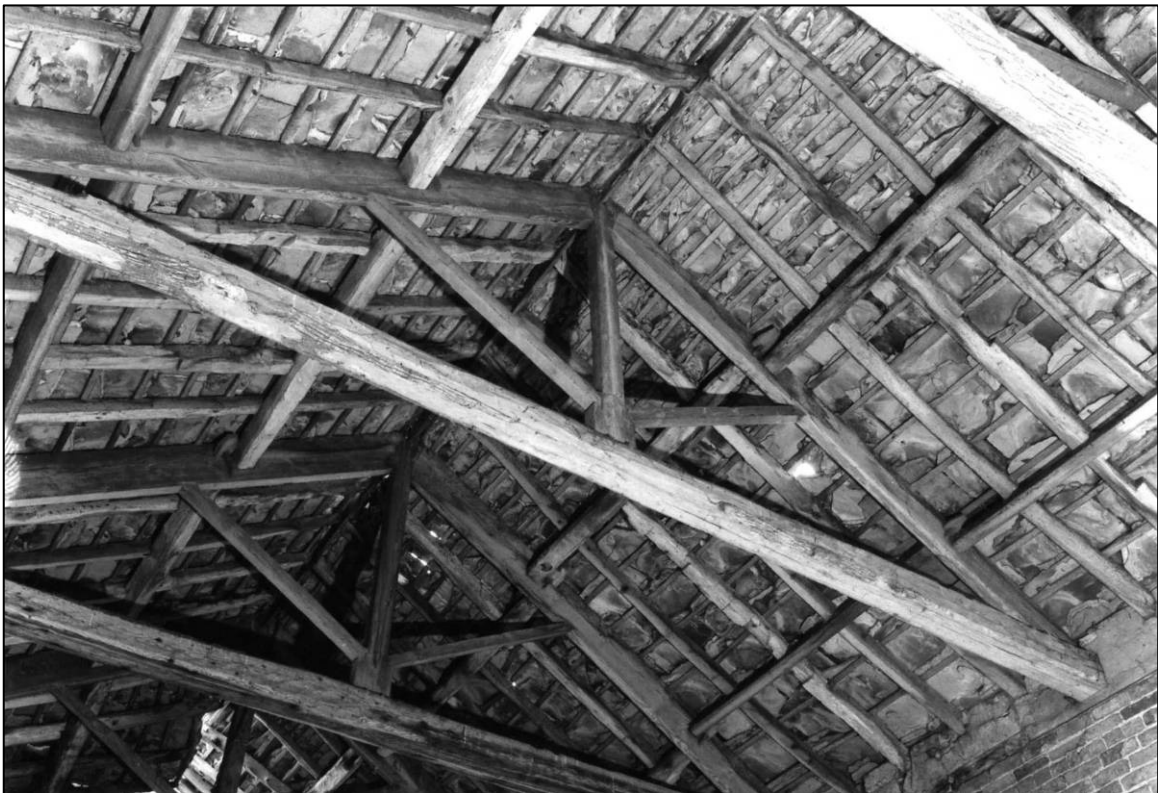
Plate 64: East barn range, interior, roof trusses, looking SW (photo 5/17).
