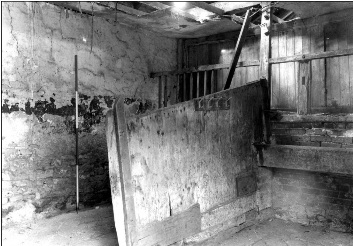
Plate 12: West coach house and stable range, S cell, details of fittings, looking NW (photo 1/17).
