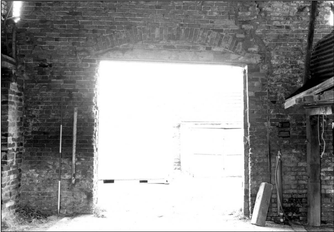
Plate 49: East barn range, interior, cart entrance, looking E (photo 5/8).
