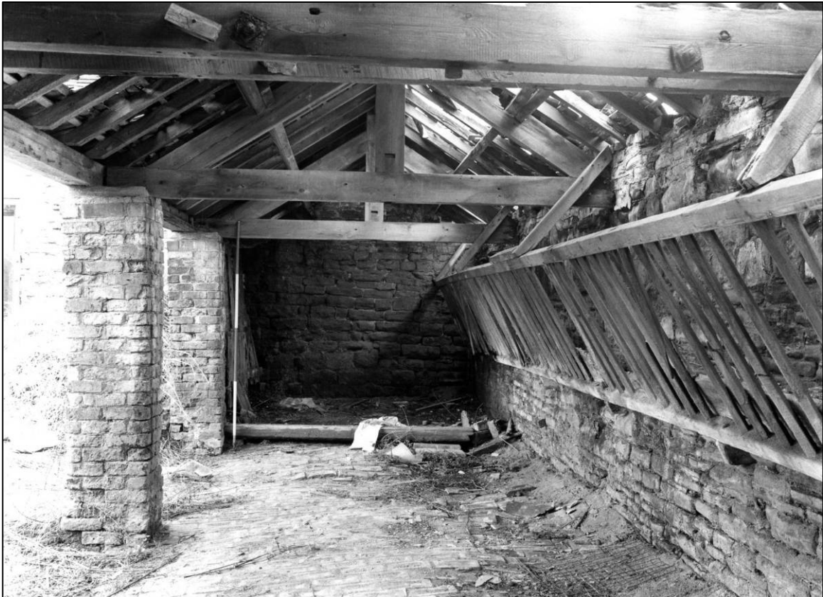
Plate 28: North cattle shade range, interior, showing hay rake, looking W (photo 2/19).
