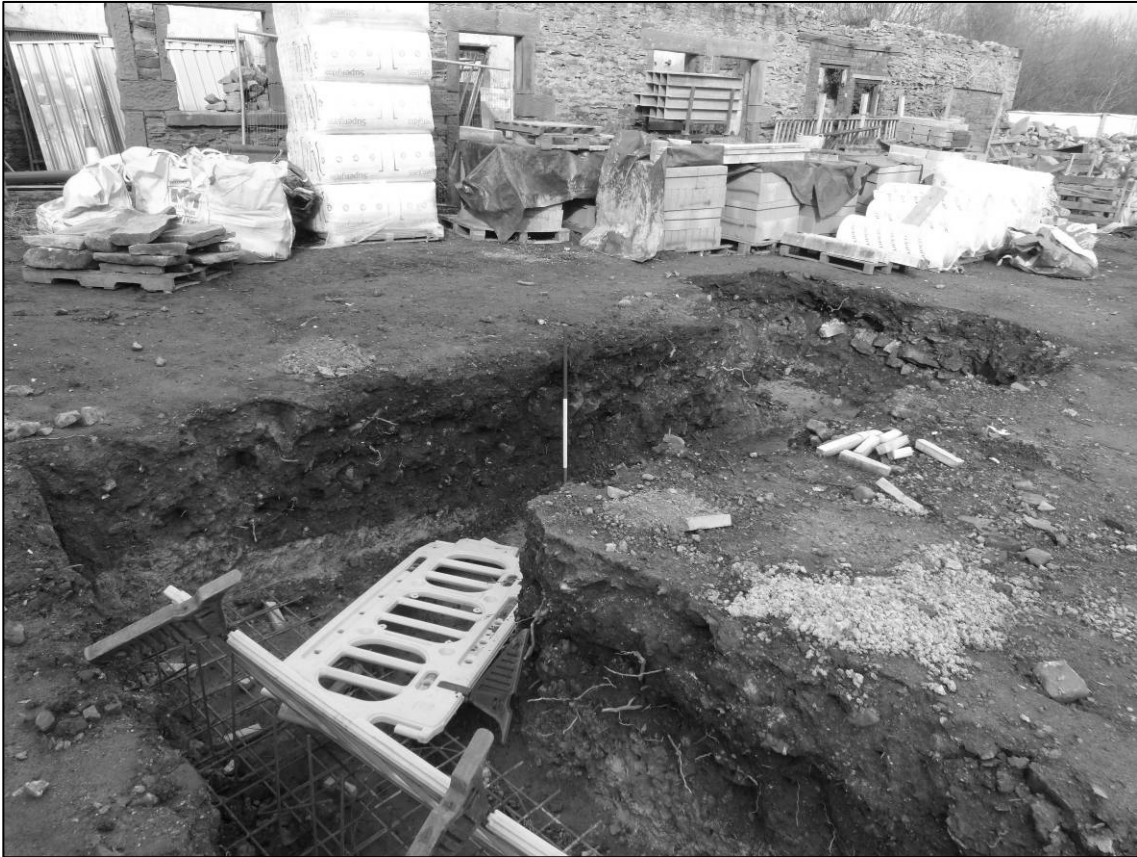
Plate 119: Trench 3, general view, looking NW (photo 10/947).
