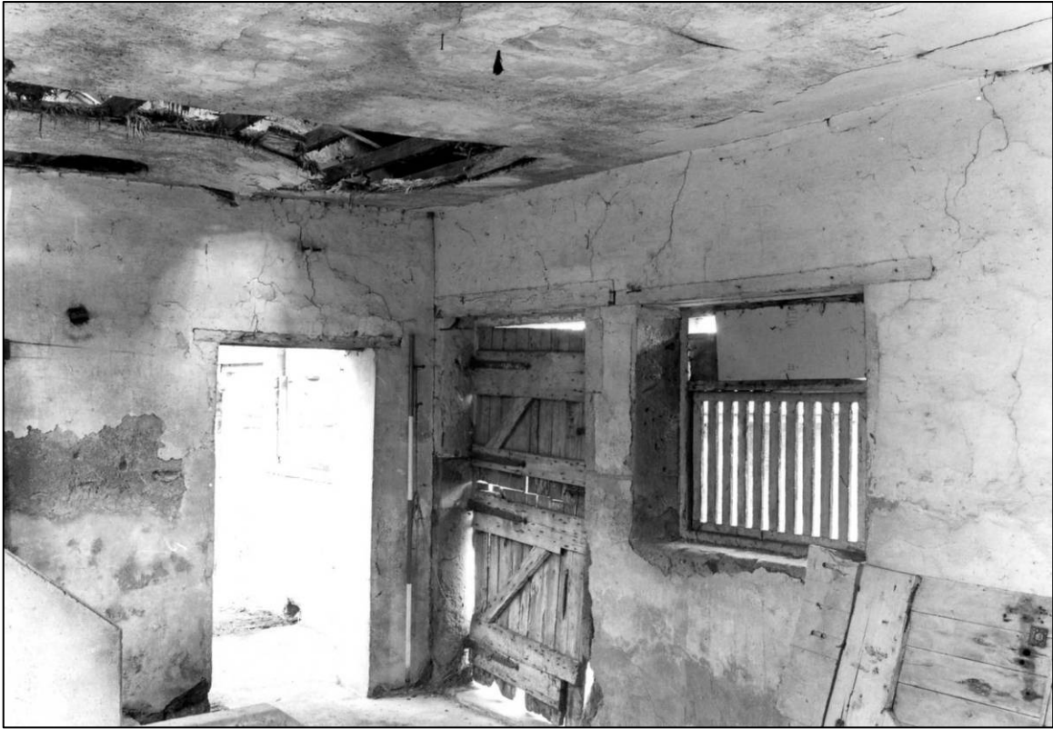
Plate 17: West coach house and stable range, central cell, looking NE (photo 2/9).
