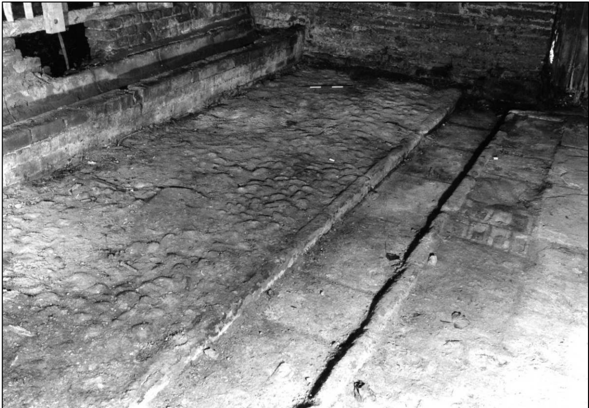
Plate 46: East barn range, S ground floor cell, drain, looking W (photo 4/15).
