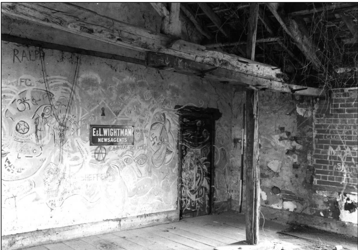
Plate 58: East barn range, S first floor cell, looking NE (photo 5/12).
