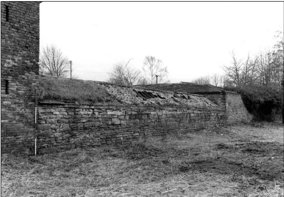
Plate 26: North cattle shade range, N elevation, looking SW (photo 3/12).
