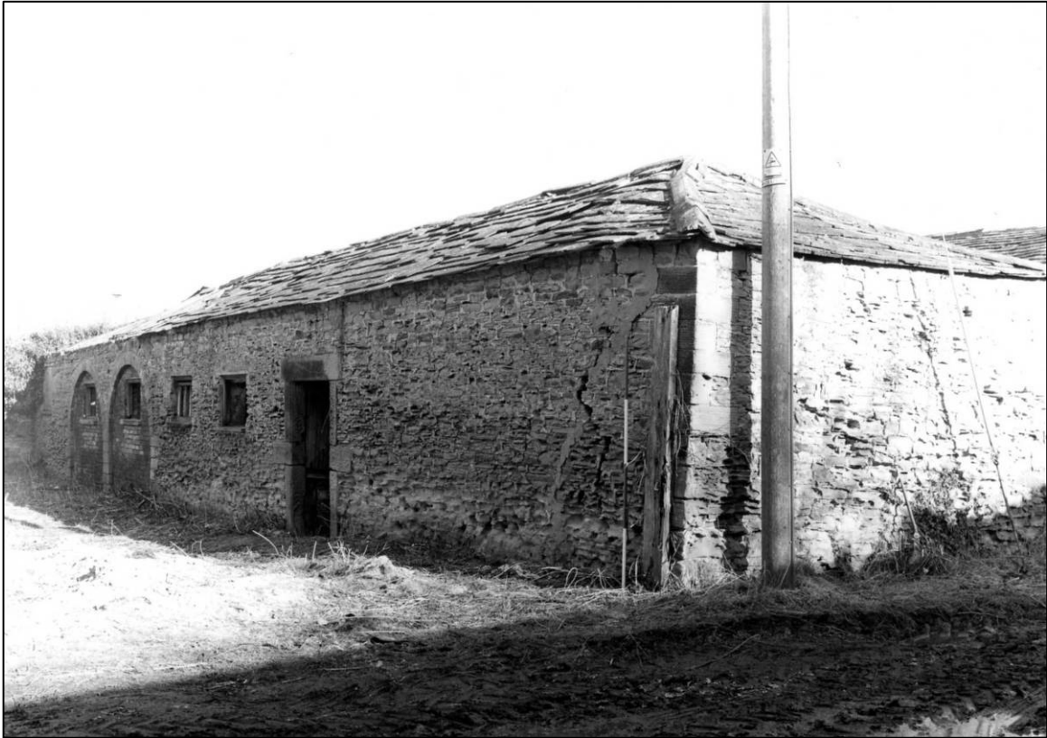
Plate 3: West coach house and stable range, W elevation, looking NE (photo 1/5).
