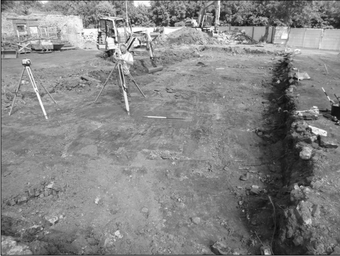
Plate 115: Trench 2, general view of ground reduction works, looking N (photo 9/088).
