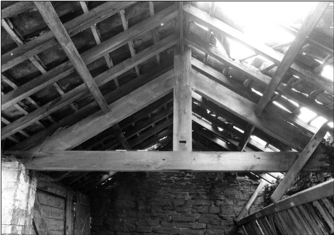
Plate 31: North cattle shade range, roof trusses, looking W (photo 3/1).
