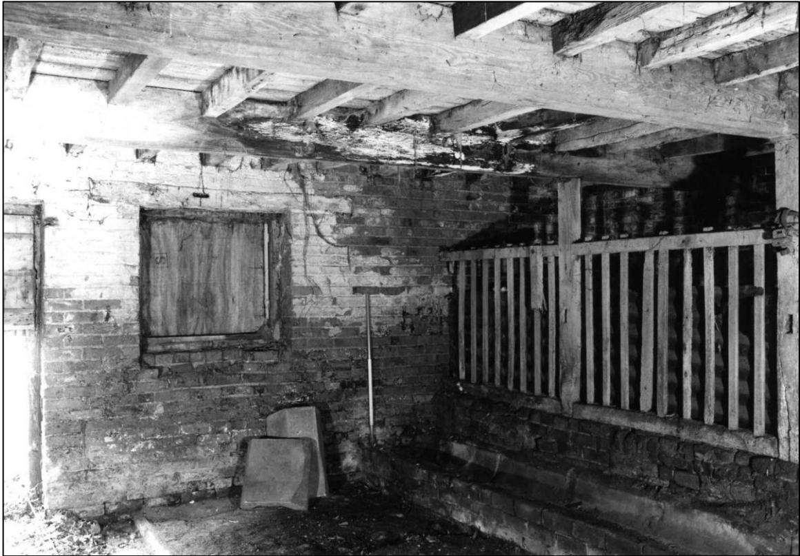
Plate 47: East barn range, S ground floor cell, looking SE (photo 4/16).
