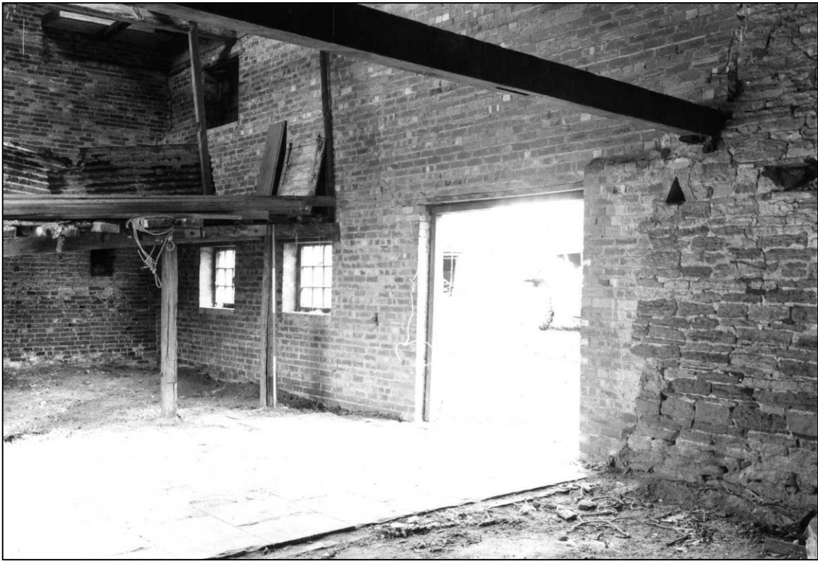
Plate 53: East barn range, interior, looking SW (photo 5/2).
