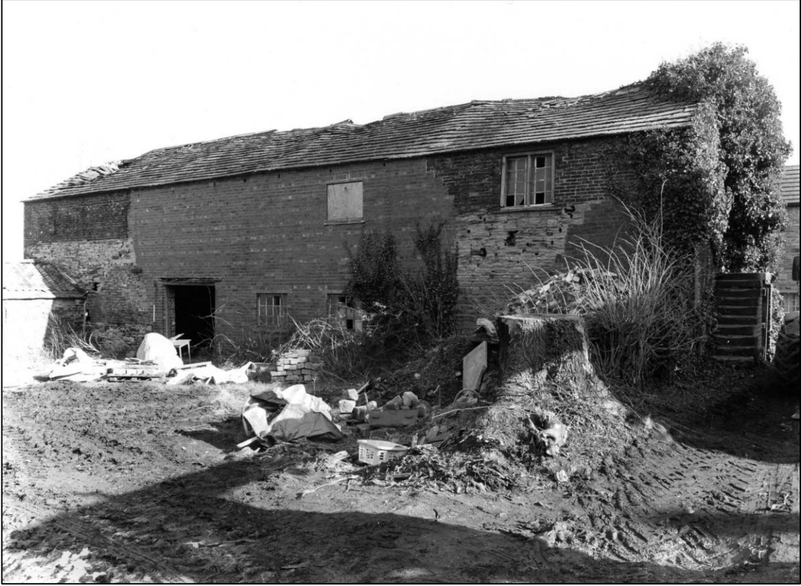
Plate 35: East barn range, W elevation, looking NE (photo 1/16).
