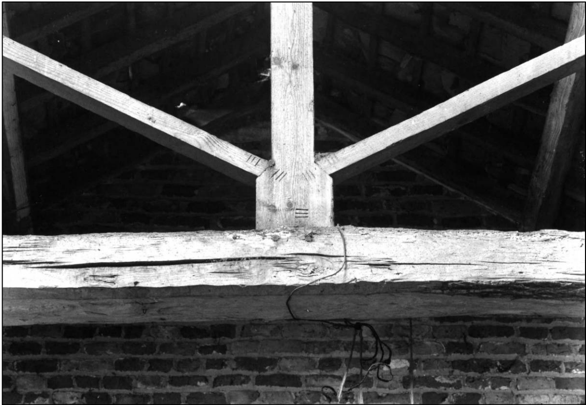
Plate 65: East barn range, interior, typical carpenters' marks to roof truss, looking S (photo 5/18).
