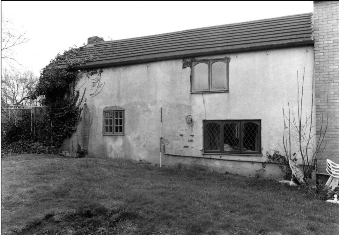
Plate 73: Barn Cottage range, E elevation, S part, looking S (photo 4/2).
