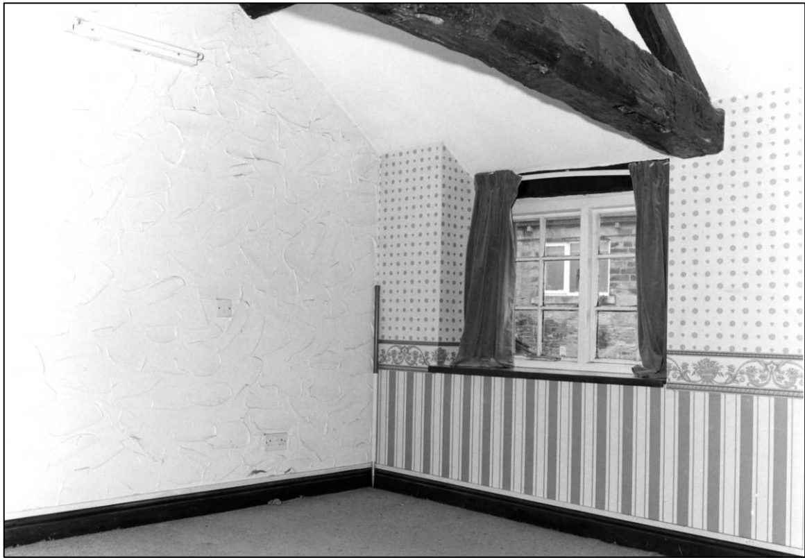
Plate 103: Barn Cottage range, S part, N first floor room (Room 9), looking SW (photo 6/13).
