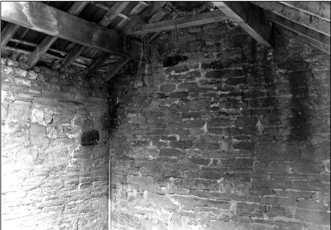
Plate 30: North cattle shade range, E cell, interior, looking NE (photo 6/2).
