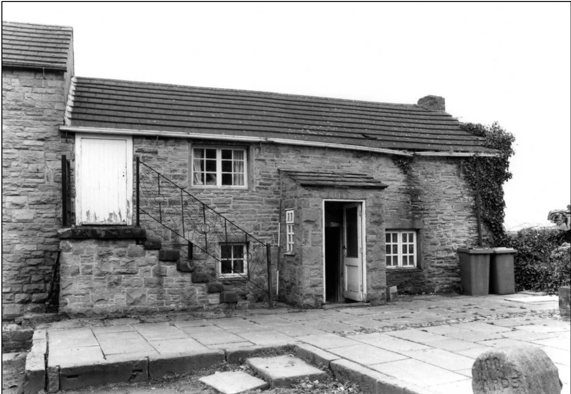
Plate 71: Barn Cottage range, W elevation, S part, looking SE (photo 3/18).
