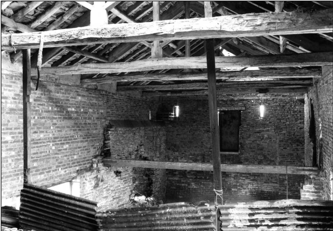
Plate 62: East barn range, interior, upper level, looking N (photo 5/14).
