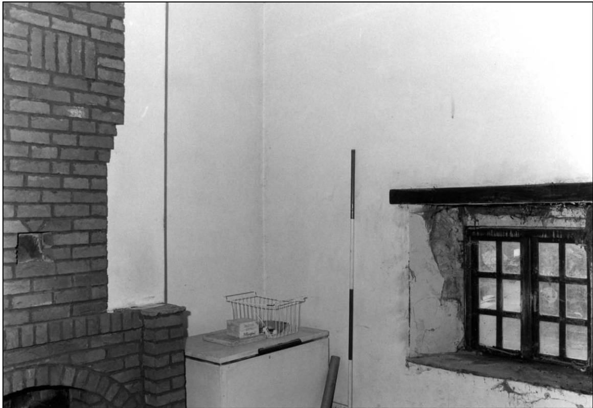
Plate 95: Barn Cottage range, S part, S ground floor room (Room 7), looking SW (photo 4/5).
