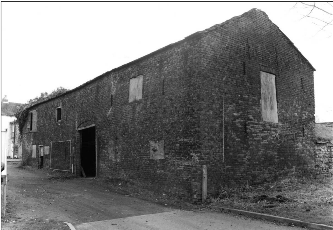
Plate 40: East barn range, E elevation and N gable, looking SW (photo 3/9).
