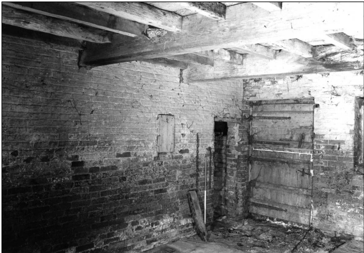
Plate 48: East barn range, S ground floor cell, looking NE (photo 4/17).
