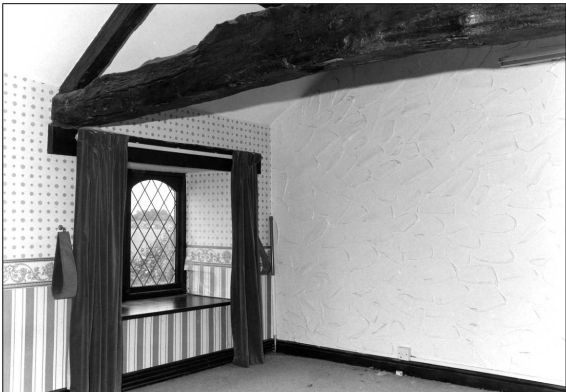
Plate 102: Barn Cottage range, S part, N first floor room (Room 9), looking SE (photo 6/12).
