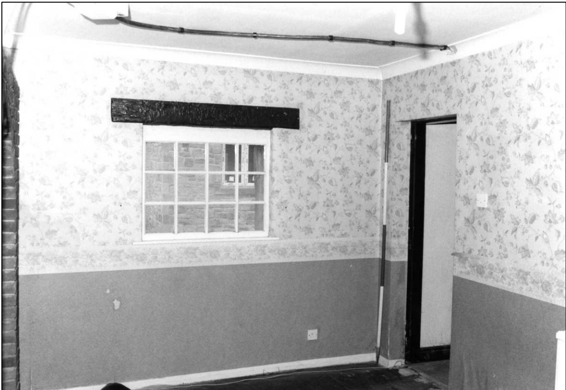
Plate 80: Barn Cottage range, N part, S ground floor room (Room 2), looking W (photo 11/10).
