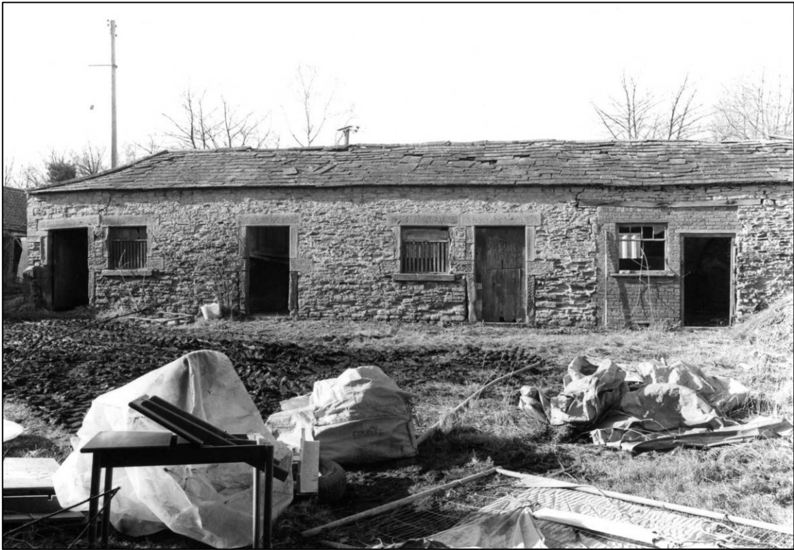
Plate 9: West coach house and stable range, E elevation, looking W (photo 1/7).
