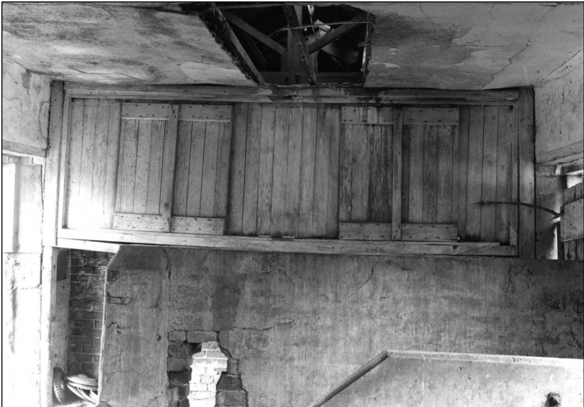
Plate 18: West coach house and stable range, central cell, fodder cupboard, looking S (photo 2/5).
