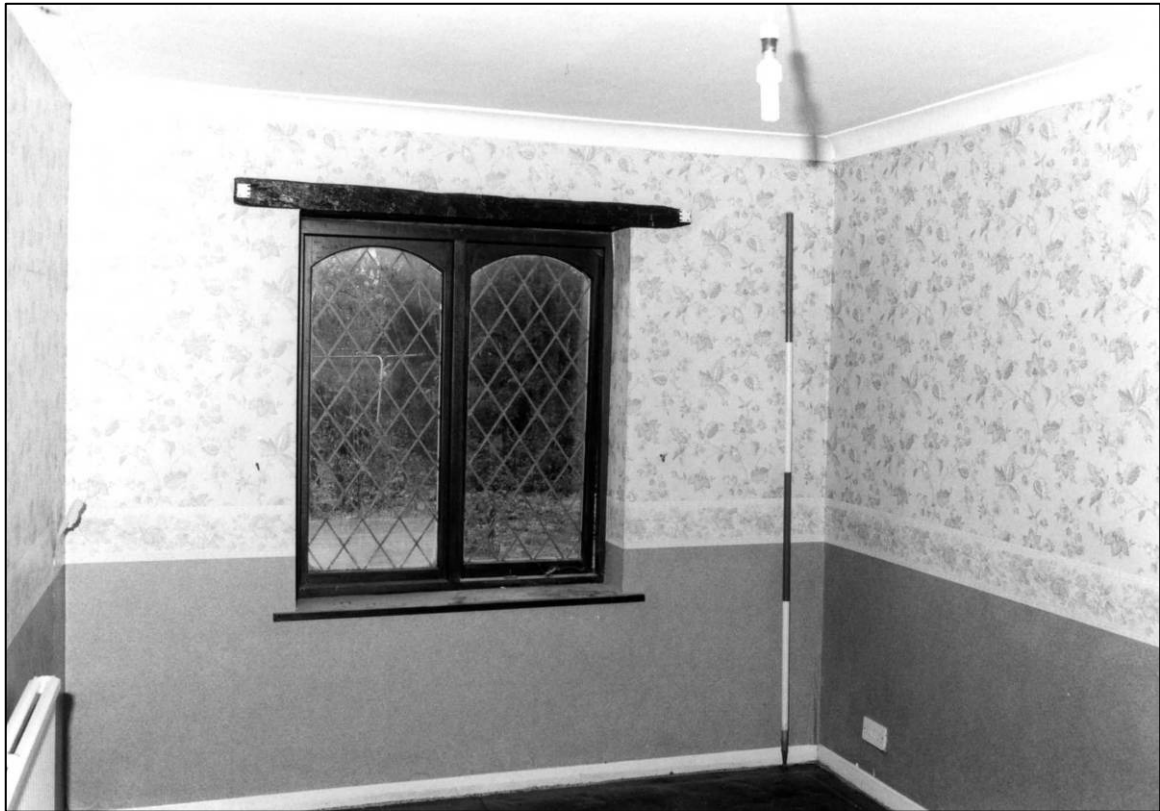
Plate 81: Barn Cottage range, N part, S ground floor room (Room 2), looking E (photo 11/11).
