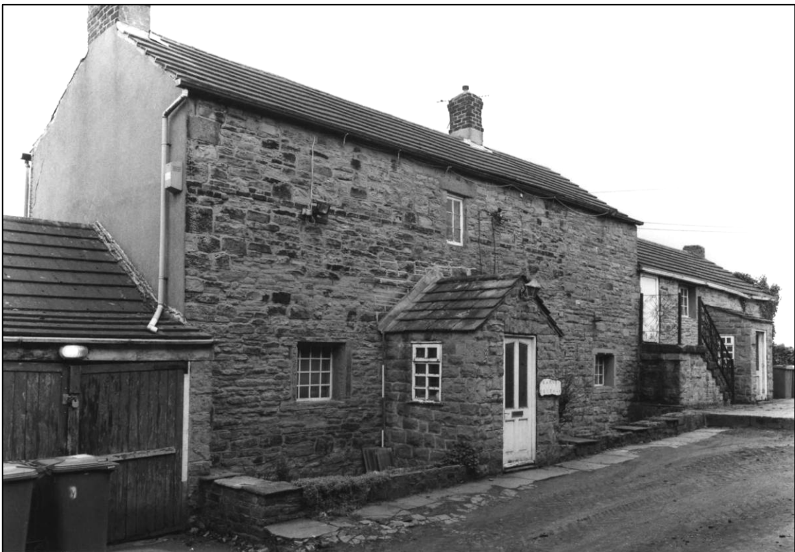
Plate 68: Barn Cottage range, W elevation, N part, looking SE (photo 3/16).
