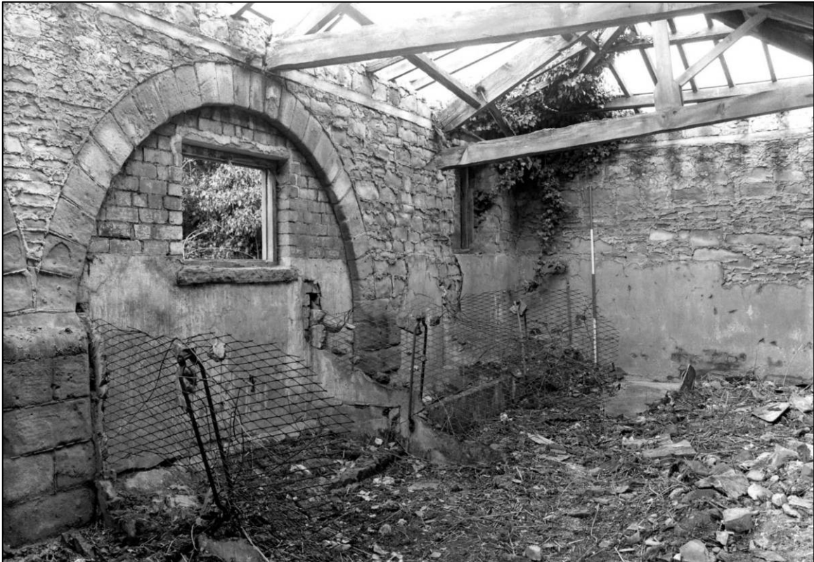
Plate 21: West coach house and stable range, N cell, looking NW (photo 2/11).
