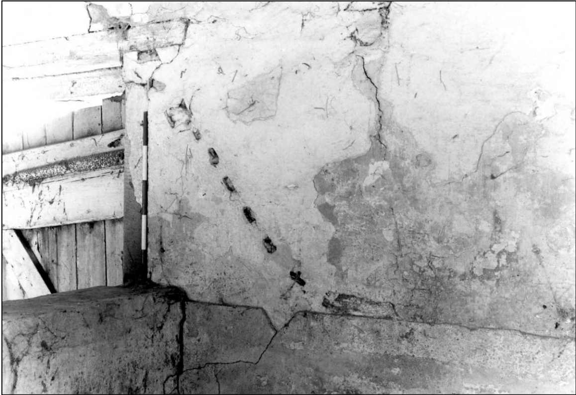
Plate 15: West coach house and stable range, central cell, mortices of curved fitting to W wall, looking W (photo 2/8).
