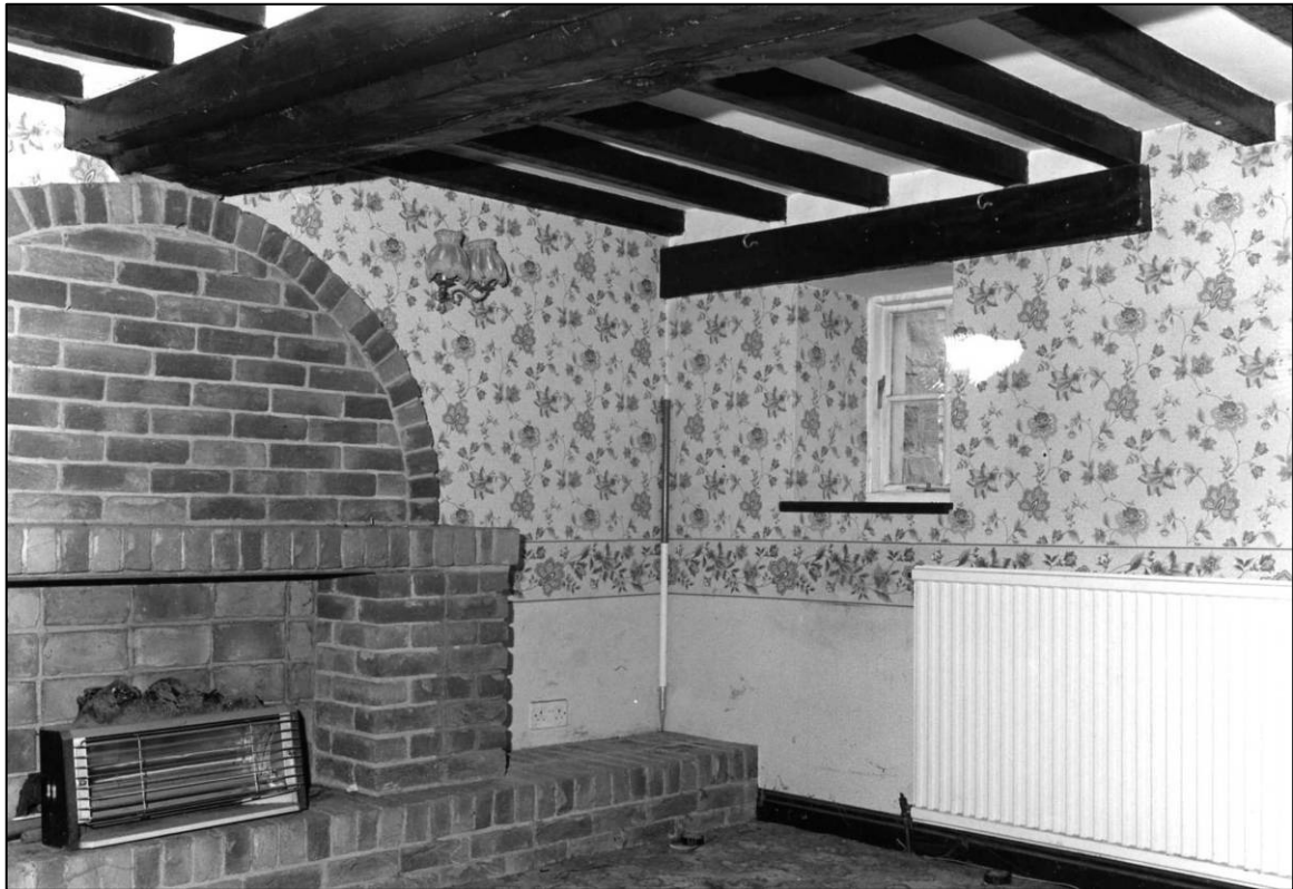
Plate 99: Barn Cottage range, S part, N ground floor room (Room 8), looking SW (photo 6/8).
