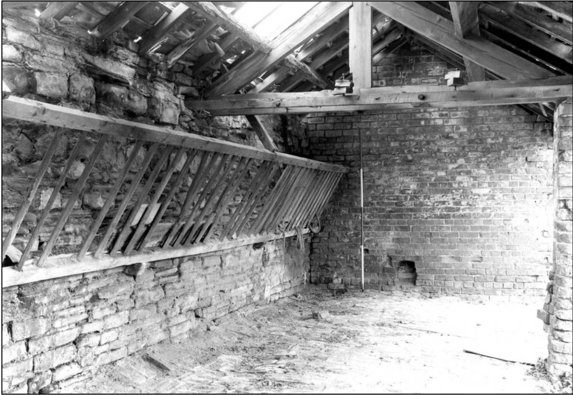
Plate 27: North cattle shade range, interior, showing hay rake, looking E (photo 2/17).
