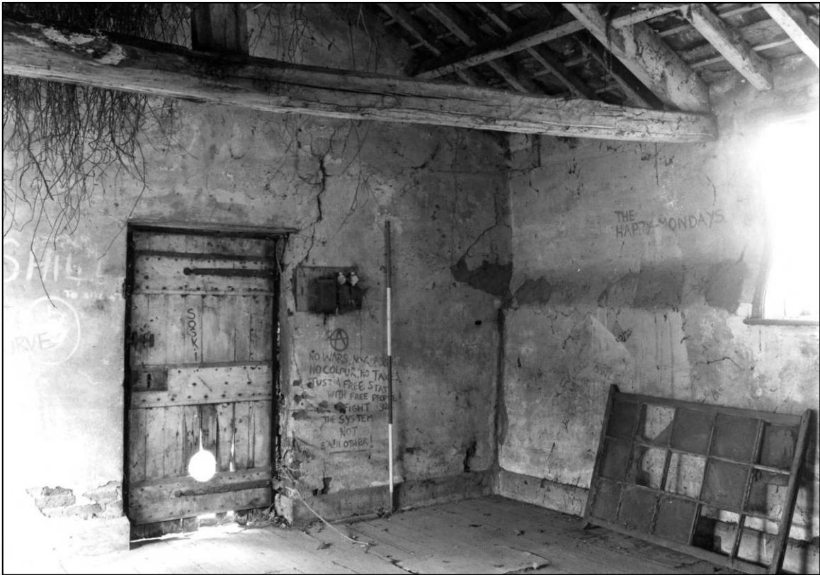
Plate 59: East barn range, S first floor cell, looking SW (photo 5/13).
