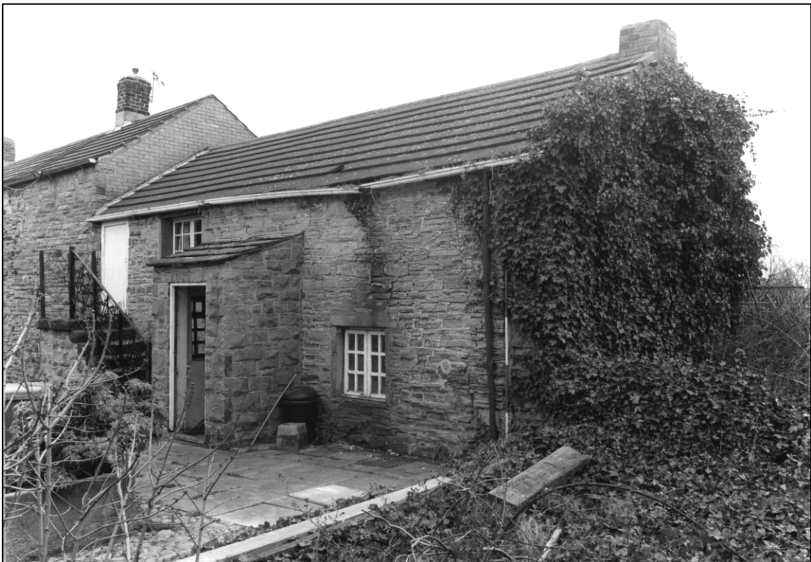
Plate 72: Barn Cottage range, W elevation, S part and S gable, looking NE (photo 4/1).
