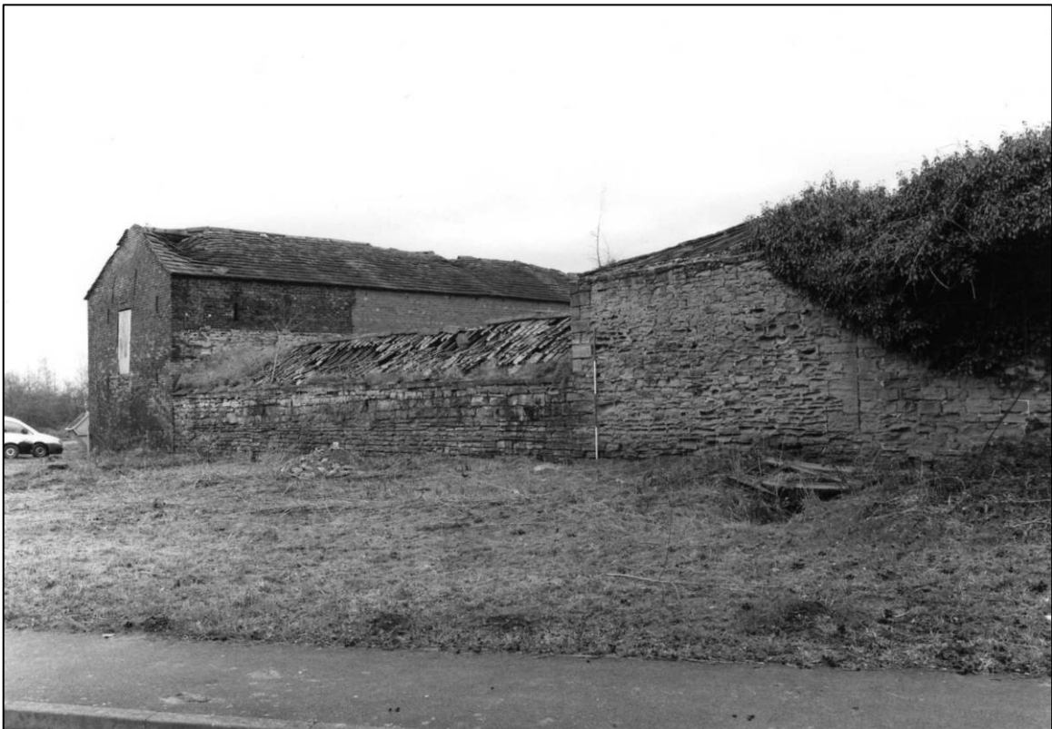
Plate 2: North side of farm buildings, with single storey cattle shade range to centre, looking SE (photo 3/13).
