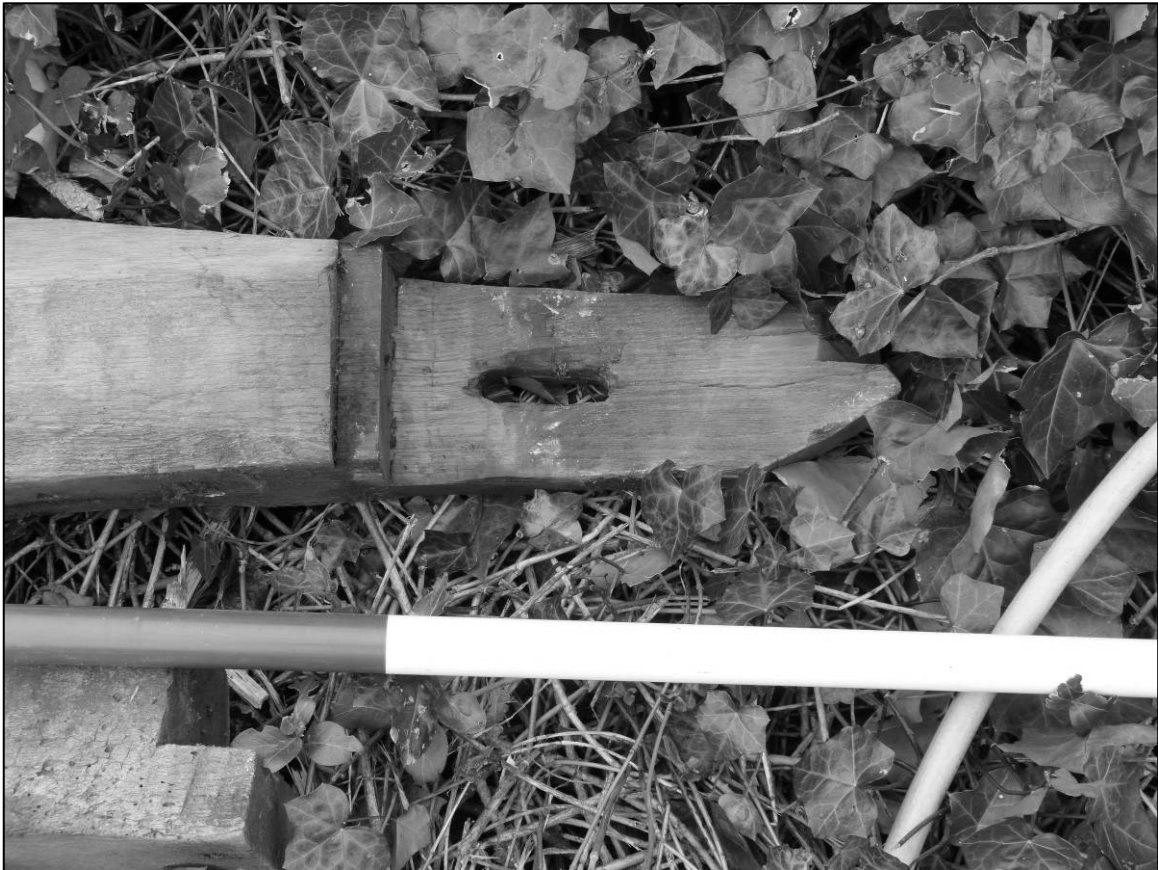
Plate 109: Barn Cottage range, S part, example of re-used common rafter (photo 10/952).
