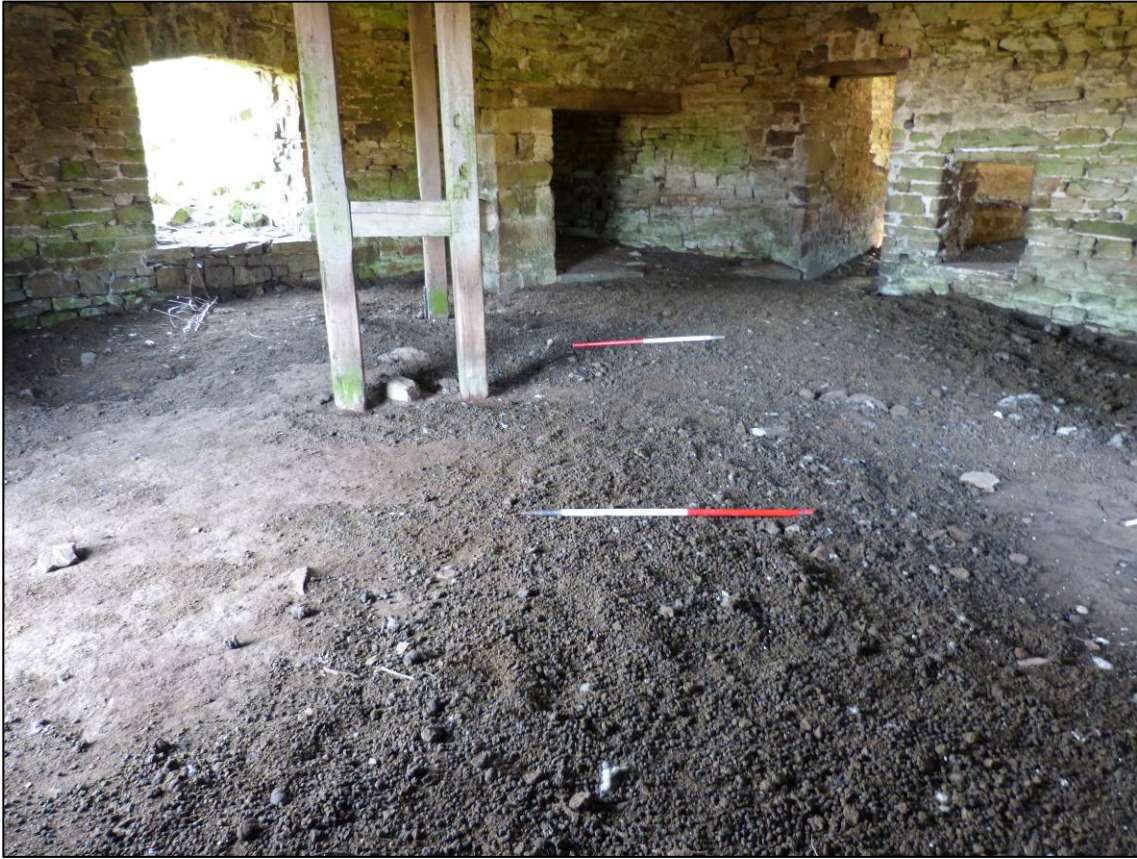
Plate 3: Bellows Room, prior to clearance, looking SE (photo 1/194).
