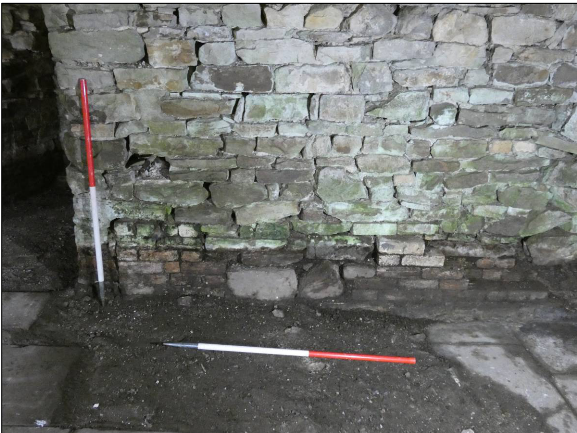
Plate 22: Furnace Room, south side of store room, after clearance and cleaning, showing remains of slag hearth, looking N (photo 4/153).
