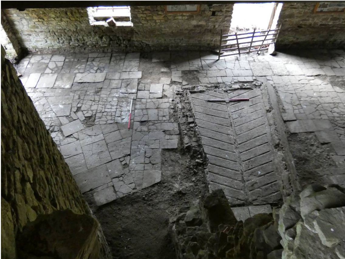
Plate 19: East side of furnace room, after clearance and cleaning, showing sheep dip and differential wear to flagstone floor, looking S (photo 4/160).
