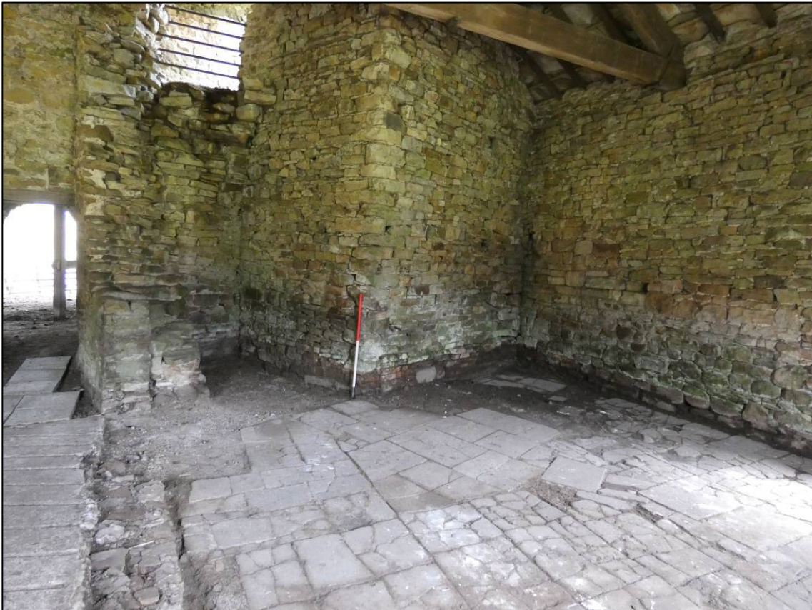
Plate 21: North-east corner of furnace room, after clearance and cleaning, showing store room and slag hearth position, looking NE (photo 4/173).
