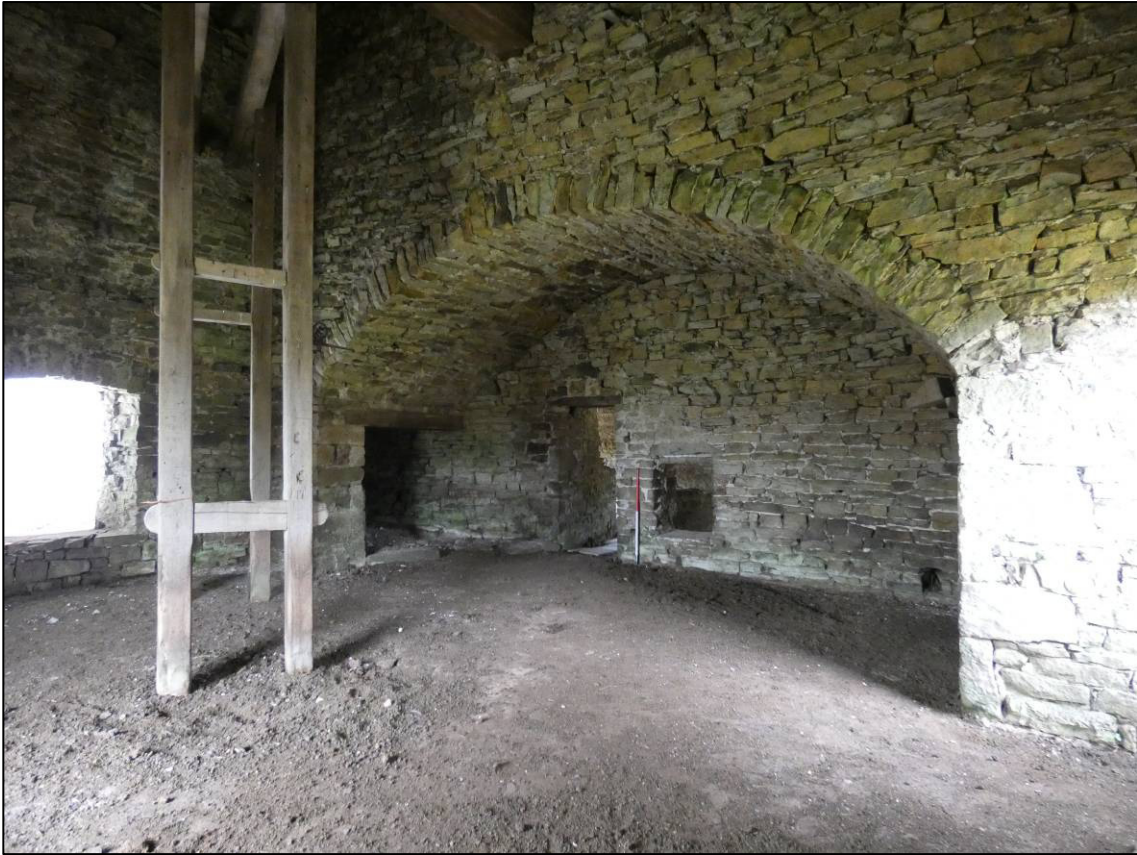
Plate 7: Bellows Room, after limited clearance, looking SE (photo 4/180).
