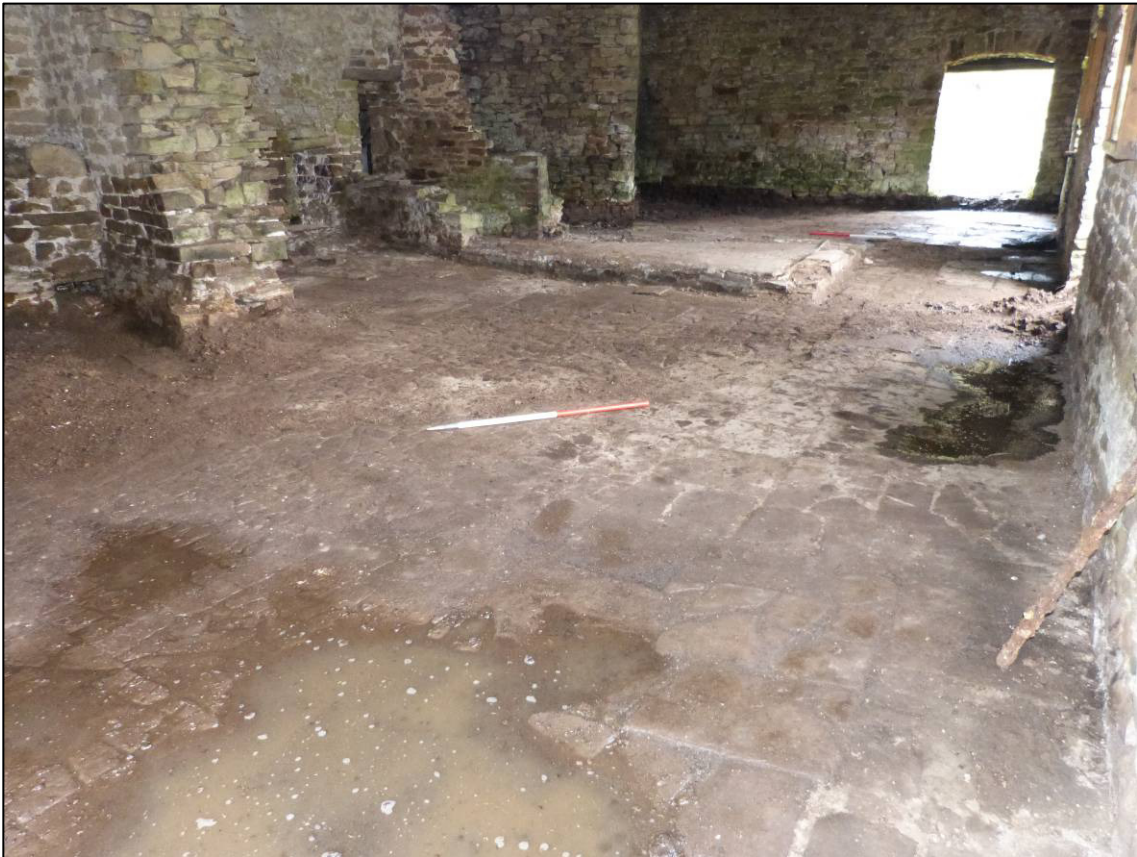
Plate 5: Furnace Room, after clearance, looking E (photo 3/360).
