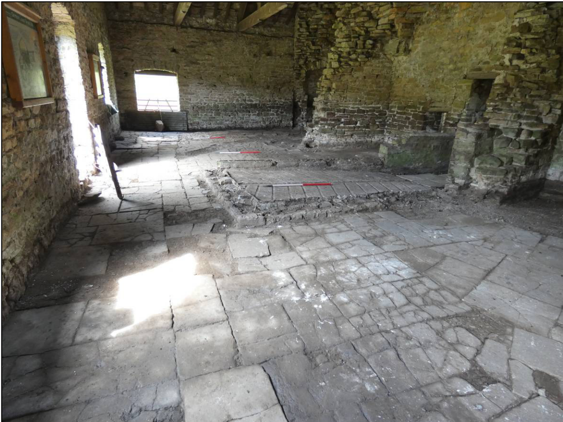
Plate 13: General view of furnace room, after clearance and cleaning, looking W (photo 4/125).
