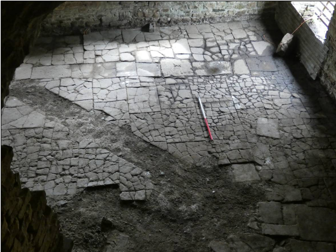
Plate 16: Flagstone floor in west side of furnace room, after clearance and cleaning, looking S (photo 4/168).
