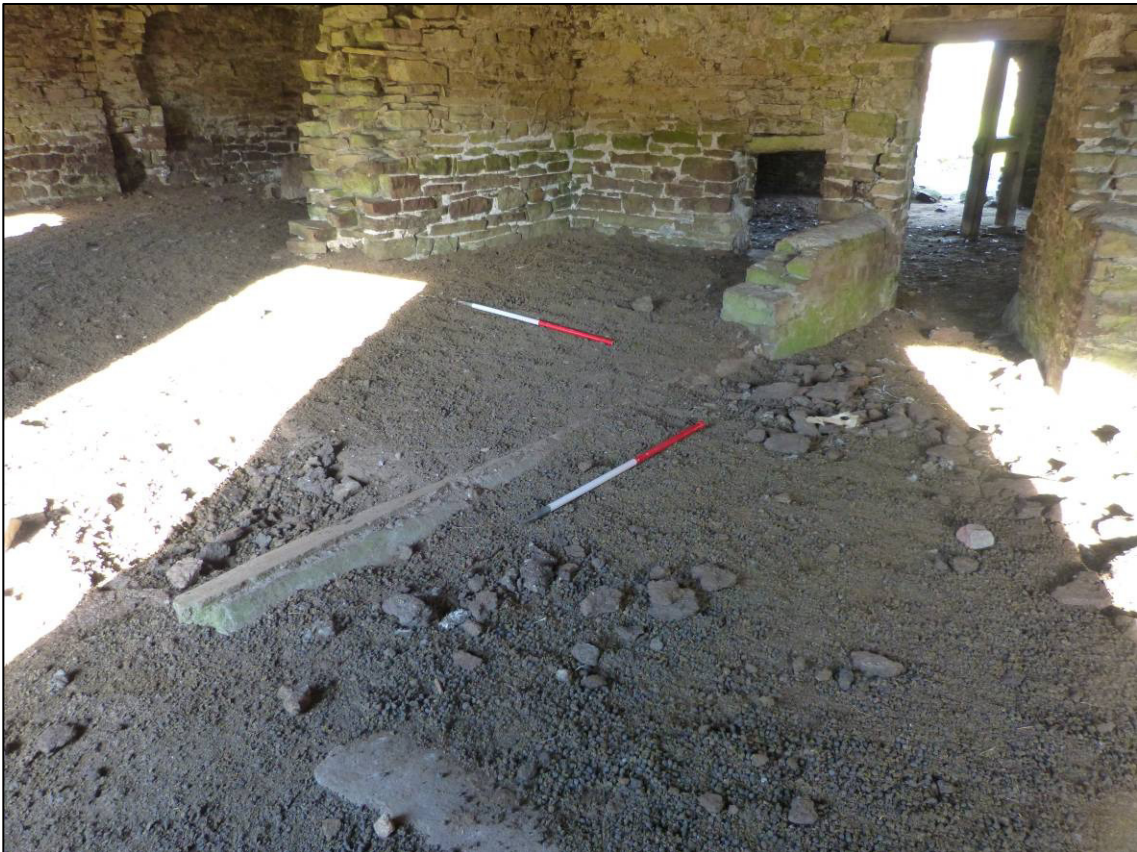
Plate 2: Furnace Room, prior to clearance, looking NW (photo 1/182).
