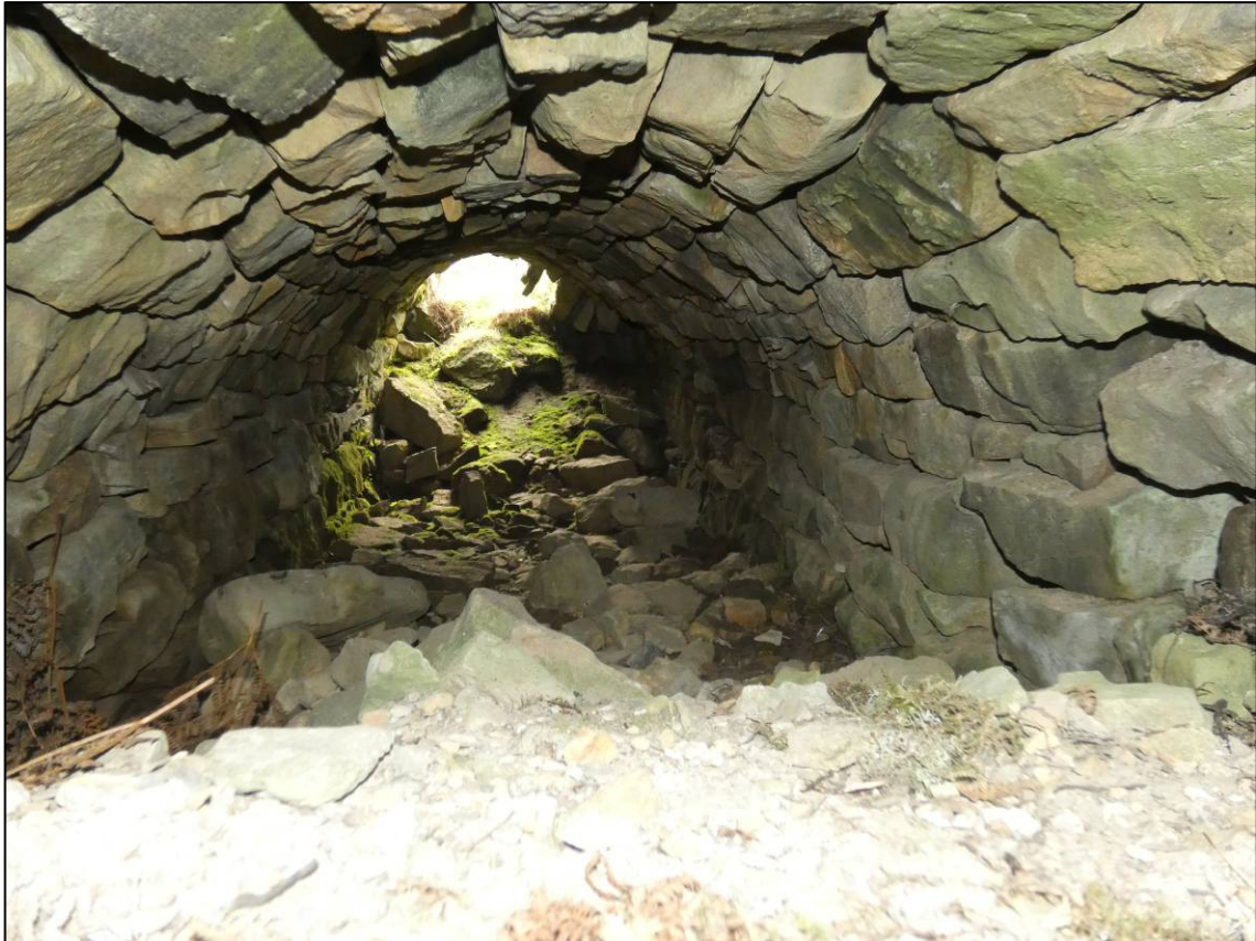
Plate 7: Interior of culvert to Swinston Hush watercourse, looking W (photo 2/333).
