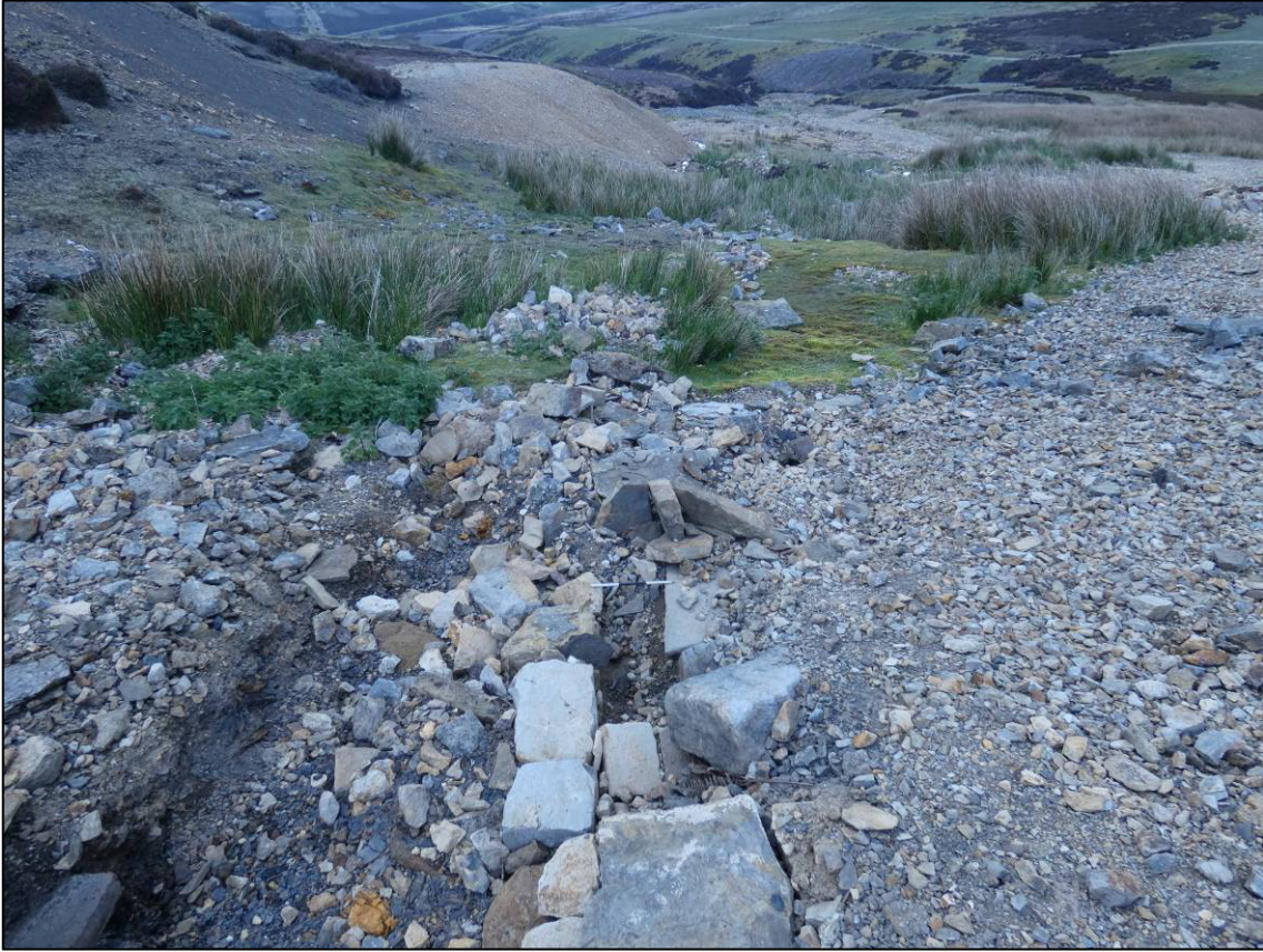
Plate 23: Culvert to east of exposed flagstones (J), looking E (photo 2/363).
