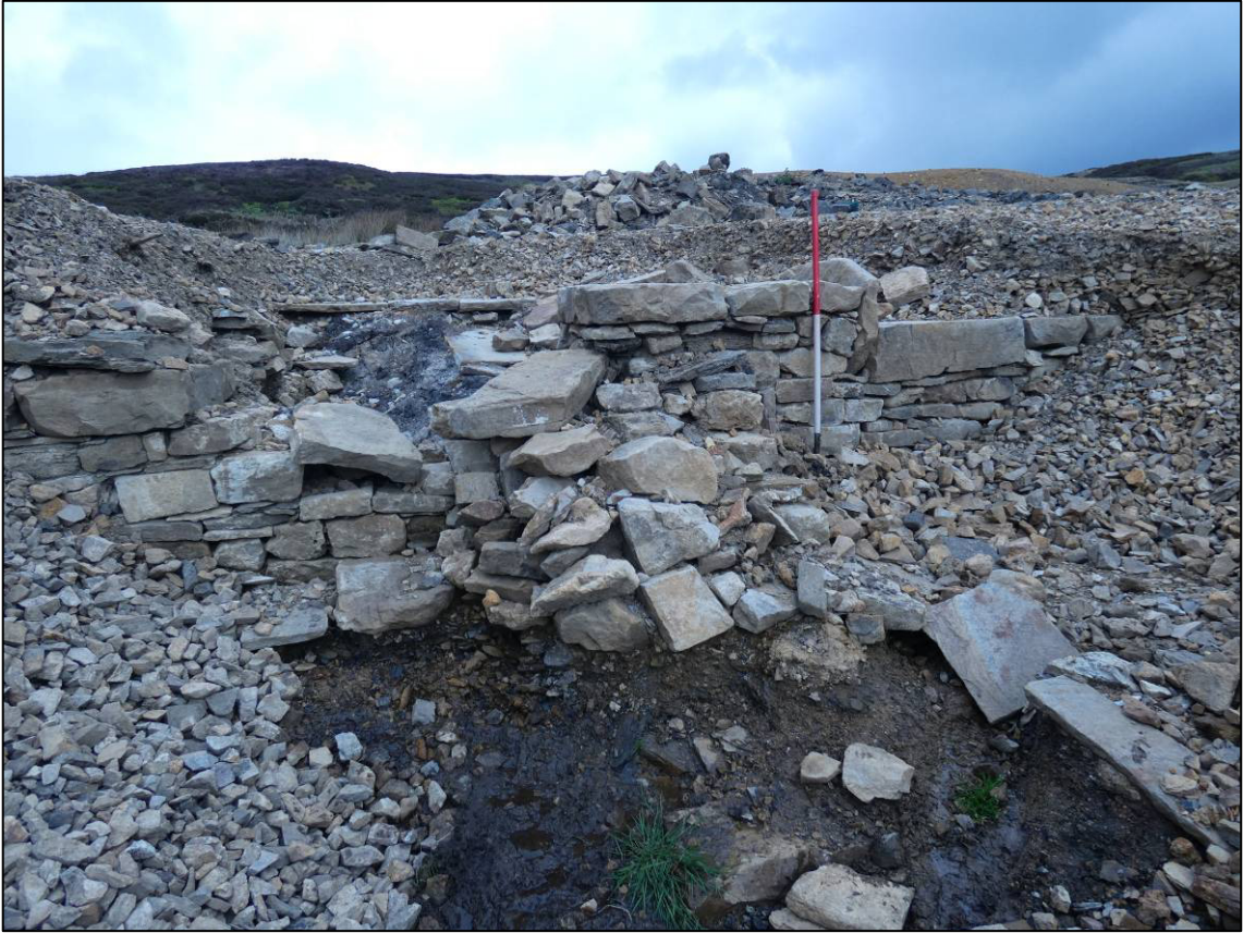
Plate 25: Main revetment wall to east end of flagstones (K), looking W (photo 2/379).
