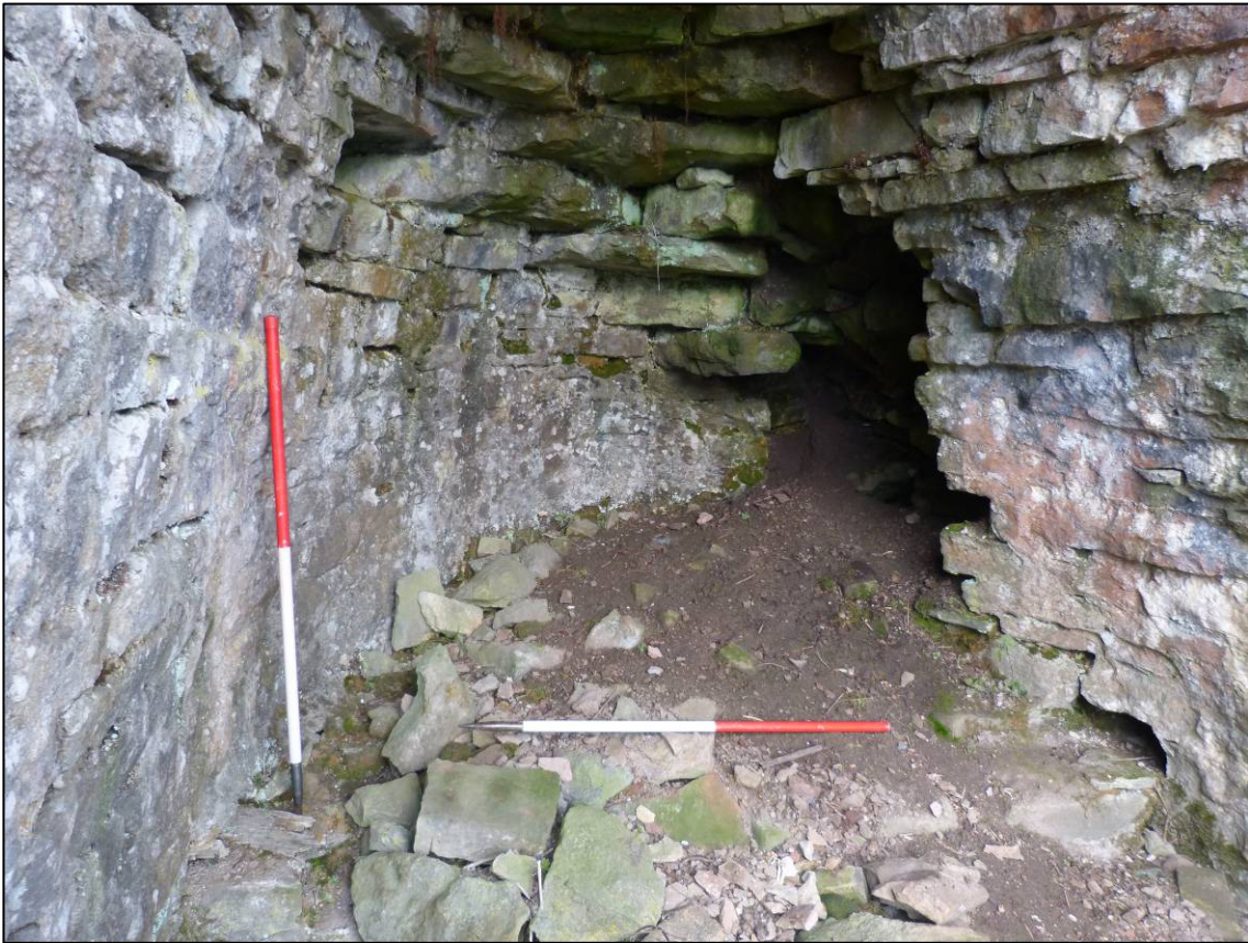
Plate 8: West draw arch, draw hole and platform, looking N (photo 1/894).
