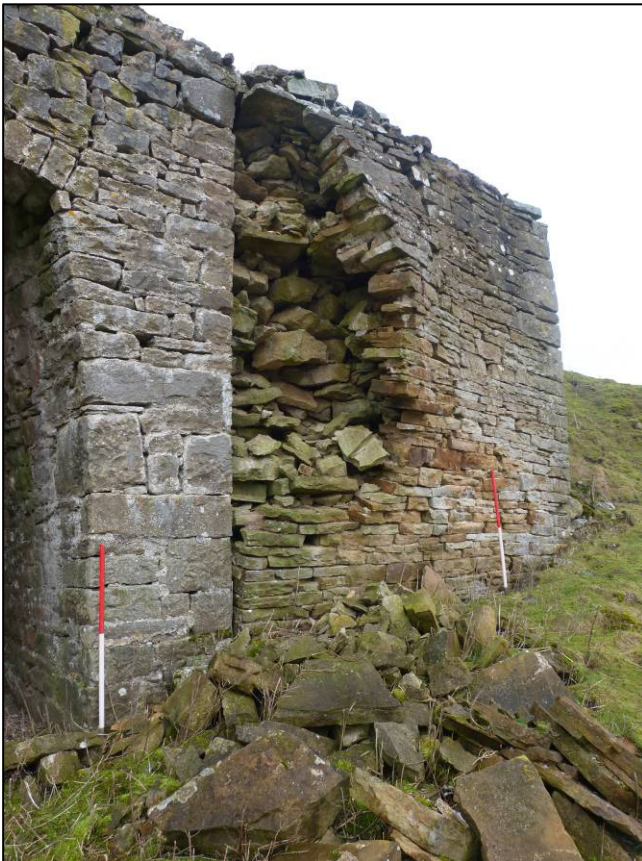
Plate 4: South elevation, E retaining wall, looking NE (photo 1/888).
