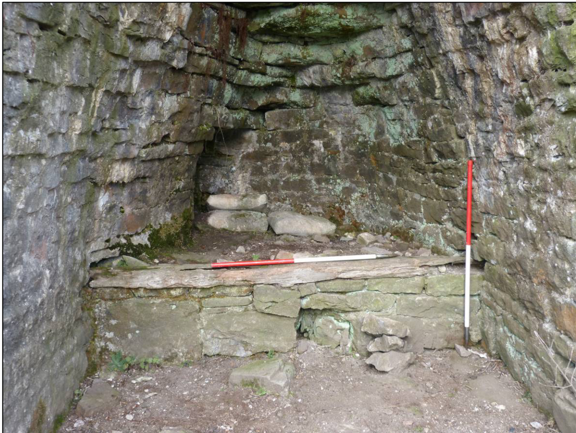
Plate 12: East draw arch, draw hole and platform, looking N (photo 1/900).
