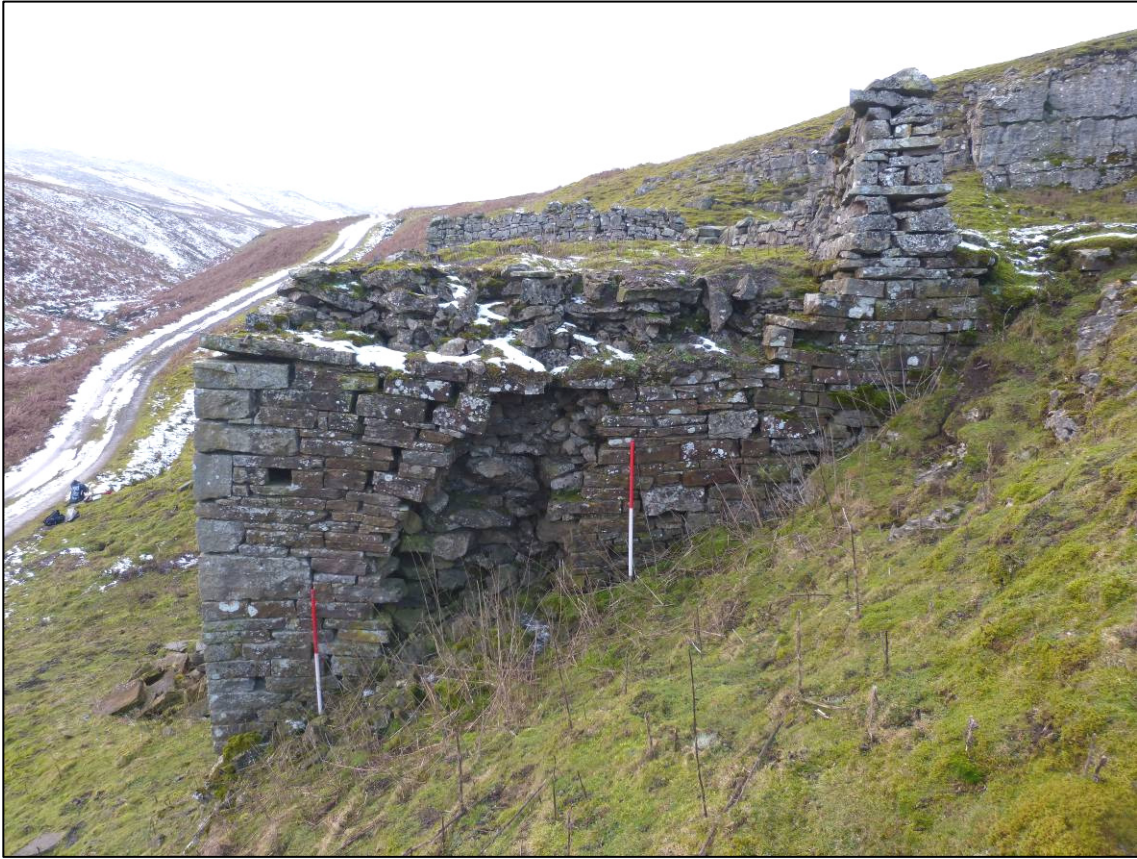
Plate 16: East elevation, east retaining wall, looking W (photo 1/915).
