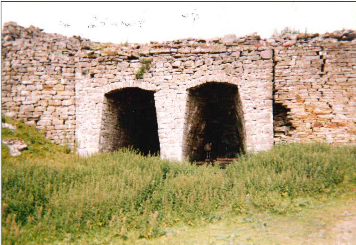
Plate 6: South elevation kiln and retaining walls, taken by David Johnson, July 2005.
