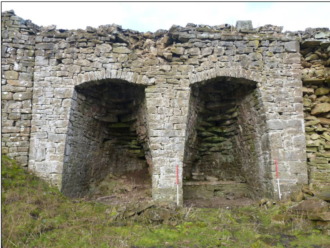
Plate 7: South elevation of kiln, looking N (photo 1/912).
