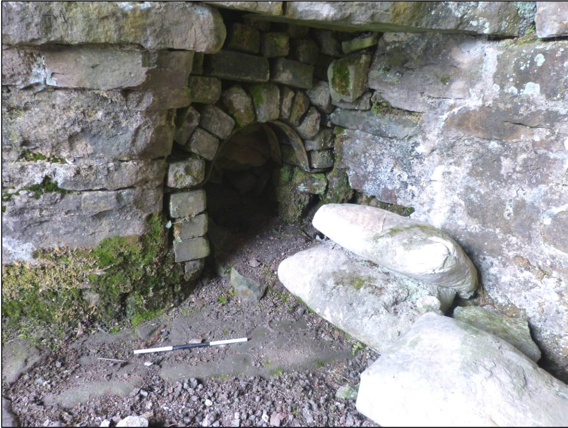
Plate 13: East draw arch, draw hole, looking NW (photo 1/904).
