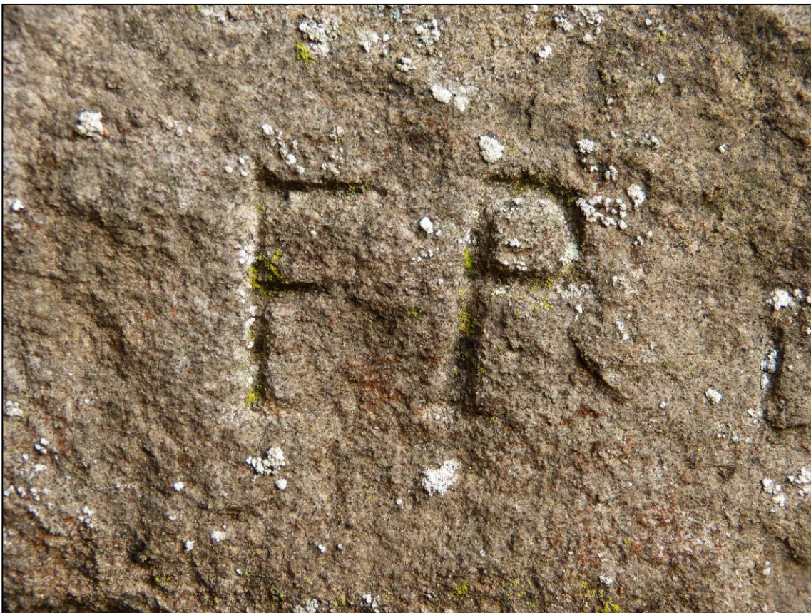
Plate 9: East draw arch, 'FP' graffiti to east wall, looking E (photo 1/931).
