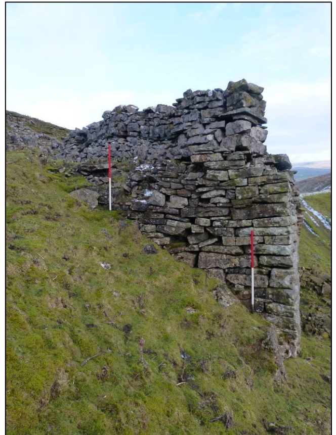
Plate 15: West elevation, west retaining wall, looking E (photo 1/928).
