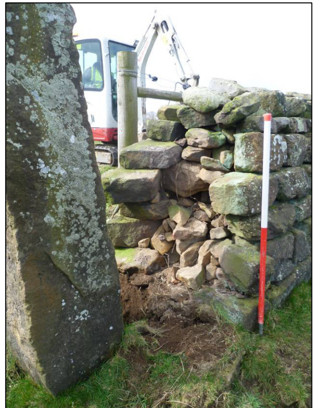
Plate 5: Western wall end during dismantling, looking SW (photo 1/303).
