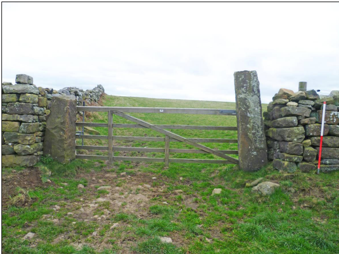
Plate 2: South side of gateway, prior to repairs, looking N (photo 1/293).
