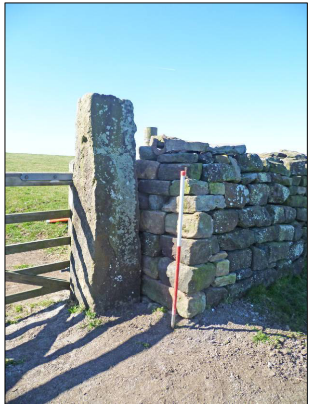
Plate 12: Rebuilt western wall end, looking SW (photo 2/339).
