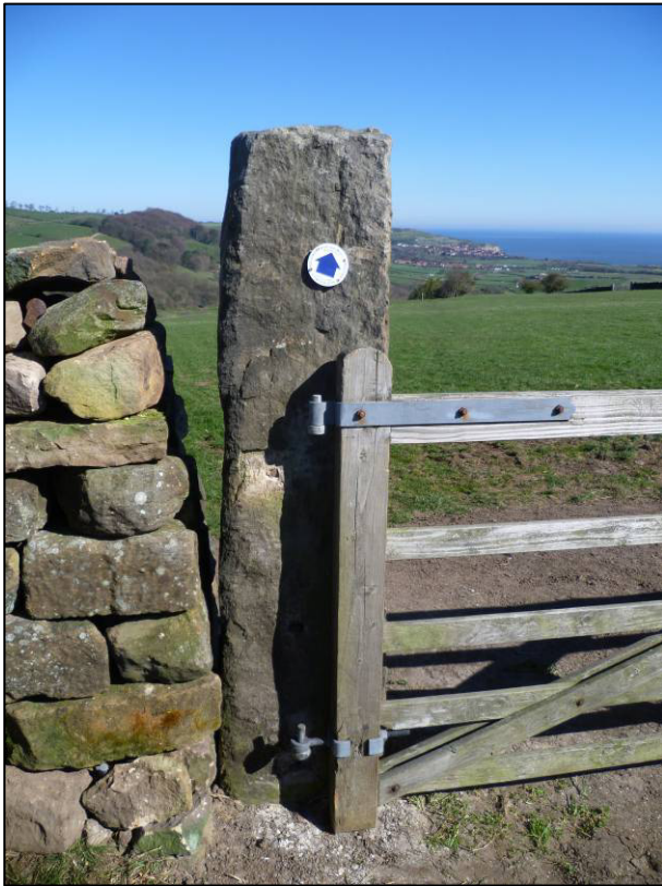
Plate 13: Repositioned western gatepost and rebuilt wall end, looking N (photo 2/351).
