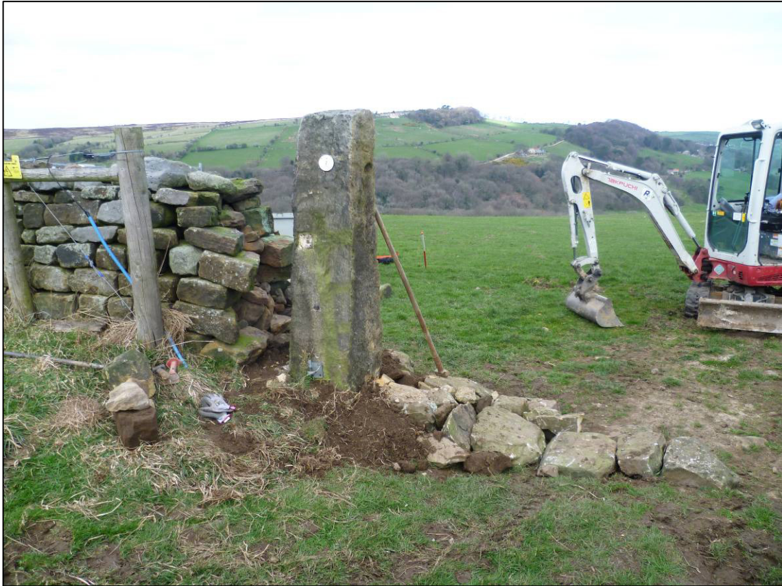
Plate 10: Straightened western gatepost, looking N (photo 1/310).
