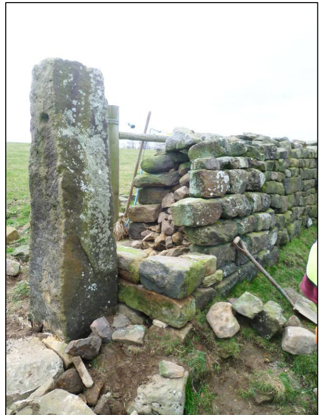
Plate 9: Rebuilding western wall end, looking SW (photo 1/312).
