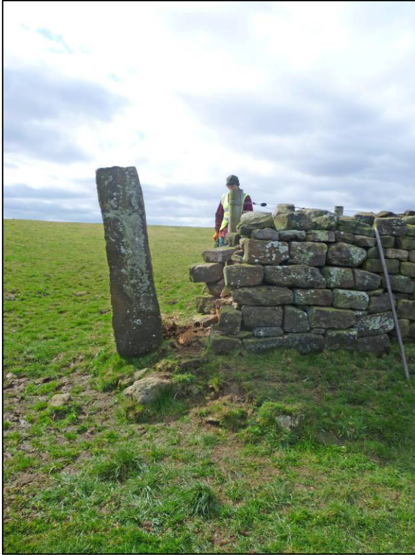
Photo 6: Western wall end after dismantling, looking S (photo 1/302).
