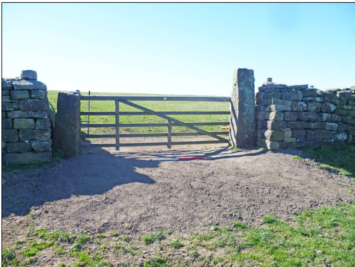
Plate 17: Repaired gateway, looking S (photo 2/349).
