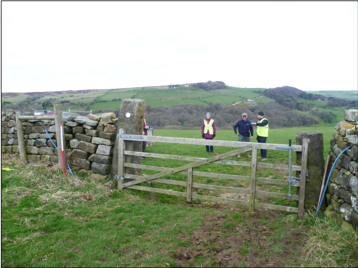
Plate 3: North side of gateway, prior to repairs, looking S (photo 1/295).
