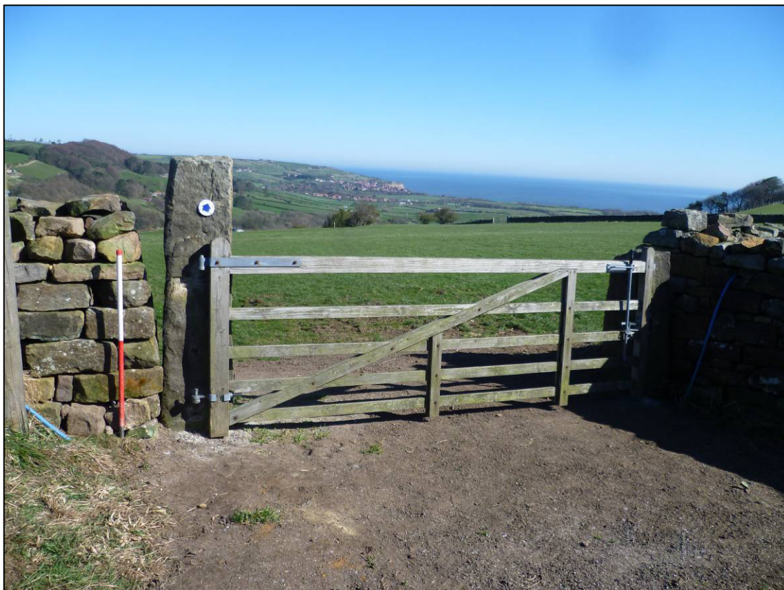
Plate 16: Repaired gateway, looking N (photo 2/344).
