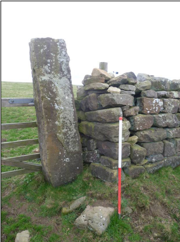
Photo 4: Western wall end and gatepost prior to repair, looking SW (photo 1/298).
