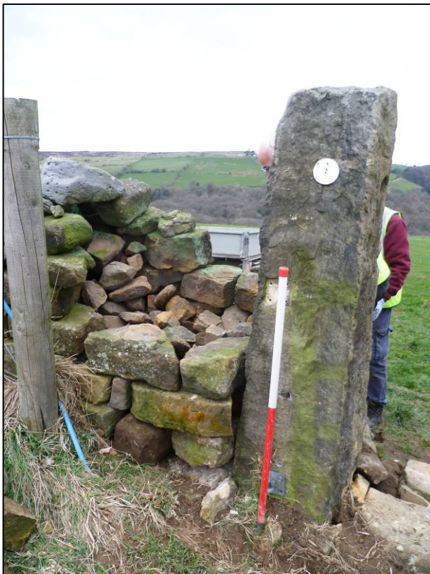
Plate 11: Rebuilding western wall end, looking N (photo 1/314).
