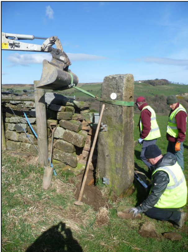
Photo 8: Straightening western gatepost, looking N (plate 1/304).
