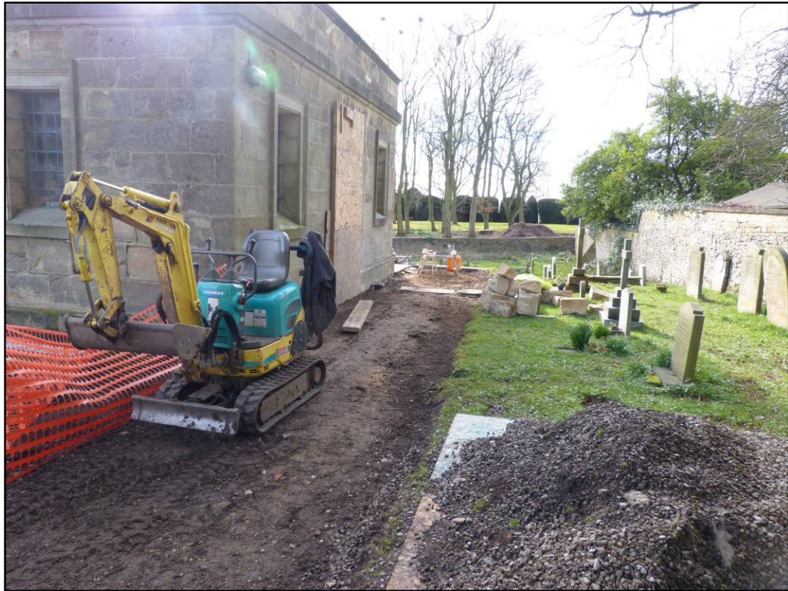
Plate 3: Resurfacing of footpath to west of church, looking south.
