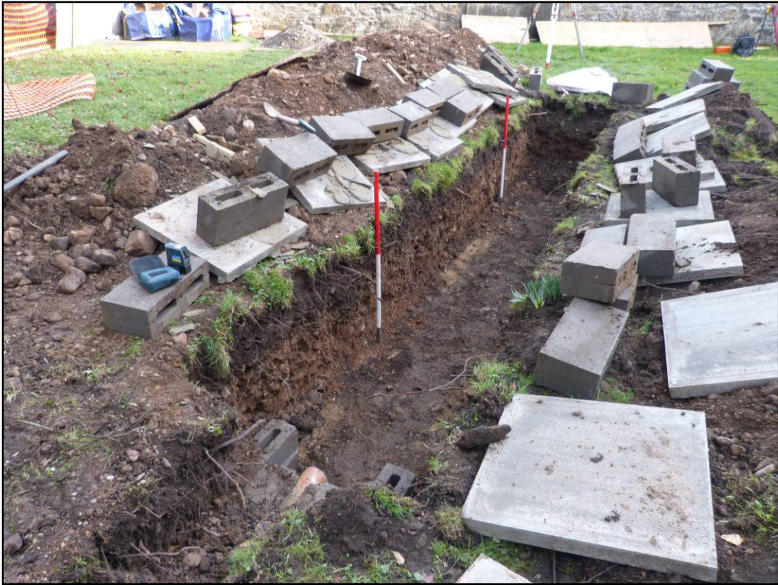
Plate 1: Main drainage trench, north side of church, looking north.
