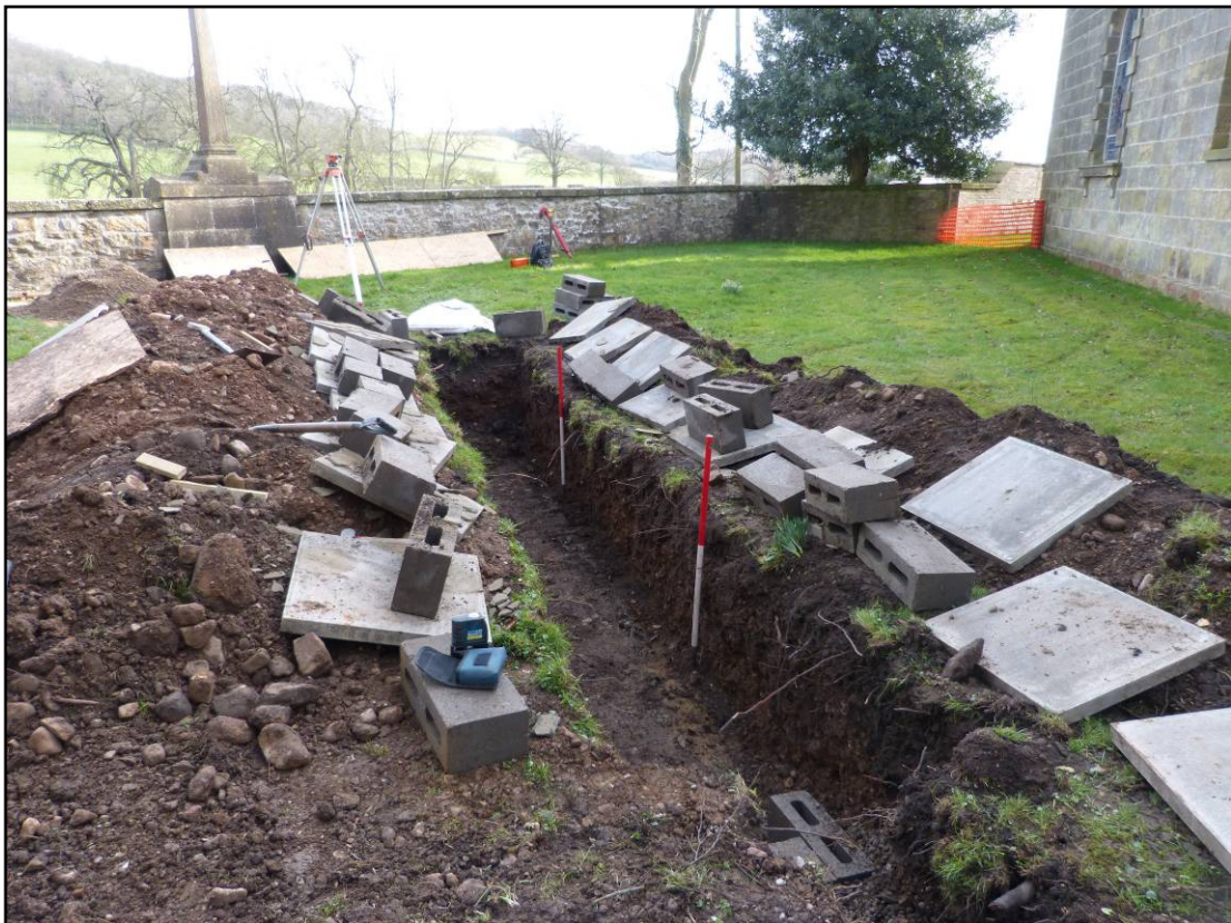
Plate 2: Main drainage trench, north side of church, looking south-east.
