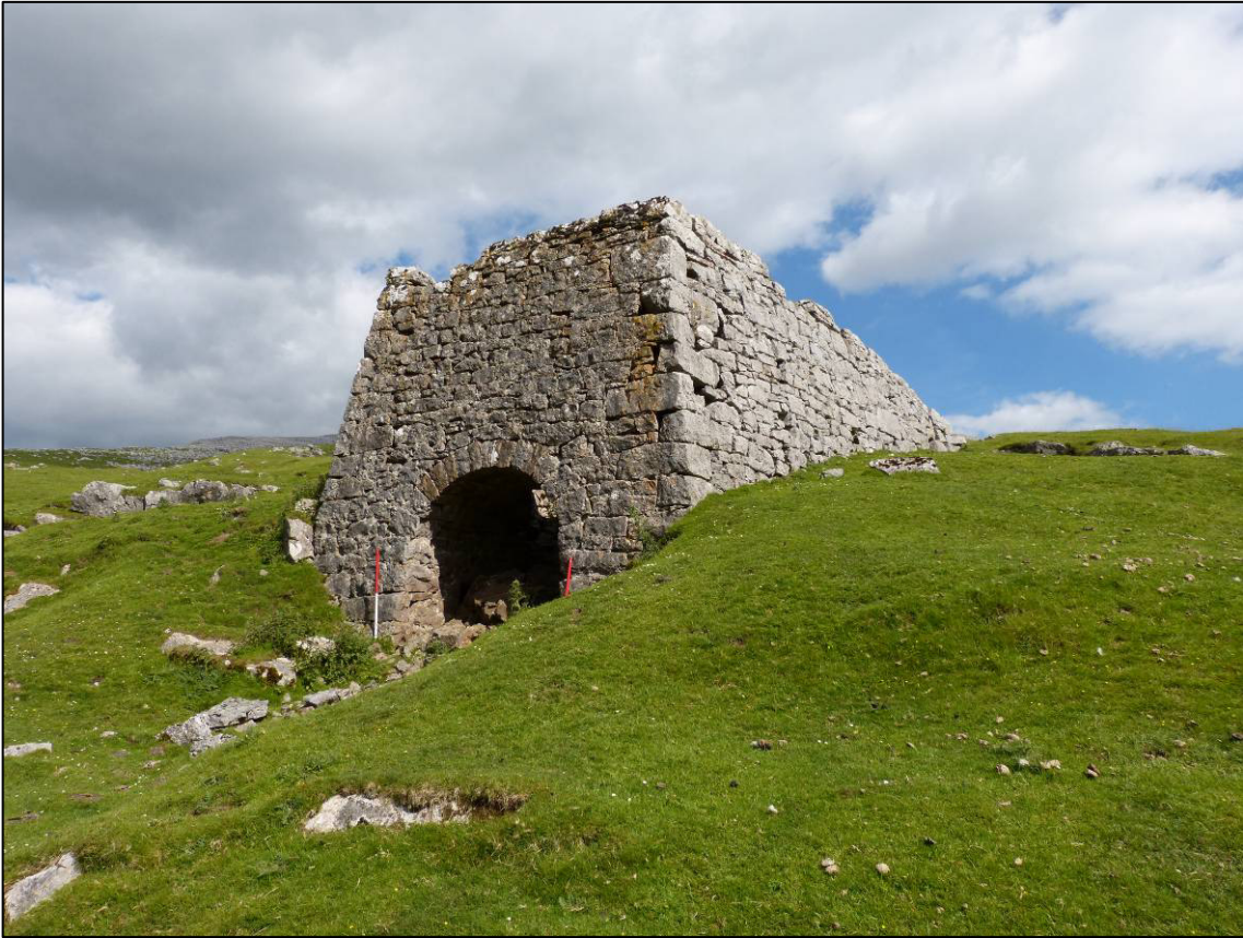
Plate 9: Kiln 2, looking NE (photo 1/141).
