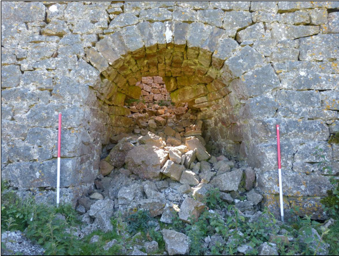
Plate 13: Kiln 2, draw arch in west elevation, looking E (photo 1/122).
