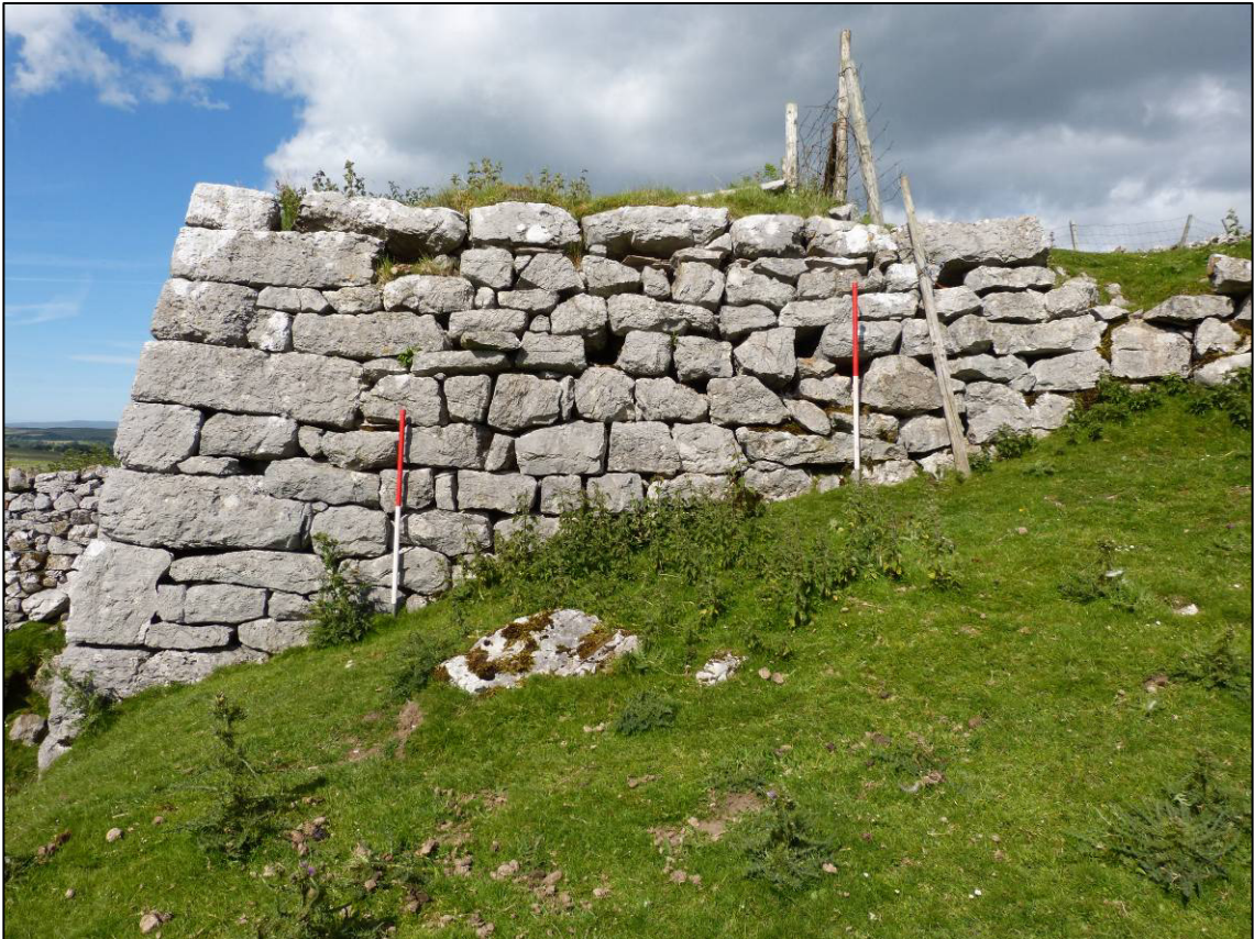
Plate 2: Kiln 1, south elevation, looking N (photo 1/148).
