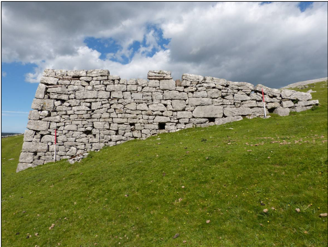
Plate 12: Kiln 2, south elevation, looking N (photo 1/132).
