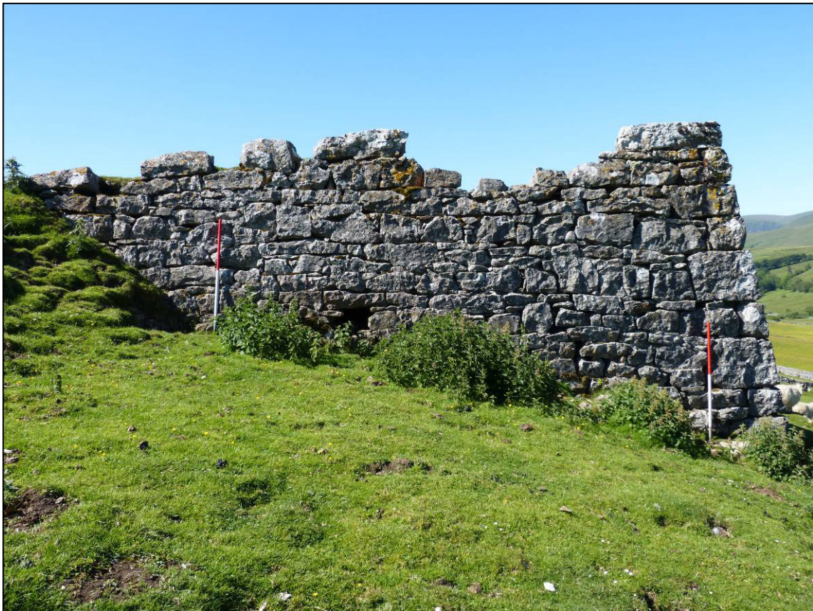
Plate 10: Kiln 2, N elevation, looking S (photo 1/108).
