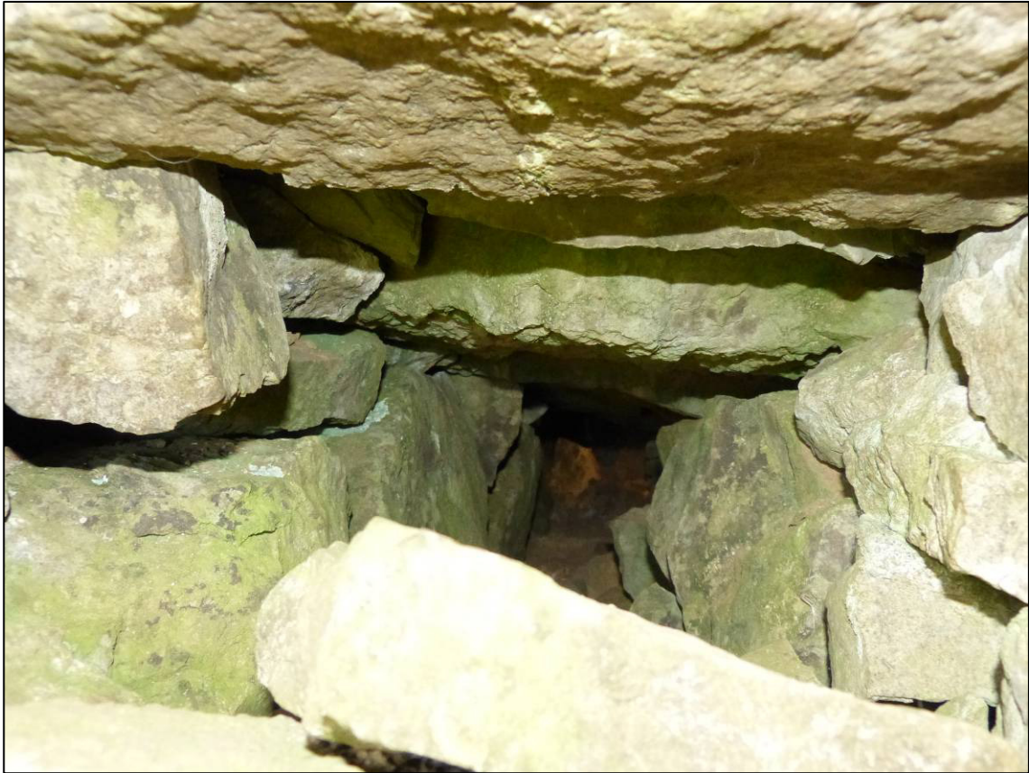
Plate 11: Kiln 2, flue passage in north elevation, looking S (photo 1/143).
