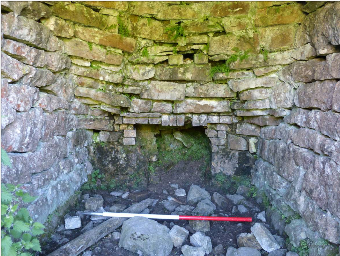
Plate 4: Kiln 1, draw arch interior, looking E (photo 1/105).
