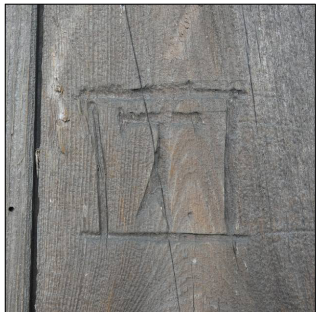
Plate 16: Cart entrance, graffiti to exterior of harrung door, looking NW (photo 1/049).
