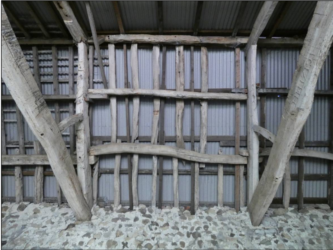
Plate 25: Central bay, north roof slope, looking NW (photo 1/102).
