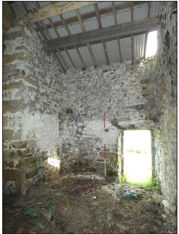
Plate 22: Internal south wall, west part, looking SE (photo 1/064).
