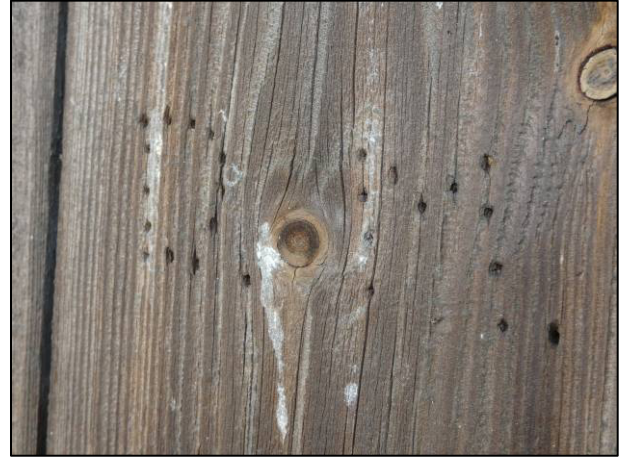
Plate 18: Cart entrance, graffiti to exterior of harr-hung door, looking NW (photo 1/051).
