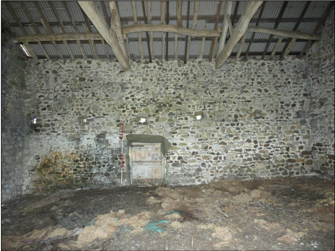
Plate 20: Internal north wall, looking NW (photo 1/079).
