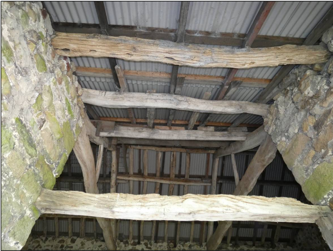
Plate 14: Roof structure over cart entrance, looking NW (photo 1/062).
