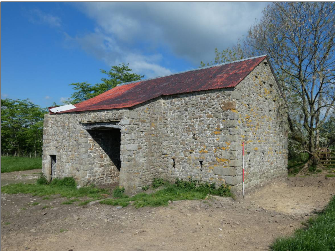
Plate 2: South elevation and east gable, looking W (photo 1/006).
