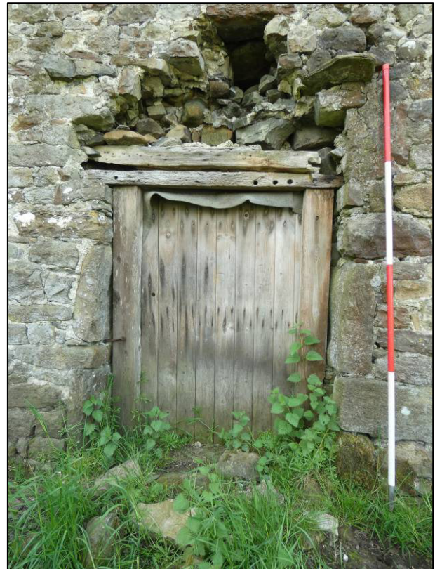
Plate 7: North elevation, low doorway, looking SE (photo 1/021).
