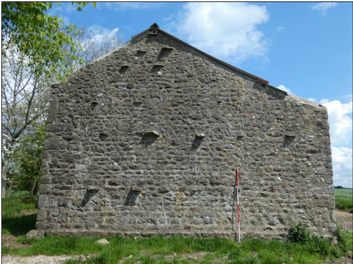
Plate 10: West gable, looking NE (photo 1/041).
