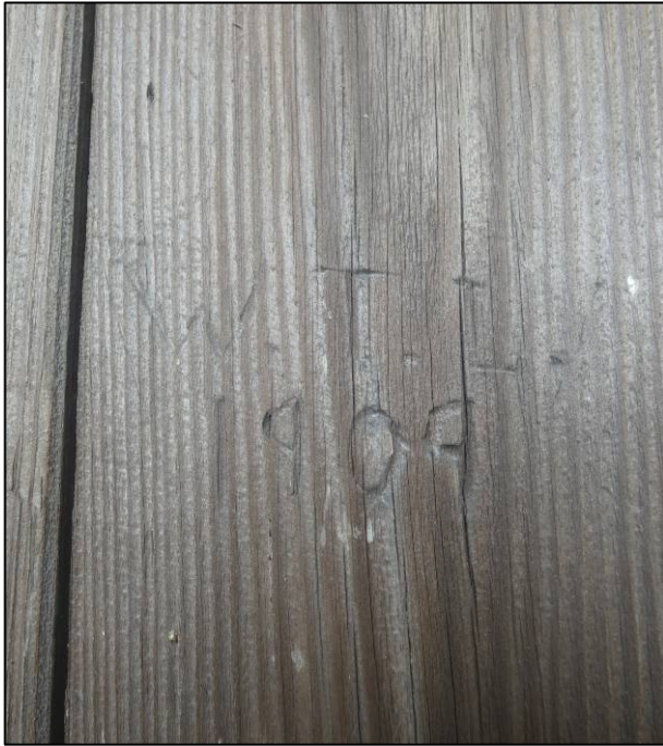
Plate 17: Cart entrance, graffiti to exterior of harr-hung door, looking NW (photo 1/050).
