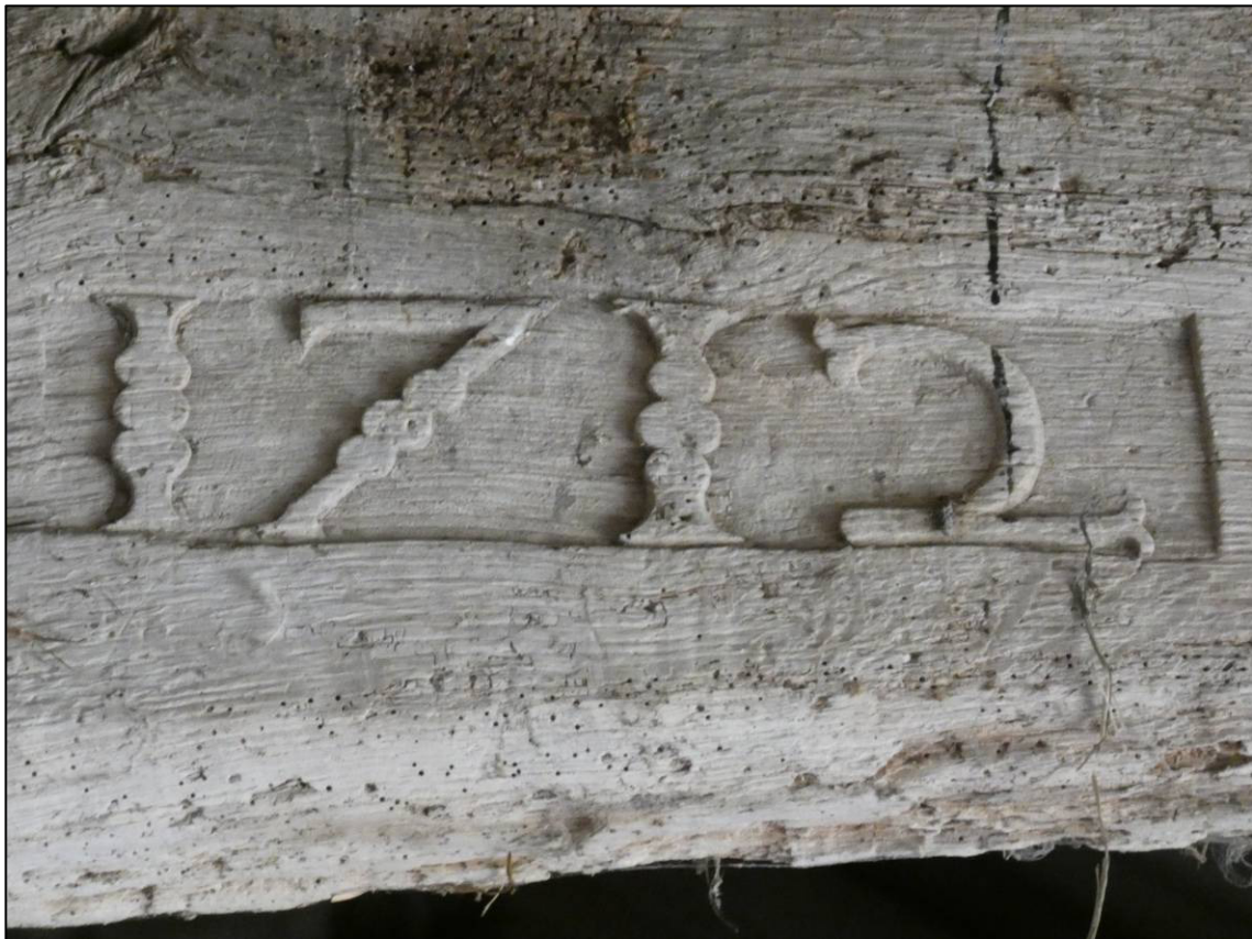
Plate 28: East roof truss, west face, inscription ('1712'), looking NE (photo 1/101).
