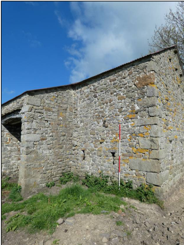
Plate 12: South elevation, east of cart entrance, looking W (photo 1/009).
