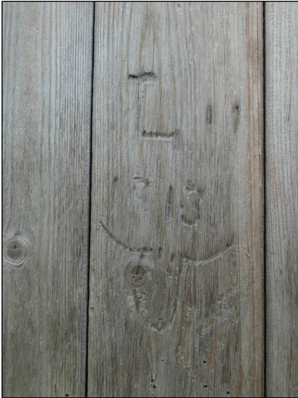
Plate 8: North elevation, graffiti to exterior of doorway, looking SE (photo 1/027).
