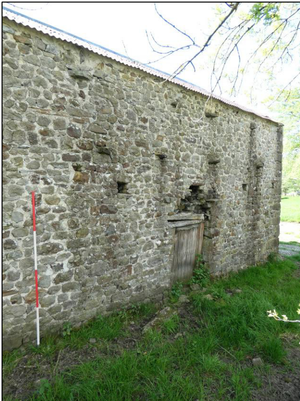
Plate 6: North elevation, looking S (photo 1/025).
