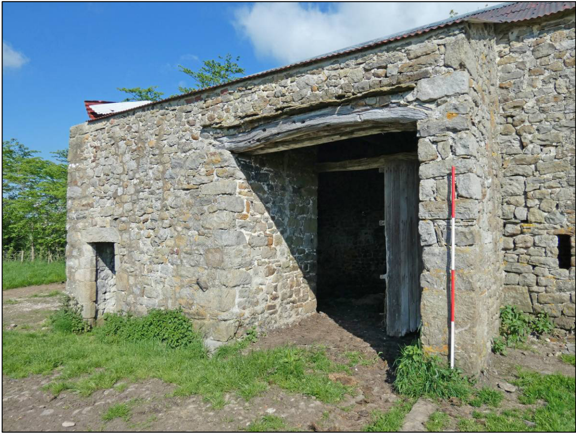
Plate 11: South elevation, projecting west part, looking W (photo 1/012).
