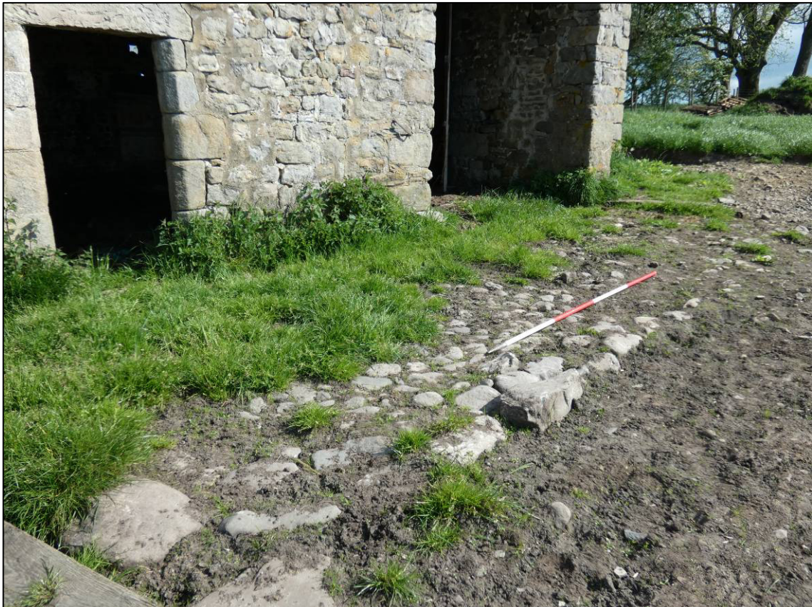
Plate 4: Yard and cobbled surfaces to south of barn, looking NE (photo 1/030).
