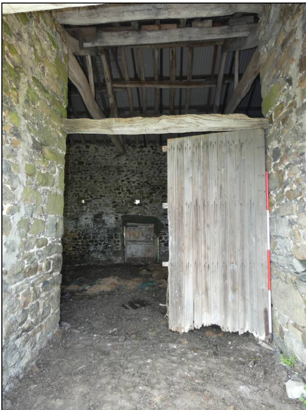
Plate 15: Cart entrance, doorway, looking NW (photo 1/048).
