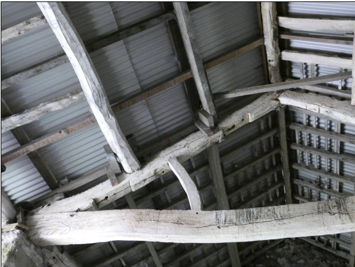
Plate 24: West roof truss, east face, south end, looking SW (photo 1/106).
