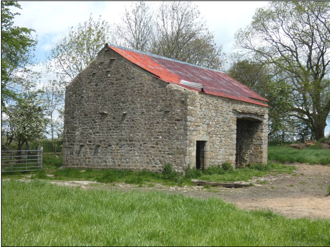
Plate 3: General view to barn, looking N (photo 1/034).
