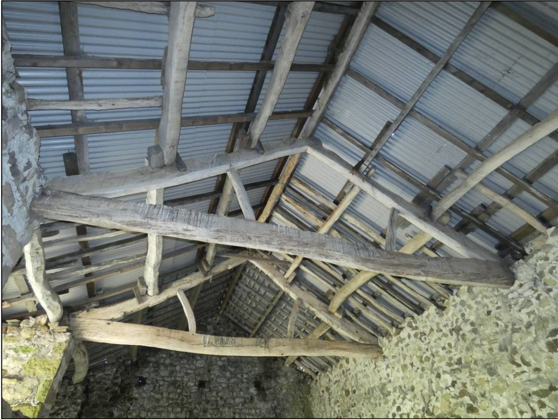
Plate 23: Roof trusses, east faces, looking SW (photo 1/092).
