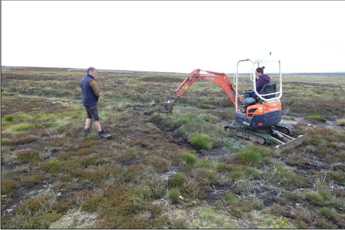
Plate 5: Area 3 - start of drain excavation, looking NE (photo 1/693).
