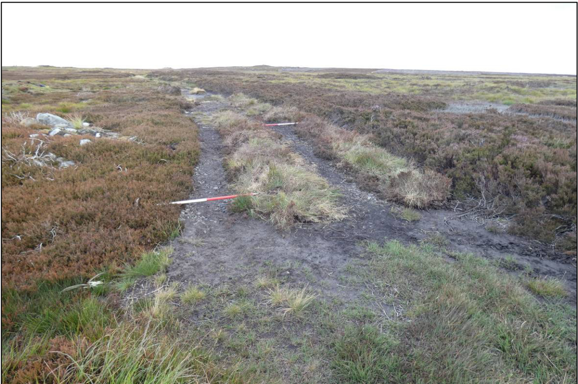
Plate 12: Area 6 - repairs to ruts complete with re-turving, looking N (photo 2/868).
