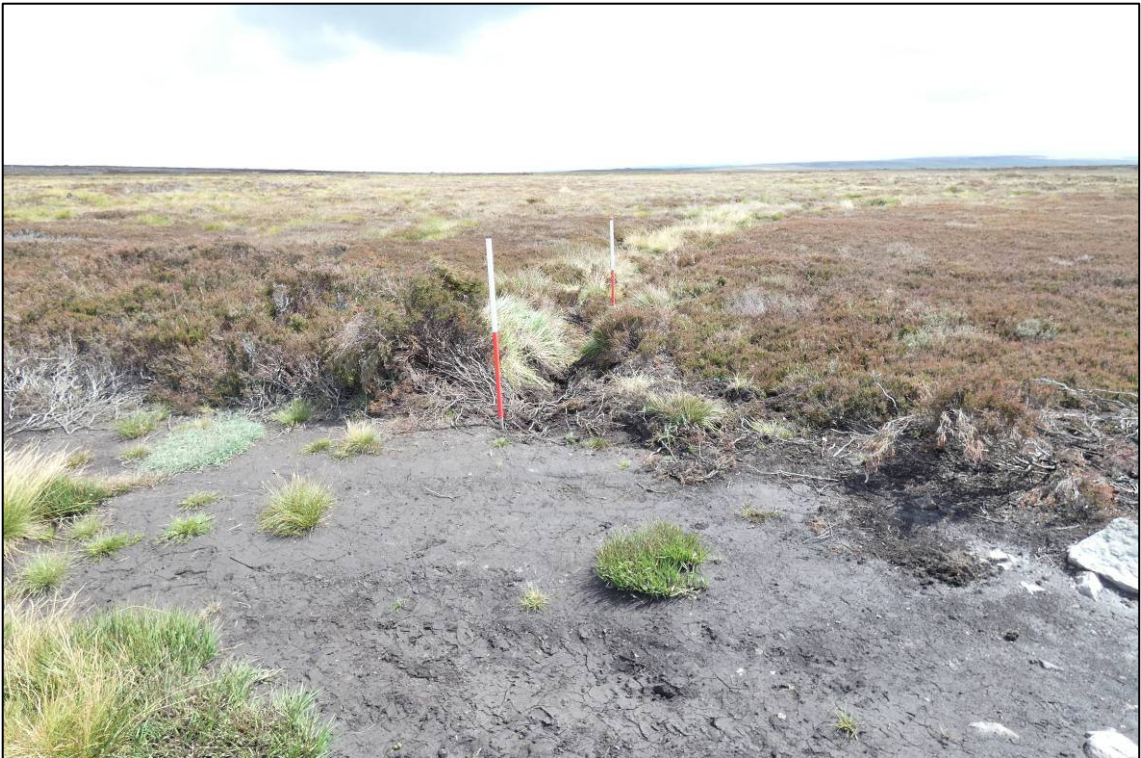
Plate 14: Area 7 - drain complete, looking E (photo 2/871).
