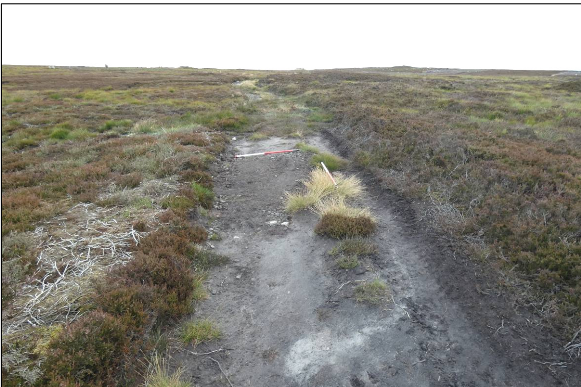
Plate 8: Area 4 - repairs complete, looking N (photo 2/858).
