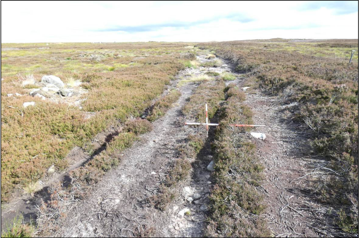
Plate 11: Area 6 - vehicle ruts prior to repair, looking N (photo 1/684).
