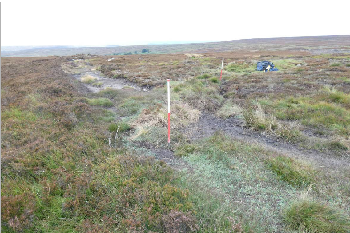
Plate 6: Area 3 - drain and bank across track complete, looking SW (photo 2/854).
