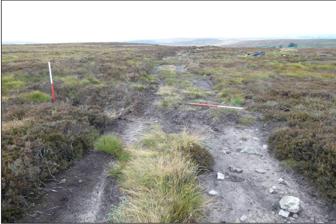
Plate 3: Area 1 - drain and bank across track complete, looking S (photo 2/849).
