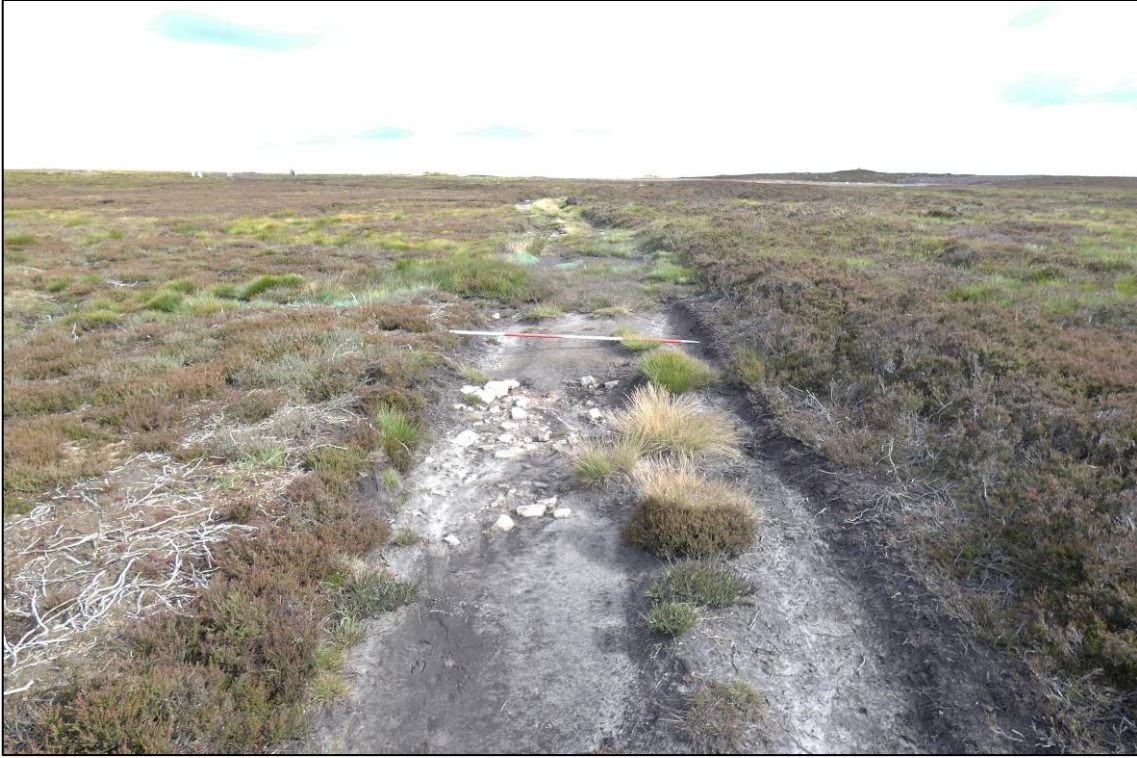
Plate 7: Area 4 - stone rubble in track prior to repairs, looking N (photo 1/678).
