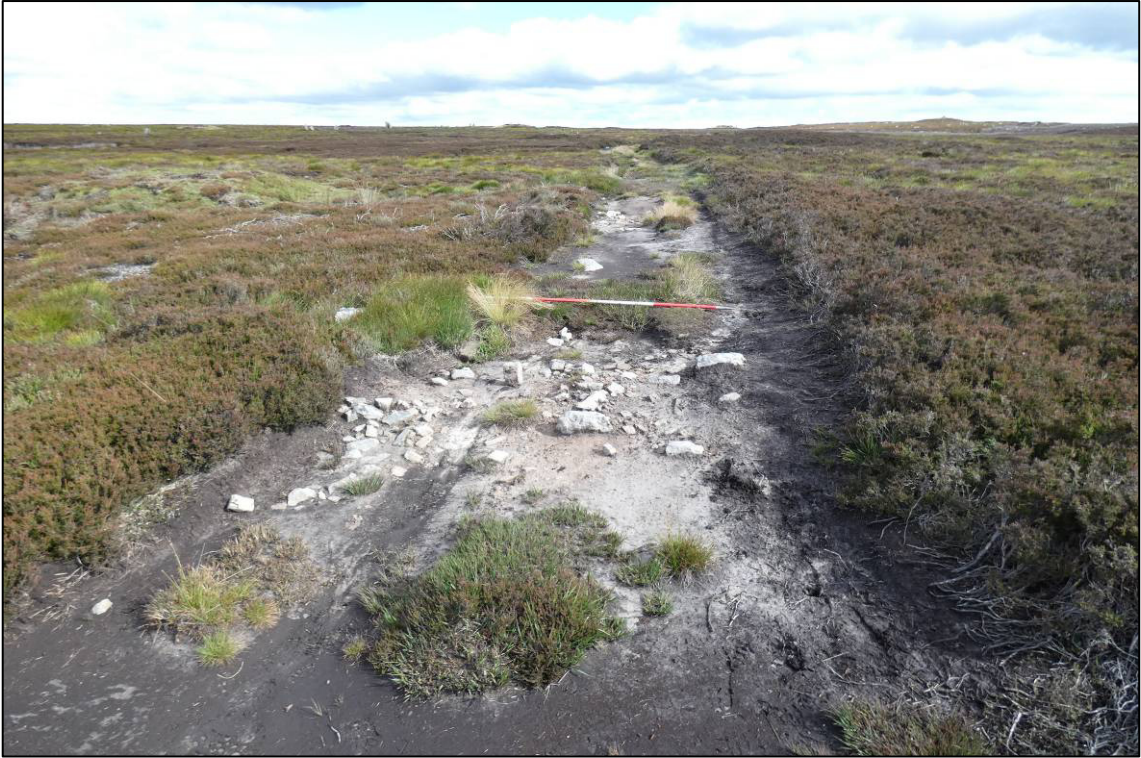
Plate 9: Area 5 - stone rubble in track prior to repairs, looking N (photo 1/677).
