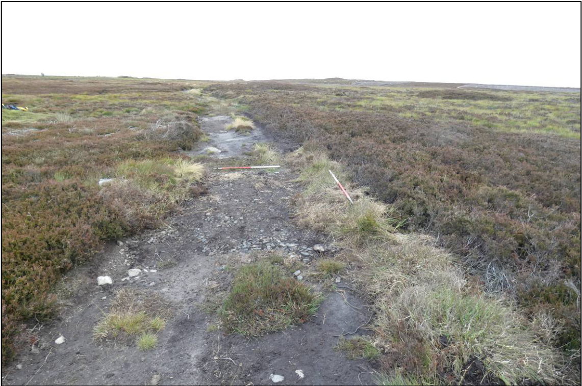
Plate 10: Area 5 - repairs complete, looking N (photo 2/862).
