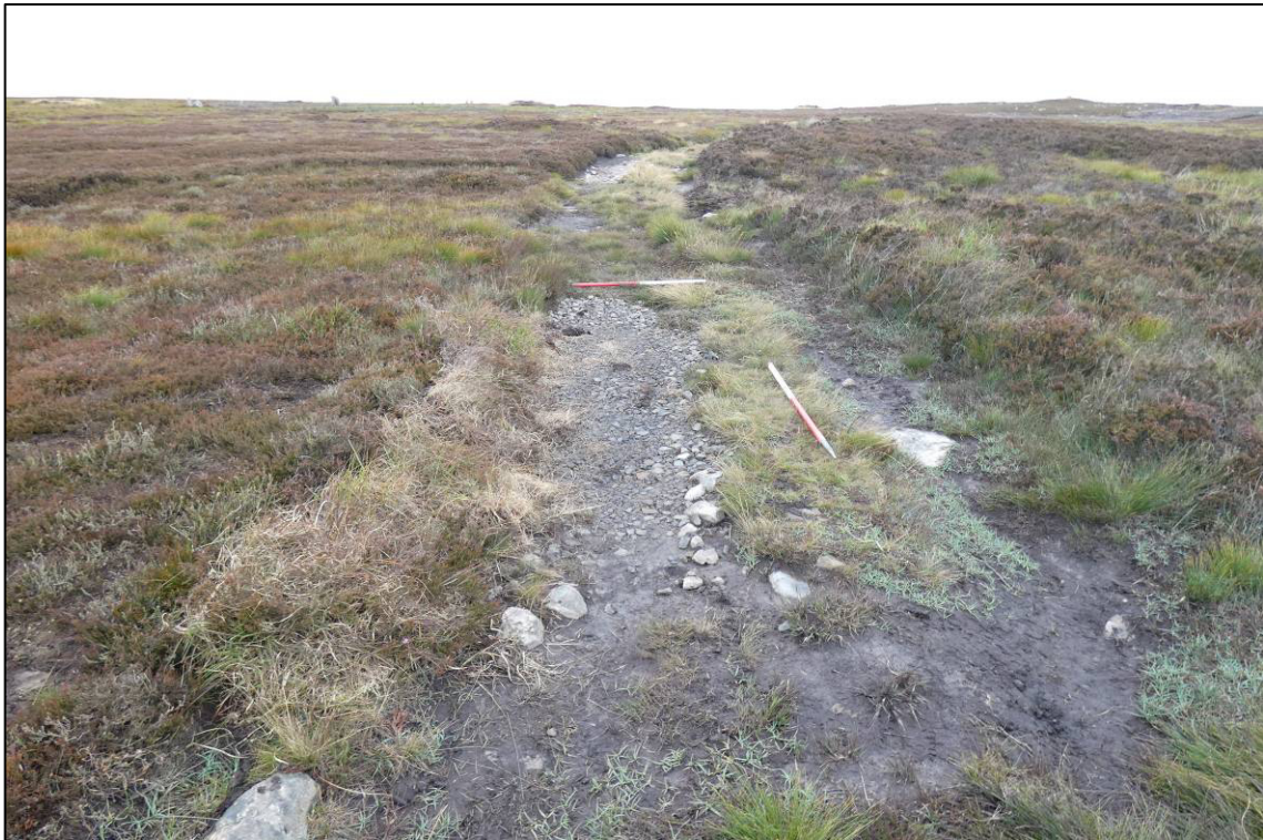
Plate 4: Area 2 - infilling of ruts complete, looking N (photo 2/852).
