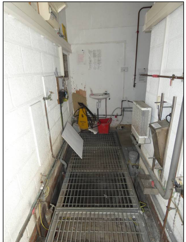
Plate 10: No. 48 Newborough (public conveniences), ground floor plant area, looking W.
