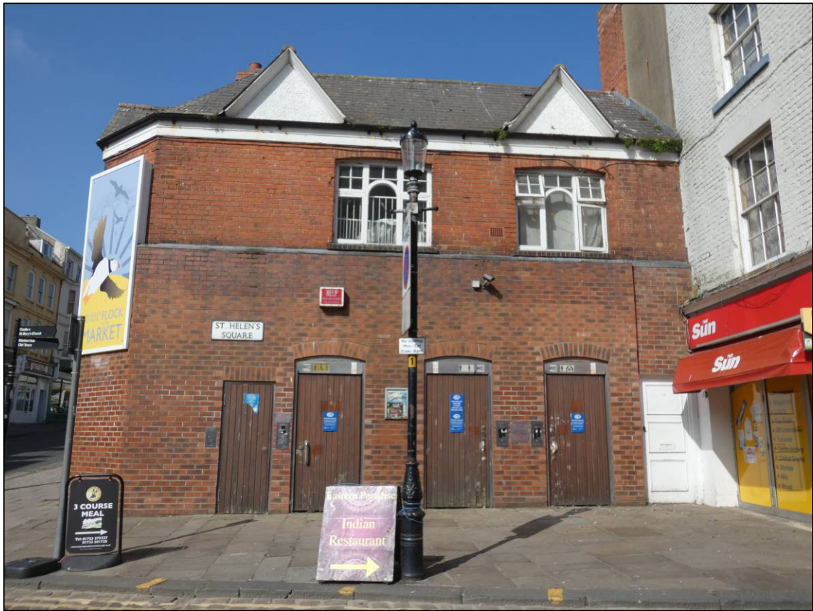
Plate 11: No. 48 Newborough (public conveniences), east elevation, looking W.
