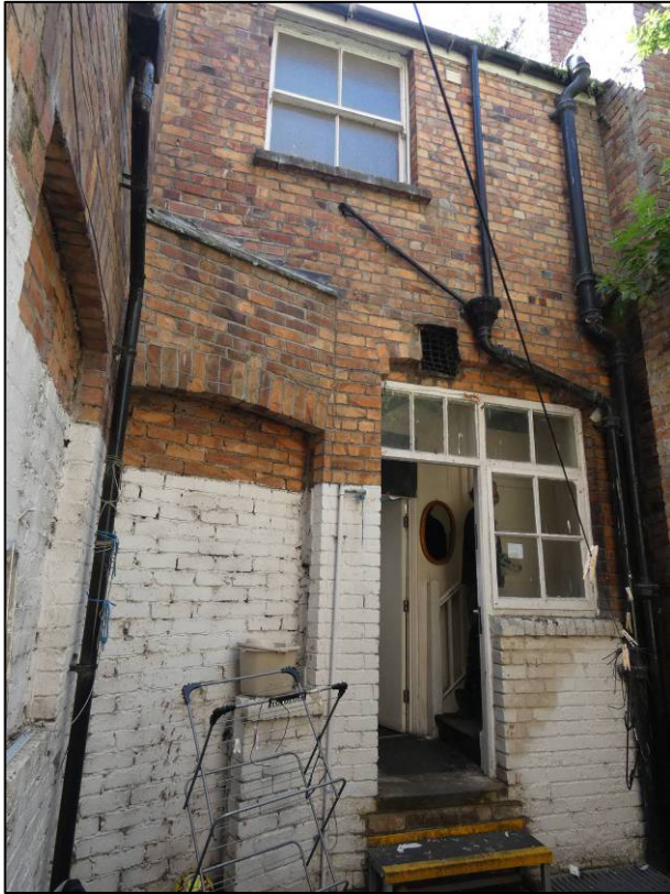
Plate 15: No. 49 Newborough, north elevation from rear yard, looking S.
