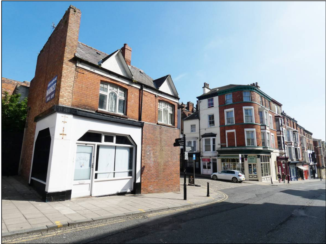
Plate 6: Nos 48-49 Newborough and south-east corner buildings of St Helen's Square, looking E.
