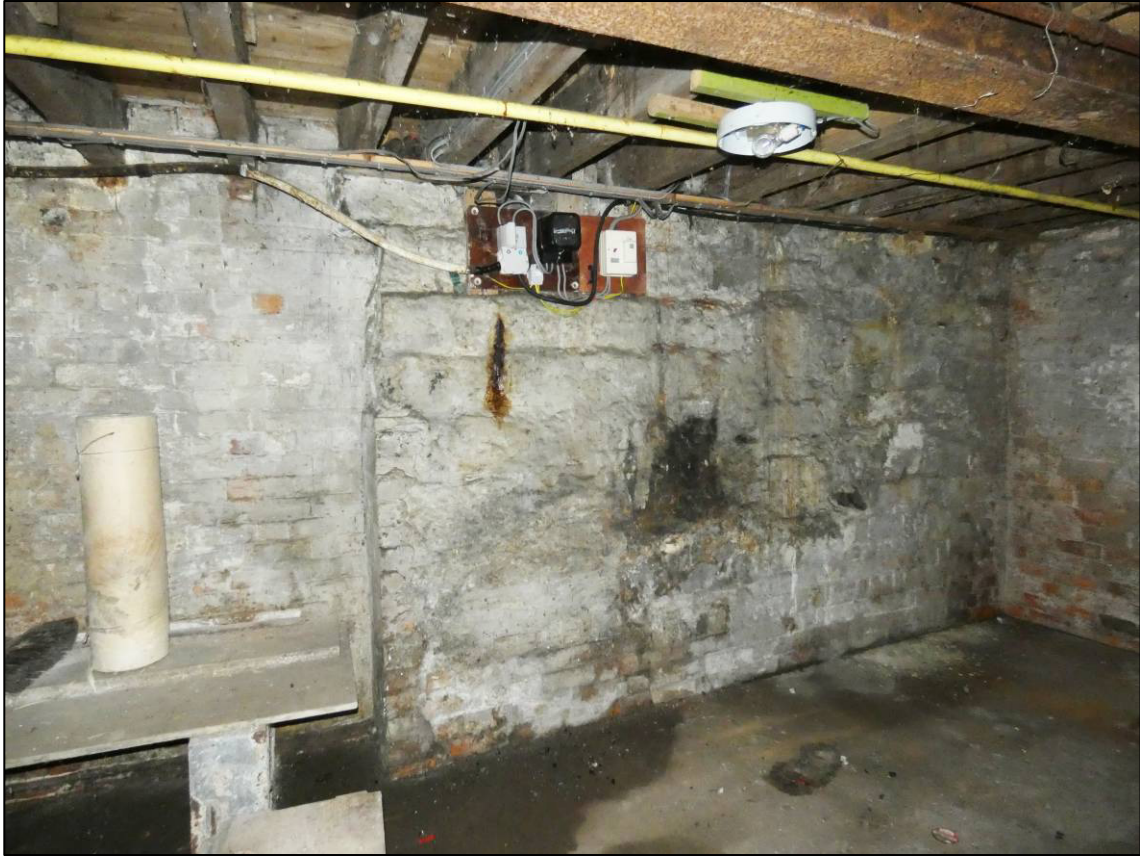
Plate 13: No. 49 Newborough, cellar, showing stonework to west wall, looking NW.
