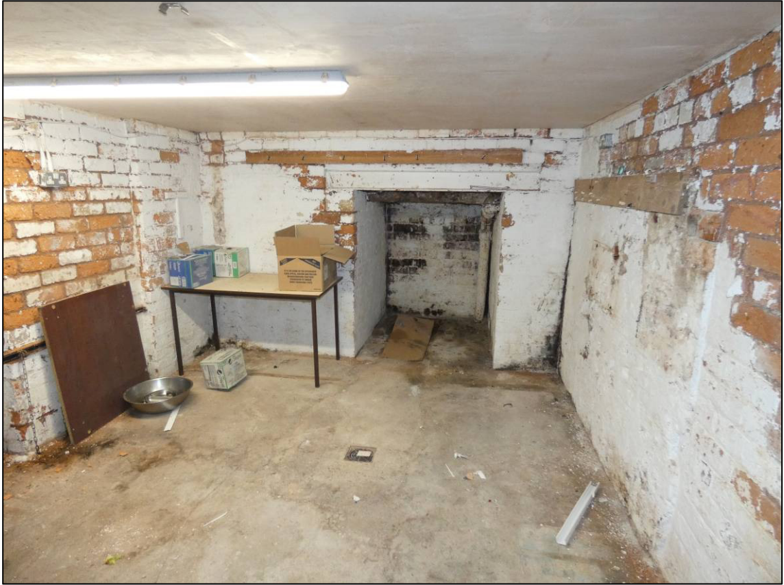
Plate 30: No. 2 St Helen's Square (The Shakespeare Hotel), cellar, looking E.
