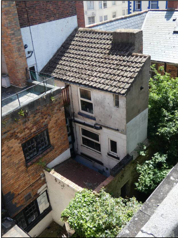
Plate 18: No. 1 St Helen's Square, north elevation of rear wing, looking SE.
