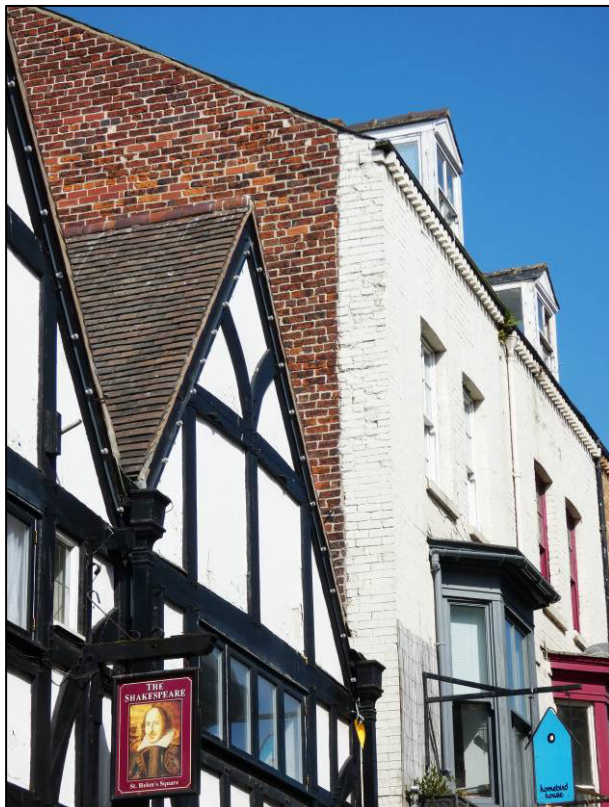
Plate 4: No. 4 St Helen's Square, south elevation upper part, showing staggered joint, looking N.
