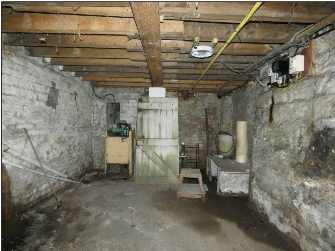
Plate 12: No. 49 Newborough, cellar, looking S.
