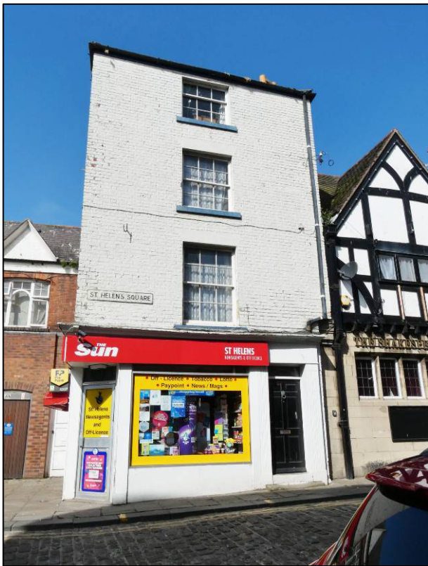
Plate 20: No. 1 St Helen's Square, east elevation, looking W.
