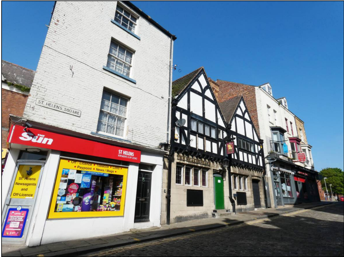
Plate 24: St Helen's Square, west side, looking NW.
