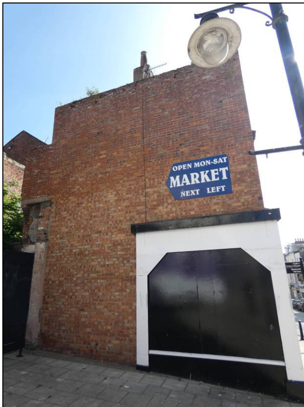
Plate 9: West elevation of no. 49 Newborough, looking E.
