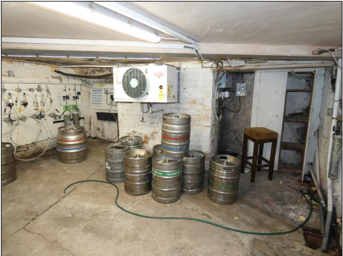
Plate 31: No. 3 St Helen's Square (The Shakespeare Hotel), cellar, looking N.
