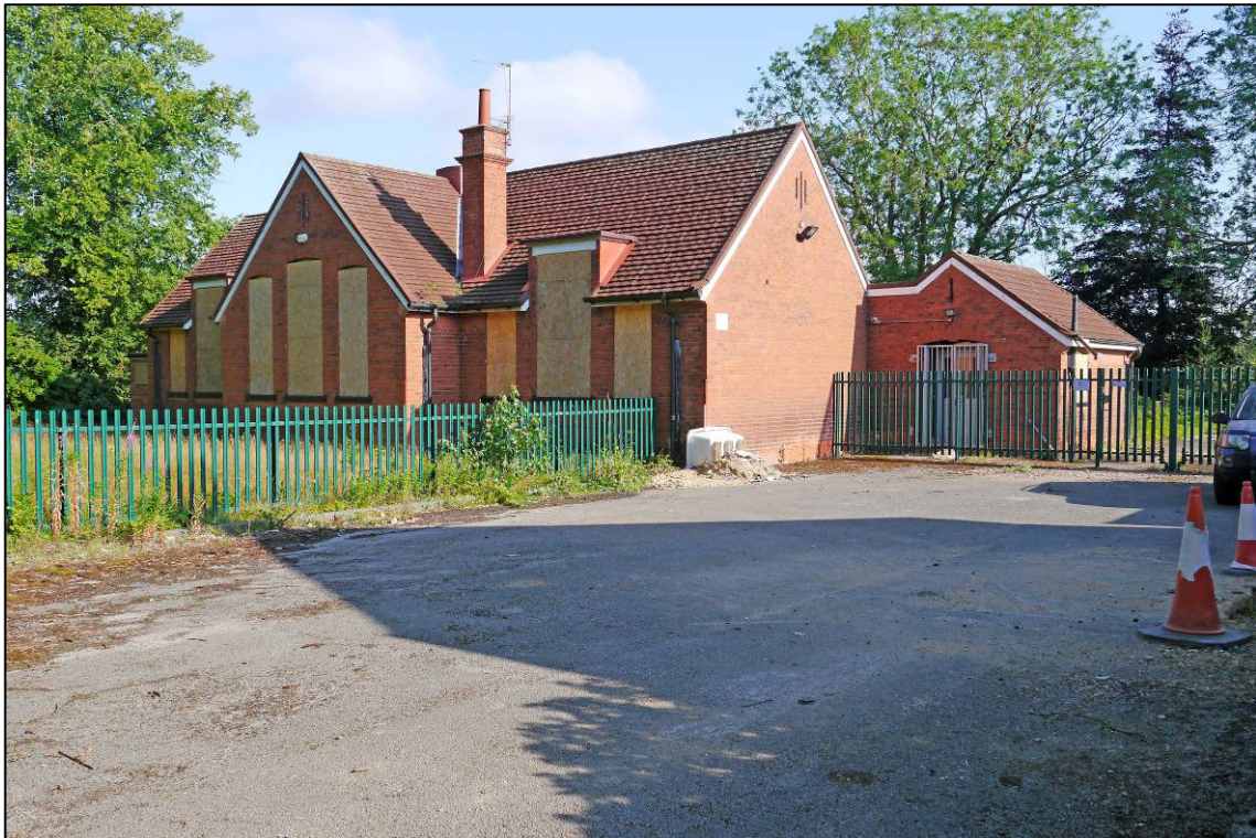
Plate 2: 1911 school building (Block 1), south and east elevations, looking N (photo 1/217).
