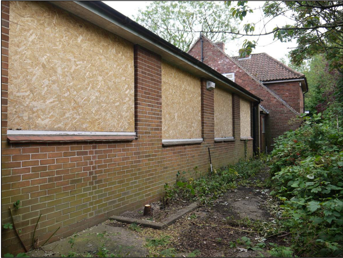
Plate 42: 1960 kitchen and dining block (Block 4), west elevation, looking S (photo 1/175).
