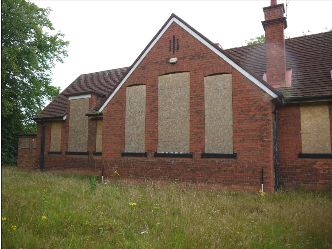
Plate 9: 1911 school building (Block 1), central projection to south elevation, looking N (photo 1/139).
