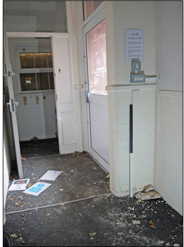
Plate 18: 1911 school building (Block 1), east end of internal corridor (G/001), former girls' entrance, looking SE (photo 1/003).
