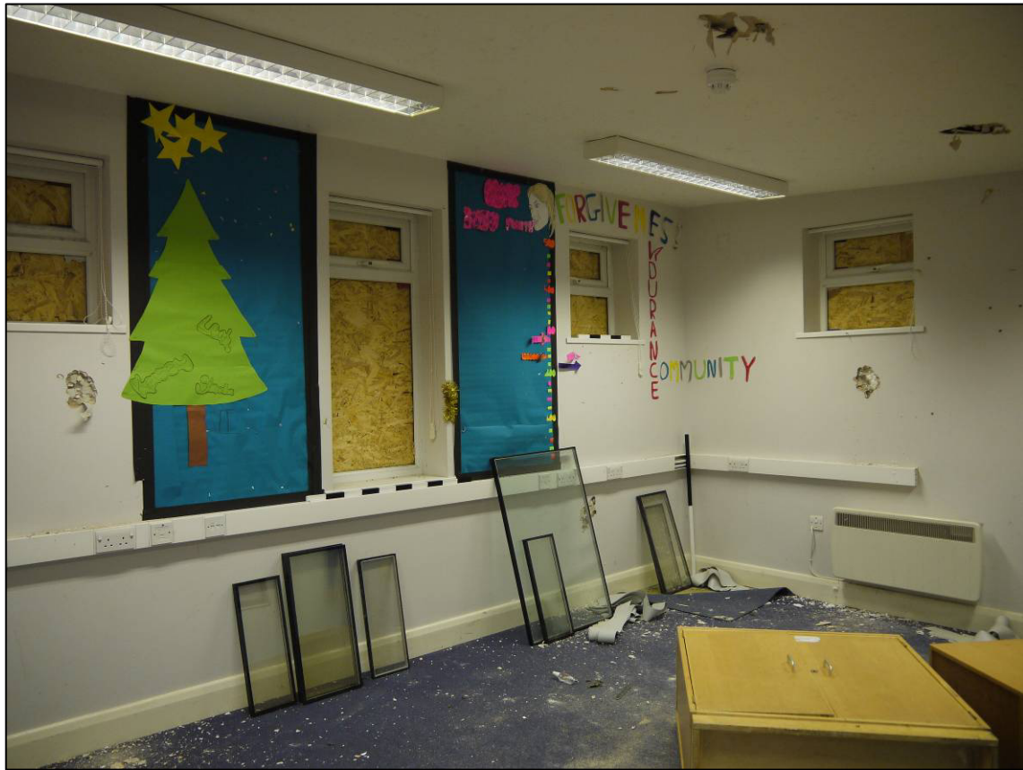
Plate 29: 1970s classroom (Block 2), interior, looking E (photo 1/108).
