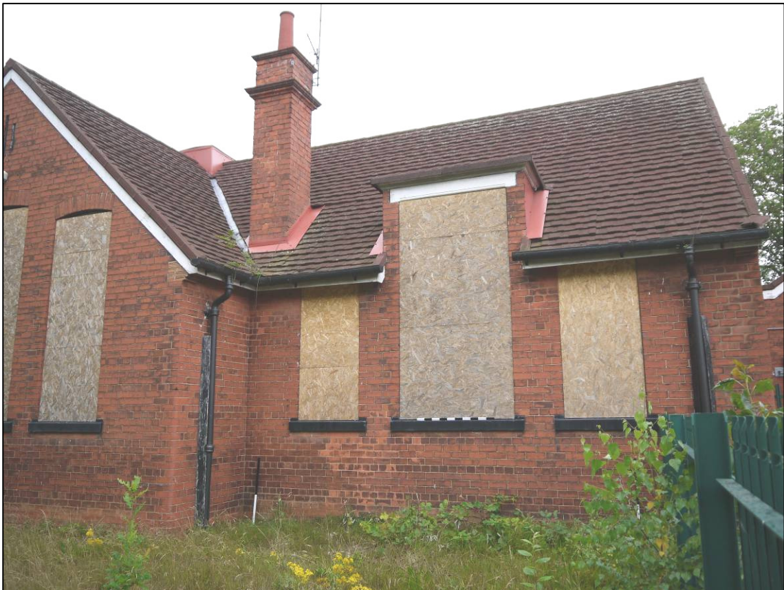
Plate 8: 1911 school building (Block 1), east end of south elevation, looking N (photo 1/143).
