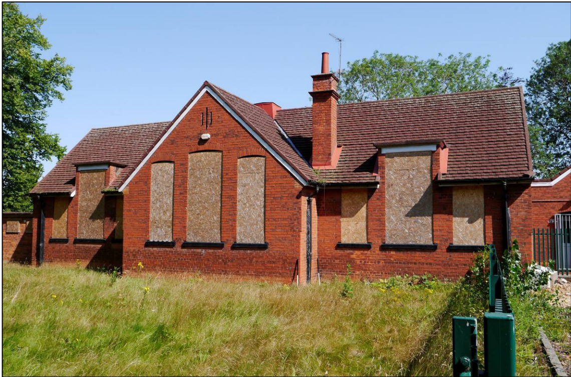
Plate 7: 1911 school building (Block 1), south elevation, looking N (photo 1/154).
