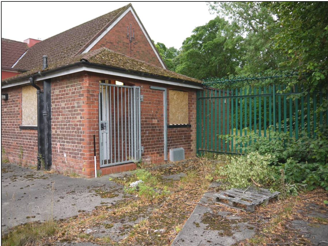
Plate 16: 1911 school building (Block 1), west elevation with former boys' entrance, looking S (photo 1/121).
