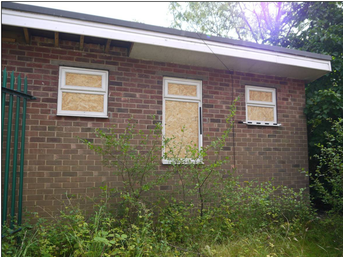
Plate 28: 1970s classroom (Block 2), north elevation, looking W (photo 1/155).
