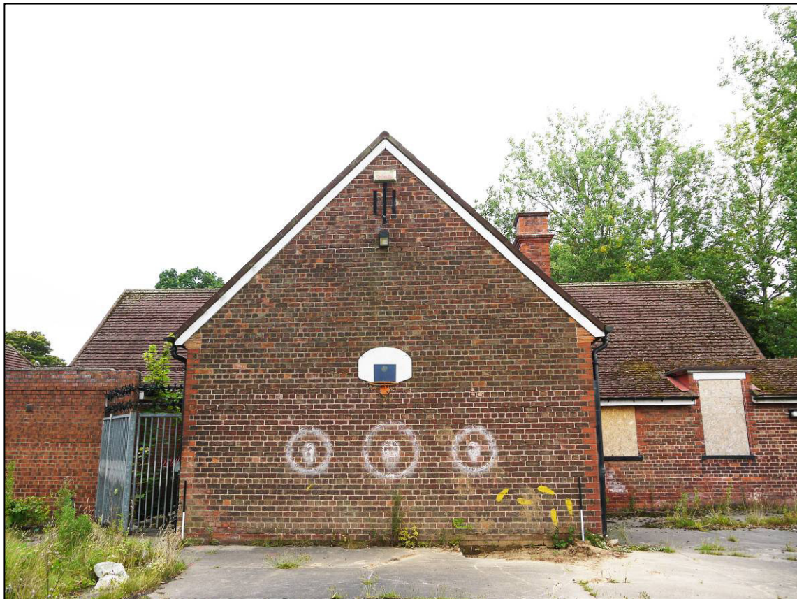
Plate 12: 1911 school building (Block 1), central projection to north elevation, looking SW (photo 1/125).
