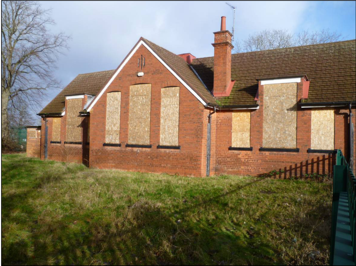
Plate 1: Main School Building (Block 1), front elevation, looking NW.
