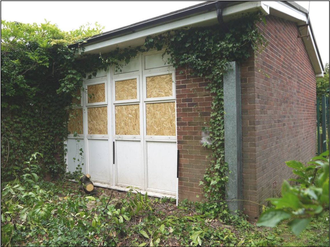
Plate 50: 1955 classroom block (Block 5), east end of south elevation, looking N (photo 1/192).
