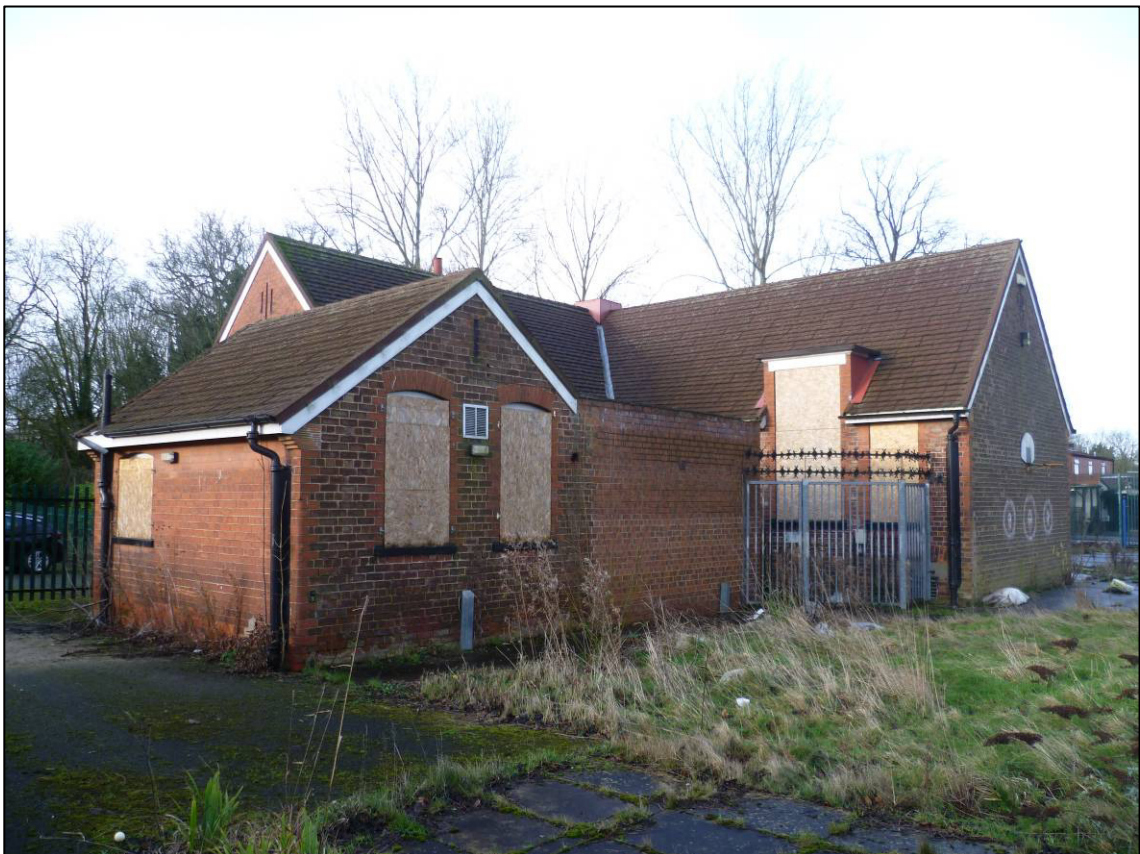
Plate 2: Main School Building (Block 1), rear elevations, looking SW.
