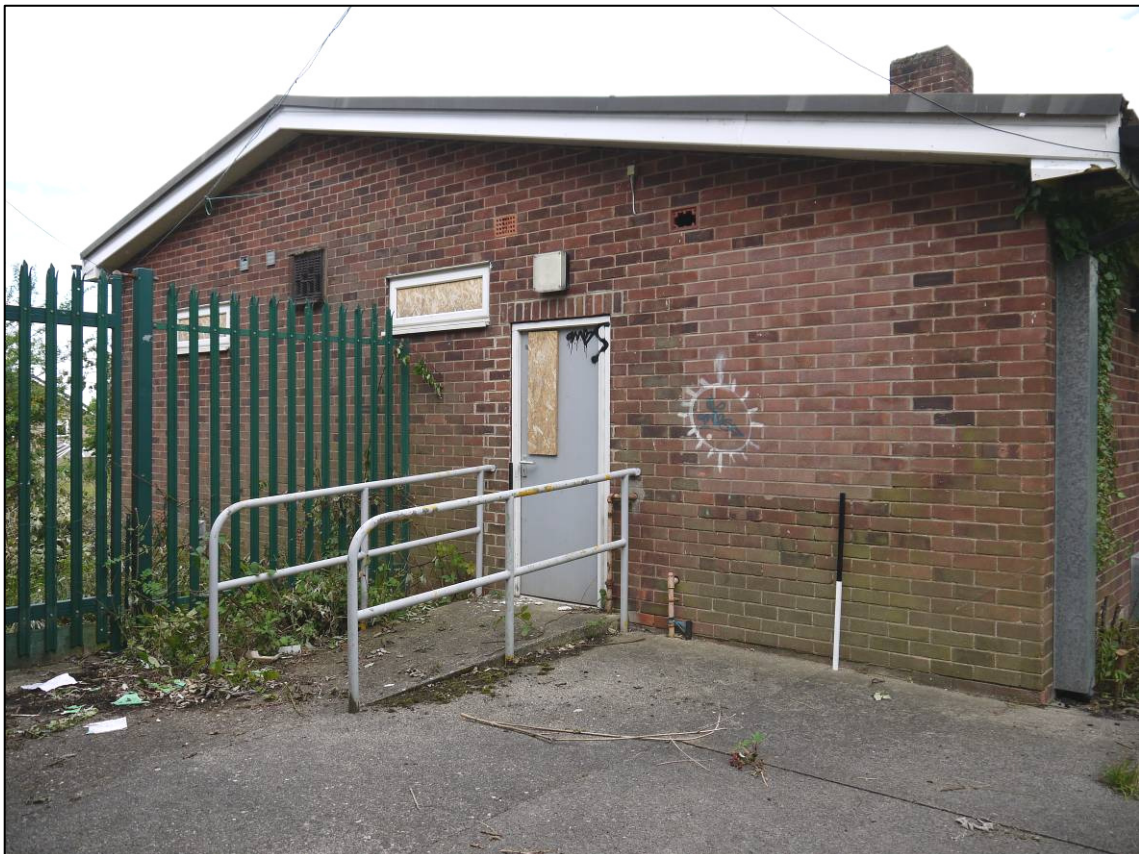
Plate 49: 1955 classroom block (Block 5), west elevation, looking E (photo 1/187).
