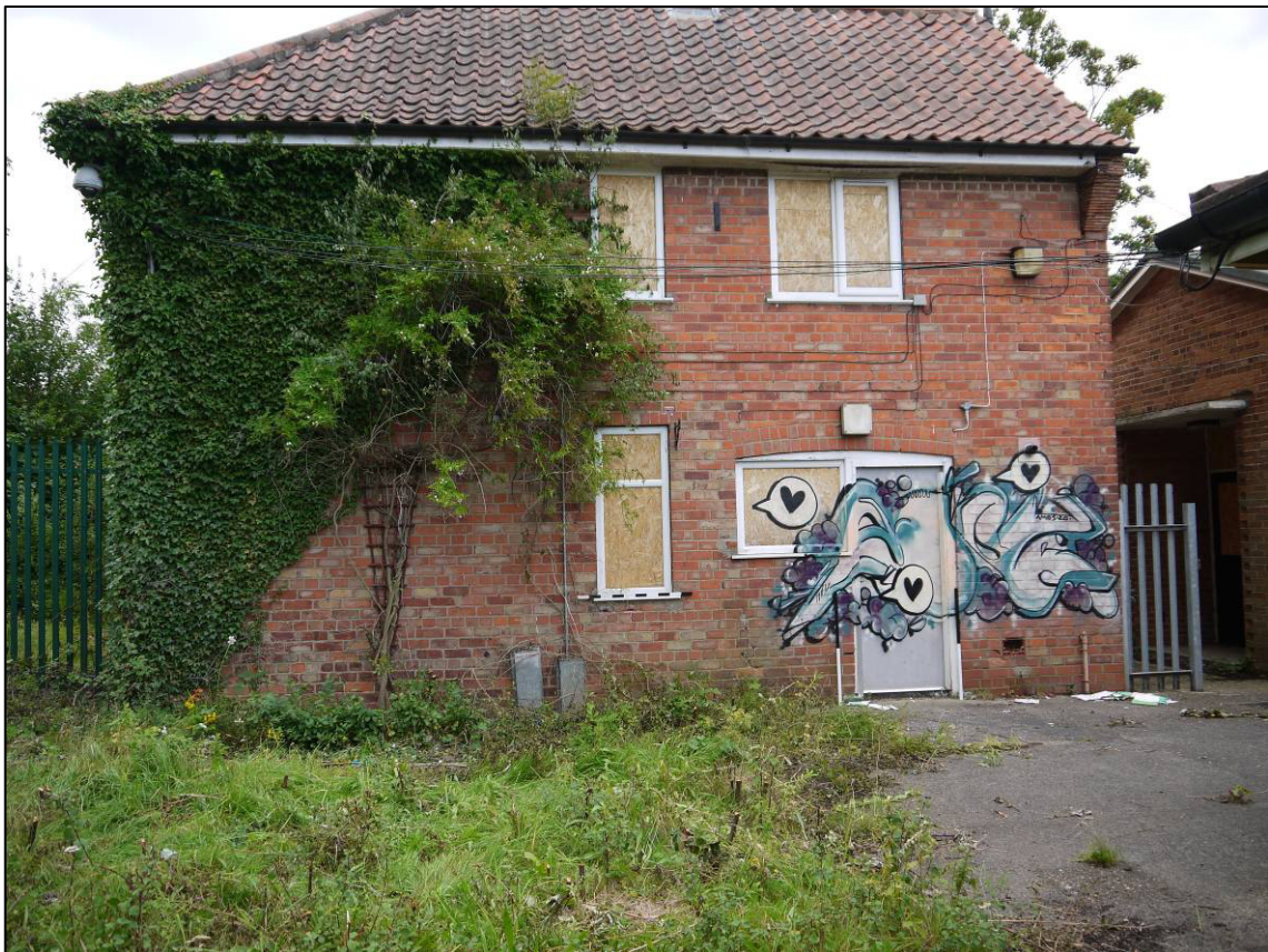
Plate 33: 1923 house (Block 3), east elevation, looking NW (photo 1/169).
