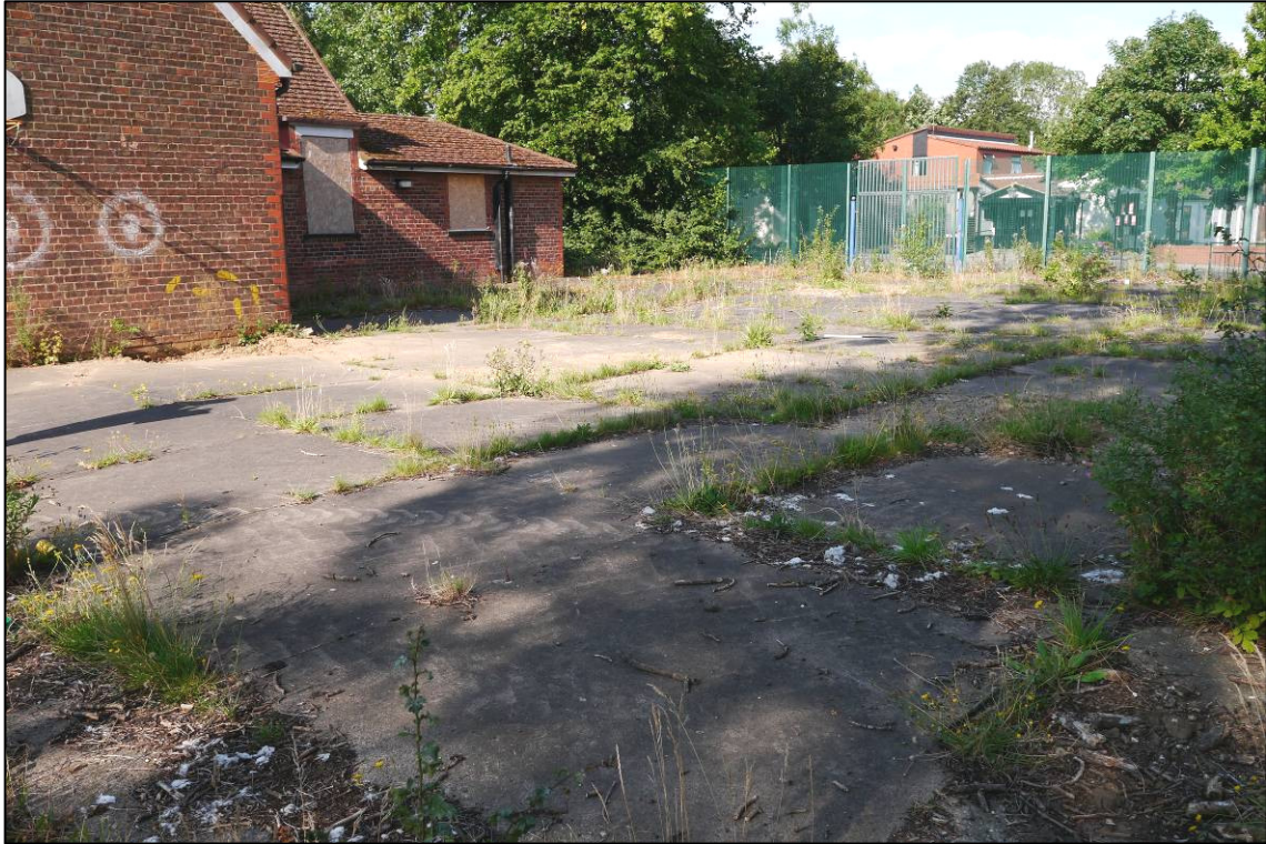
Plate 3: Boys' playground to north of 1911 school building (Block 1), looking N (photo 1/207).
