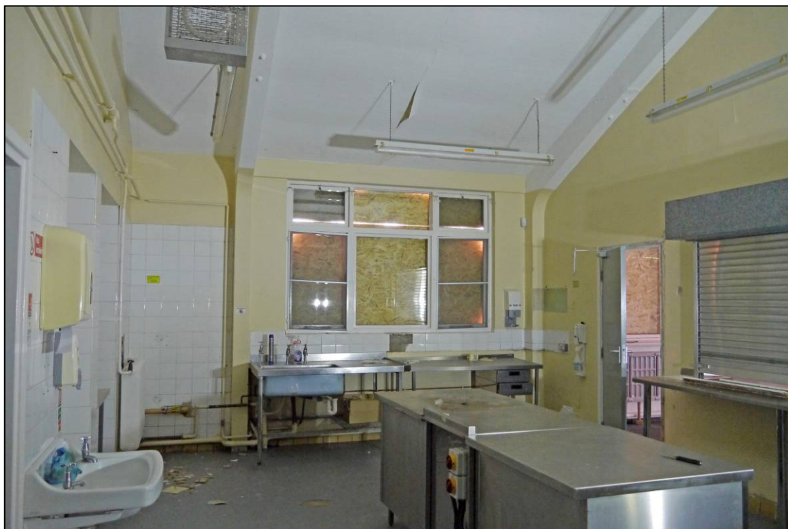
Plate 47: 1960 kitchen and dining block (Block 4), kitchen (G/002), looking SE (photo 1/080).
