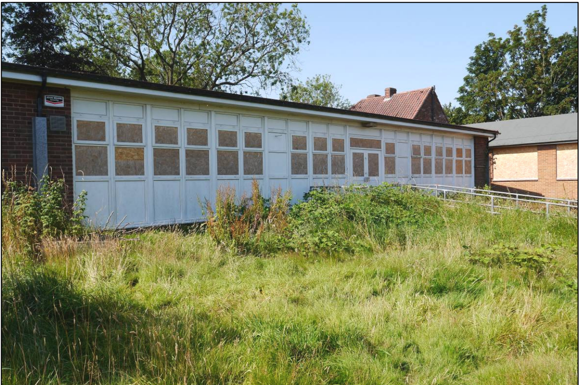
Plate 51: 1955 classroom block (Block 5), north elevation, looking S (photo 1/198).
