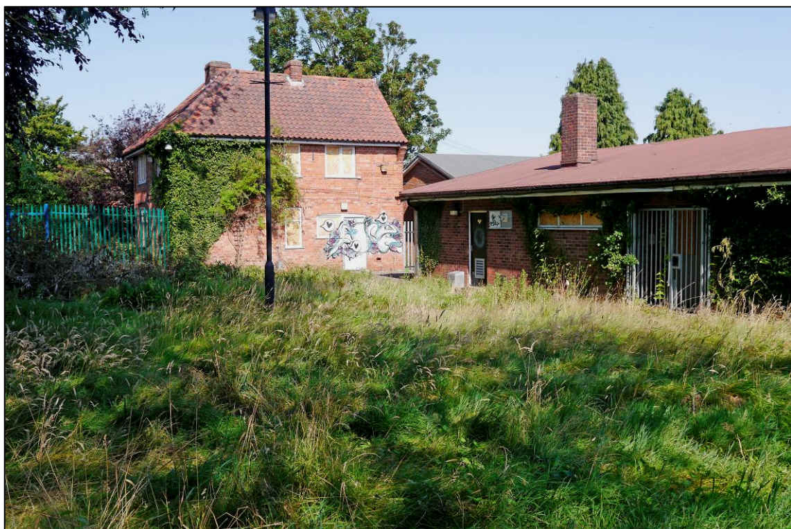
Plate 30: General view of 1923 house (Block 3) and 1955 classrooms (Block 5), looking N (photo 1/174).
