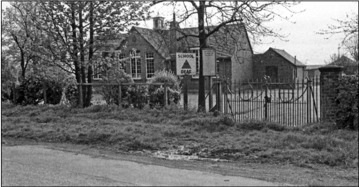
View of Sutton School for the Deaf, showing front elevation and entrance gates, looking NE from Saltshouse Road, c.1964.
