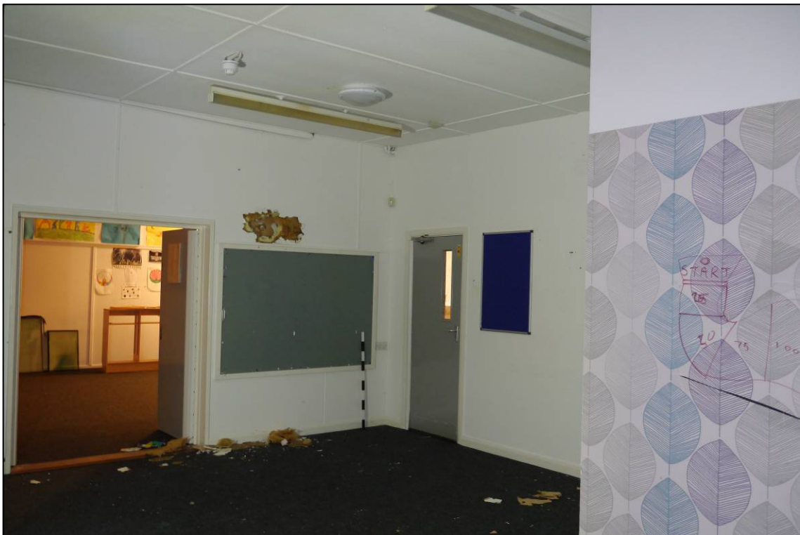
Plate 55: 1955 classroom block (Block 5), classroom (G/008), looking S (photo 1/098).
