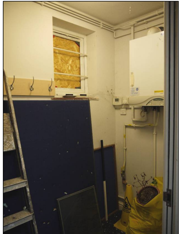
Plate 36: 1923 house (Block 3), ground floor store (G/005), showing barred window to north wall, looking E (photo 1/054).
