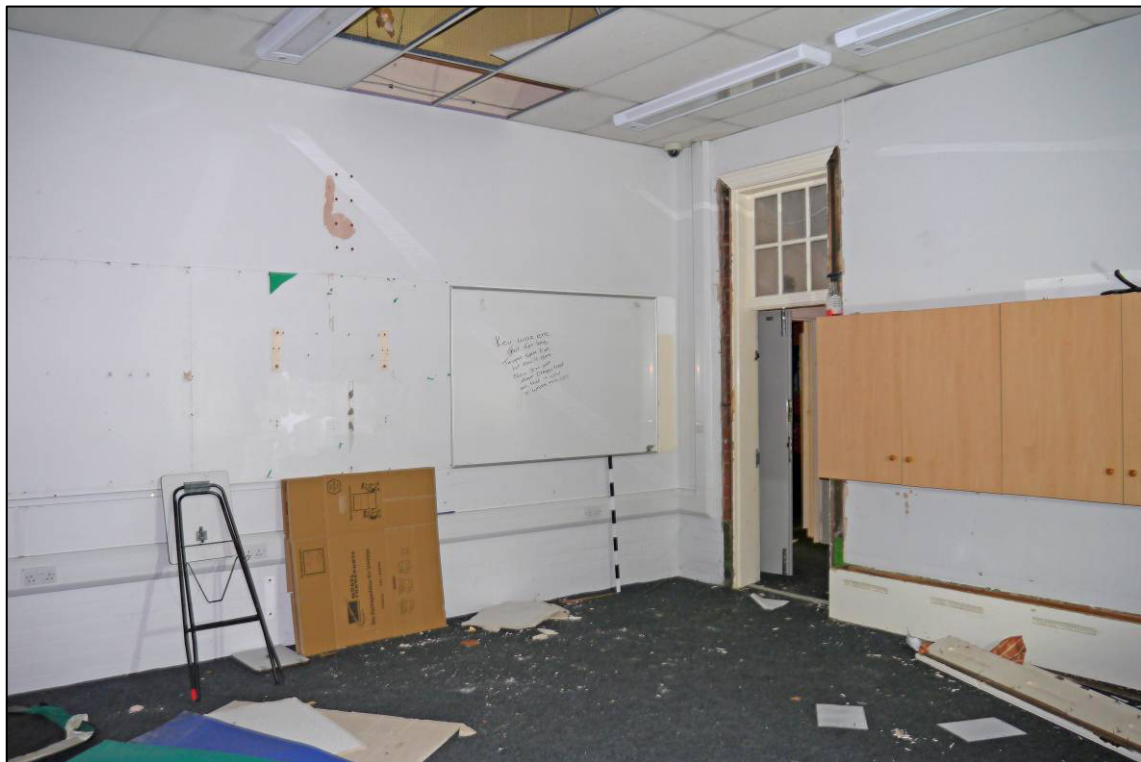
Plate 19: 1911 school building (Block 1), classroom (G/004), looking N (photo 1/017).
