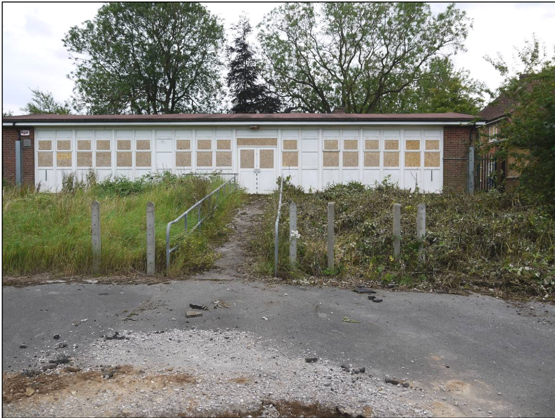
Plate 52: 1955 classroom block (Block 5), north elevation with ramped access, looking SW (photo 1/195).
