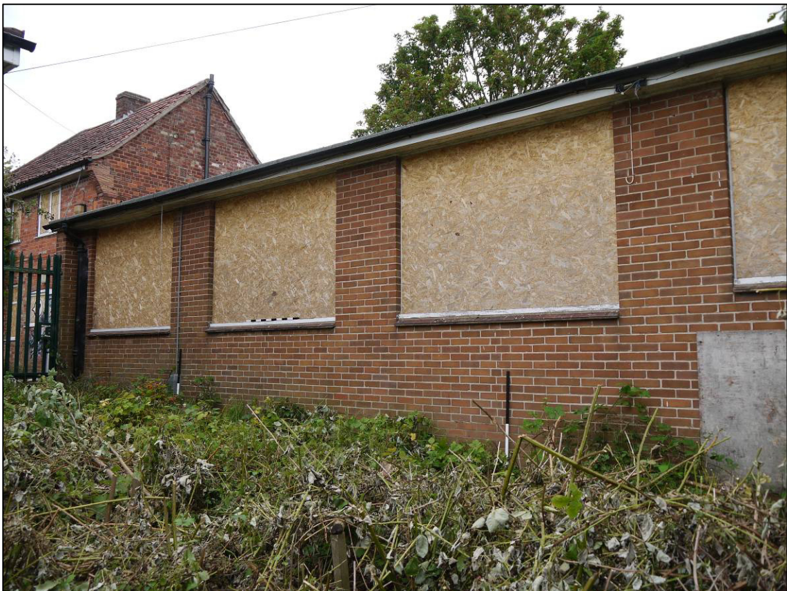
Plate 43: 1960 kitchen and dining block (Block 4), east elevation, looking SW (photo 1/179).
