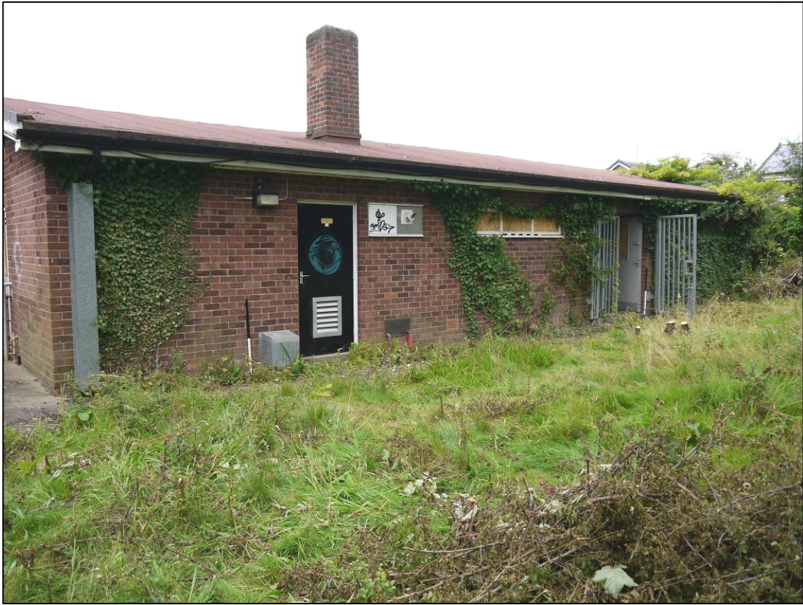
Plate 48: 1955 classroom block (Block 5), west end of south elevation, looking E (photo 1/188).
