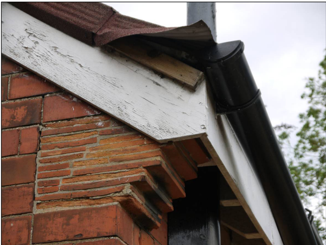
Plate 6: 1911 school building (Block 1), detail of tiled kneeler on south elevation, looking NW (photo 1/147).
