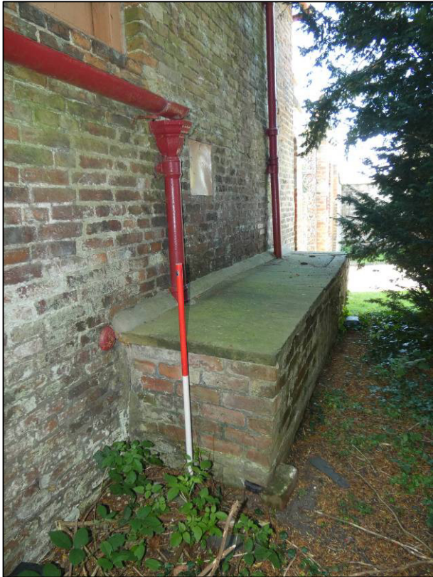
Plate 10: North external elevation, water tank at west end, looking SW (photo 1/622).
