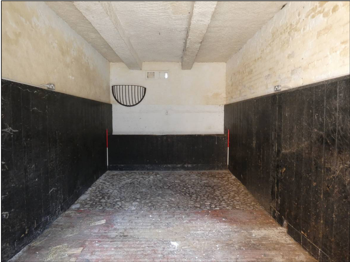
Plate 32: East range, ground floor loose box (GF2), looking NE (photo 1/696).
