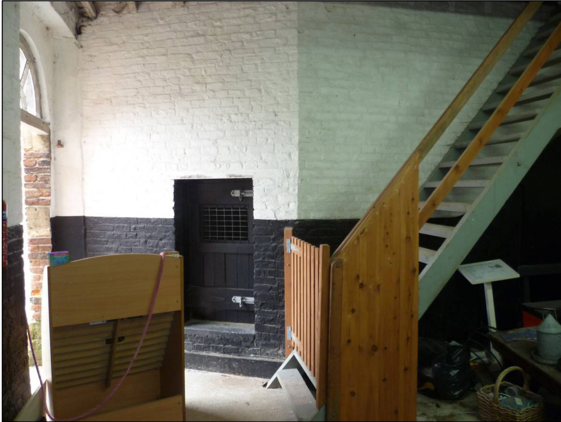
Plate 27: North range, east end, ground floor room (GF1), door in angled west wall, looking W (photo 5/903).
