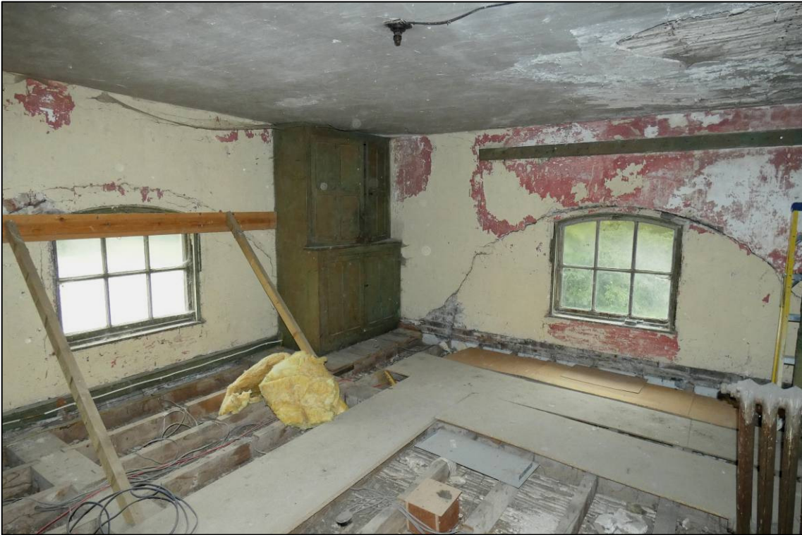
Plate 72: South range, first floor room (1F5), looking SE (photo 3/559).
