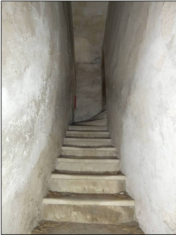
Plate 77: South range, western stairs to first floor rooms, looking NW (photo 1/796).
