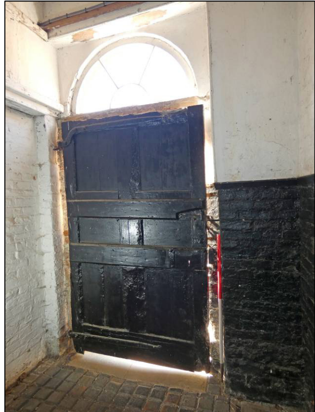
Plate 38: East range, ground floor passage (GF4), looking SW (photo 1/727).
