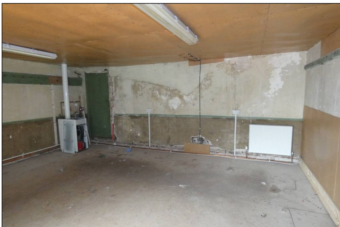
Plate 67: South range, first floor room (1F6), north wall, looking NW (photo 3/573).
