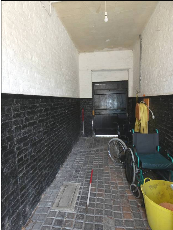
Plate 37: East range, ground floor passage (GF4), looking NE (photo 1/722).
