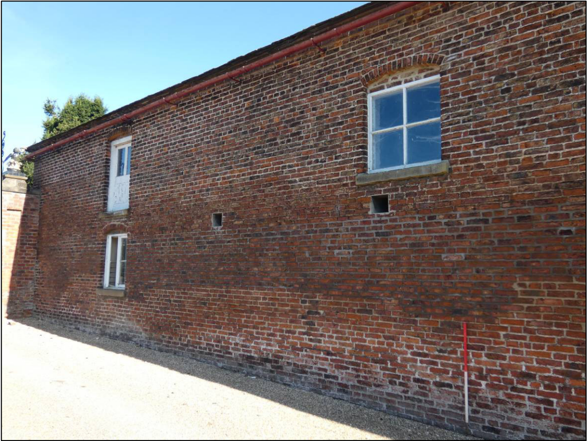
Plate 19: West external elevation, north end, looking N (photo 1/616).
