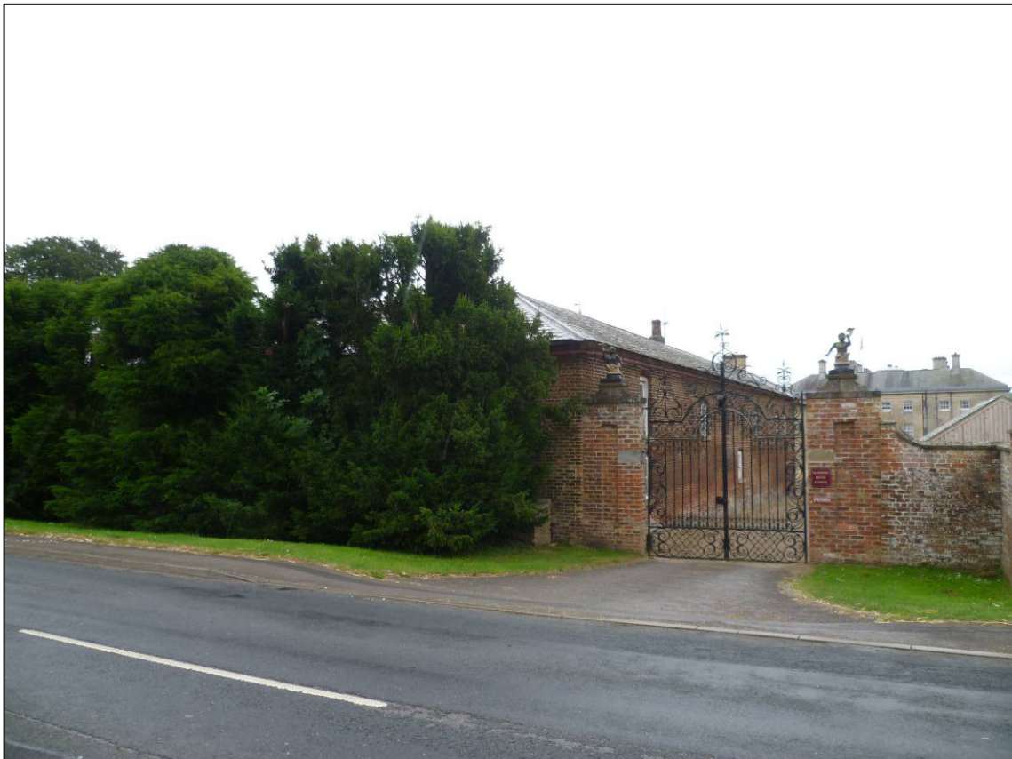
Plate 9: North external elevation and entrance gates, looking SE (photo 5/914).
