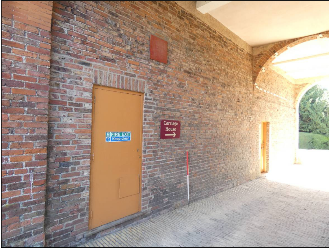
Plate 53: South range, ground floor passage (GF10), east wall, looking E (photo 1/628).
