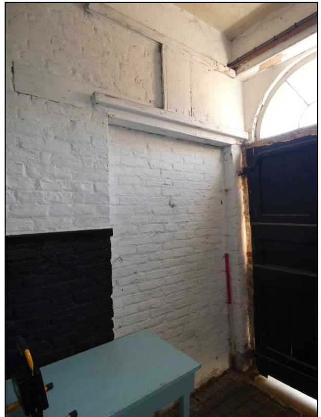
Plate 40: East range, ground floor passage (GF4), blocked opening to south wall, looking S (photo 1/729).
