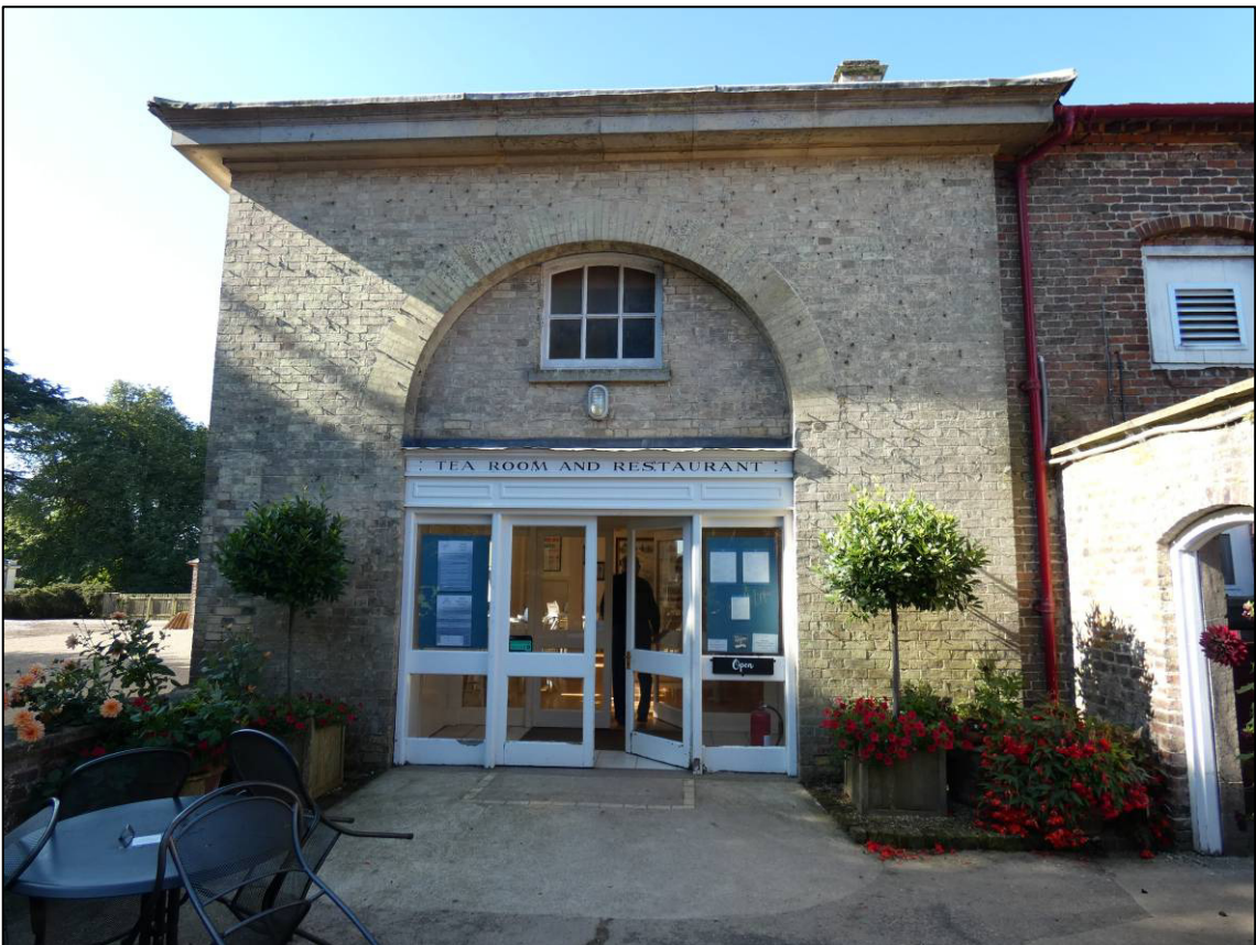
Plate 16: East external elevation, south end, 1818 facade, looking SW (photo 1/598).
