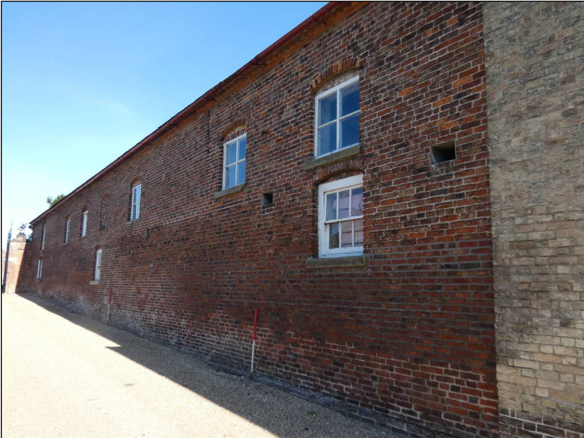
Plate 18: West external elevation, looking N (photo 1/609).
