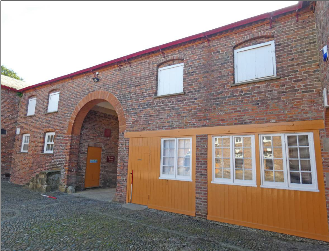
Plate 23: South courtyard elevation, looking E (photo 1/645).
