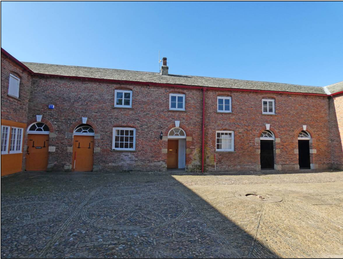
Plate 25: West courtyard elevation, looking W (photo 1/647).
