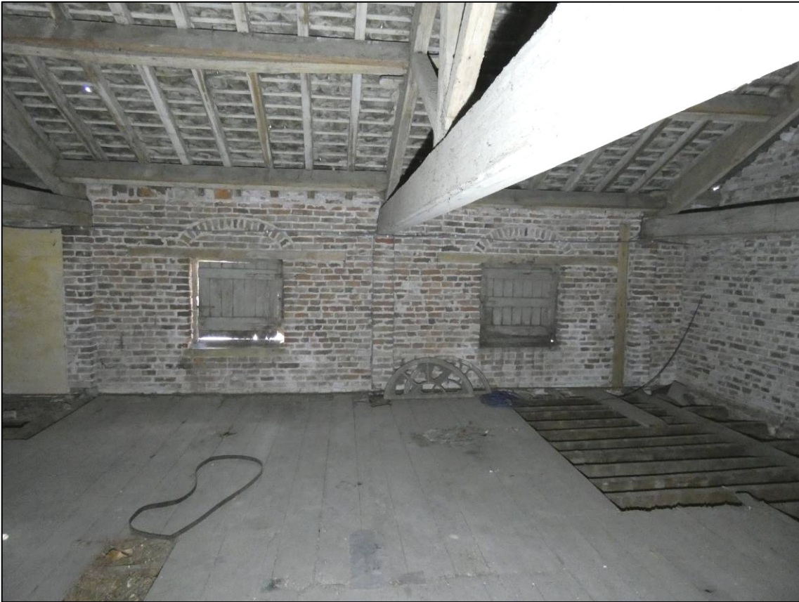
Plate 60: East range, first floor room (1F3), west wall, looking SW (photo 1/790).
