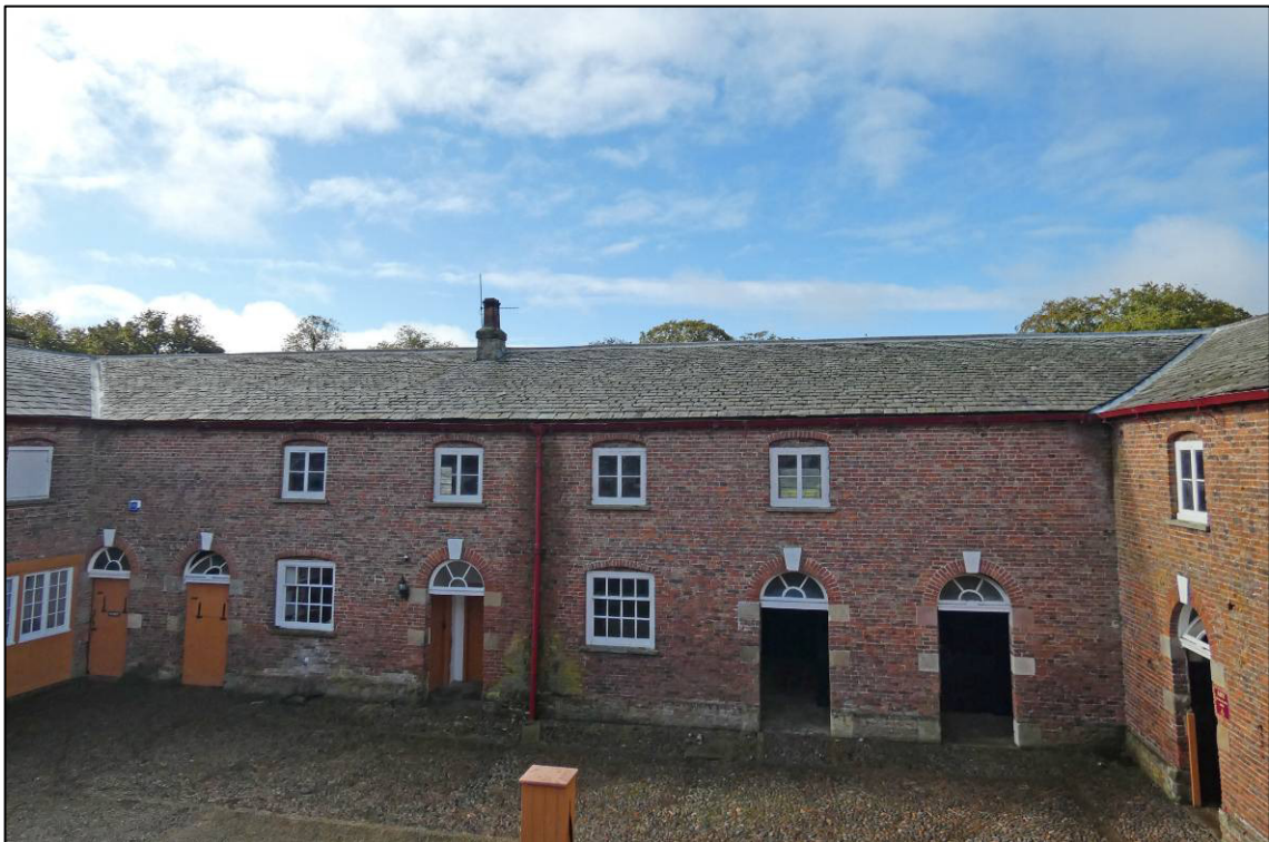
Plate 2: West courtyard elevation and roof, looking SW (photo 2/158).
