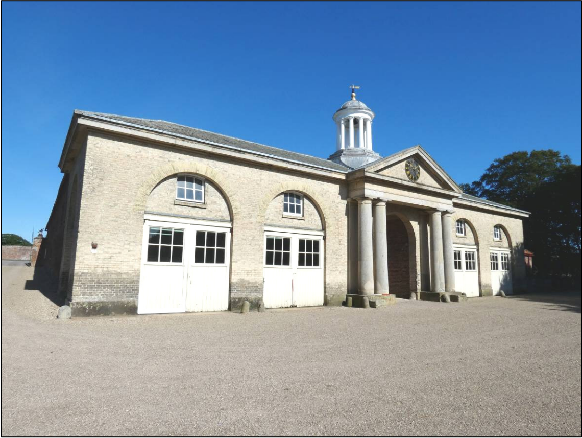
Plate 15: South external elevation, 1818 facade, looking N (photo 1/606).
