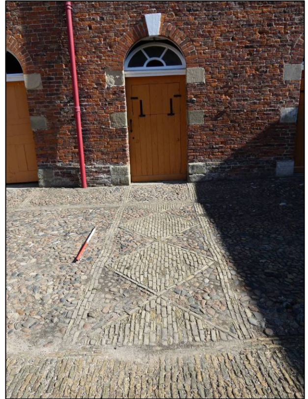
Plate 8: Courtyard mosaic, detail of east side design to doorway, looking NE (photo 1/661).
