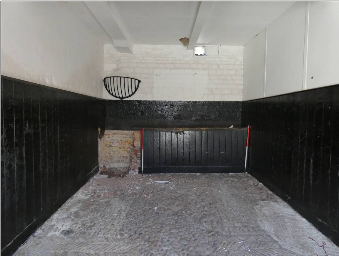
Plate 42: East range, ground floor loose box (GF5), looking NE (photo 1/734).
