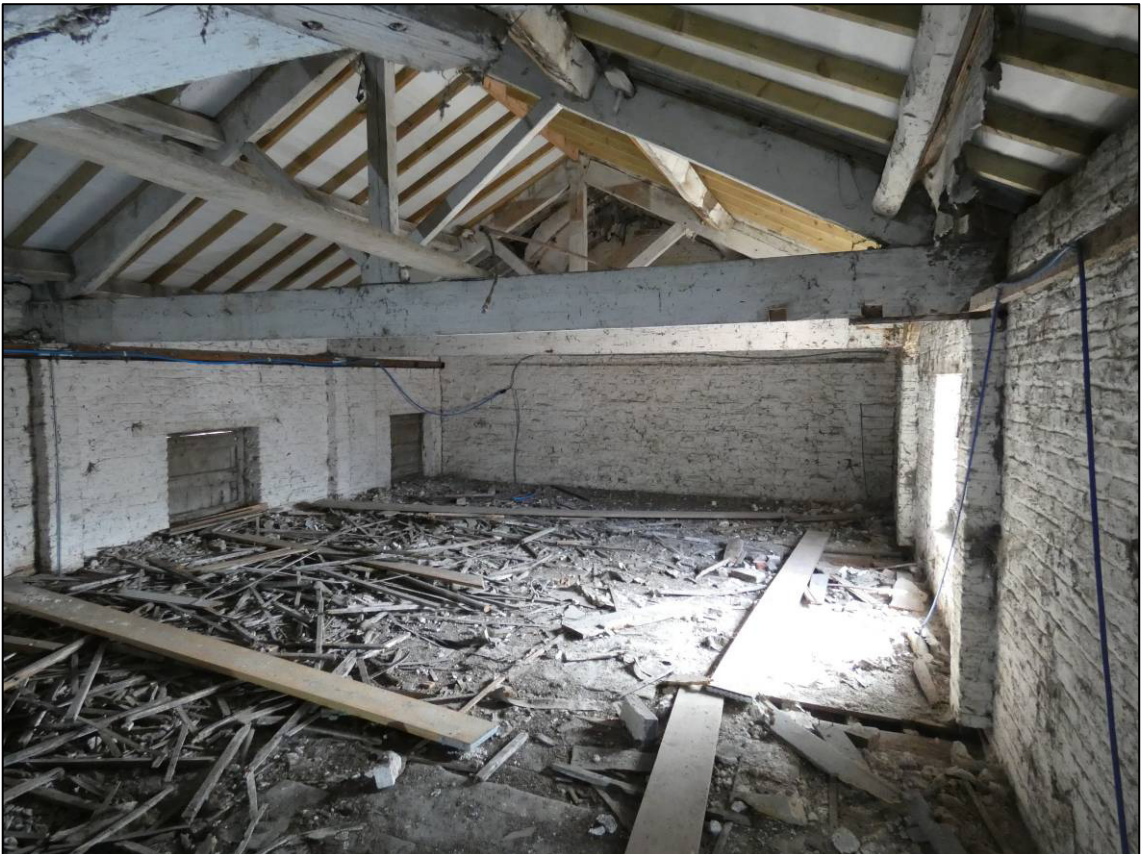
Plate 59: East range, first floor room (1F2), looking SE (photo 1/844).
