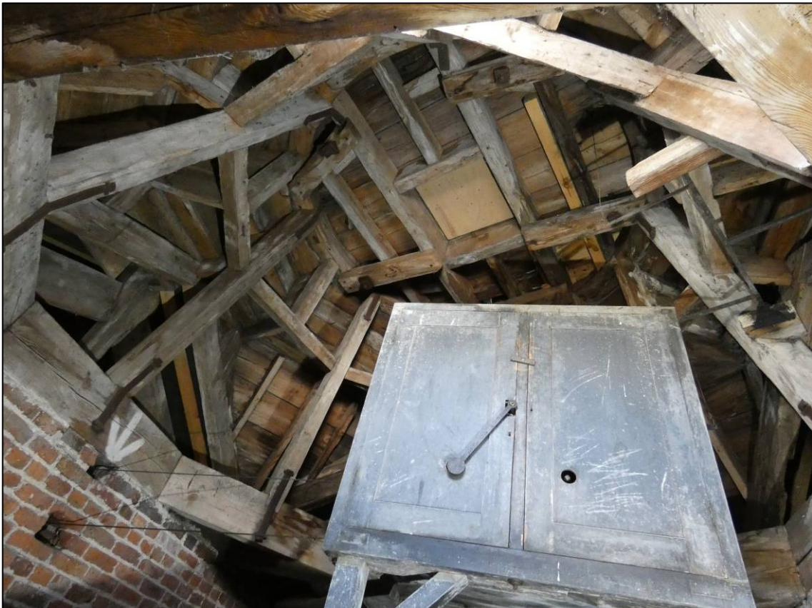
Plate 83: South range, first floor room (1F8), frame for cupola and case for clock mechanism, looking SE (photo 1/824).
