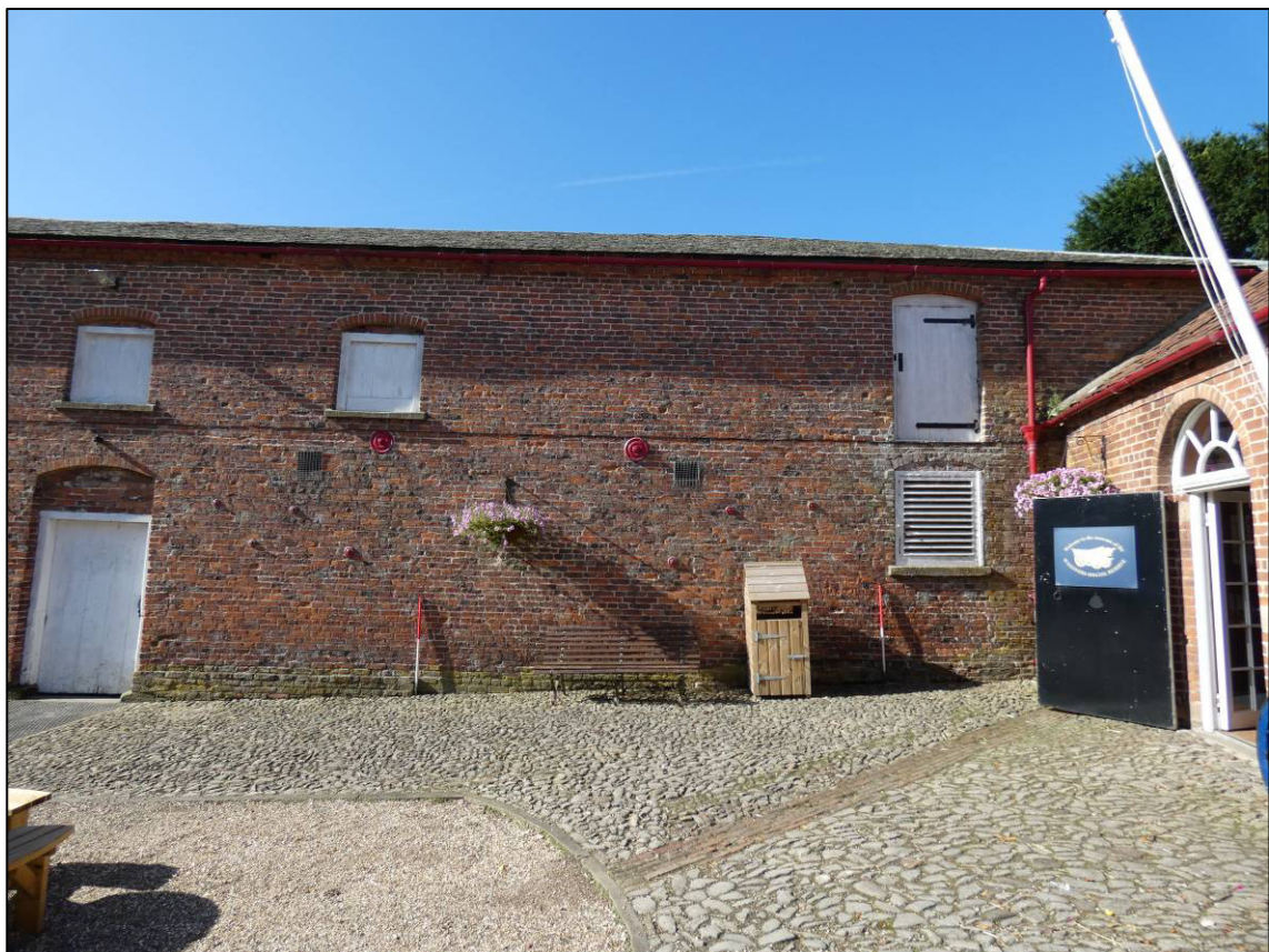
Plate 12: East external elevation, north end, looking SW (photo 1/590).
