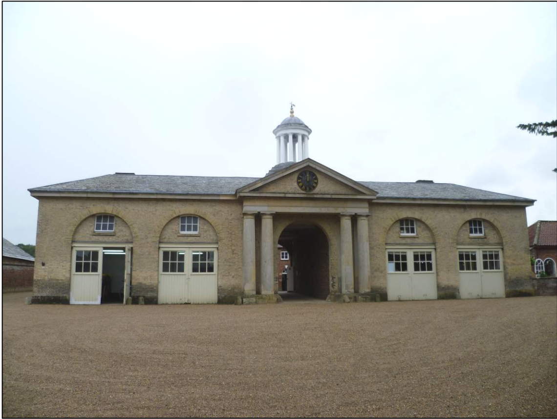
Plate 1: South external elevation, 1818 facade, looking NW (photo 5/917).
