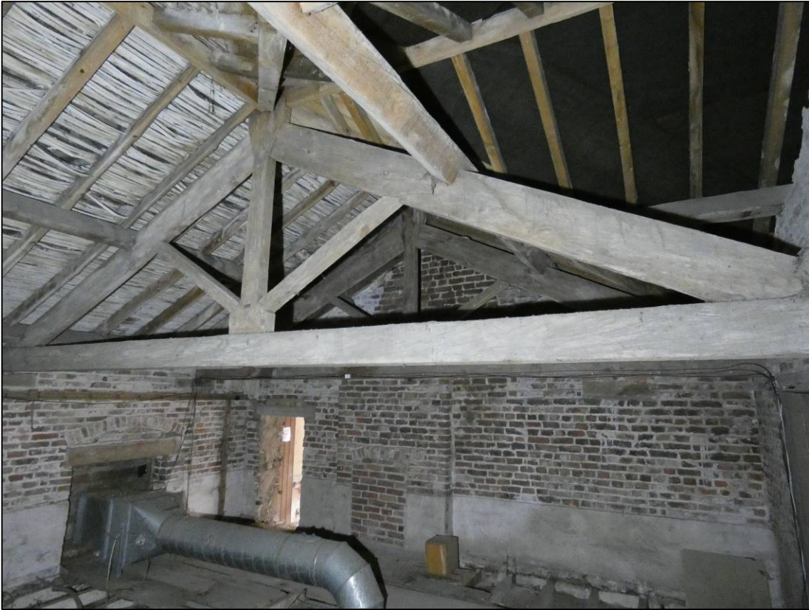
Plate 75: South range, first floor room (1F4), truss, looking SE (photo 1/784).
