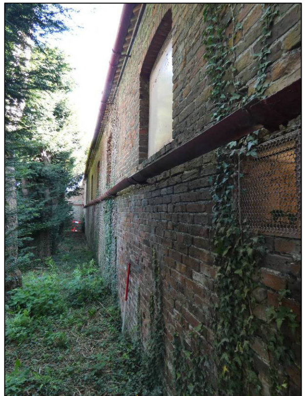
Plate 11: North external elevation, looking NE (photo 1/623).
