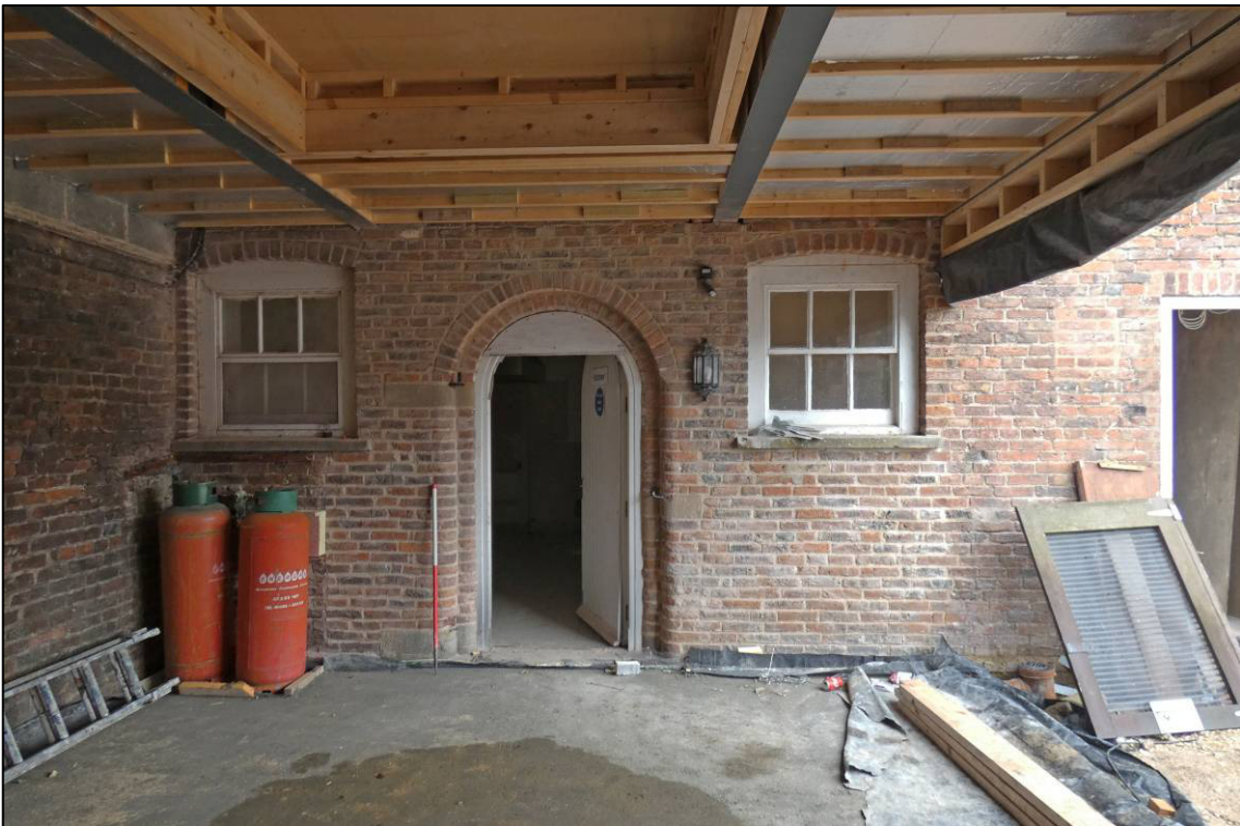
Plate 14: East external elevation, S end, during alterations, looking SW (photo 3/598).
