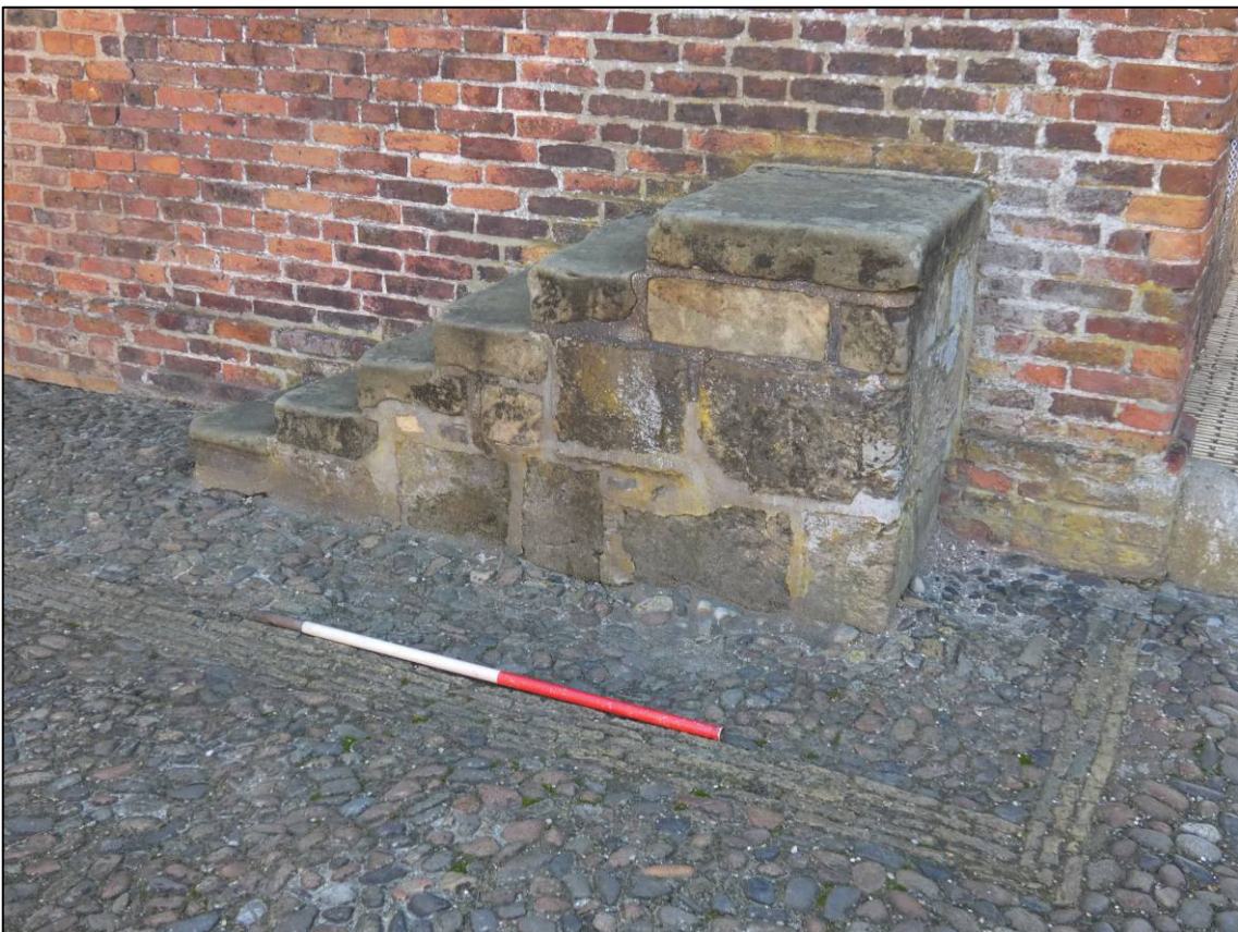
Plate 24: South courtyard elevation, mounting steps, looking E (photo 1/646).
