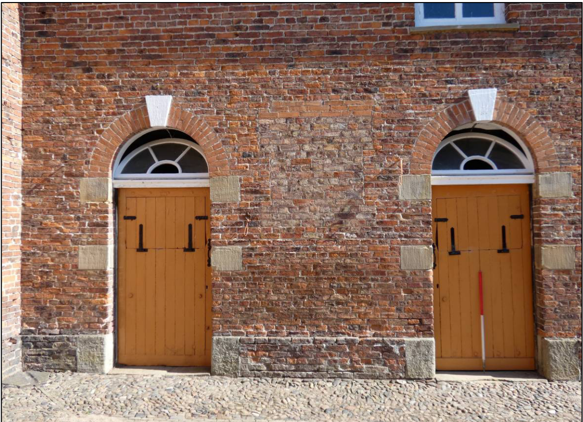
Plate 22: East courtyard elevation, north end, looking NE (photo 1/658).
