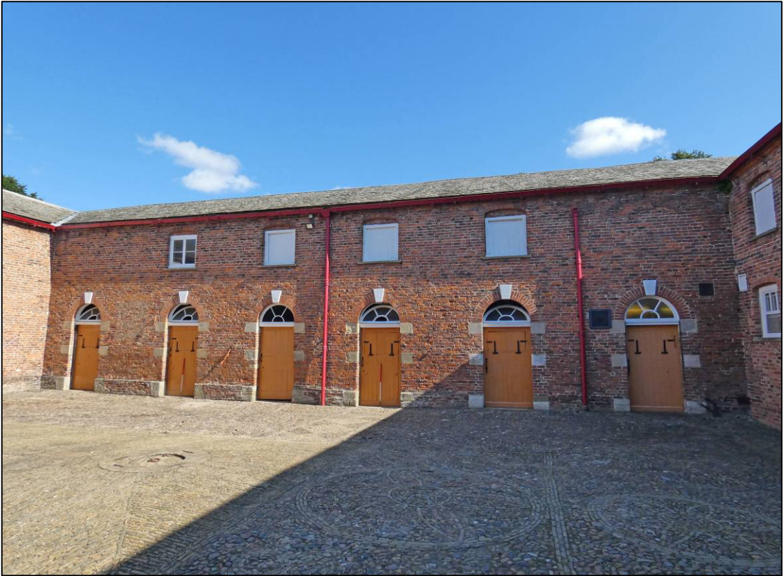
Plate 21: East courtyard elevation, looking NE (photo 1/654).
