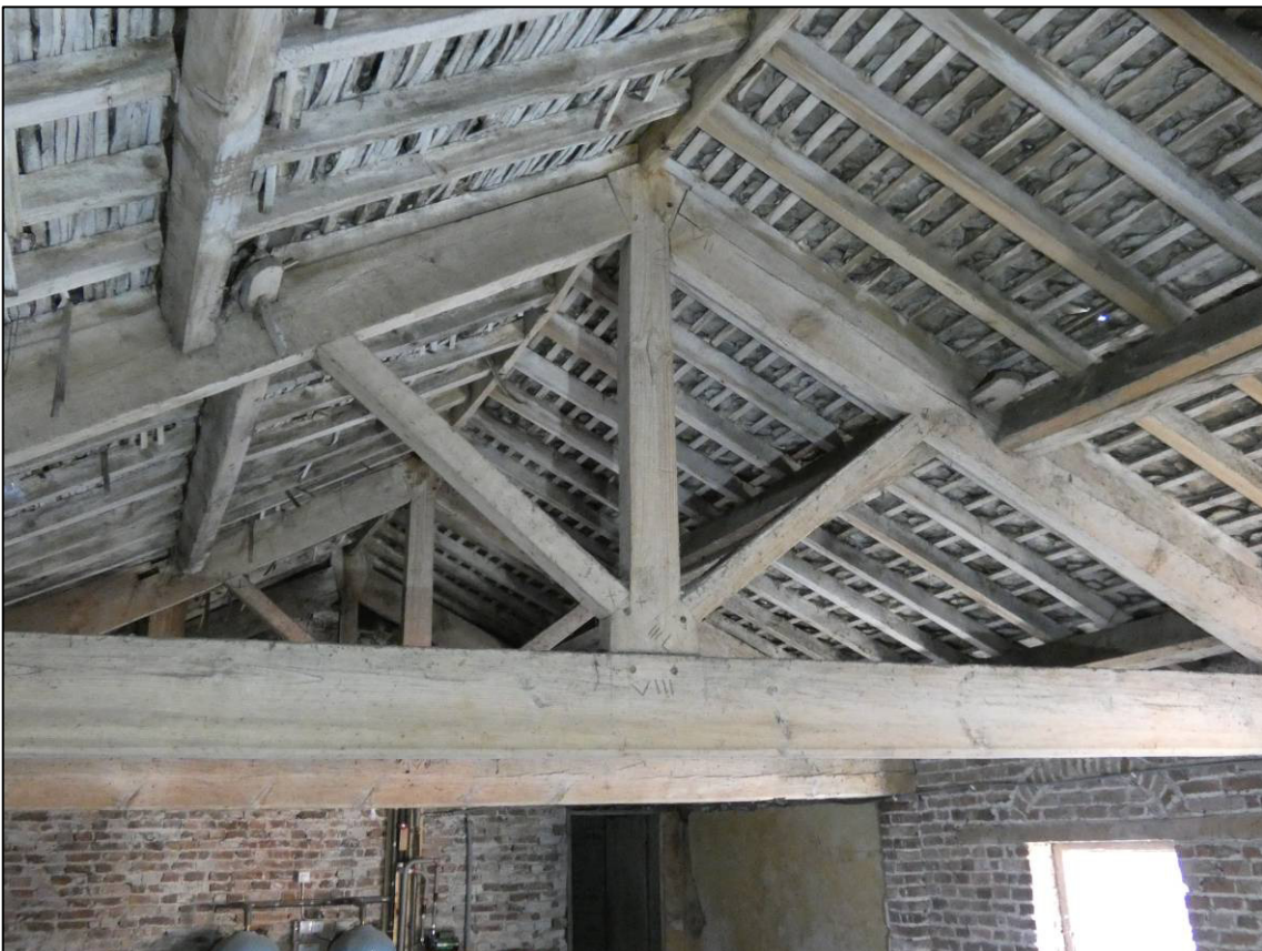
Plate 61: East range, first floor room (1F3), truss, looking SE (photo 2/152).
