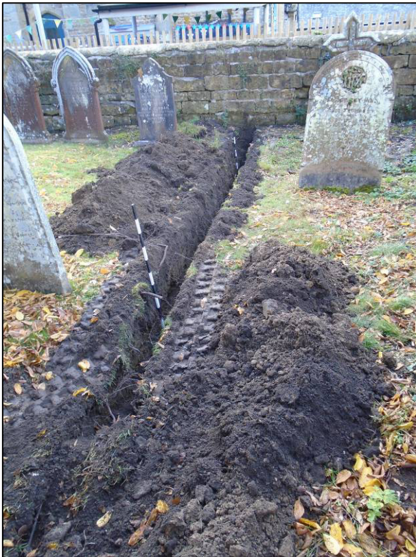
Plate 5: Excavation of foul water pipe trench, looking W.
