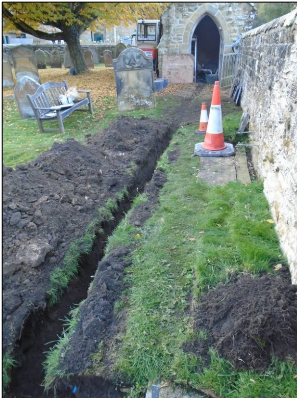
Plate 2: Excavation of fresh water pipe trench, looking W towards Hearst House
