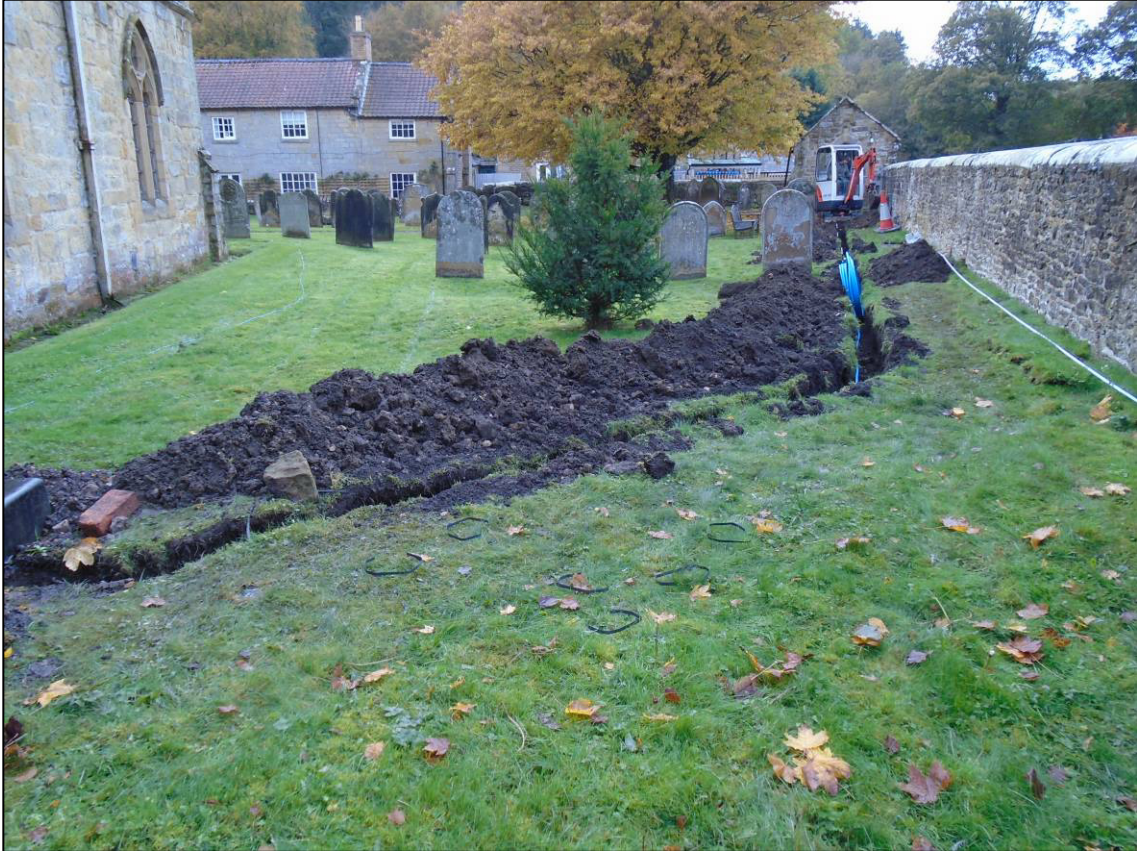
Plate 1: Excavation of fresh water pipe trench, looking W.
