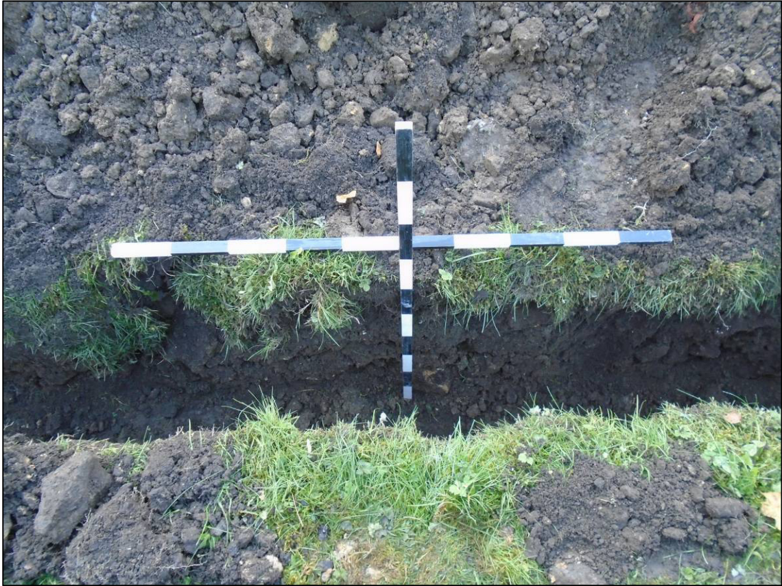
Plate 4: Typical section of fresh water pipe trench, looking SW.
