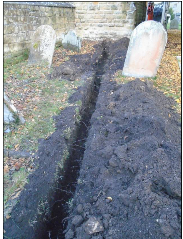
Plate 6: Excavation of foul water pipe trench, looking E towards Hearst House.
