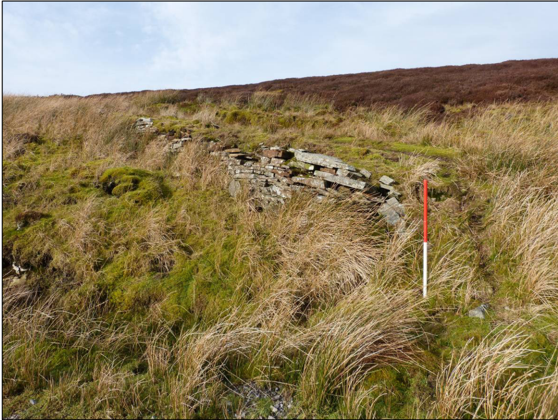
Plate 1: Causeway to Lad Gill (Site 2/1), revetment wall to south side, looking W (photo 1/024).
