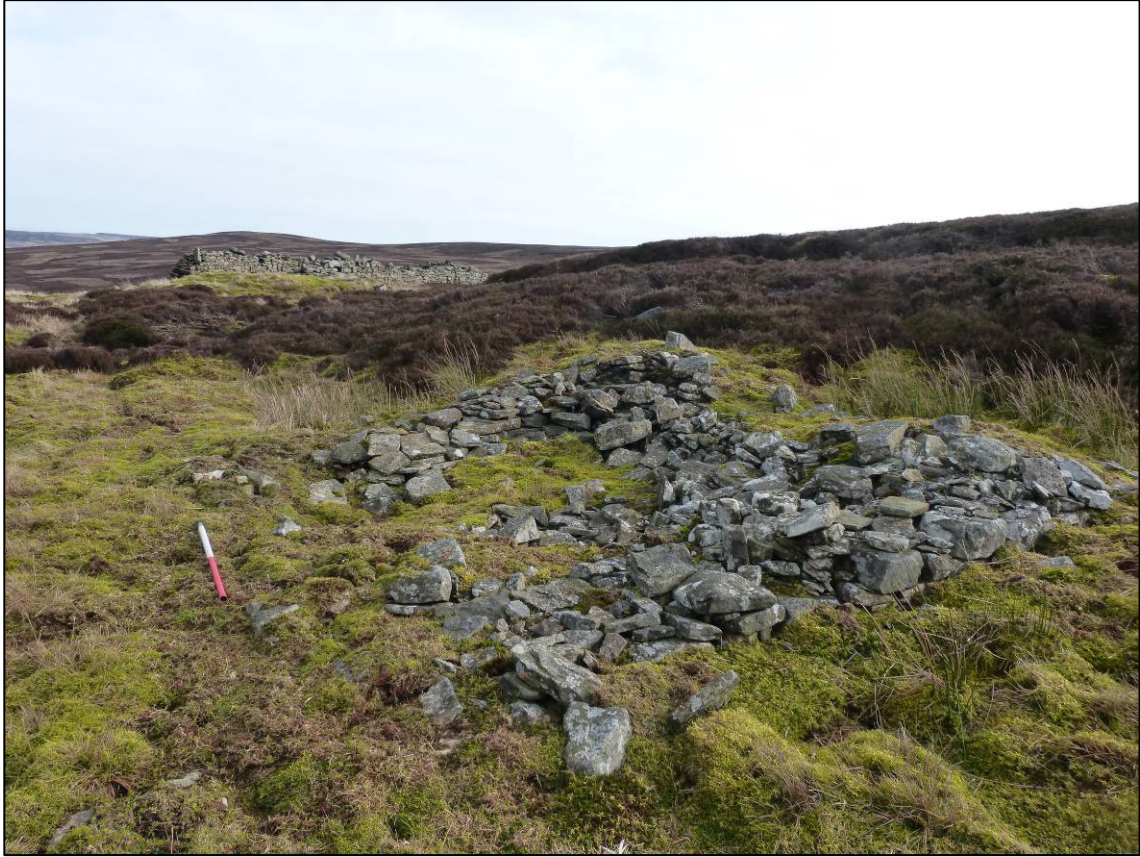
Plate 5: Structure in Lad Gill complex (Site 2/3), looking E (photo 1/037).
