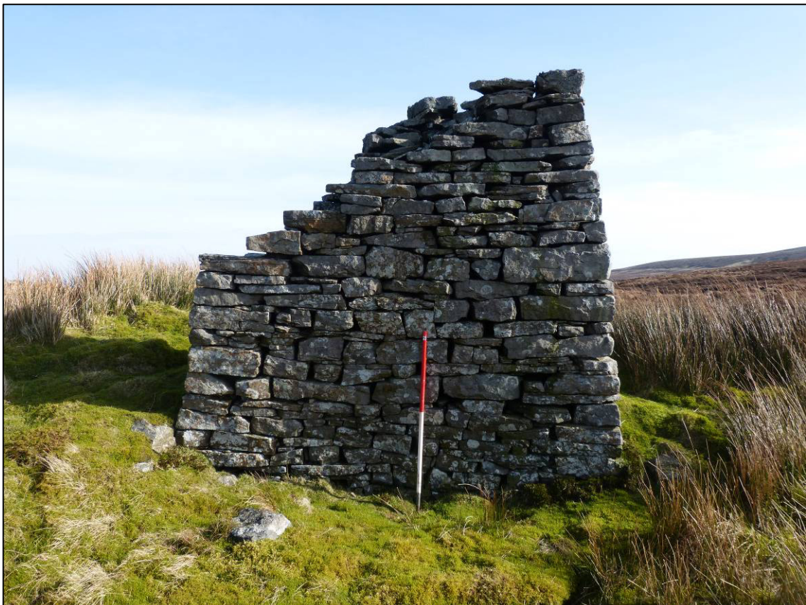
Plate 24: William Gill colliery (Site 14), east pier of whim circle, looking E (photo 2/148).
