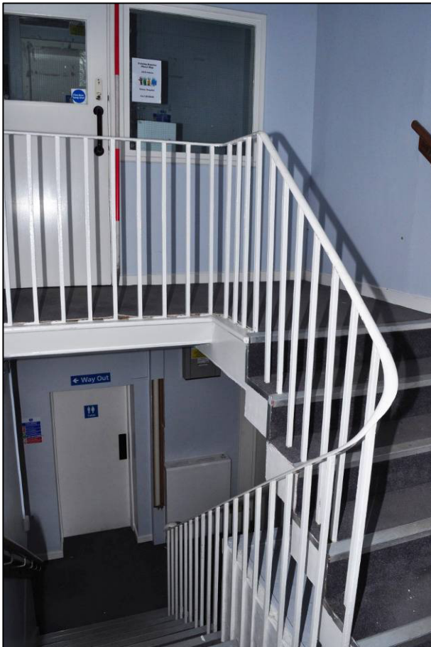
Plate 95: West range, later part, room 1F1 (landing), looking E (photo 1/2996).
