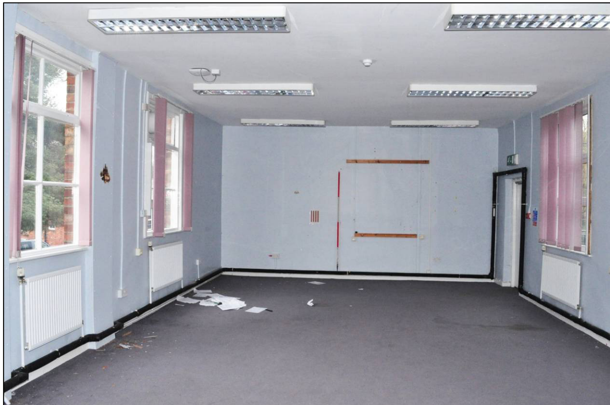
Plate 98: West range, later part, room 1F4, looking S (photo 1/3003).
