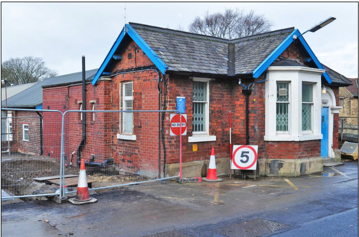
Plate 8: Porter's Lodge, west and south elevations, looking NE (photo 1/2931).
