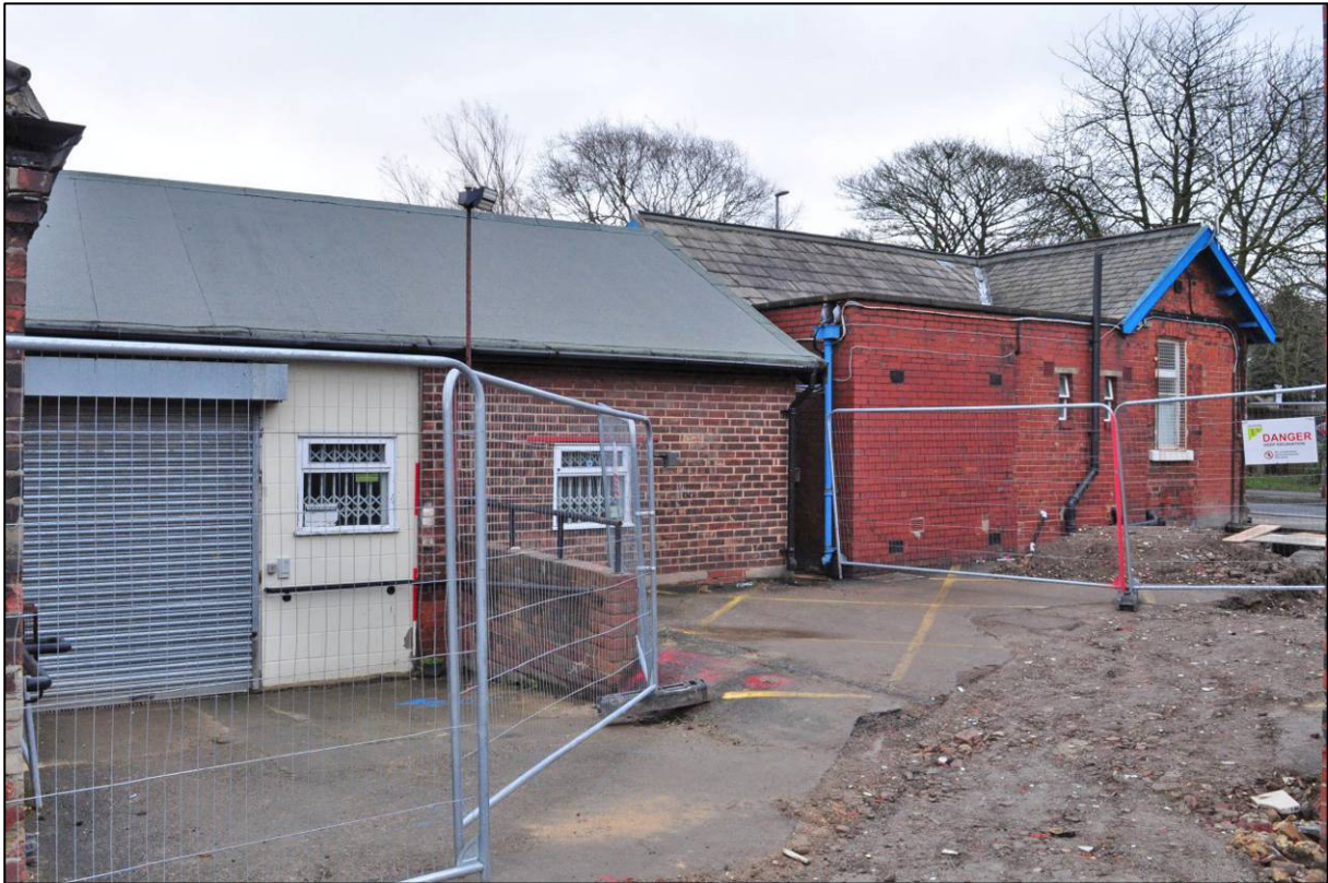
Plate 59: East range, southern extension, west elevation, with Porter's Lodge, looking SE (photo 1/2981).
