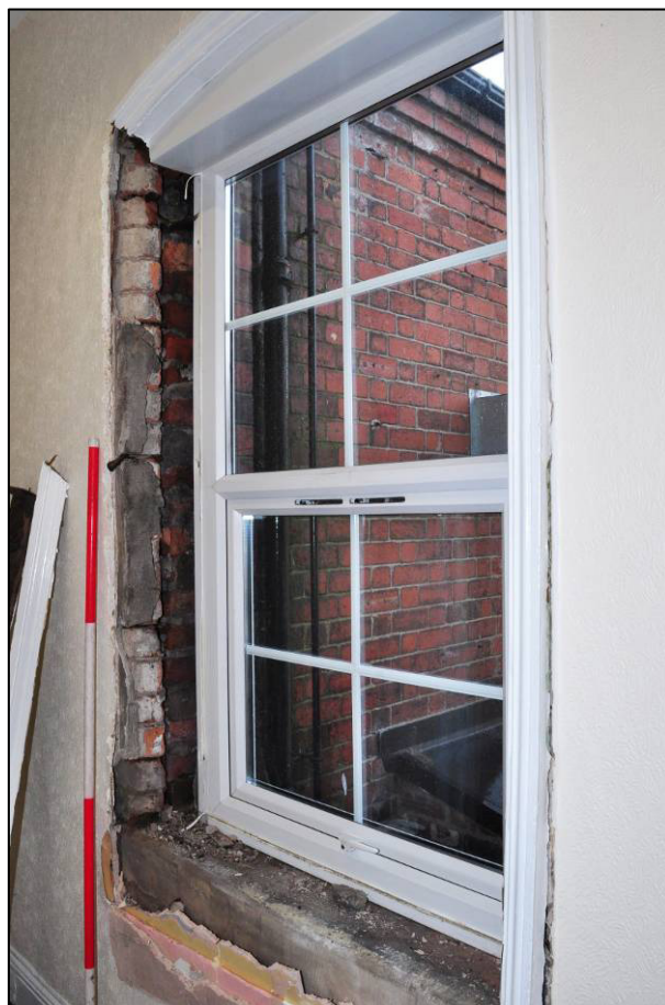
Plate 37: Entrance Block, main corridor G4, window detail, looking NW (photo 1/2854).
