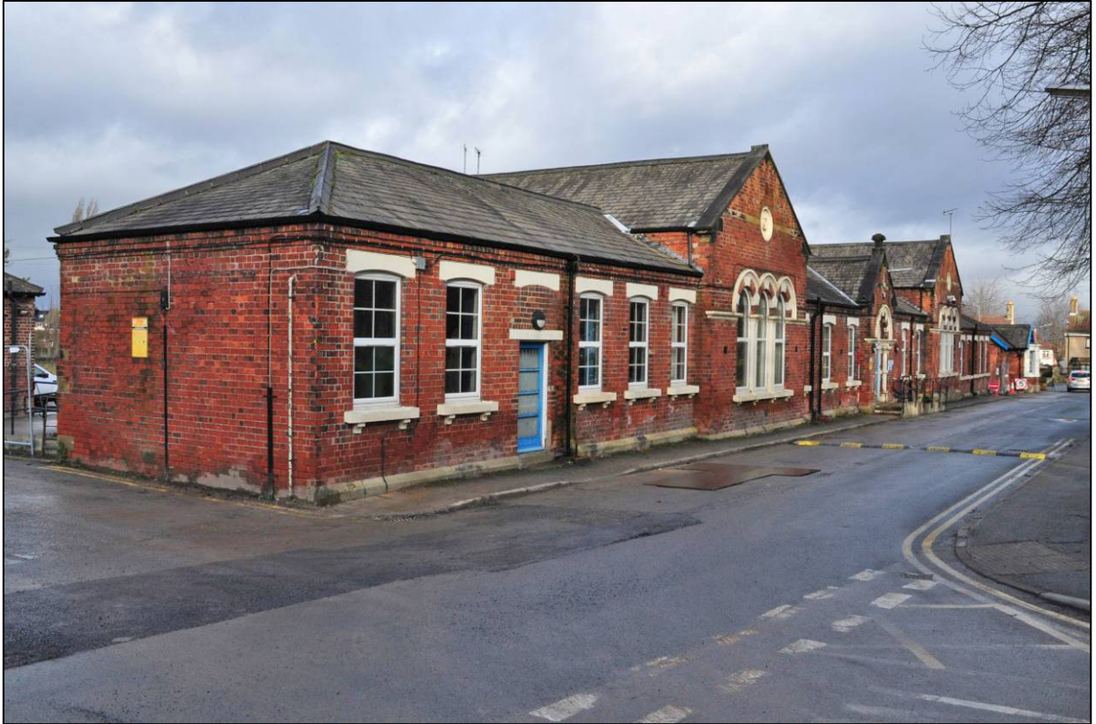
Plate 20: Entrance Block, south elevation, looking NE (photo 1/2948).
