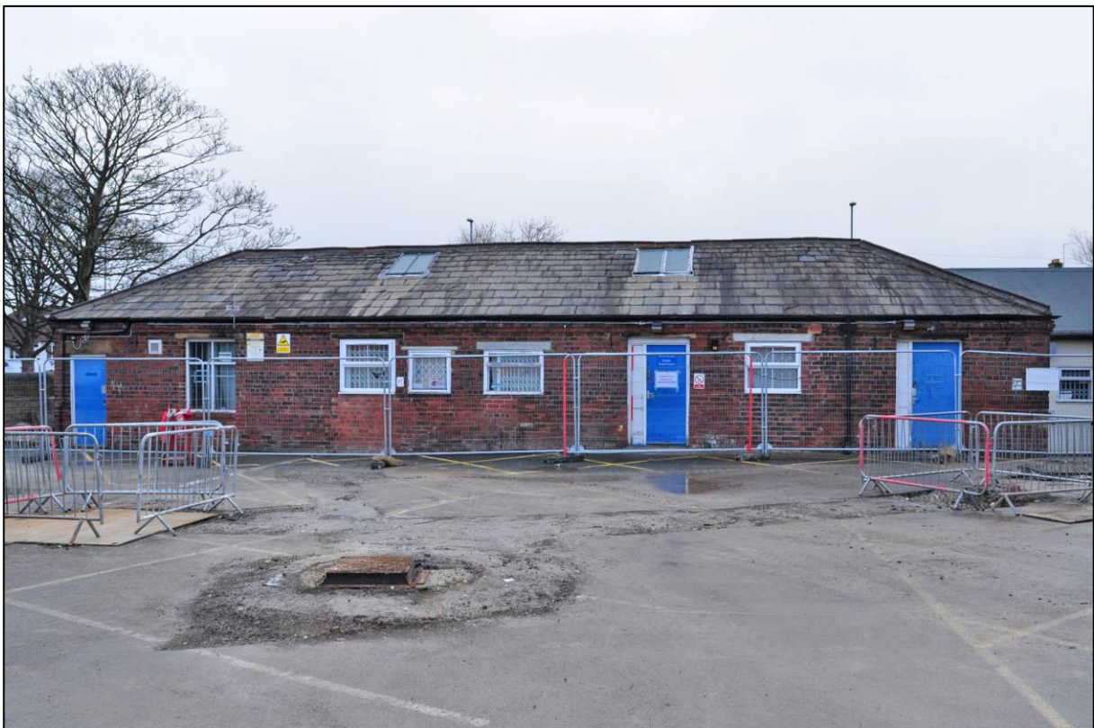
Plate 56: East range, original part, west elevation, looking E (photo 1/2979).
