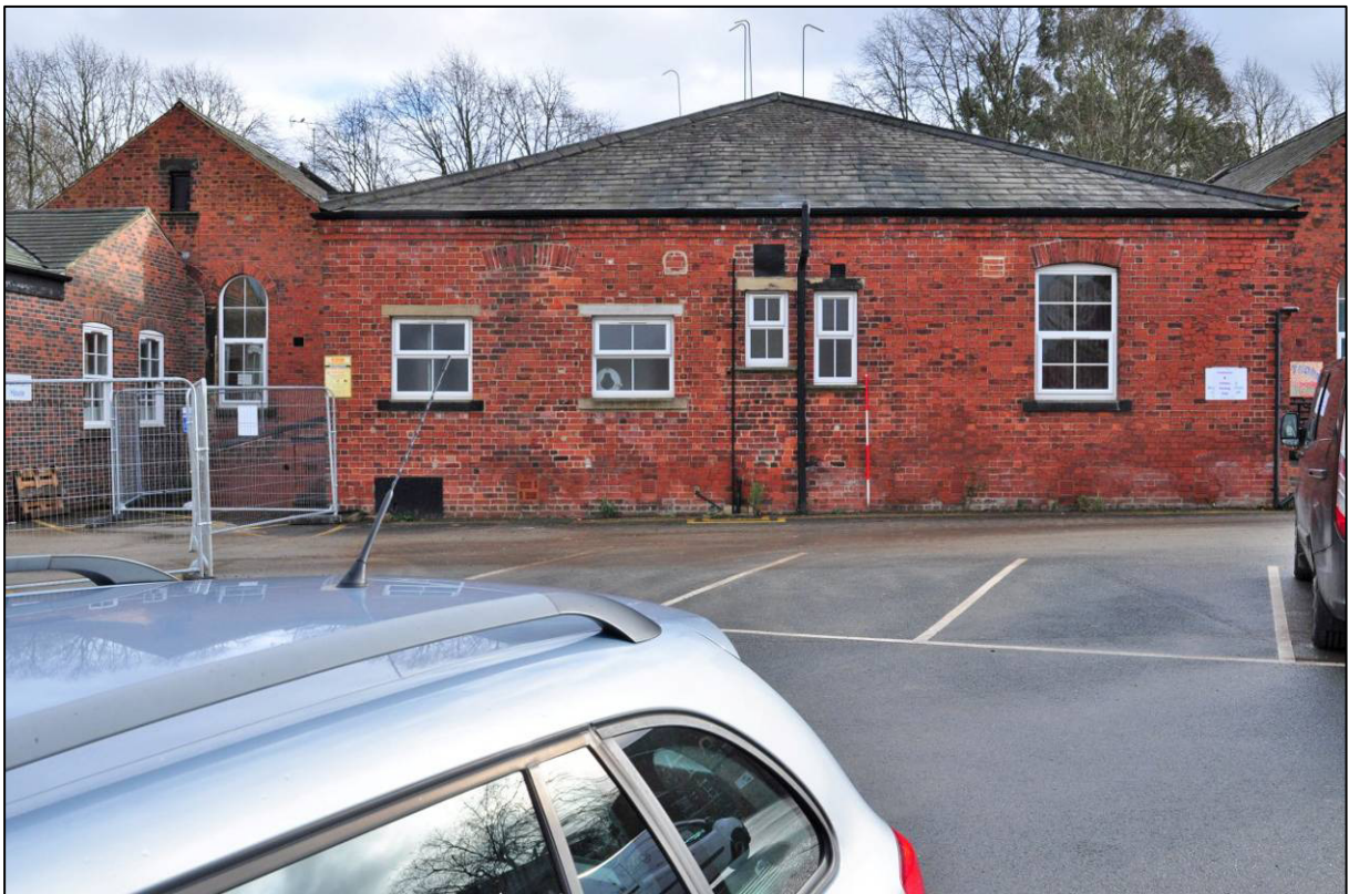
Plate 29: Entrance Block, north elevation, central projection, looking S (photo 1/2964).
