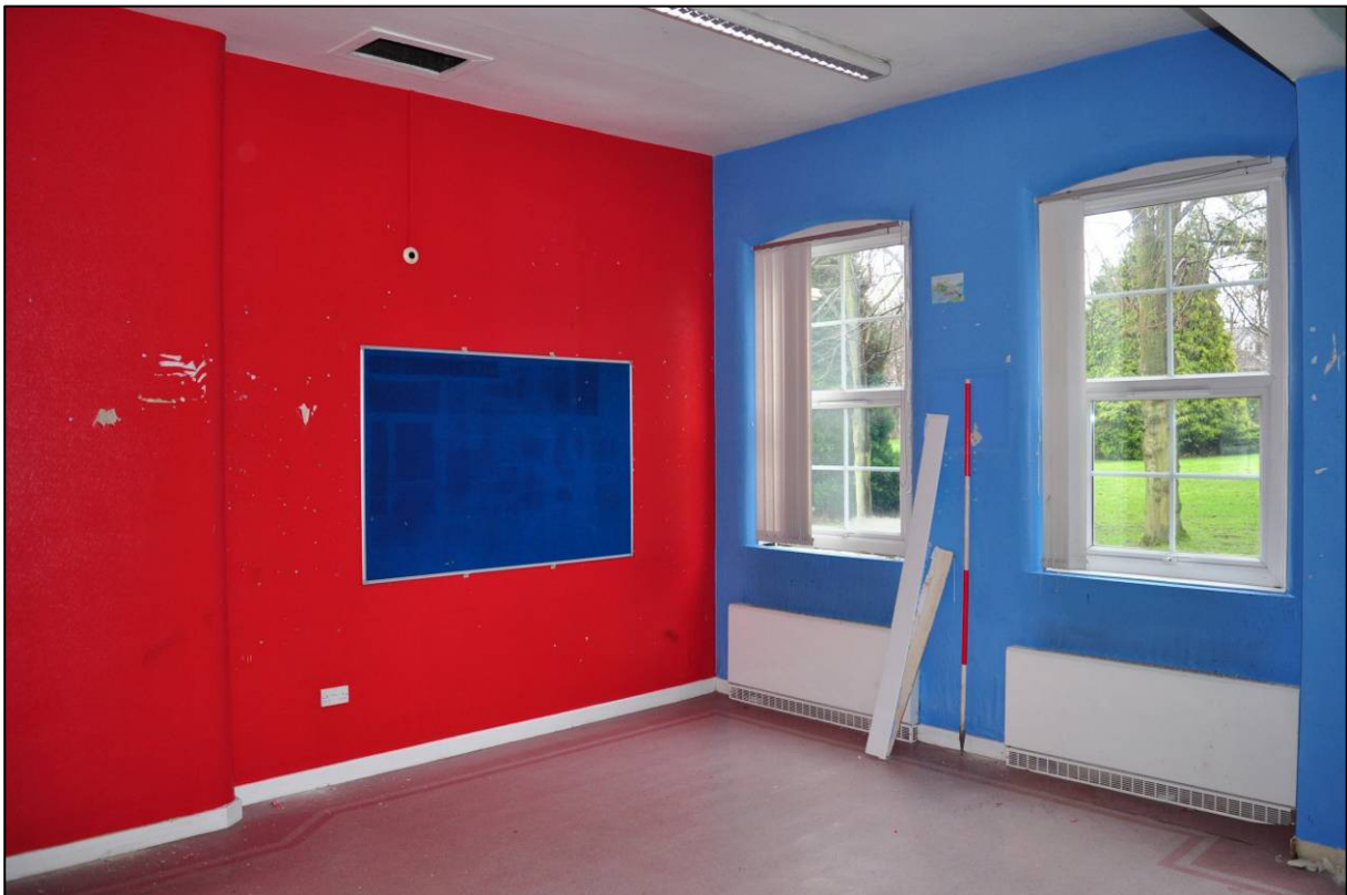
Plate 54: Entrance Block, room G15 (former Male Probationers' Ward), looking SE (photo 1/2865).
