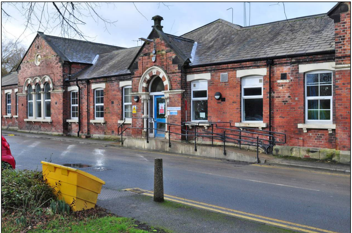
Plate 14: Entrance Block, central part of south elevation, looking NW (photo 1/2947).
