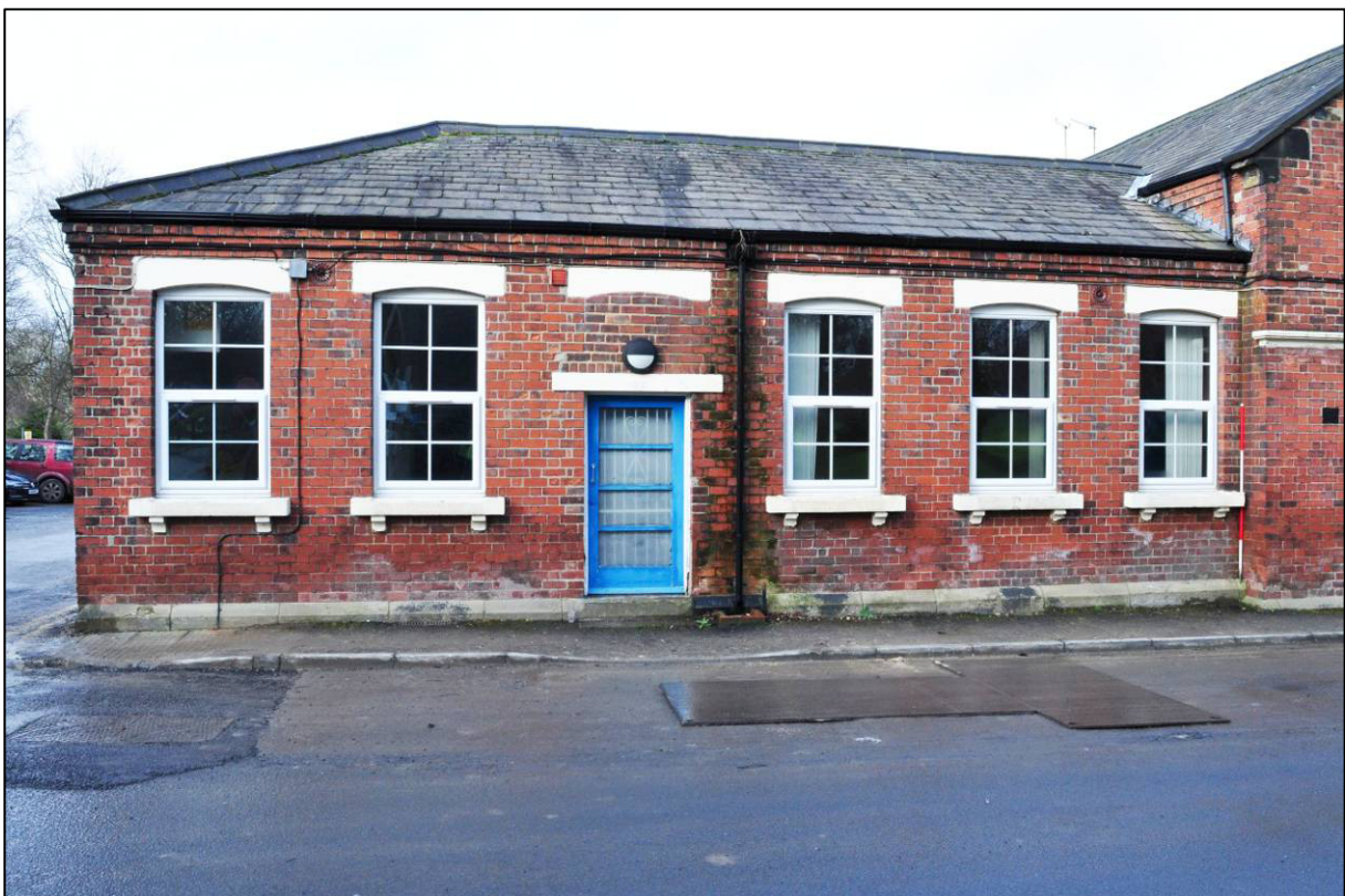
Plate 23: Entrance Block, west end of south elevation, looking N (photo 1/2954).
