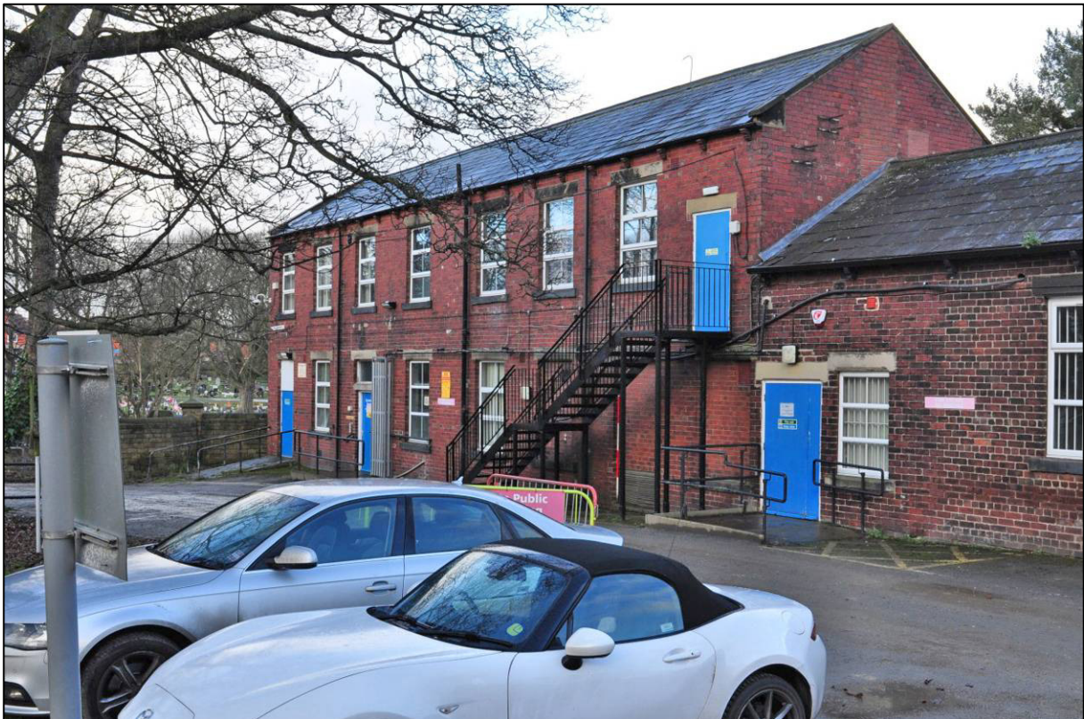
Plate 82: West range, later part, west elevation, looking NE (photo 1/3011).
