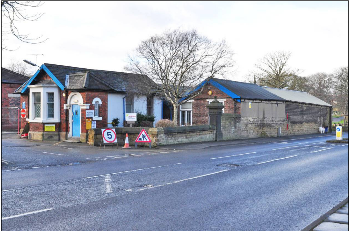
Plate 3: East range, south gable and east elevation, with Porter's Lodge, looking NW (photo 1/2921).
