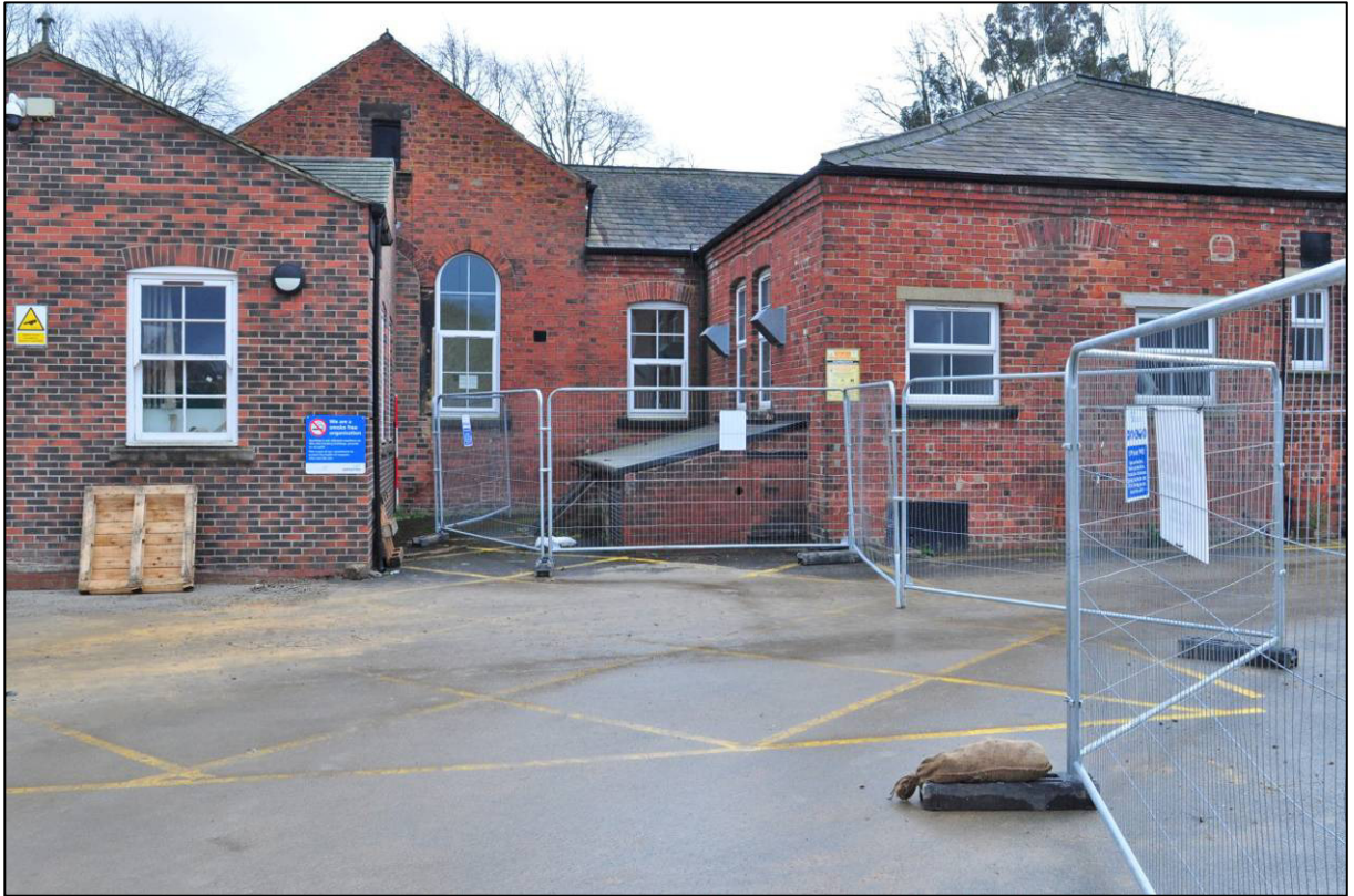
Plate 30: Entrance Block, central part of north elevation, looking S (photo 1/2966).
