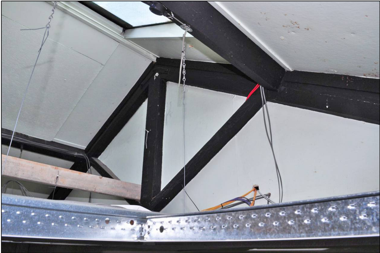
Plate 63: East range, original part, room G19, roof truss, looking SE (photo 1/2908).
