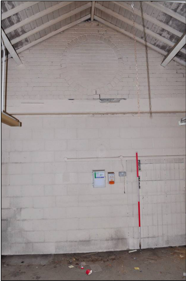
Plate 76: East range, southern extension, room G23, blocked circular vent in gable apex, looking N (photo 1/2881).
