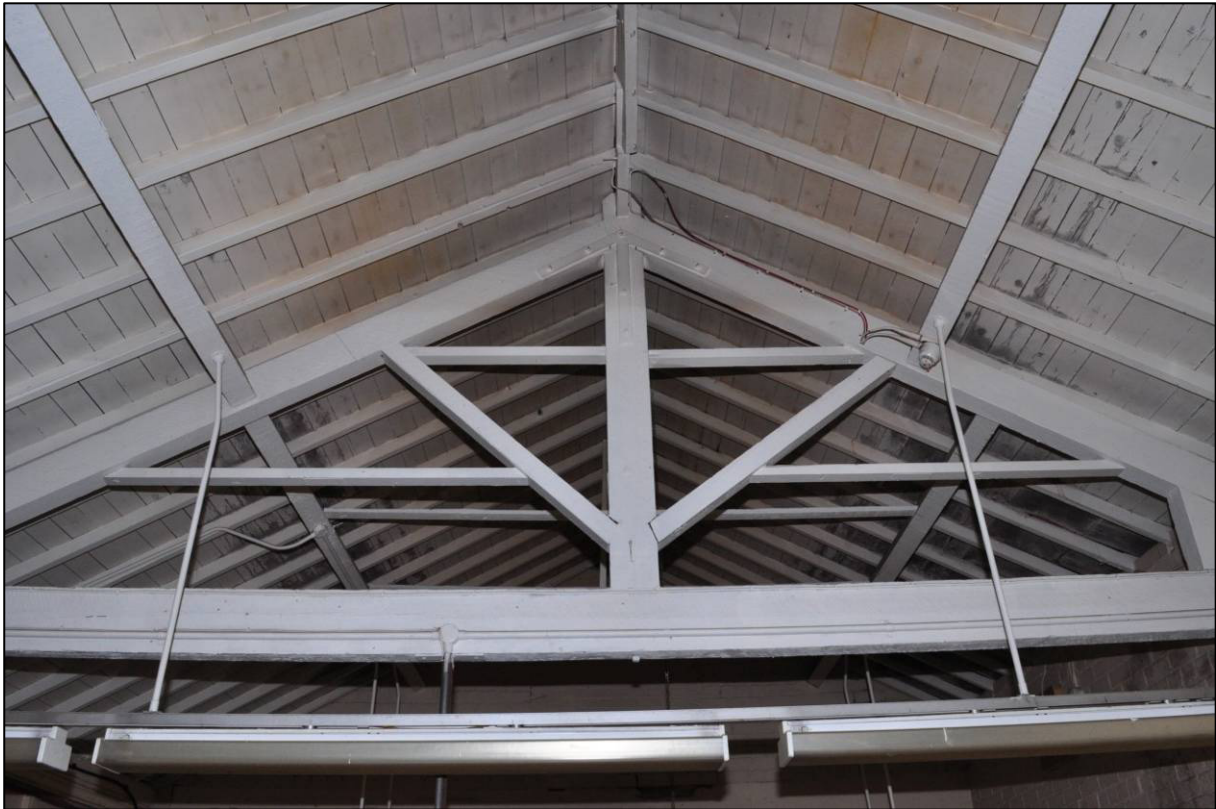
Plate 77: East range, southern extension, room G23, roof truss, looking S (photo 1/2880).
