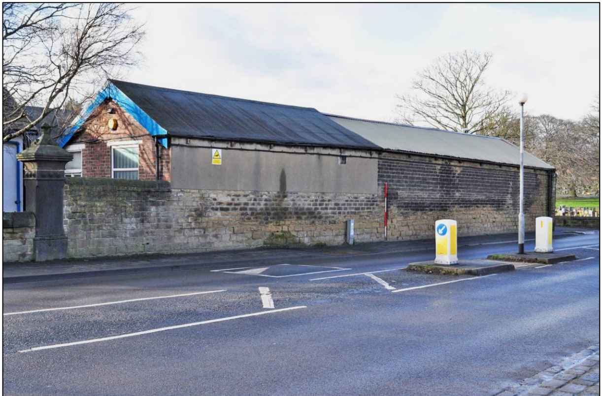
Plate 2: East range, south gable and east elevation, showing earlier boundary wall, looking NW (photo 1/2918).
