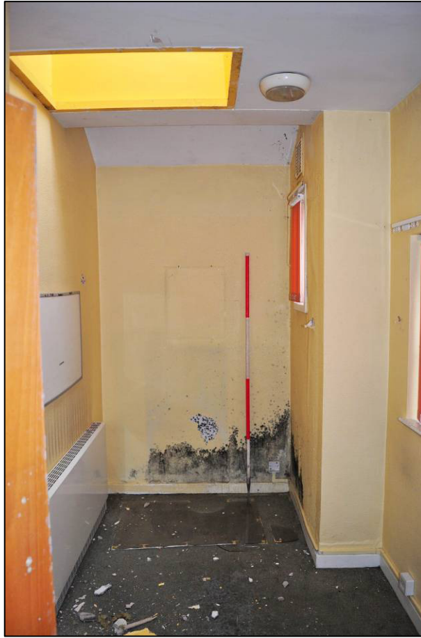
Plate 53: Entrance Block, room G17, looking N (photo 1/2866).
