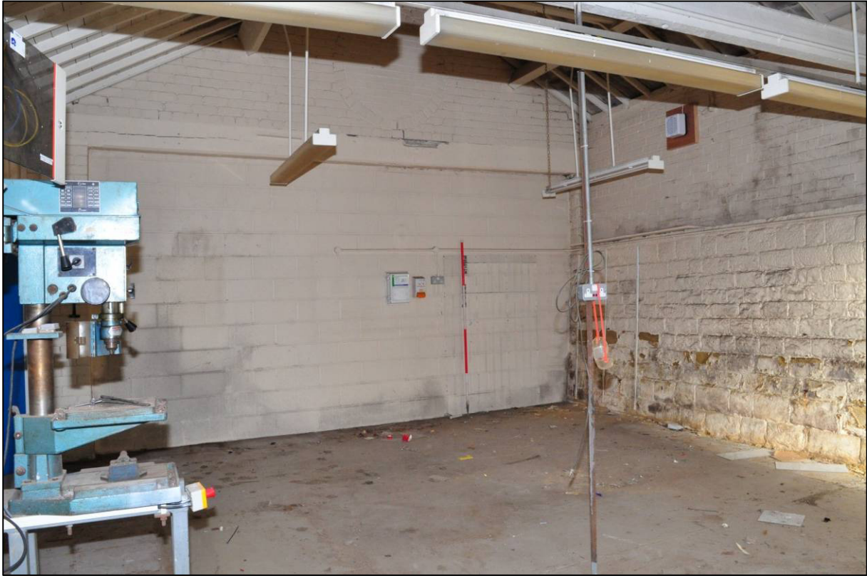
Plate 75: East range, southern extension, room G23, looking NE (photo 1/2879).
