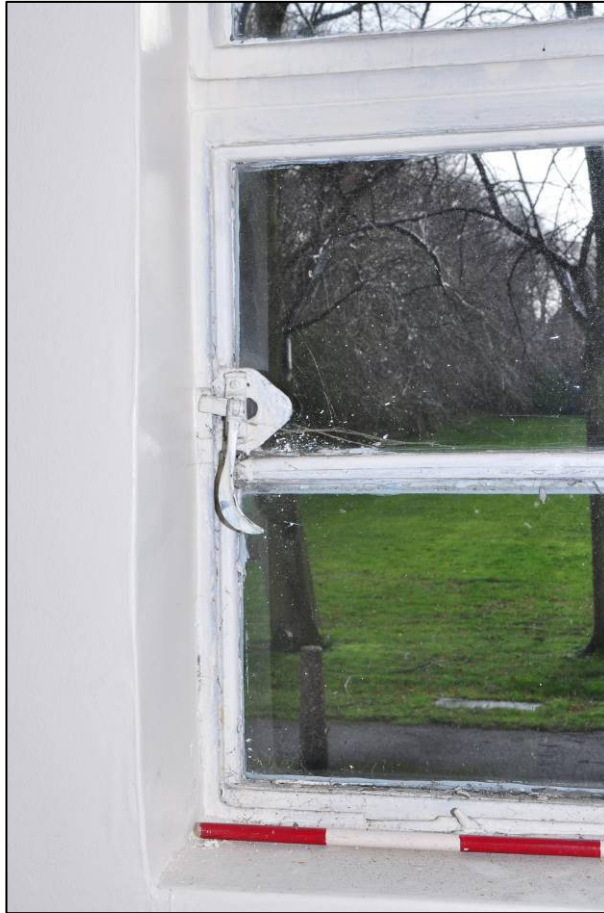
Plate 47: Entrance Block, room G10, window detail, looking S (photo 1/2848).
