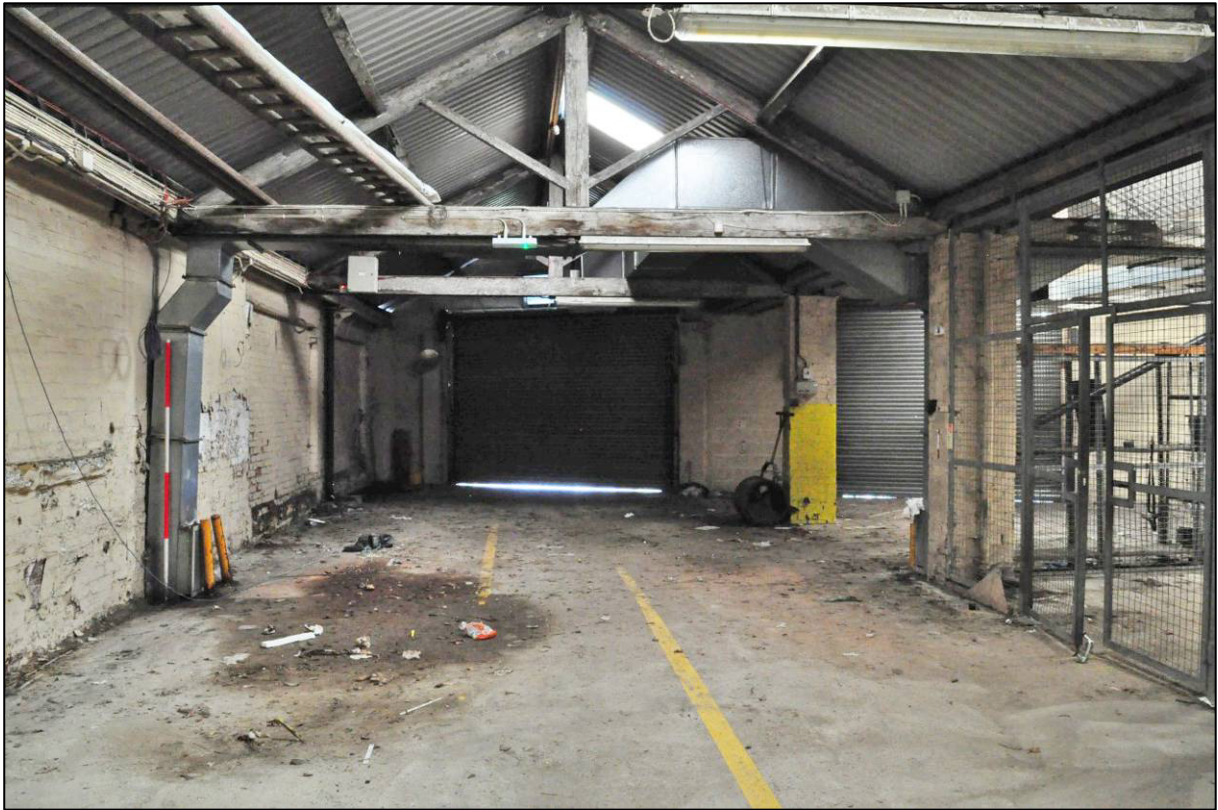
Plate 69: East range, eastern extension, room G22, looking N (photo 1/2885).
