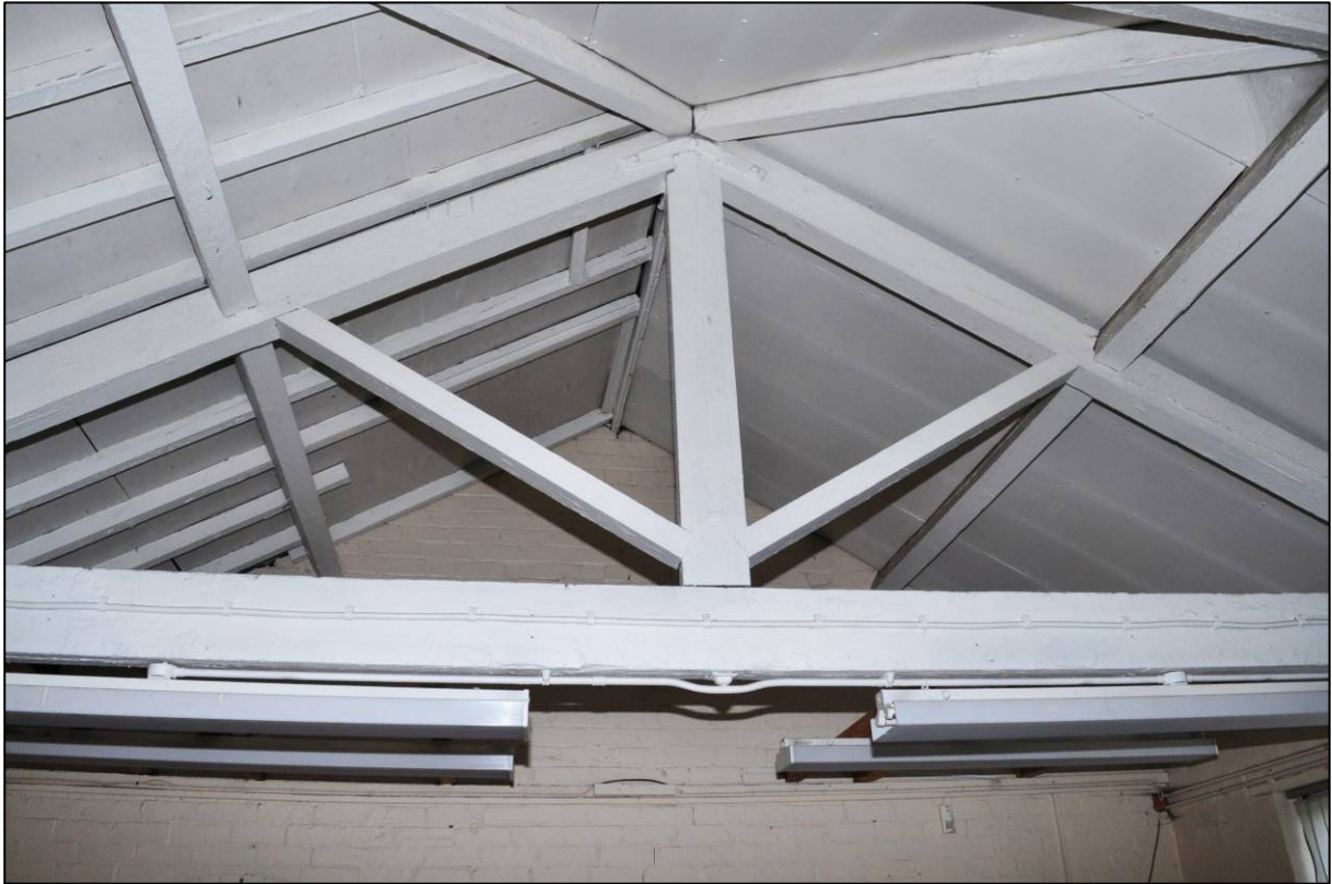
Plate 67: East range, original part, room G21, roof truss, looking S (photo 1/2912).
