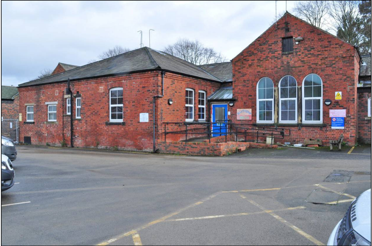
Plate 28: Entrance Block, north elevation, central projection, looking SE (photo 1/2963).
