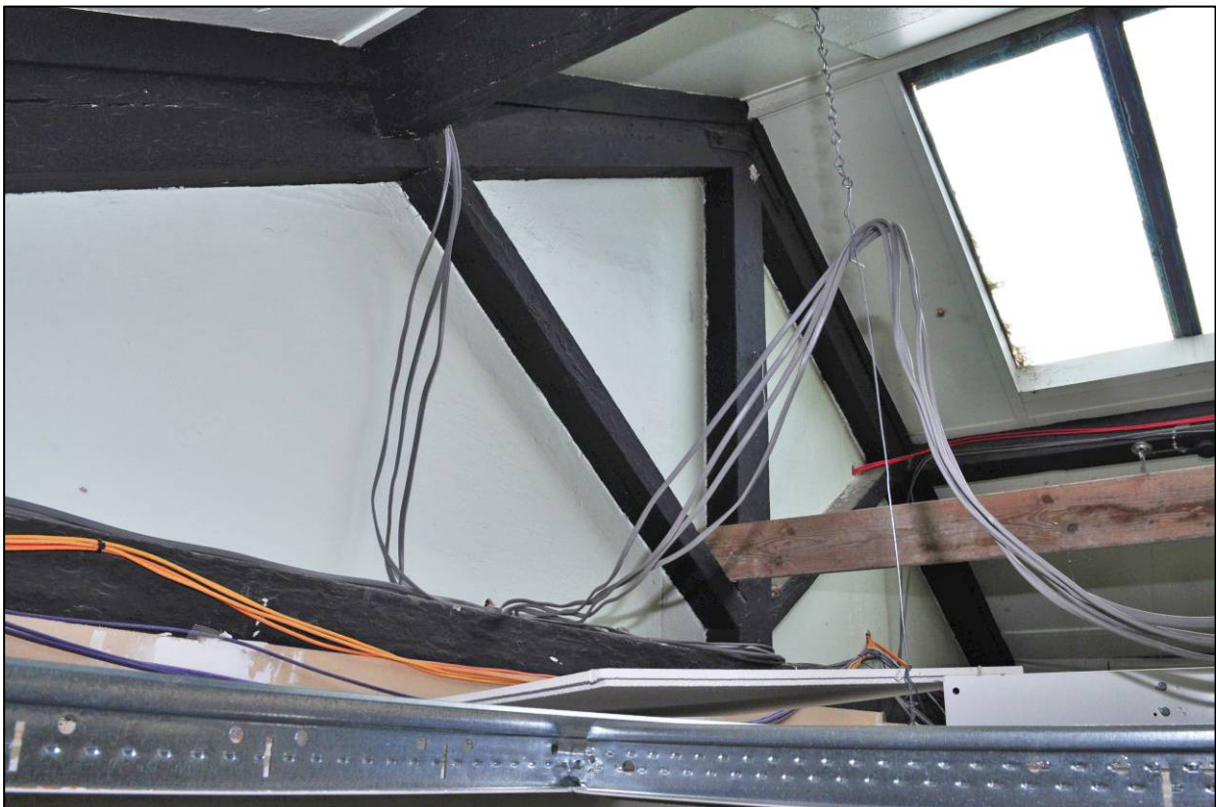
Plate 62: East range, original part, room G19, roof truss, looking SW (photo 1/2907).
