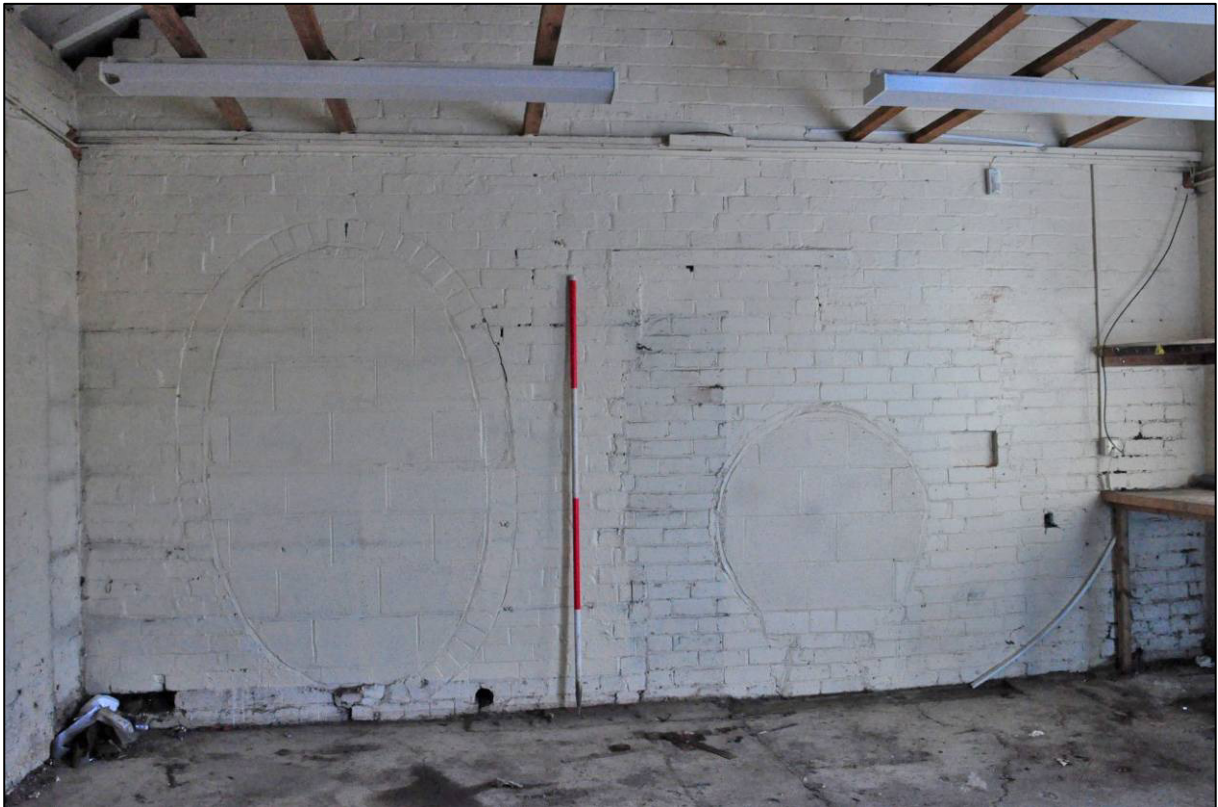
Plate 66: East range, original part, room G21, blocked openings in south wall, looking S (photo 1/2913).
