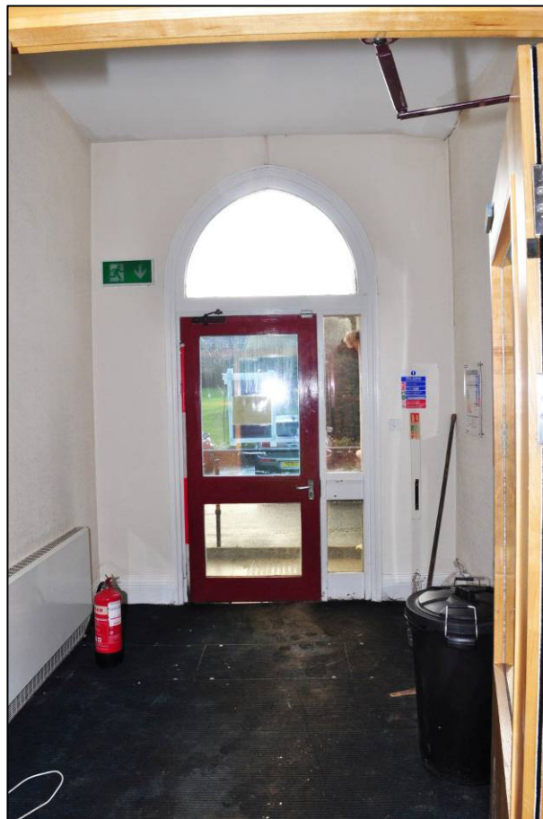
Plate 33: Entrance Block, room G3 (Principal Entrance lobby), looking S (photo 1/2837).
