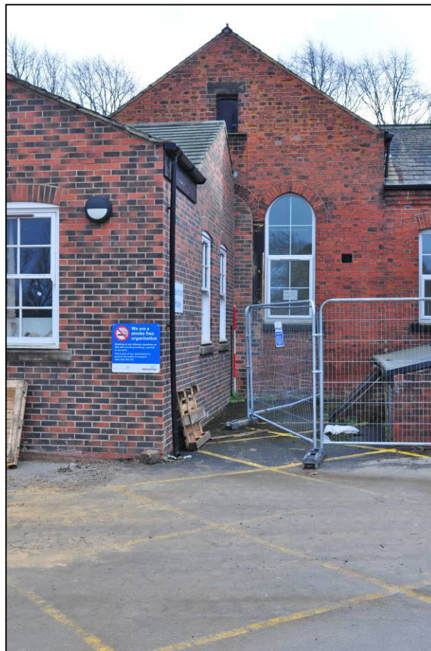
Plate 31: Entrance Block, north elevation, east projection, looking S (photo 1/2971).
