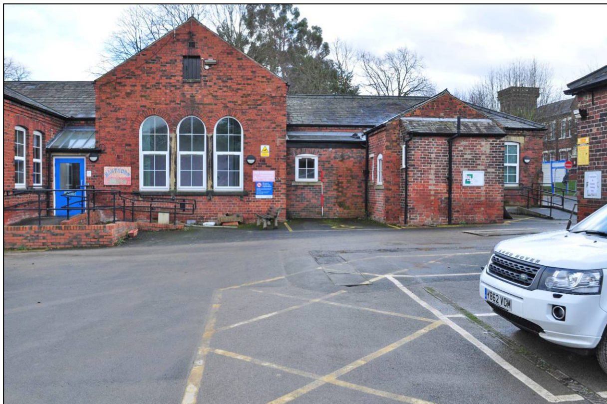
Plate 27: Entrance Block, west end of north elevation, looking S (photo 1/2961).
