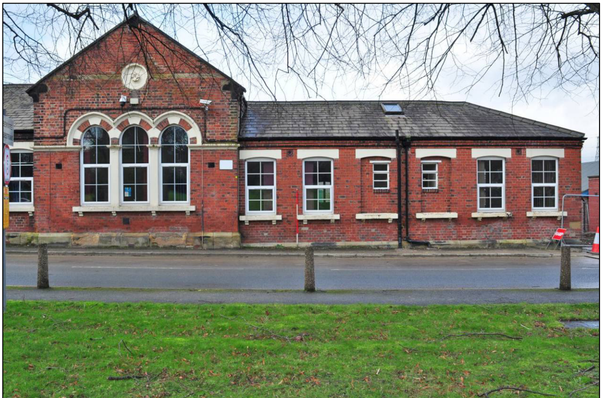
Plate 19: Entrance Block, east end of south elevation, looking N (photo 1/2938).
