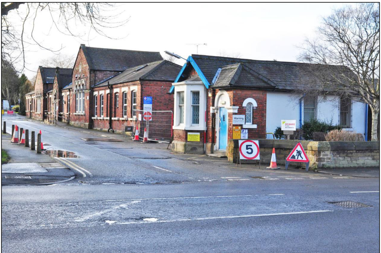
Plate 6: Porter's Lodge and Entrance Block, looking W (photo 1/2924).
