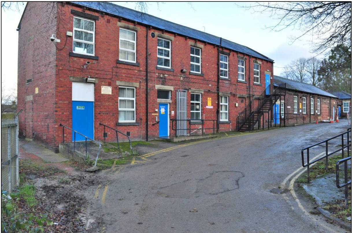
Plate 84: West range, later part, west elevation, looking SE (photo 1/3015).
