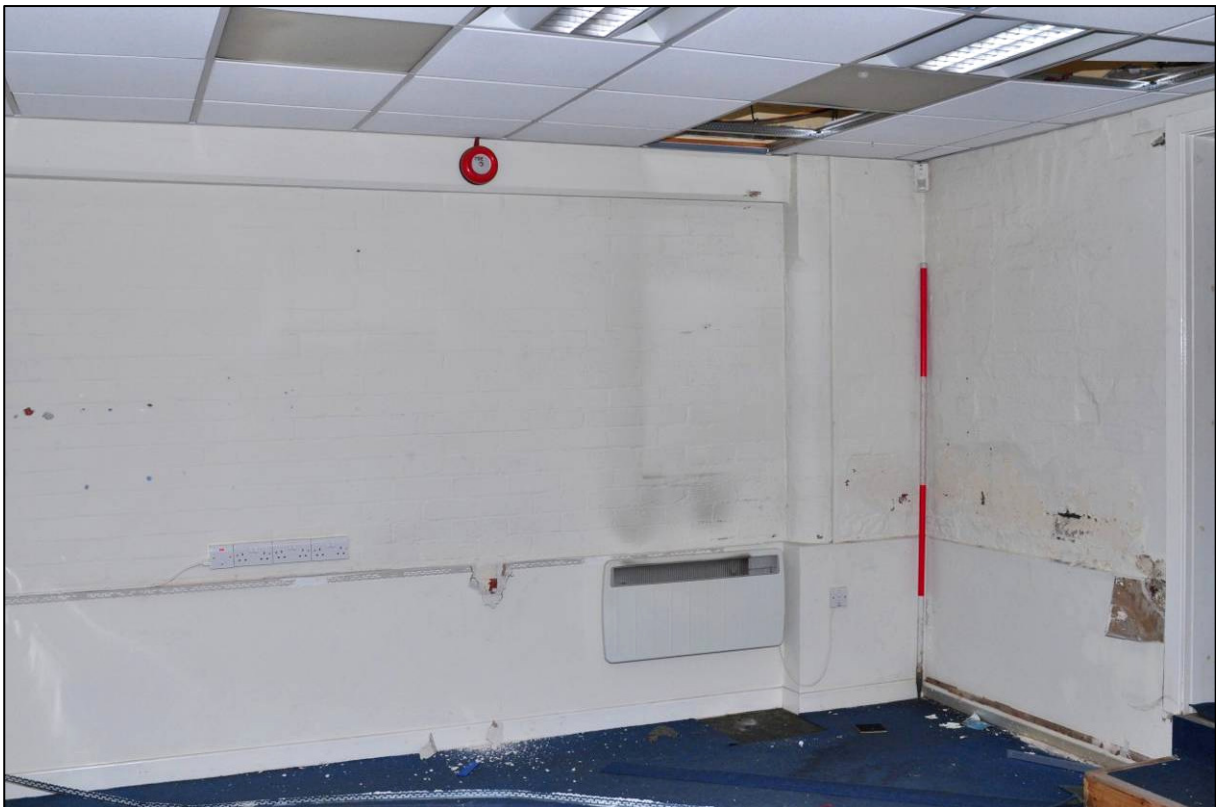
Plate 64: East range, original part, room G20, blocked openings, looking SE (photo 1/2909).
