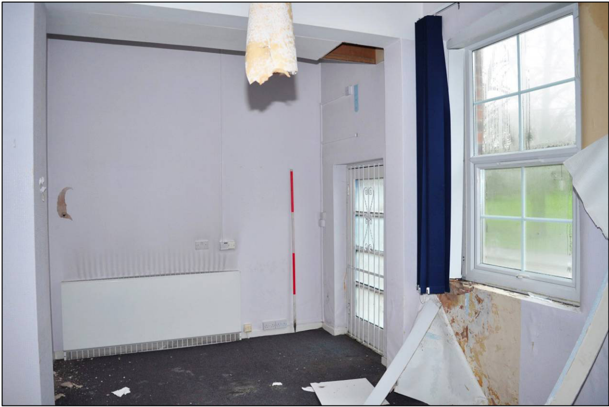
Plate 55: Entrance Block, room G16 (former Male Probationers' Ward), looking SE (photo 1/2868).
