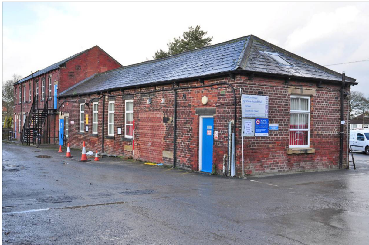
Plate 78: West range, original part, west and south elevations, looking NE (photo 1/3005).
