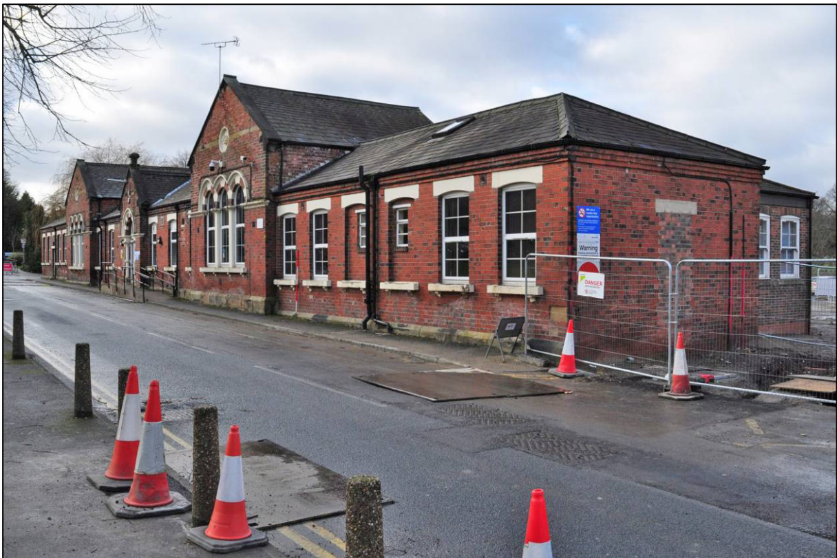
Plate 12: Entrance Block, south elevation, looking NW (photo 1/2934).
