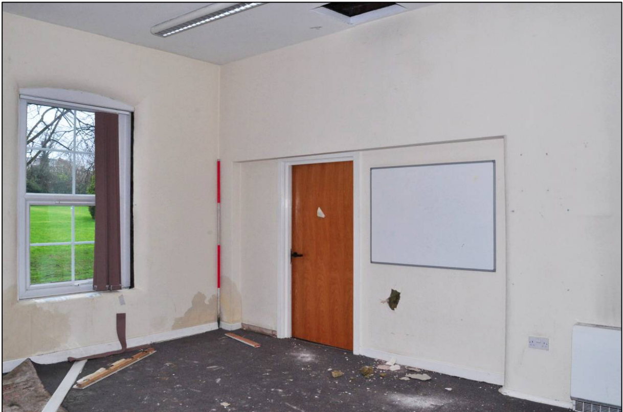
Plate 46: Entrance Block, room G11 (former Male Vagrants' Ward), looking SW (photo 1/2846).
