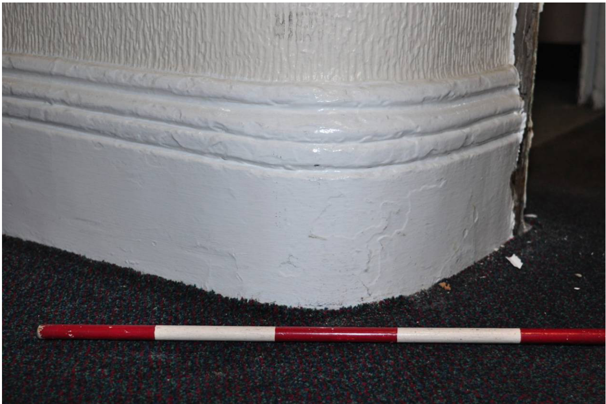
Plate 36: Entrance Block, main corridor G4, skirting detail, looking E (photo 1/2870).
