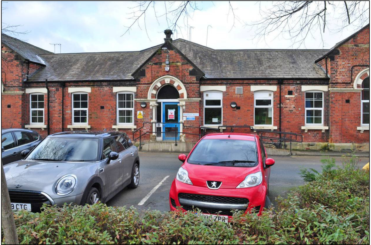
Plate 13: Entrance Block, central part of south elevation, looking N (photo 1/2942).
