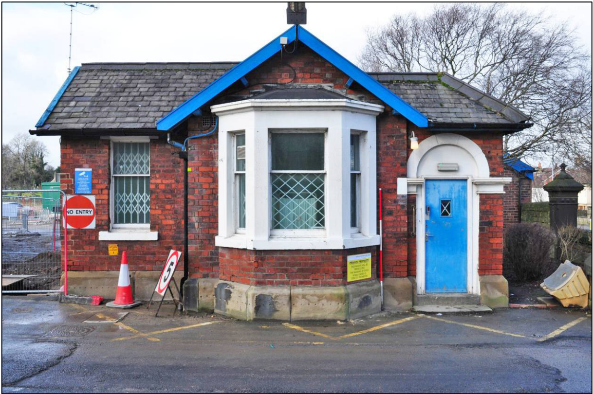
Plate 7: Porter's Lodge, south elevation, looking N (photo 1/2929).
