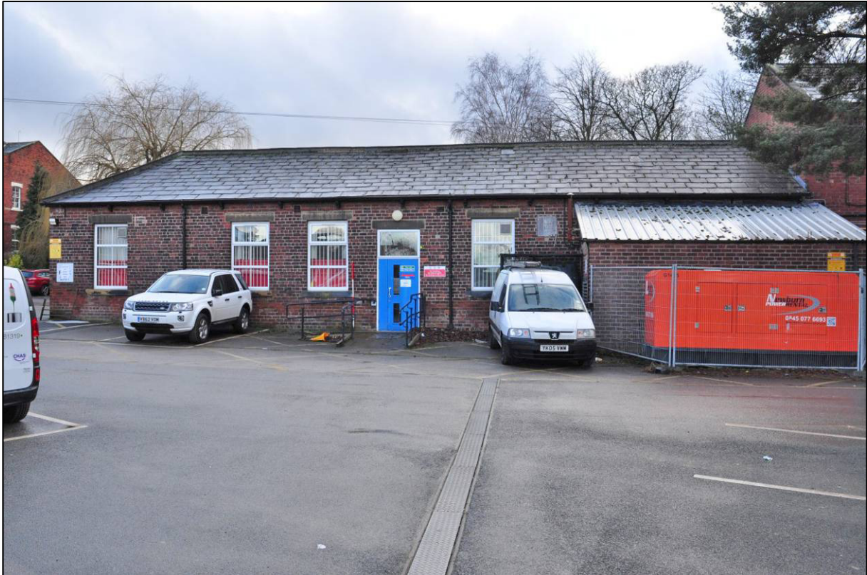
Plate 81: West range, original part, east elevation, looking W (photo 1/3021).
