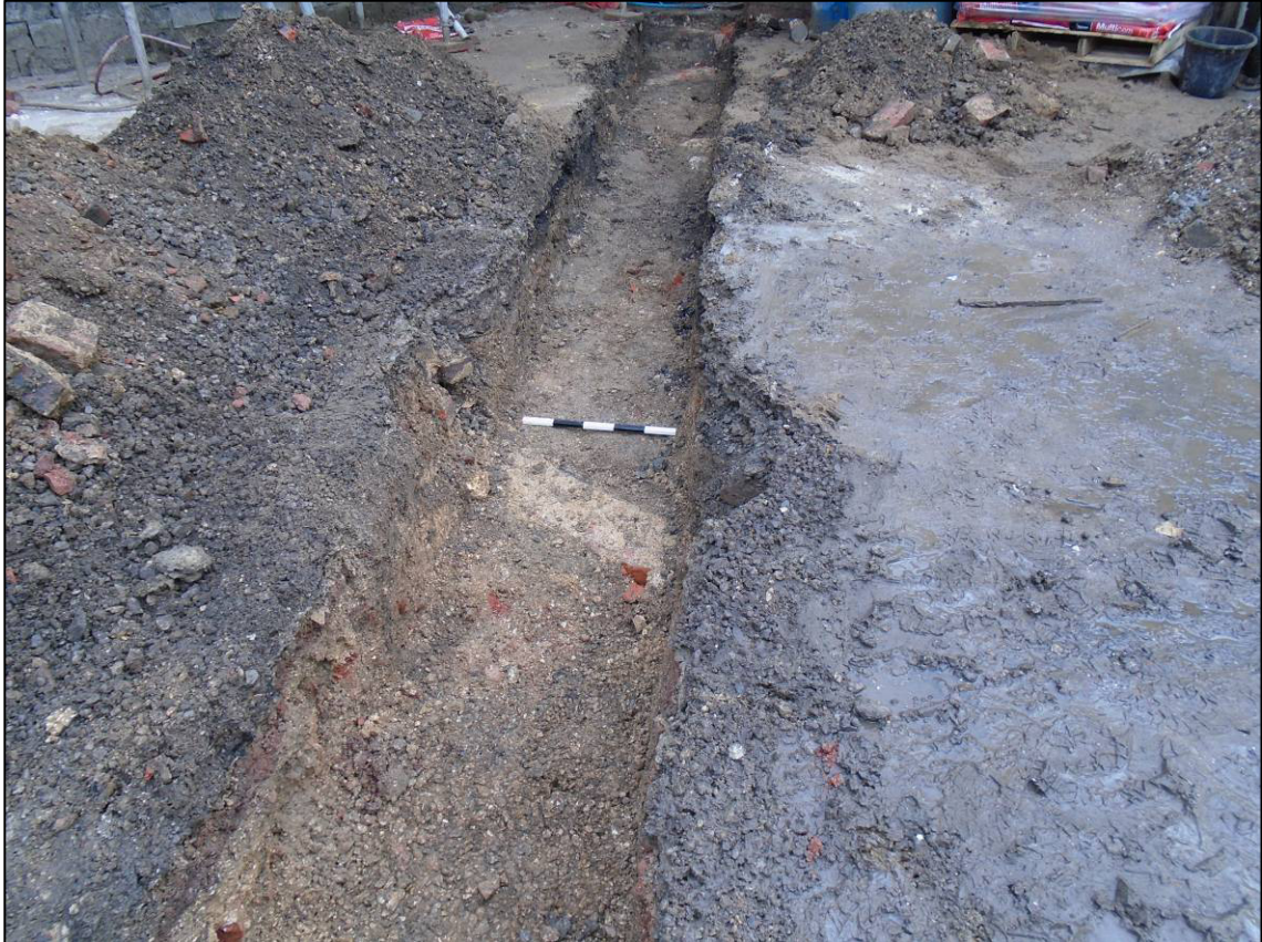
Plate 12: Wall foundation 308 in service trench, looking E.
