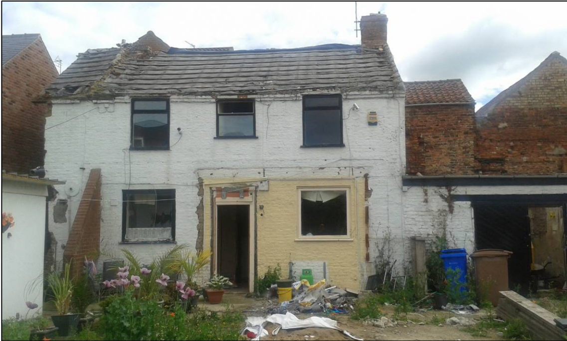
Plate 1: No. 1 Dolman Terrace prior to demolition, looking NE.
