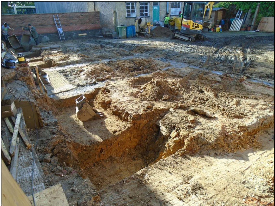
Plate 13: Completed foundations in Plots 1 and 2, looking S.
