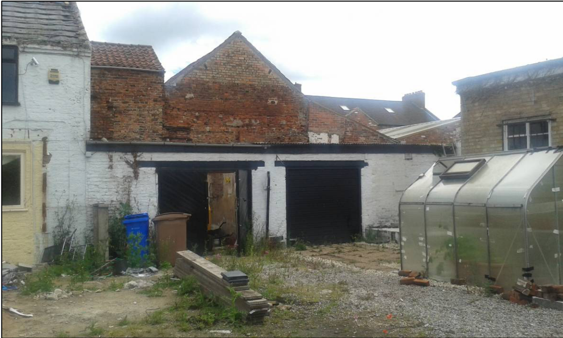
Plate 3: Garages adjacent to No. 1 Dolman Terrace, prior to demolition, looking NE.
