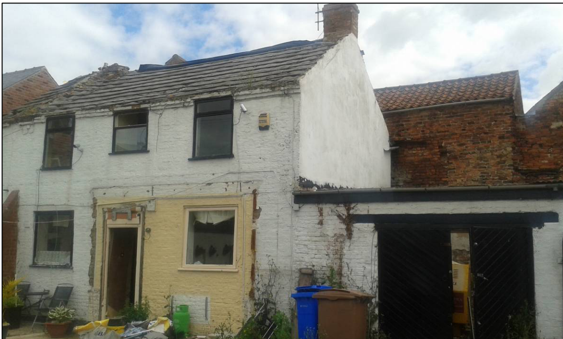
Plate 2: No. 1 Dolman Terrace and adjacent garage, prior to demolition, looking N.
