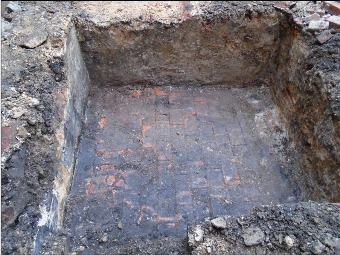
Plate 7: Coal cellar in Plot 1, showing brick floor (102 ) and lime plastered walls (103), looking SE.
